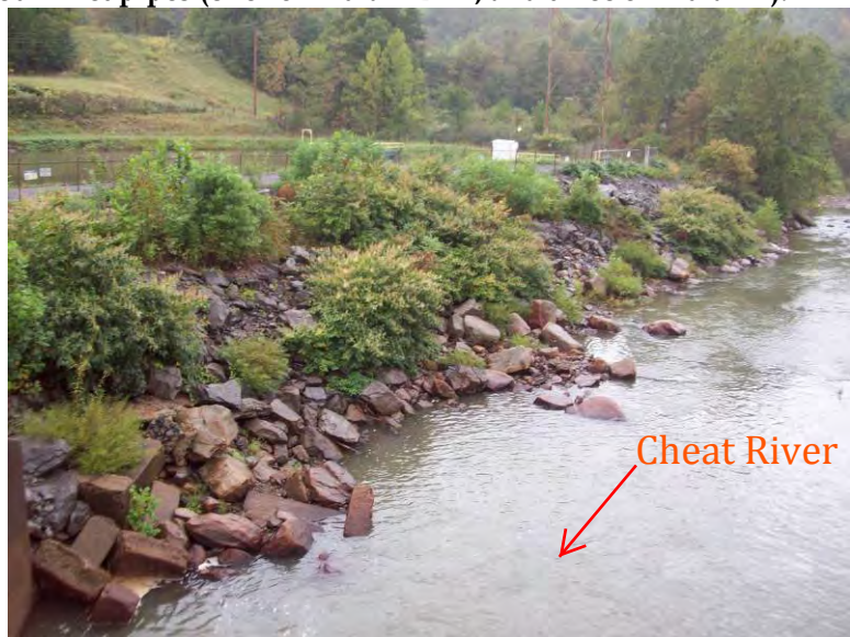
Photo 27: East embankment exterior slope, looking west. Note typical vegetation and riprap.
