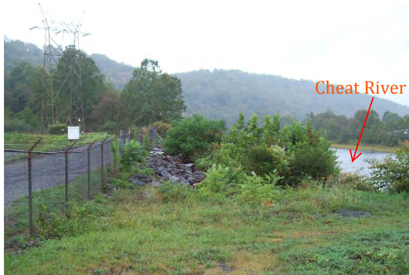
Photo 26: East embankment exterior slope, looking northwest. Note typical vegetation and riprap.
