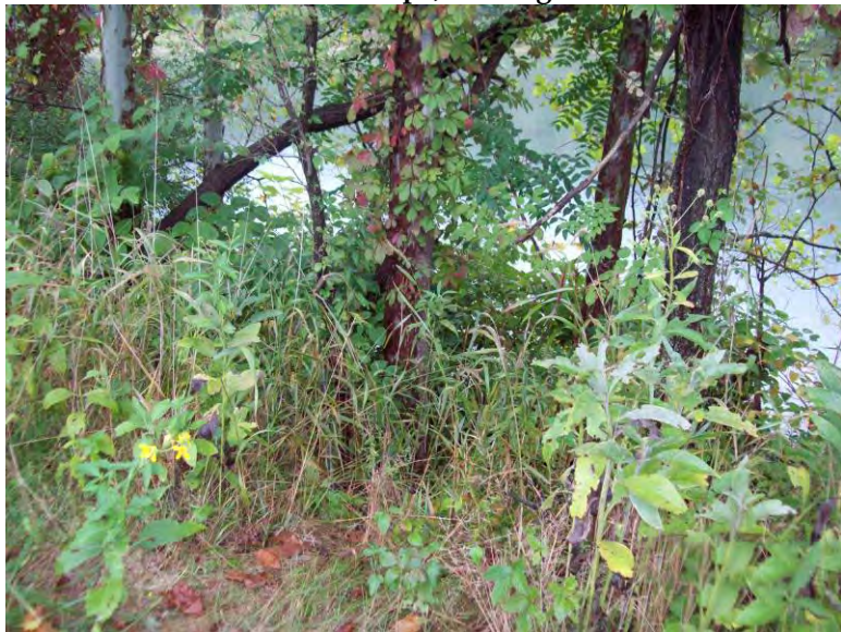
Photo 62: East embankment exterior slope looking northeast. Note typical vegetation and Cheat River in background.
