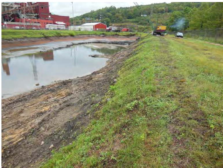
Photo 44: East embankment interior slope, looking north.
