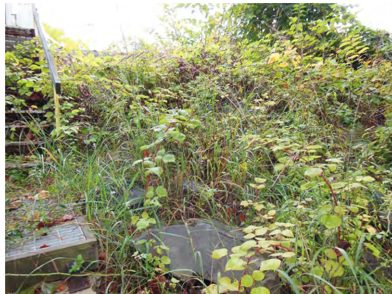
Photo 59: East embankment exterior slope at stairs to outfall, looking northwest. Note typical vegetation.
