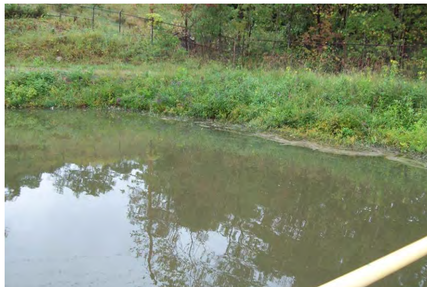
Photo 14: North embankment interior slope, looking west.
