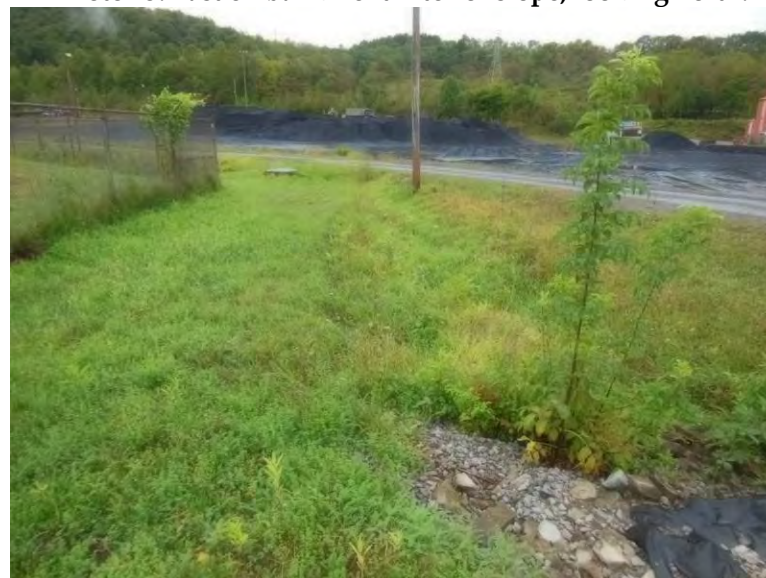
Photo 47: North embankment exterior slope, looking west.
