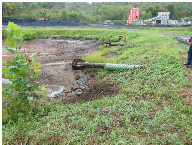
Photo 29: North embankment interior slope, looking west. Note three 8-inch-diameter inlet pipes.
