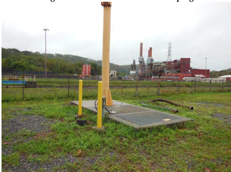
Photo 58: Sump structure near southeast corner, looking northwest.
