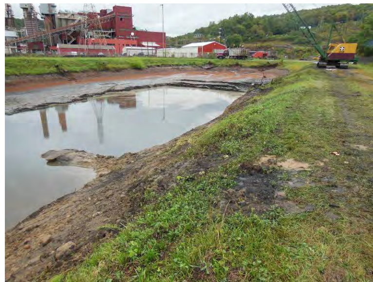
Photo 45: East embankment interior slope, looking north.
