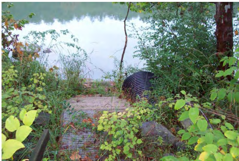
Photo 60: 36-in-dia outfall into Cheat River at east embankment exterior slope, looking east.
