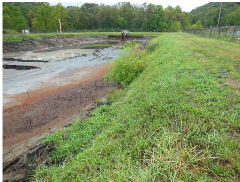
Photo 33: West embankment interior slope, looking south.
