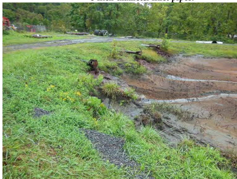
Photo 31: North embankment interior slope, looking east. Note areas of erosion at pipe discharge.
