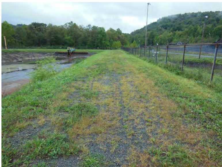
Photo 32: West embankment crest, looking south.
