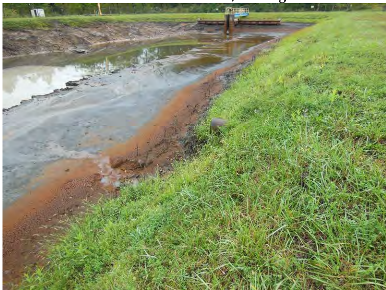
Photo 34: West embankment interior slope, looking south. Note 10-inch-diameter inlet pipe from coal pile runoff.
