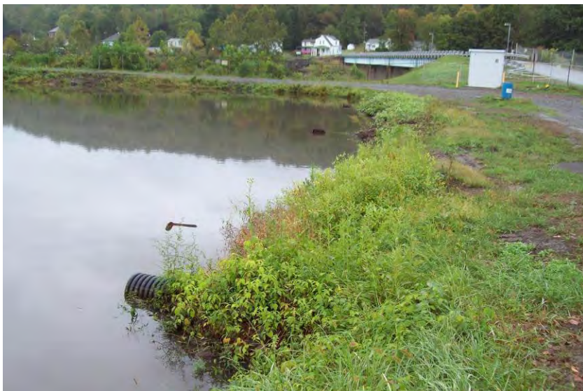
Photo 25: South embankment interior slope, looking northeast. Note four inlet pipes (one 18-in-dia HDPE, and three 8-in-dia DI).
