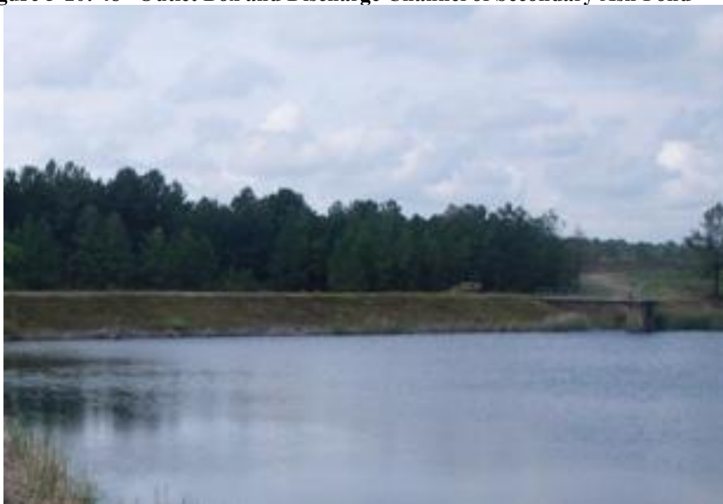
Figure 5-10: 48” Outlet Box and Discharge Channel of Secondary Ash Pond
