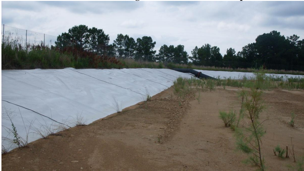
Figure 5-15: Active Bottom Ash Storage Pond Dam – interior slope
