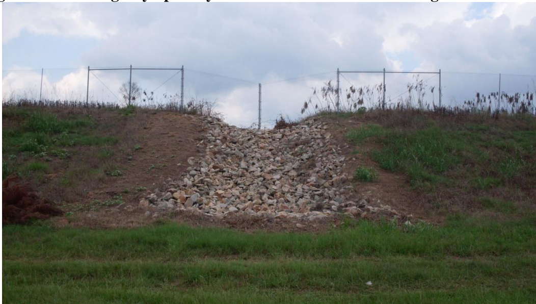
Figure 5-17: Emergency Spillway from Active Bottom Ash Storage Pond
