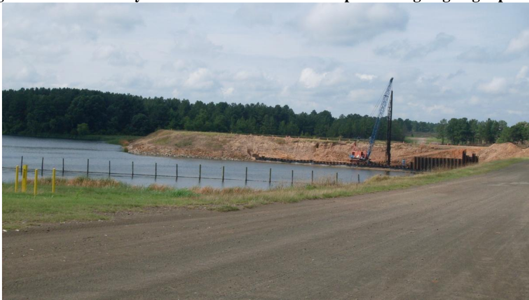
Figure 5-21: Secondary Ash Pond Dam – exterior slope showing ongoing repairs
