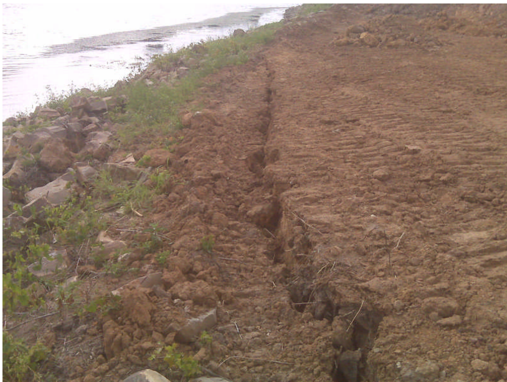
Photo 5 – Second Slip Seen at the Toe
