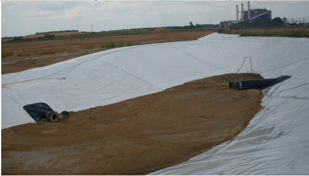
Figure 5-16: 18" Outlet Pipe from Active Bottom Ash Storage Pond
