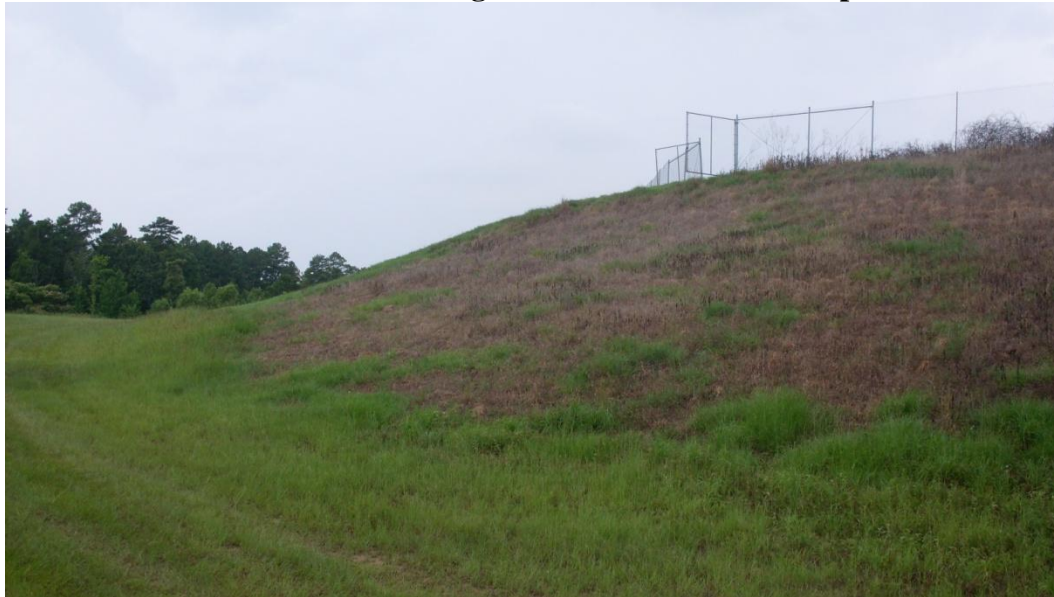
Figure 5-19: Active Bottom Ash Storage Pond Dam – exterior slope
