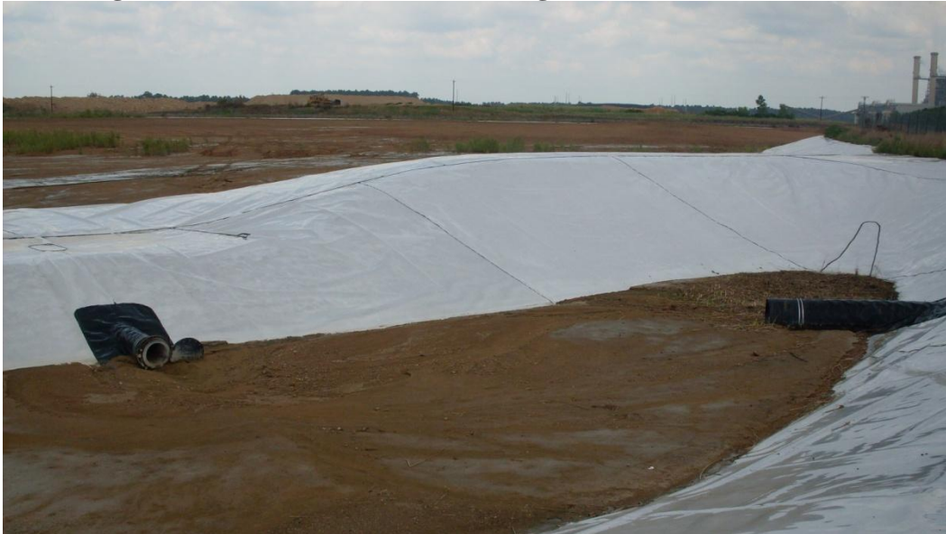
Figure 2-3: Active Bottom Ash Storage Pond Outlet
