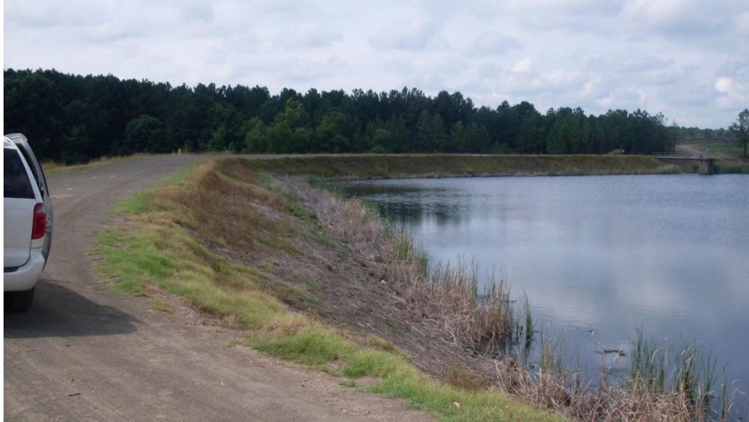
Figure 5-18: Secondary Ash Pond Dam – interior slope opposite the repairs
