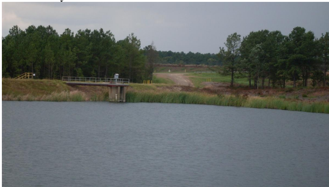
Figure 2-2: Secondary Ash Pond Outlet
