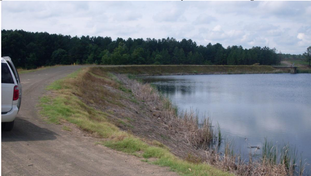
Figure 5-8: Crest around East End of Secondary Ash Pond with gravel access roadway
