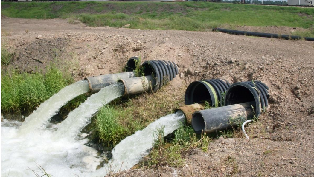
Figure 5-7: Effluent Inlet from Primary Ash Pond
