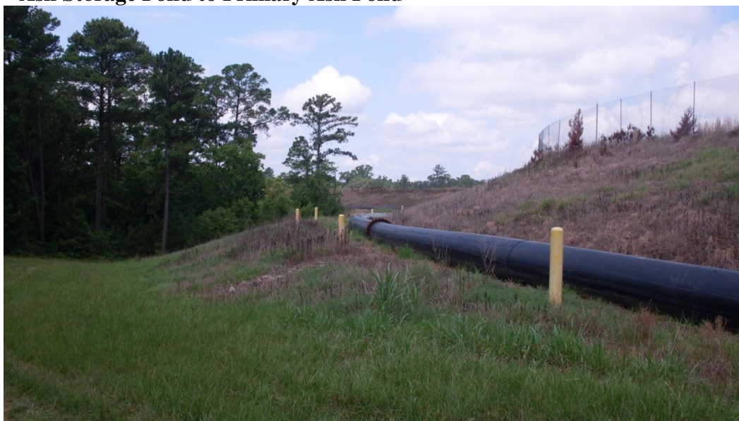
Figure 5-14: 18” HDPE Outlet Pipe Recirculating Supernatant from Active Bottom Ash Storage Pond to Primary Ash Pond
