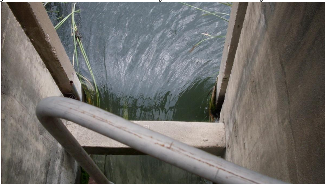
Figure 5-6: Effluent Outlet from Primary Ash Pond to Secondary Ash Pond
