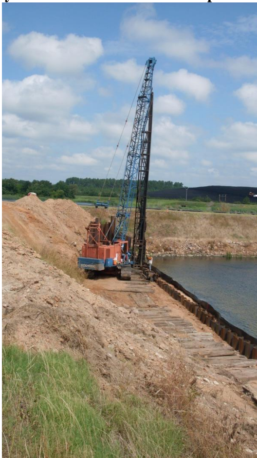
Figure 5-20: Secondary Ash Pond Dam – exterior slope showing ongoing repairs
