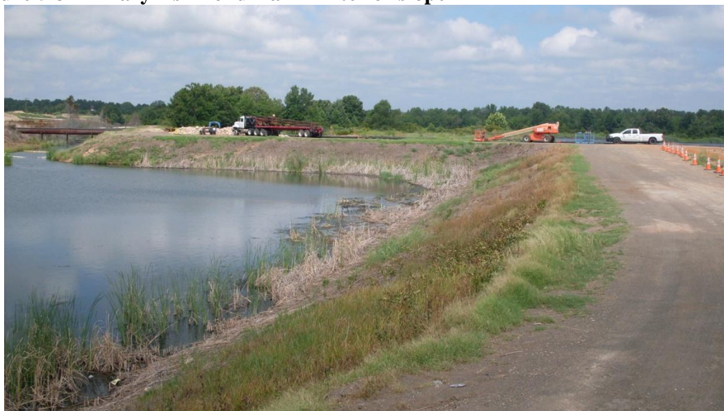
Figure 5-3 Primary Ash Pond Dam – interior slope
