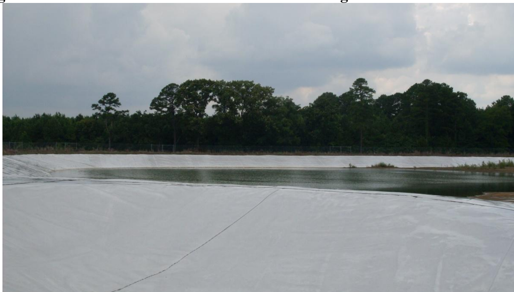
Figure 5-13: Interior Toe of Active Bottom Ash Storage Pond
