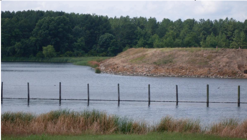
Figure 5-9: Crest and Exterior Toe around East End of Primary Ash Pond
