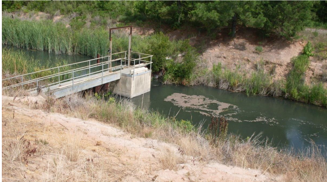
Figure 2-1: Primary Ash Pond Outlet
