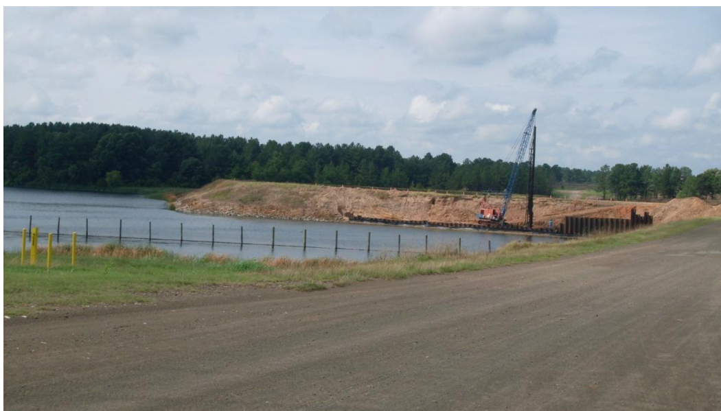
Figure 5-1: Crest around East End of Primary Ash Pond with gravel access roadway
