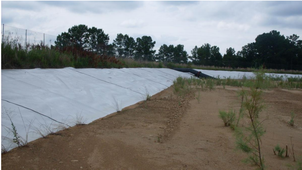
Figure 5-22: Dredge Inlet from Primary Ash Pond into Active Bottom Ash Storage Pond
