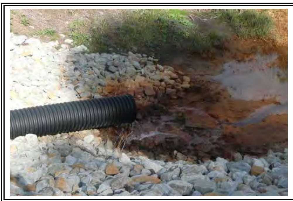
Active blanket drain outlet at No-Name Creek Dam. No Iron precipitate.
