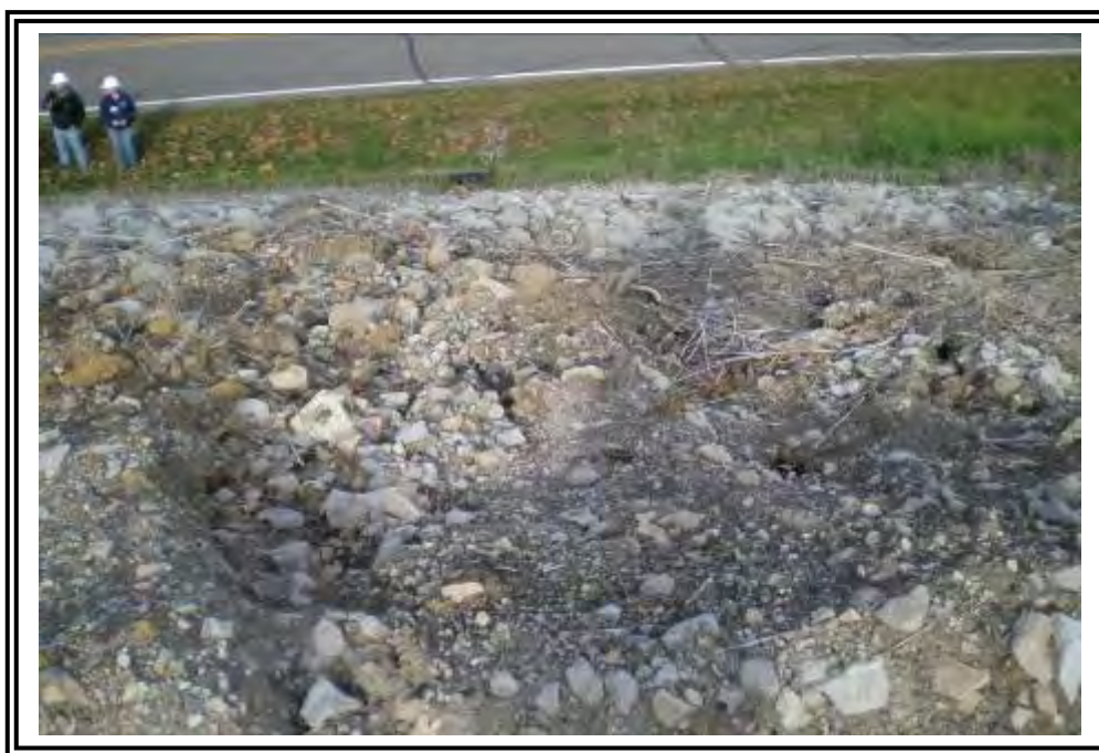
Erosion on the downstream slope of the Lower Fly Ash Dam near the crest elevation above the rip rap slope protection.
