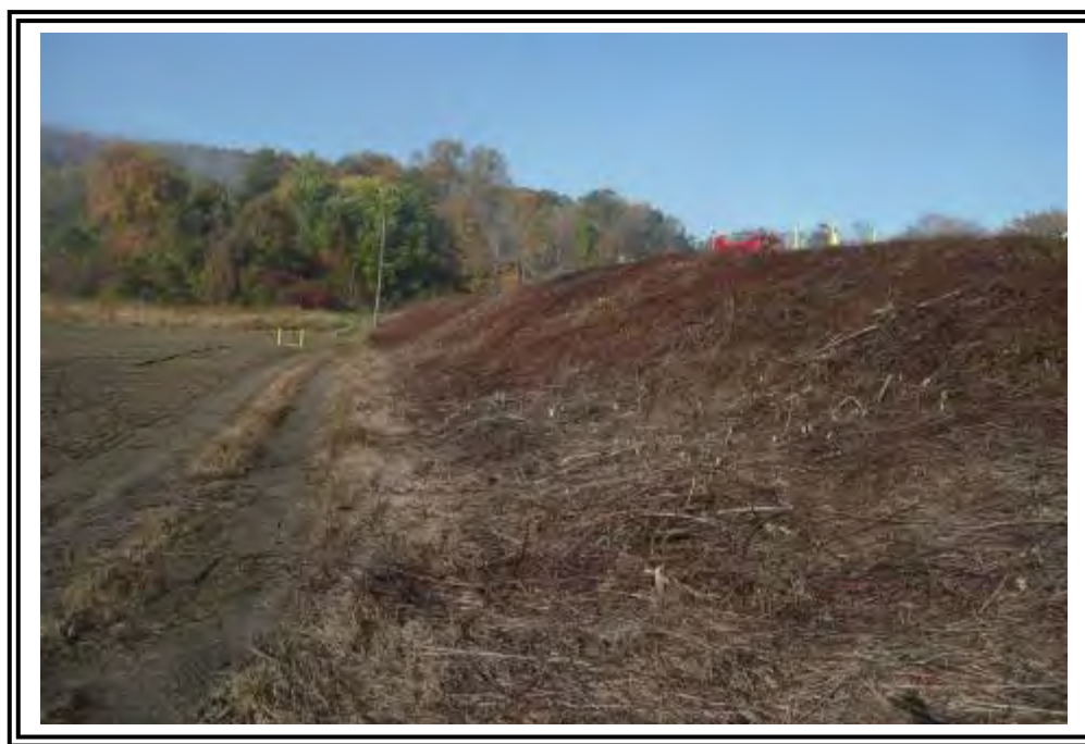
Units 1-4 Bottom Ash Pond south dike exterior slope, looking west from the southeast corner adjacent to the Muskingum River. Note recently cut heavy vegetation and woody brush.
