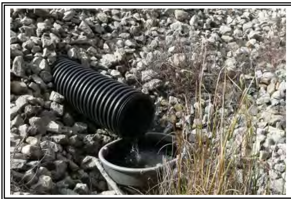
Active blanket drain outlet at Wing Dam. Note absence of iron precipitate.
