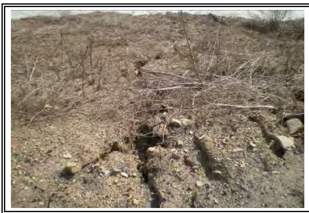
Erosion rills in upstream slope of the Middle Fly Ash Dam.
