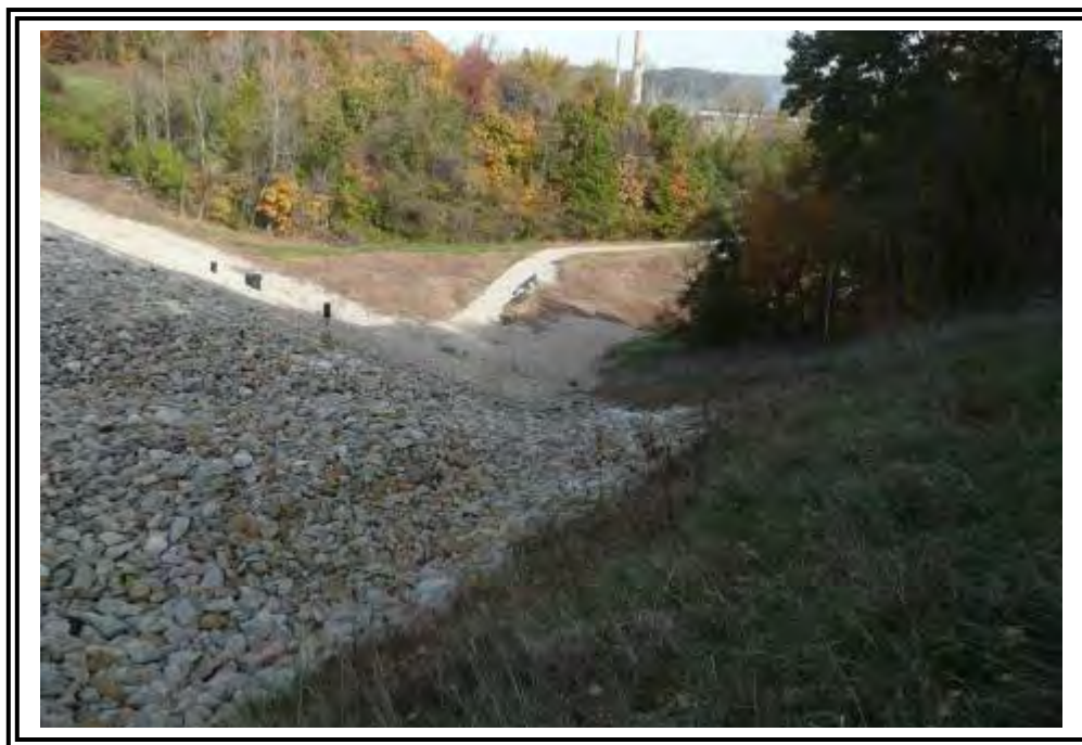
Looking downstream at Mill Stone Creek Dam right (southeast) abutment groin contact.
