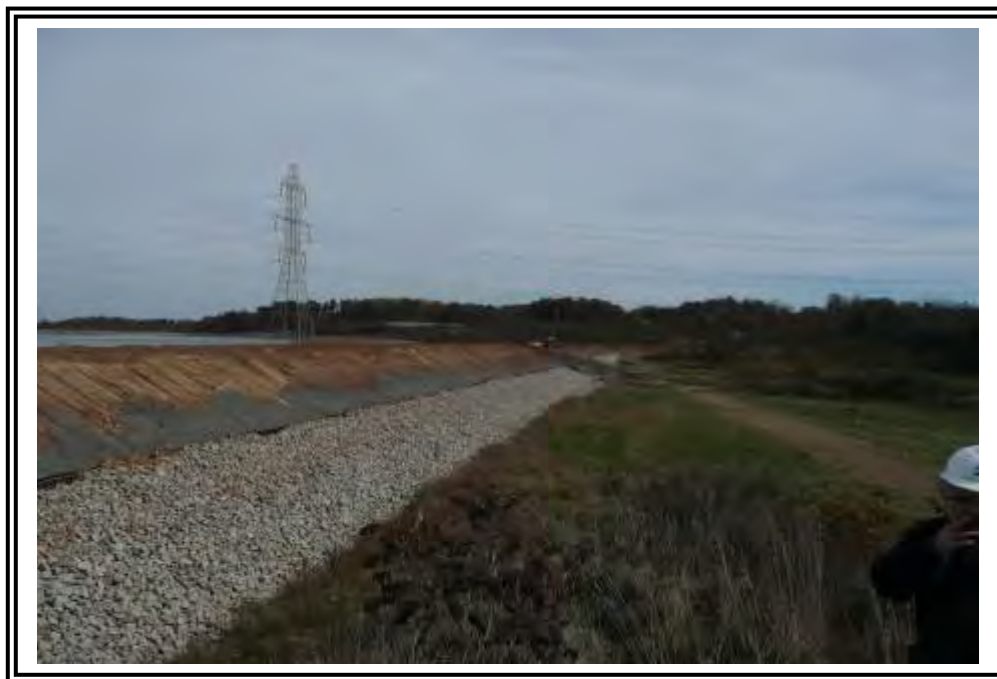
Downstream slope of the Freeboard Dam, looking east. Note zoned construction with ash and clay.
