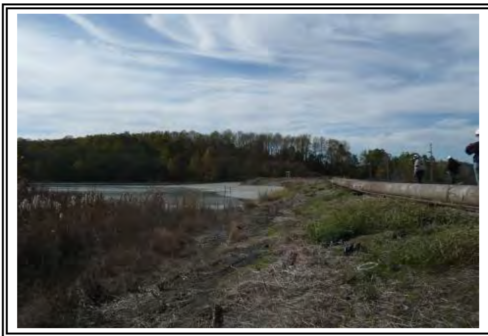
Lower Fly Ash Dam, upstream slope, looking northwest. Note dying weedy vegetation and old sluice lines at crest.
