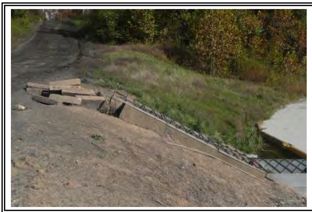
Upstream slope and inclined spillway of the Middle Fly Ash Dam, looking east. Note concrete stop logs at top of slope.
