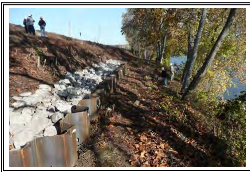
Units 1-4 Bottom Ash Pond east dike sheet pile stream bank stabilization at dike toe, looking north. Note leaning trees.
