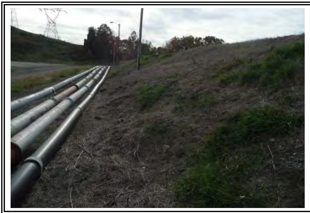
Lower Fly Ash Dam along southeast facing portion of the downstream slope adjacent to Unit 5 bottom ash sluice lines at the toe of the slope, looking southwest. Note slope undulations resulting from previous grading and dormant surficial sloughing.
