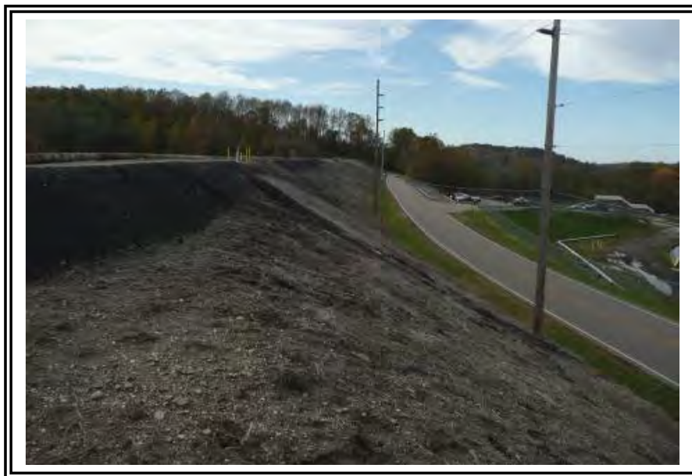
Lower Fly Ash Dam along downstream slope near crest, looking northwest. Note bottom ash material at crest elevation.
