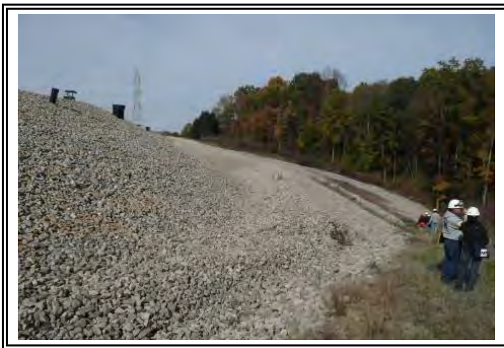
Downstream slope and abutment groin of the Wing Dam at right (southeast) abutment contact, looking northwest. Note blanket drain system inspection, access, and cleanout ports in the slope.
