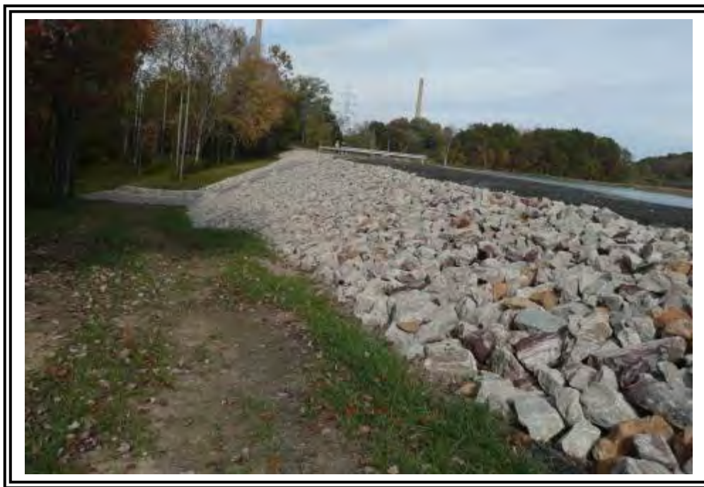
Downstream slope of emergency spillway embankment for the Middle Fly Ash Dam, looking northeast.
