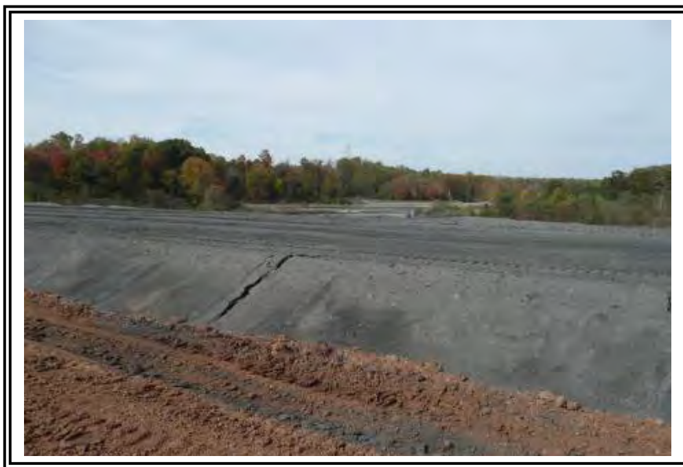
Erosion rill in exposed compacted ash being placed on the Wing Dam. Note Middle Fly Ash Reservoir in the distance.
