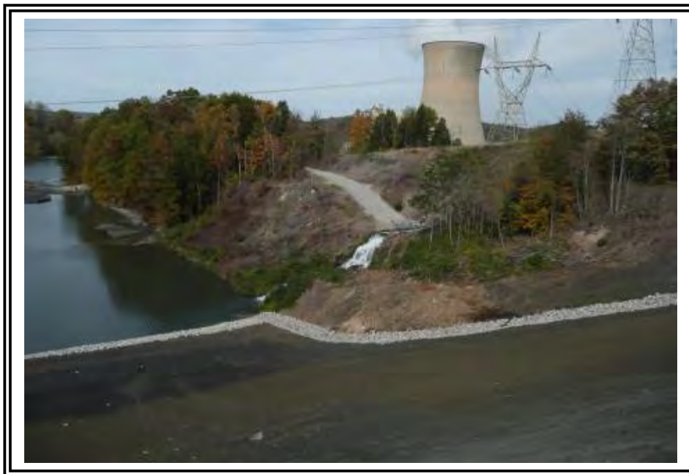
Looking downstream from the Middle Fly Ash Dam. Note effluent above right (east) abutment.
