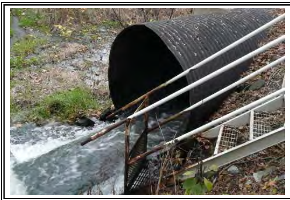
Lower Fly Ash Dam 72-inch diameter CMP spillway outlet.
