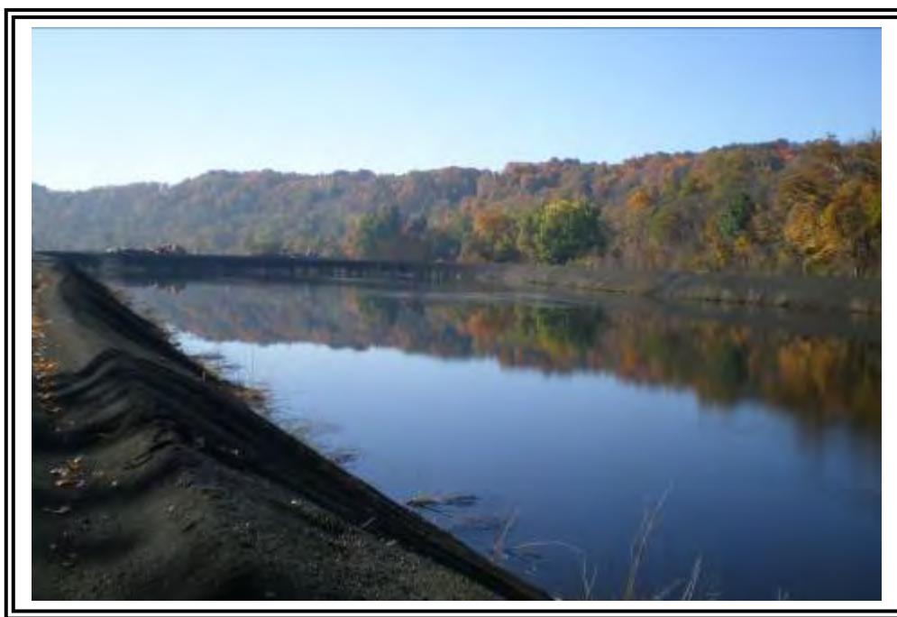
Units 1-4 Bottom Ash Pond east dike interior slope and open pond area, looking south. Note relatively steep slopes and sparse to absent vegetation.
