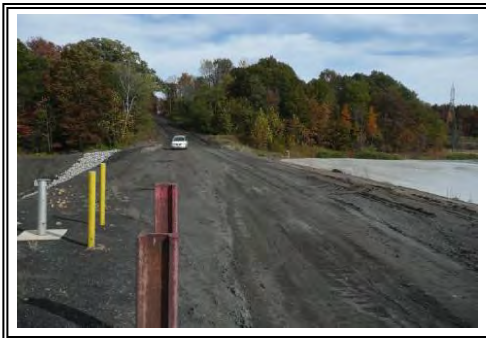
Crest of the Middle Fly Ash Dam, looking east. Note groundwater monitoring well.
