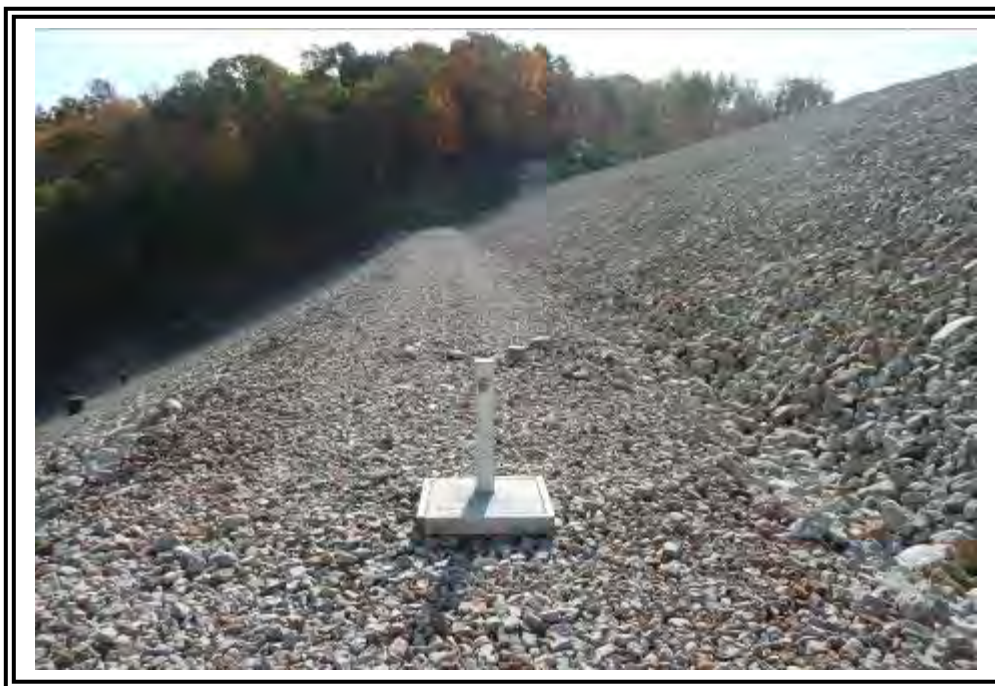
Instrumentation on bench of downstream slope of Mill Stone Creek Dam.
