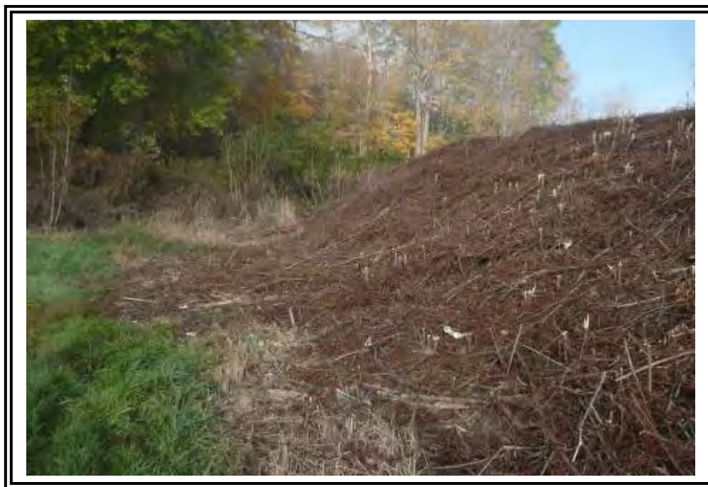
Units 1-4 Bottom Ash Pond south dike exterior slope, looking west. Note recently cut heavy vegetation and woody brush.
