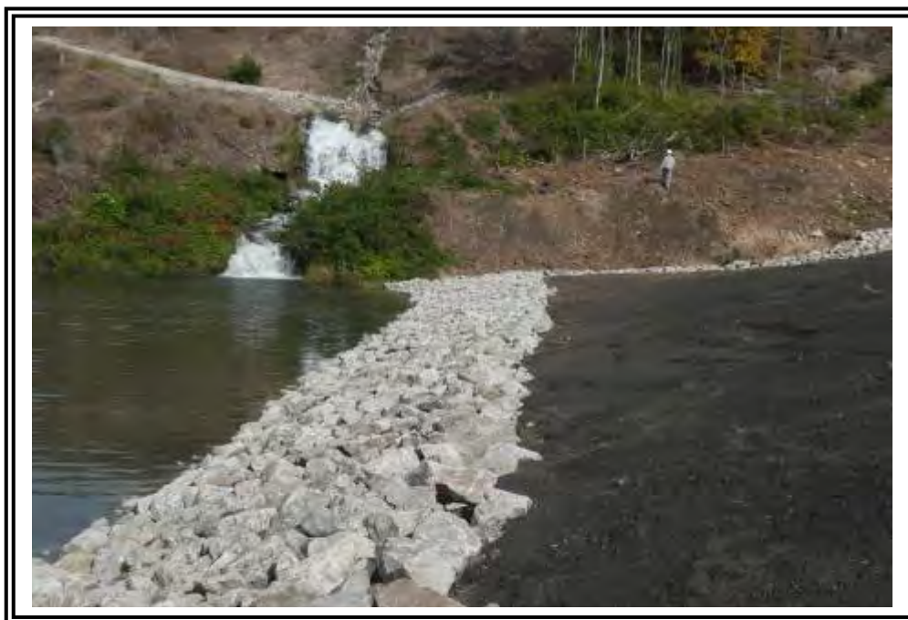
Looking east along rock toe drain and rip-rap slope protection of the Middle Fly Ash Dam.
