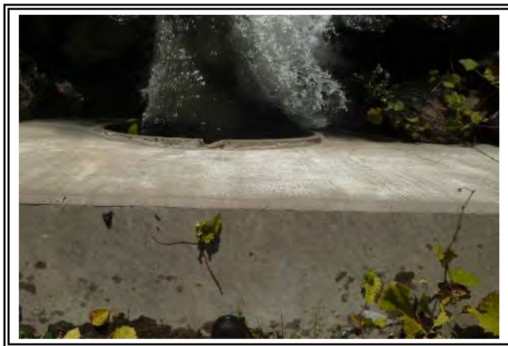
Units 1-4 Bottom Ash Pond outlet and headwall.
