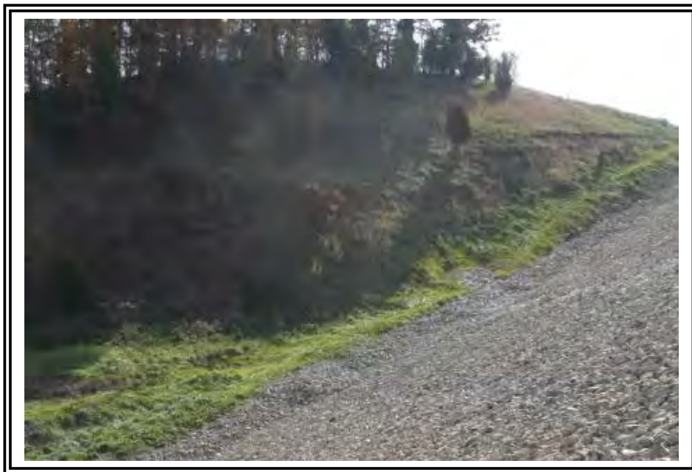
Slope at right (southeast) abutment contact where extension from groin was constructed to intercept hillside seepage, looking southeast.
