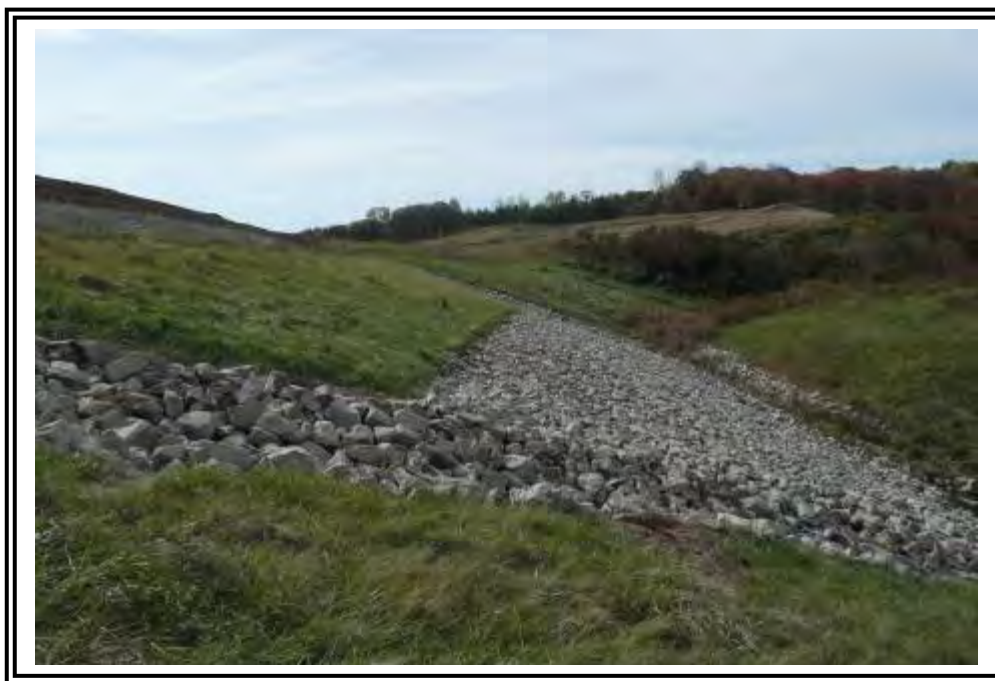
Downstream slope of the Spillway Dam showing upper grass covered slope and rip-rap protection on the lower portion of the slope, looking west.
