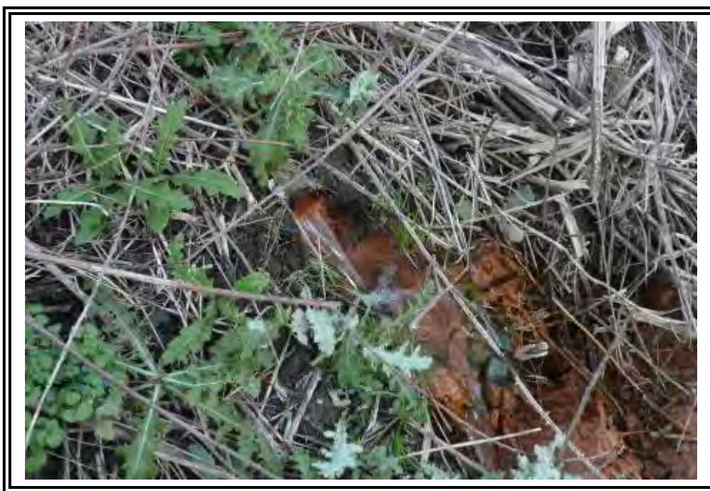
Lower Fly Ash Dam, active underdrain/toe drain outlet. Note iron precipitate.
