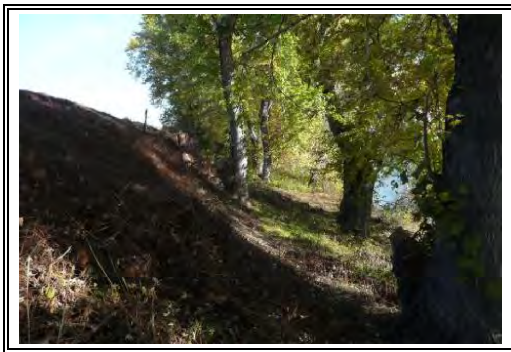
Units 1-4 Bottom Ash Pond east dike toe, looking north. Note large trees at the toe and between the dike and river bank.
