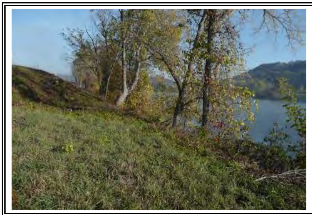
Units 1-4 Bottom Ash Pond east dike exterior slope along the Muskingum River, looking north (or upstream with respect to the river flow). Note relatively large trees at the river bank leaning towards the river.
