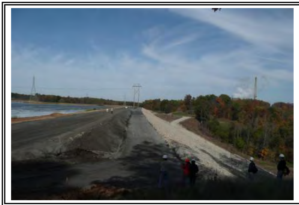
Crest and downstream fly ash construction bench of the Mill Stone Creek Dam, looking northwest.
