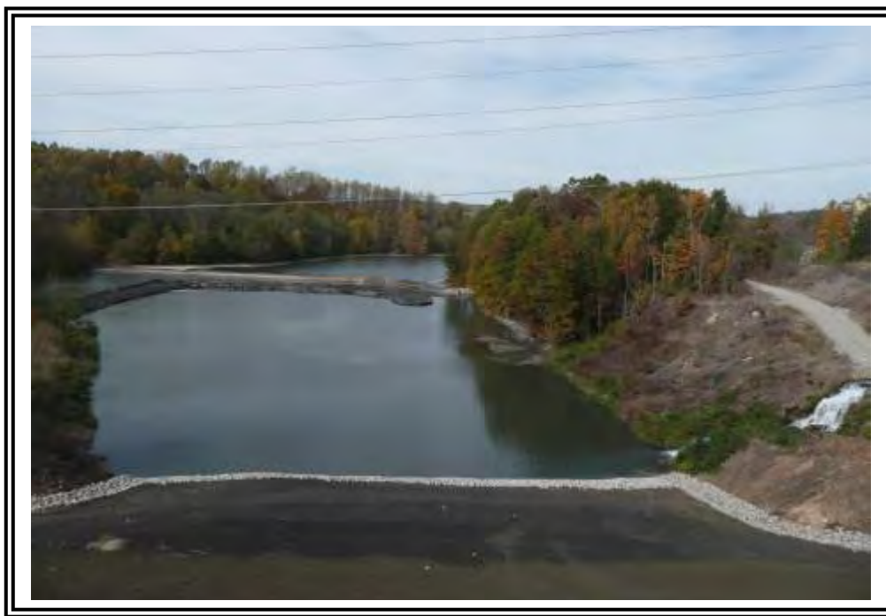
Looking downstream from the Middle Fly Ash Dam. Note ash slope construction and rip-rap toe protection.
