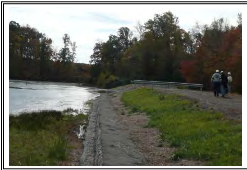
Looking southwest along upstream slope of the gabion emergency spillway.
