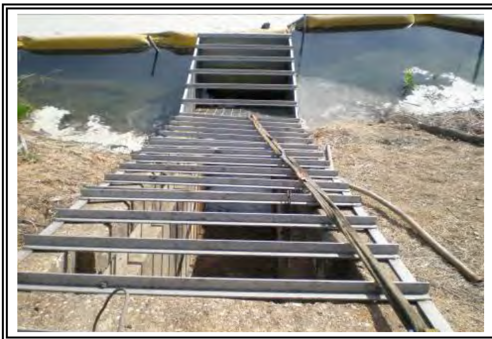
Looking down into the inclined spillway inlet of the Middle Fly Ash Dam.
