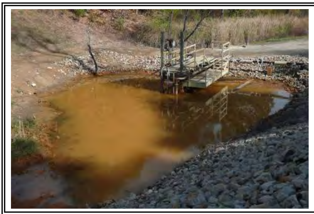
Seepage collection, treatment, and recirculation basin at No-Name Creek Dam.
