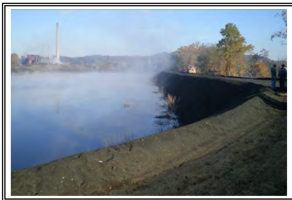
Units 1-4 Bottom Ash Pond east dike interior slope, looking east. Note relatively steep slope.
