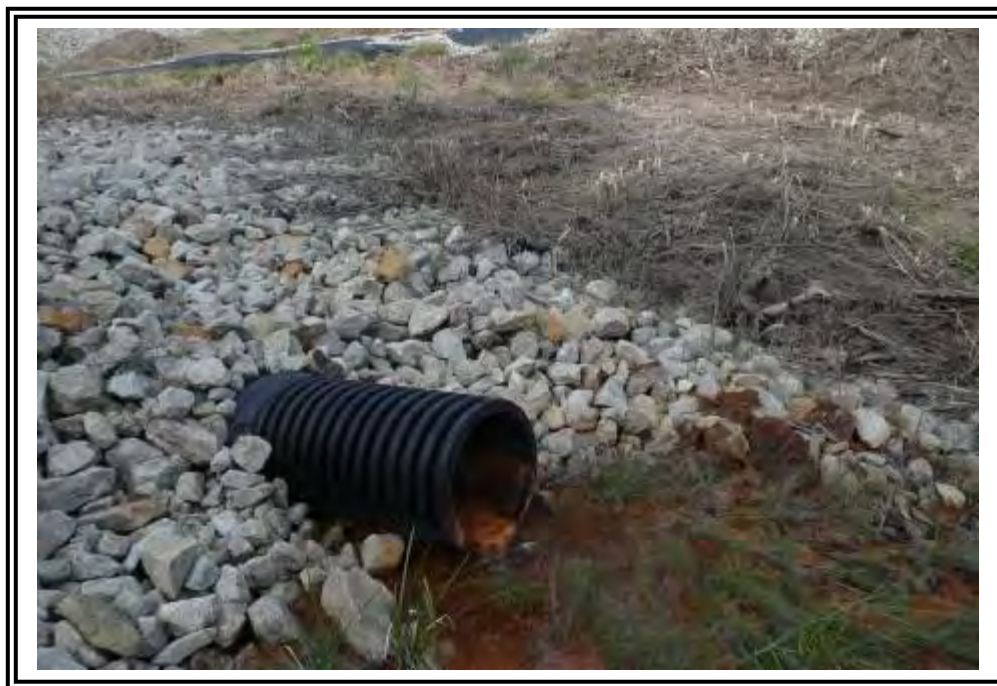
Active blanket drain outlet at Mill Stone Creek Dam. Note iron precipitate.
