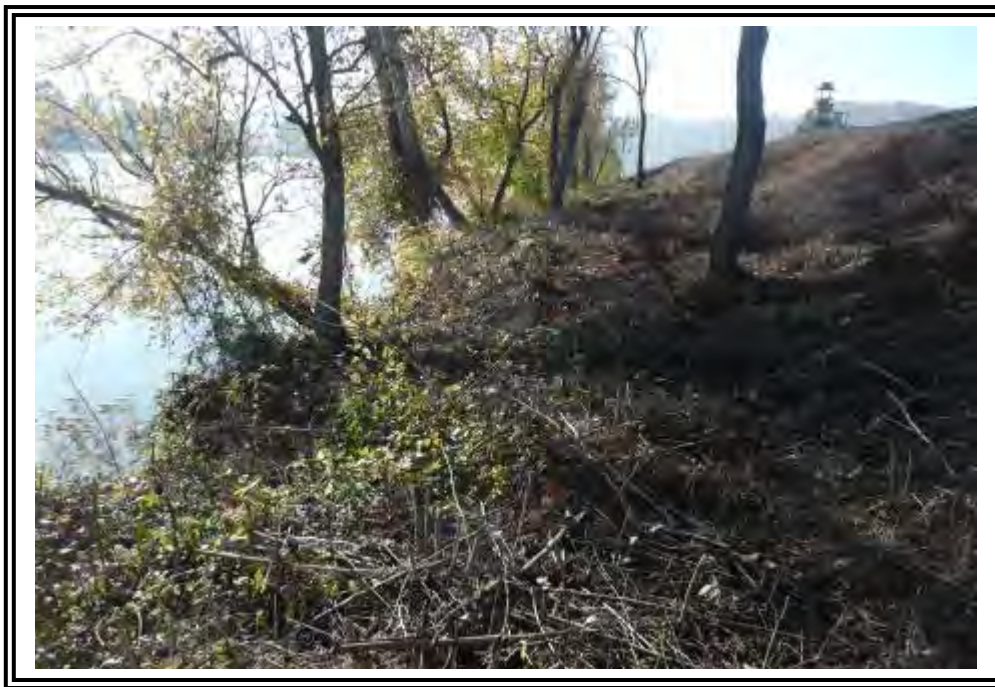
Units 1-4 Bottom Ash Pond east dike exterior slope, looking south. Note distance between river bank and dike toe.
