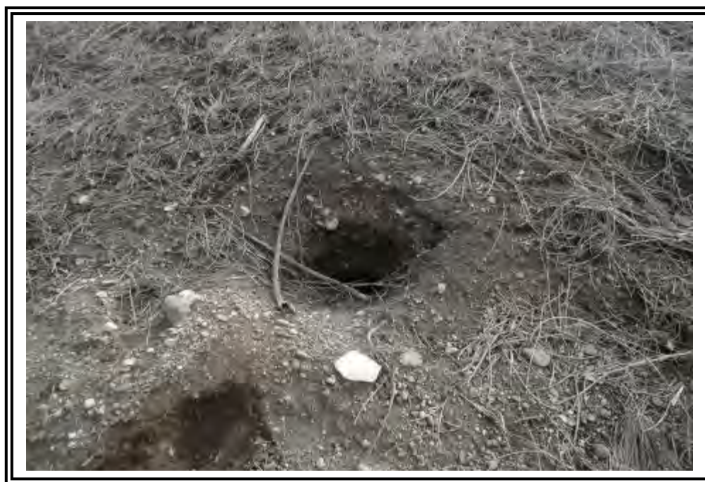
Lower Fly Ash Dam partially collapsed rodent burrow in downstream slope. Note silty sand and gravel material in embankment surface.
