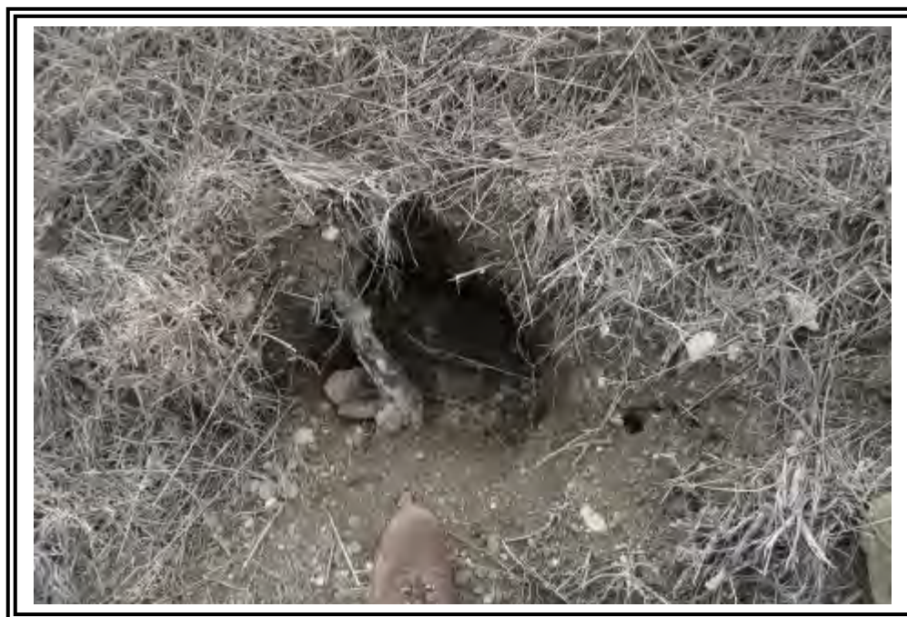
Rodent burrow on the Lower Fly Ash Dam, southeast facing downstream slope.
