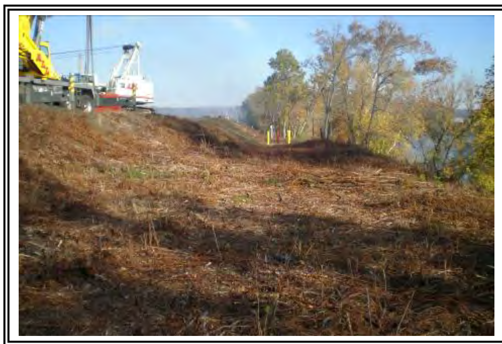
Units 1-4 Bottom Ash Pond east dike bench area and upper exterior slope. Bench is on the order of 15 to 20 feet wide in this area with evidence recently mowed dormant vegetation.
