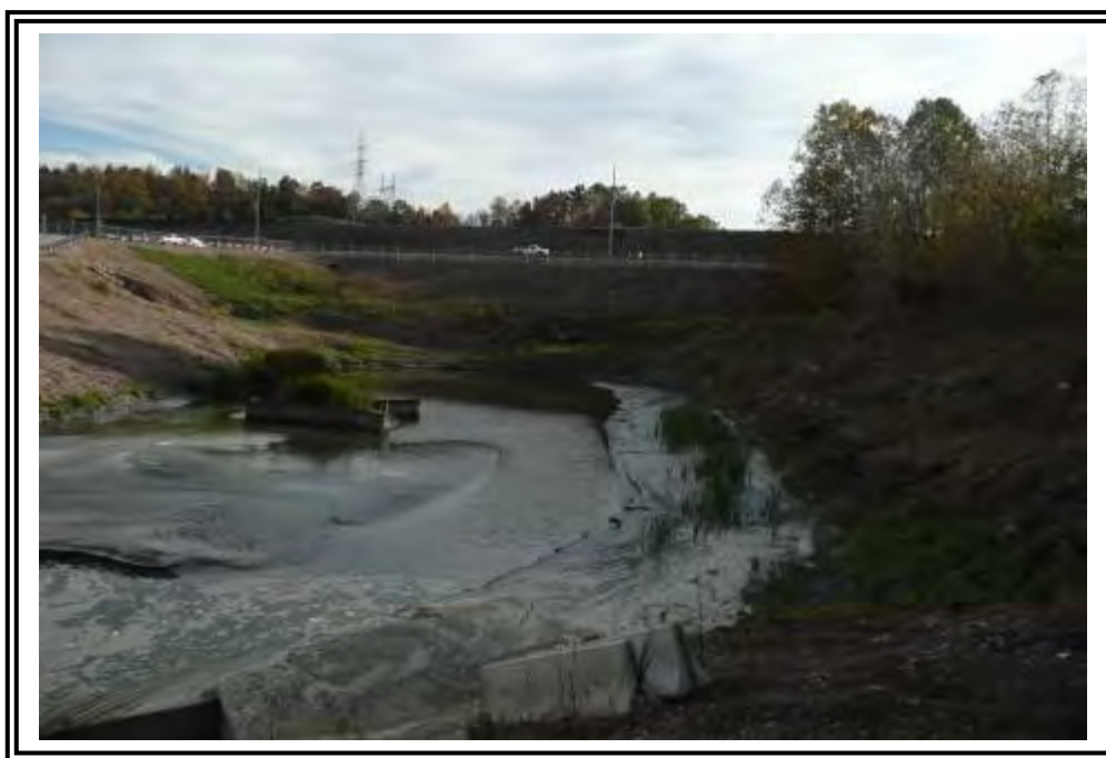
Partially incised wastewater, runoff, and seepage collection basin at toe of the Lower Fly Ash Dam.
