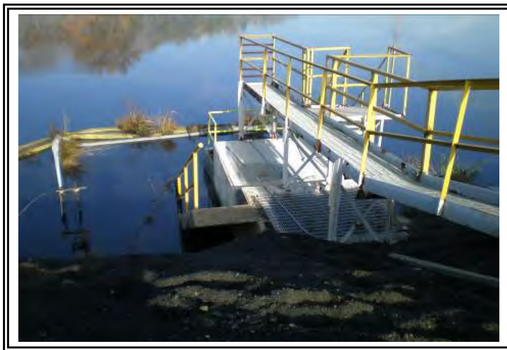
Outfall structure in the south dike of the Units 1-4 Bottom Ash Pond.
