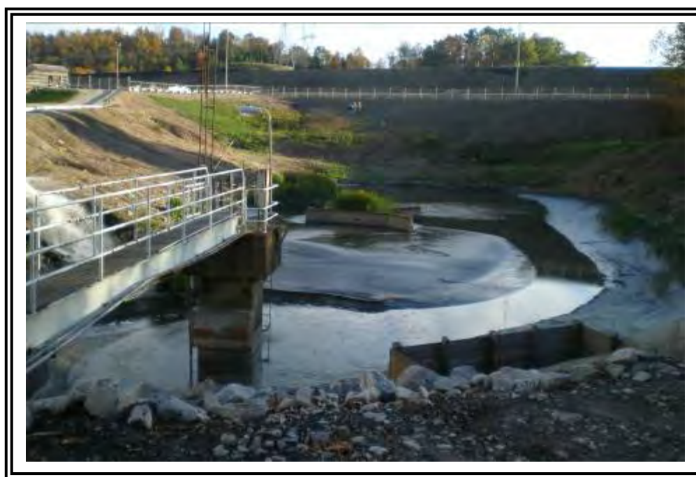
Looking south across the facility water and drainage catch basin at the toe of the Lower Fly Ash Dam. Water entering basin is circulated into the Lower Fly Ash Reservoir.
