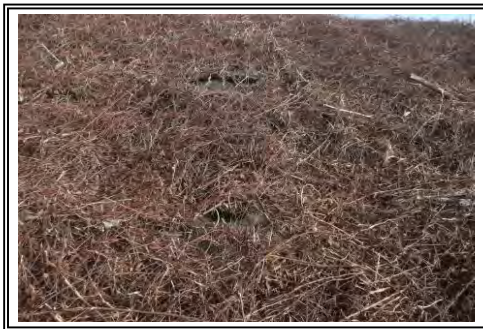
Rodent burrow on the Units 1-4 Bottom Ash Pond south dike exterior slope.
