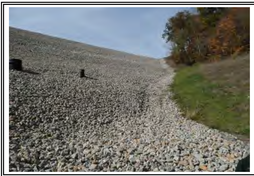
Downstream slope and left (northwest) abutment groin contact of the No-Name Creek Dam. Note blanket drain system inspection, access and cleanout ports.
