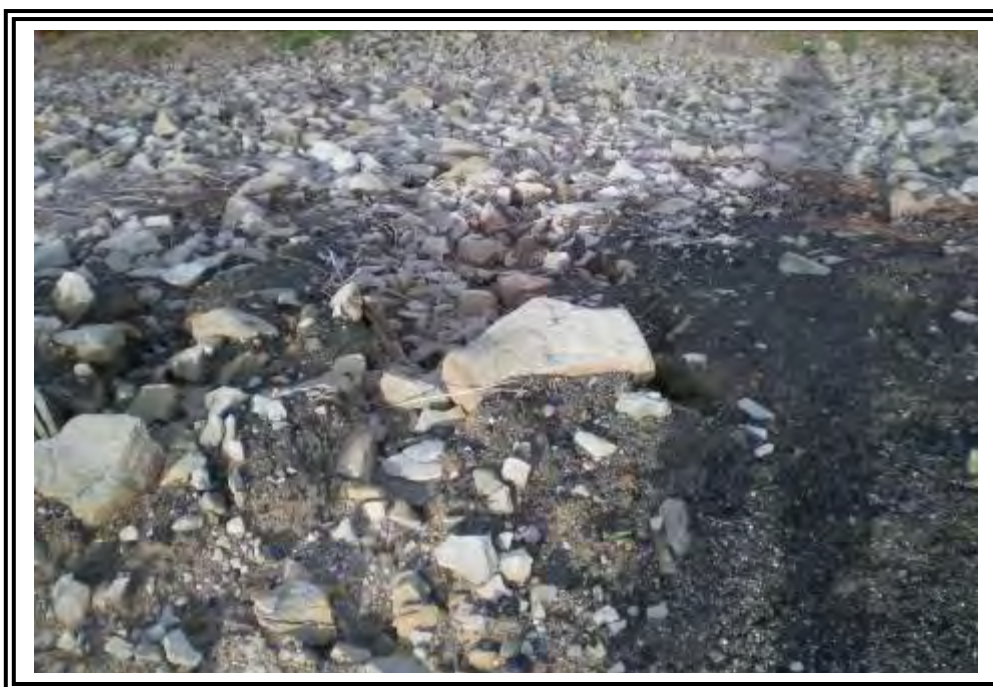
Migration of bottom ash material used to grade the crest onto the slope protection at the Lower Fly Ash Dam.
