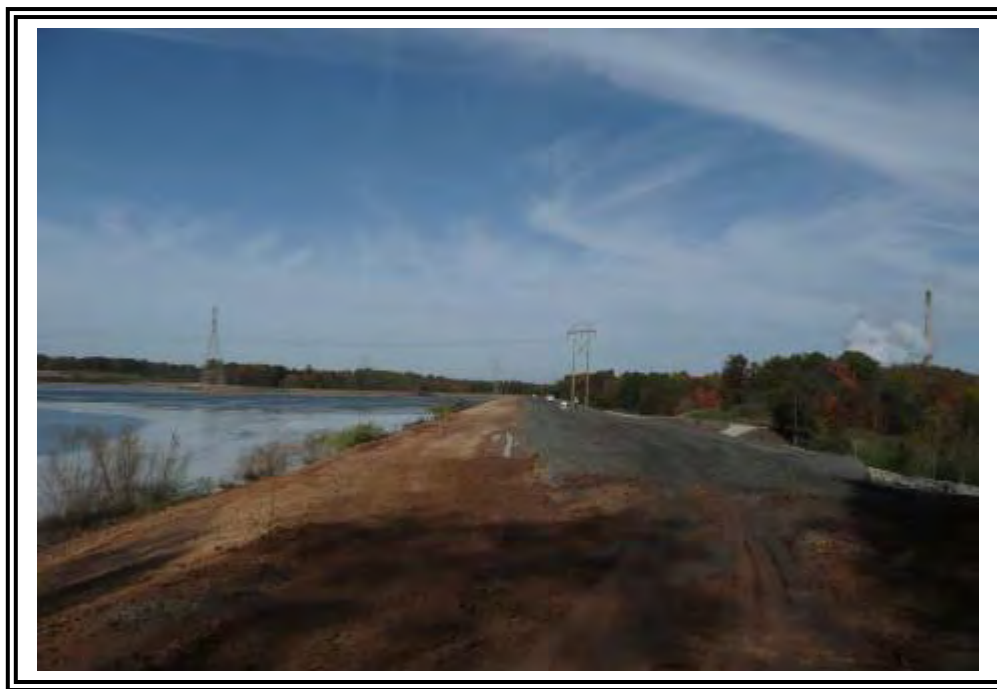
Crest area of Mill Stone Creek Dam, No-Name Creek Dam and part of Wing Dam, looking northwest. Note upstream clay zone and fly ash crest area – active construction.
