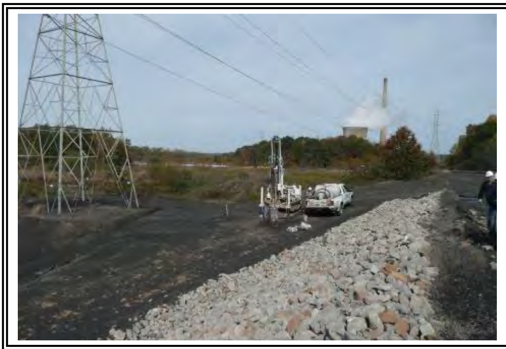
Downstream slope of the Wing Dam, looking north. The embankment makes a curve to an east-west alignment at this location. Crews were drilling for a new transmission tower foundation at the time of the site visit.
