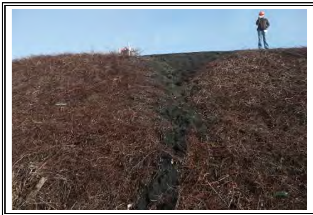
Erosion rill on the Units 1-4 Bottom Ash Pond south dike exterior slope.
