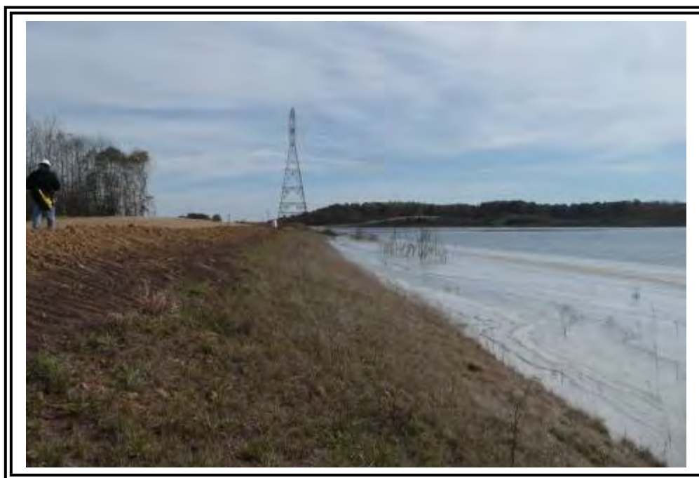
Upstream slope of the Spillway Dam, looking east towards transition to the Wing Dam. Note grass cover and moderate slope.
