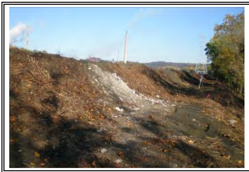
Units 1-4 Bottom Ash Pond upper east dike slope and bench area toward the central portion of the dike, looking north. Bench has narrowed to 8 to 8 feet wide.
