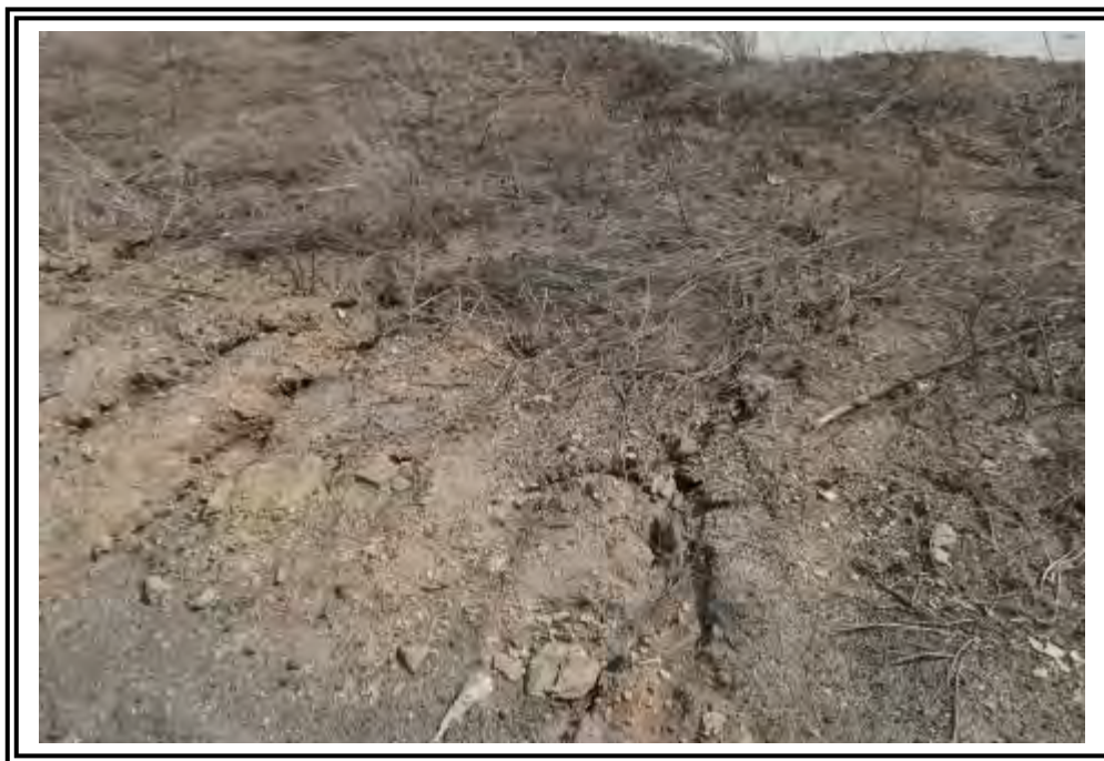
Erosion rills on upstream slope of the Middle Fly Ash Dam.
