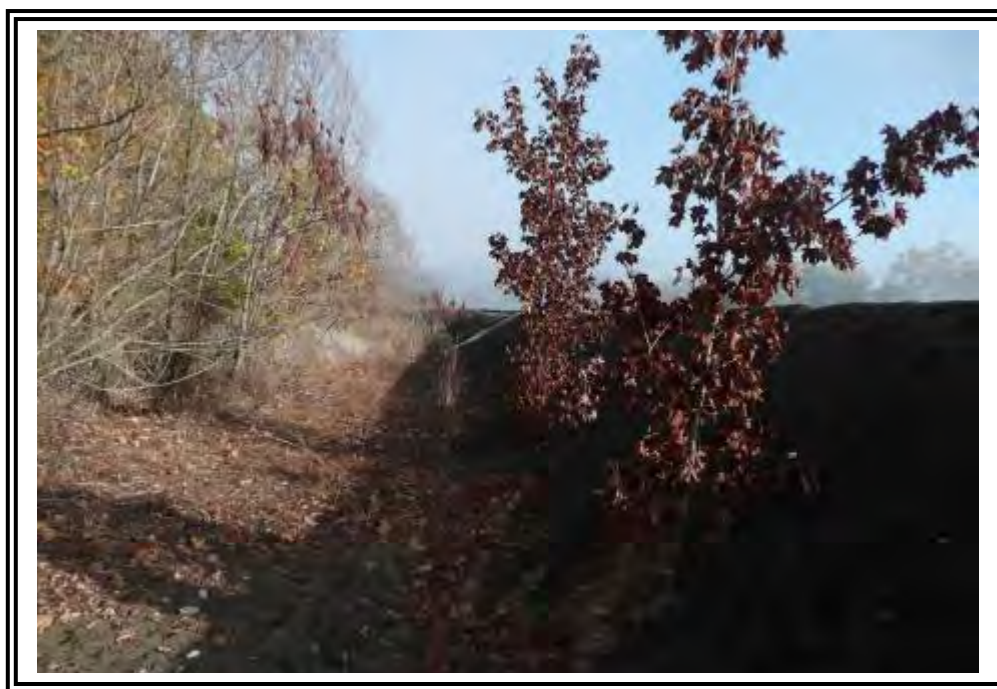
Units 1-4 Bottom Ash Pond west dike exterior slope, looking north. Note dying woody vegetation.
