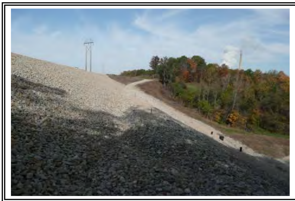
Downstream slope along mid-slope instrumentation bench at Mill Stone Creek Dam, looking northwest. Note rip-rap surface treatment.
