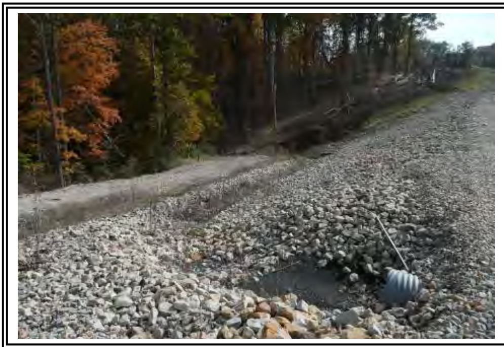
Mid-slope drainage groins and swale at toe of the Wing Dam downstream slope.
