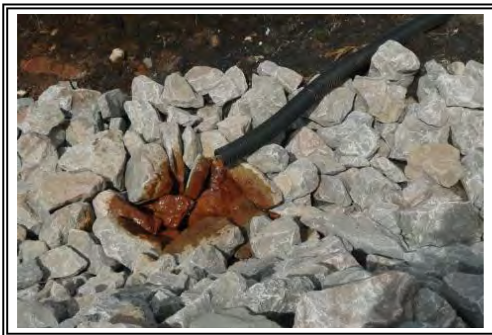
Seepage from hillside above the east abutment contact of the Middle Fly Ash Dam. Note iron precipitate.
