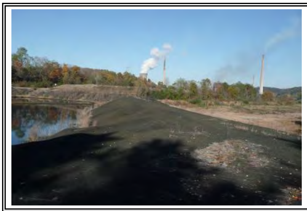
Units 1-4 Bottom Ash Pond interior dike crest and upstream slope at north end of the open pond area. Note bottom ash construction and generally sparse to absent vegetation.
