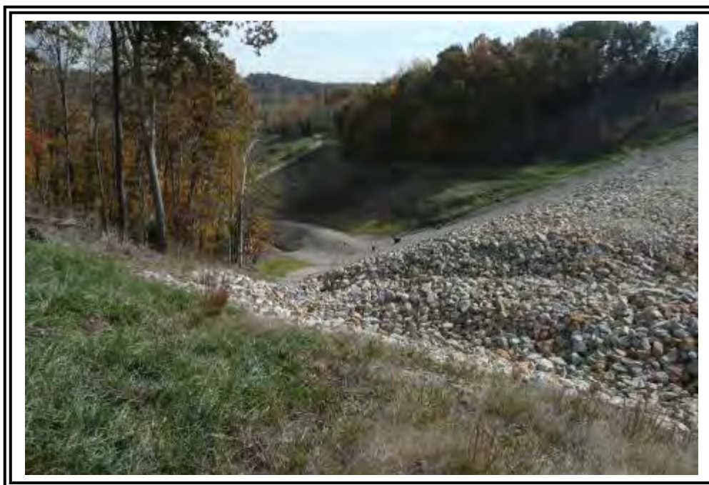
Downstream slope near crest of No-Name Creek Dam at left (northwest) abutment groin contact.
