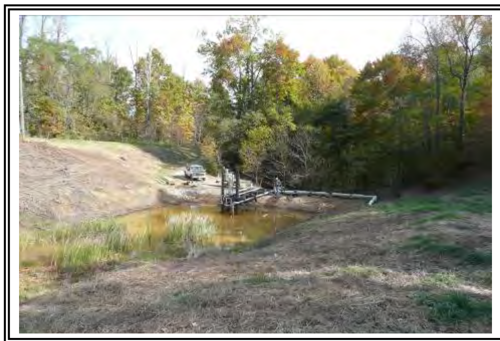
Seepage collection, treatment and recirculation basin at Mill Stone Creek Dam.
