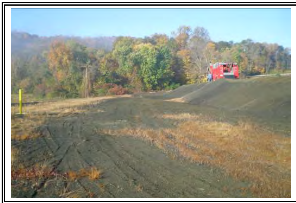
Units 1-4 Bottom Ash Pond south dike upper exterior slope and bench area, looking west. Note bench width in this area is on the order of 30 to 40 feet.
