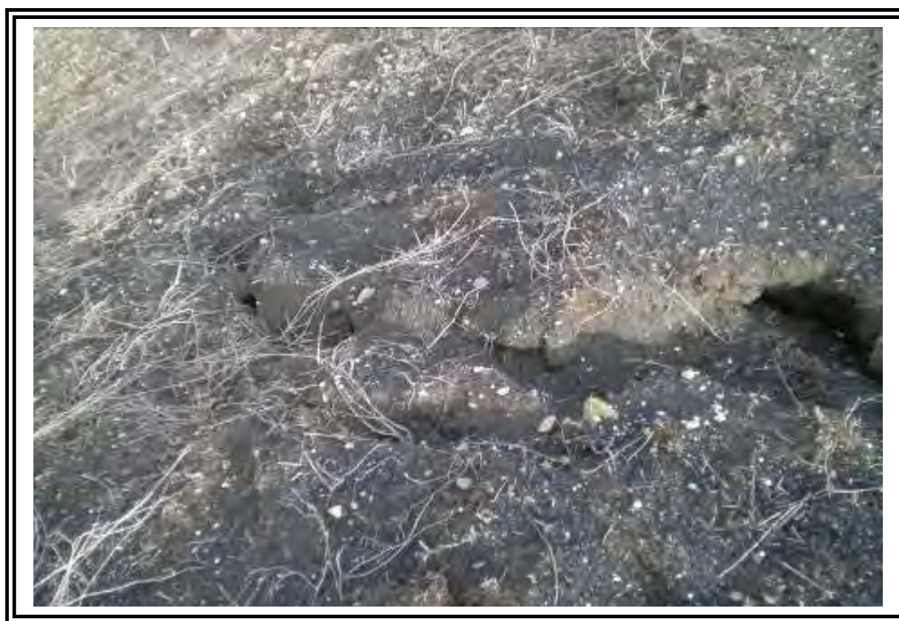
Erosion rills in bottom ash and soil surface on downstream slope of the Lower Fly Ash Dam.
