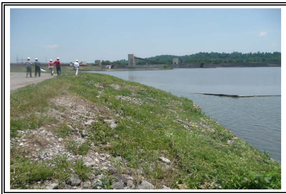
Intermediate dike, looking east.
