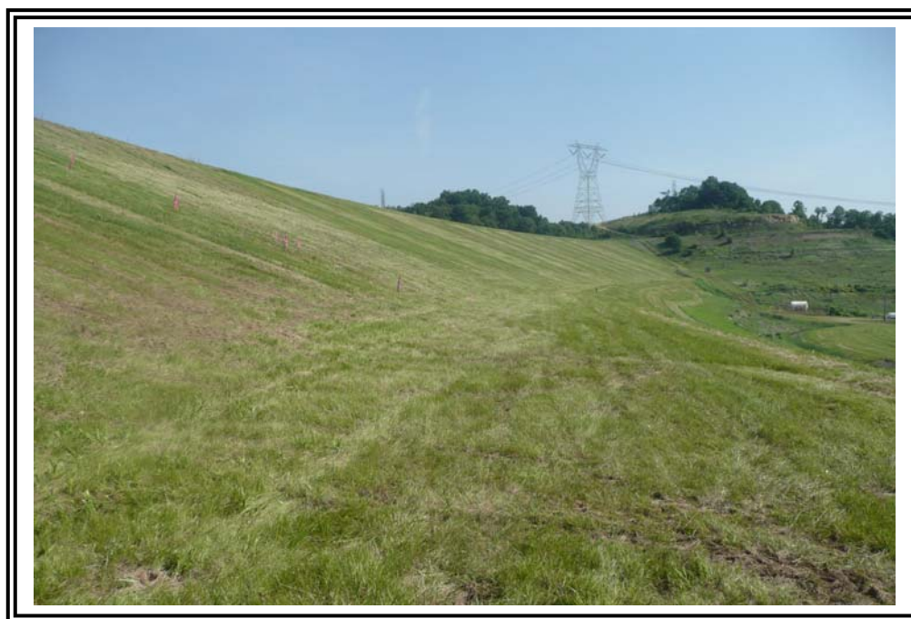
View along the bench on the downstream slope looking north. Note survey monitoring points, monitoring wells, and inclinometers.
