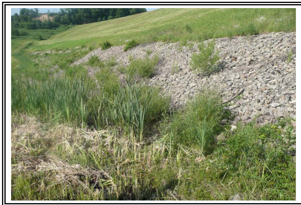
Toe drain area shows vegetative signs of being perennially wet.
