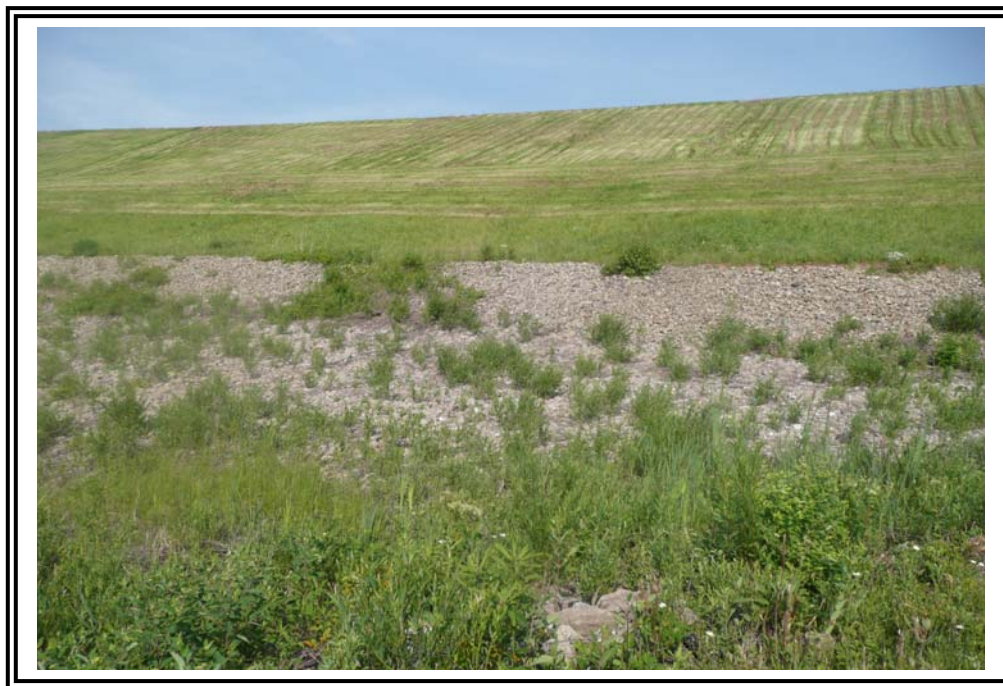
Toe drain covered with 6-inch diameter rip rap.
