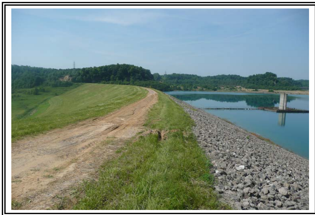
Dam crest from left (south) abutment. Note area of tire ruts appears to be from wet area resulting from runoff from the abutment.
