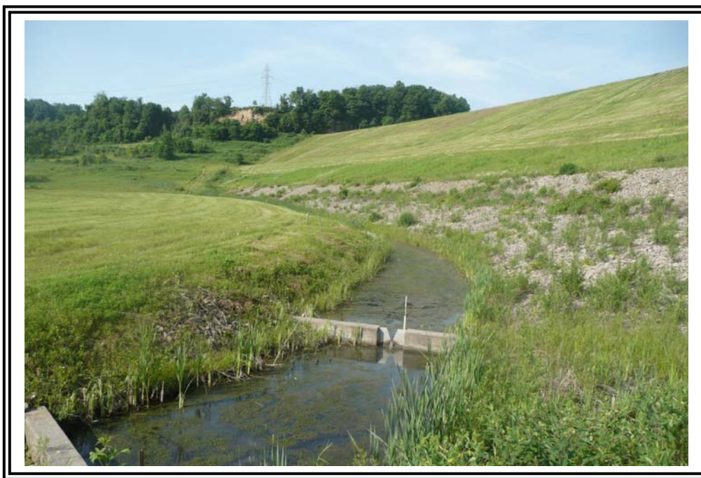
Drainage swale along toe of dam. Note monitoring weir structures. Much of the flow observed here was reportedly from recent rainfall runoff.
