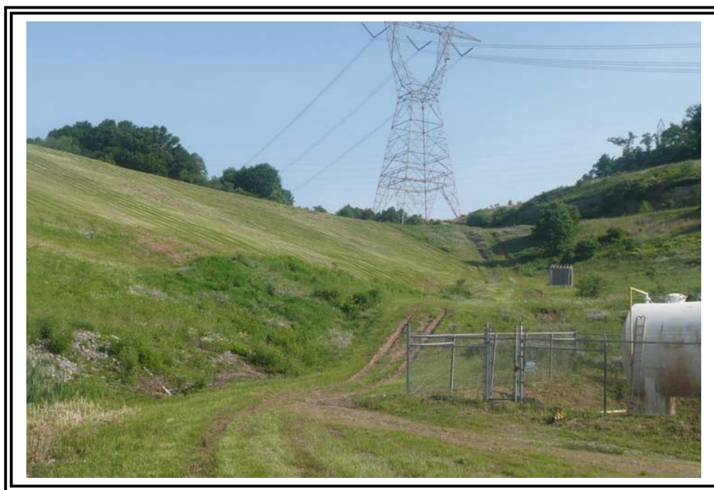
Left (north) downstream abutment contact.
