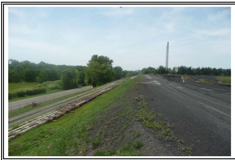
Crest and downstream slope alignment of east dike looking south. Note east dike is benched to allow an access road and sluice pipe placement.
