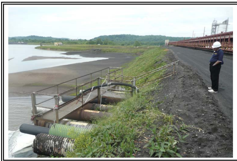
Crest and upstream slope alignment of north dike, looking west. Coal conveyor runs the length of the north dike crest.
