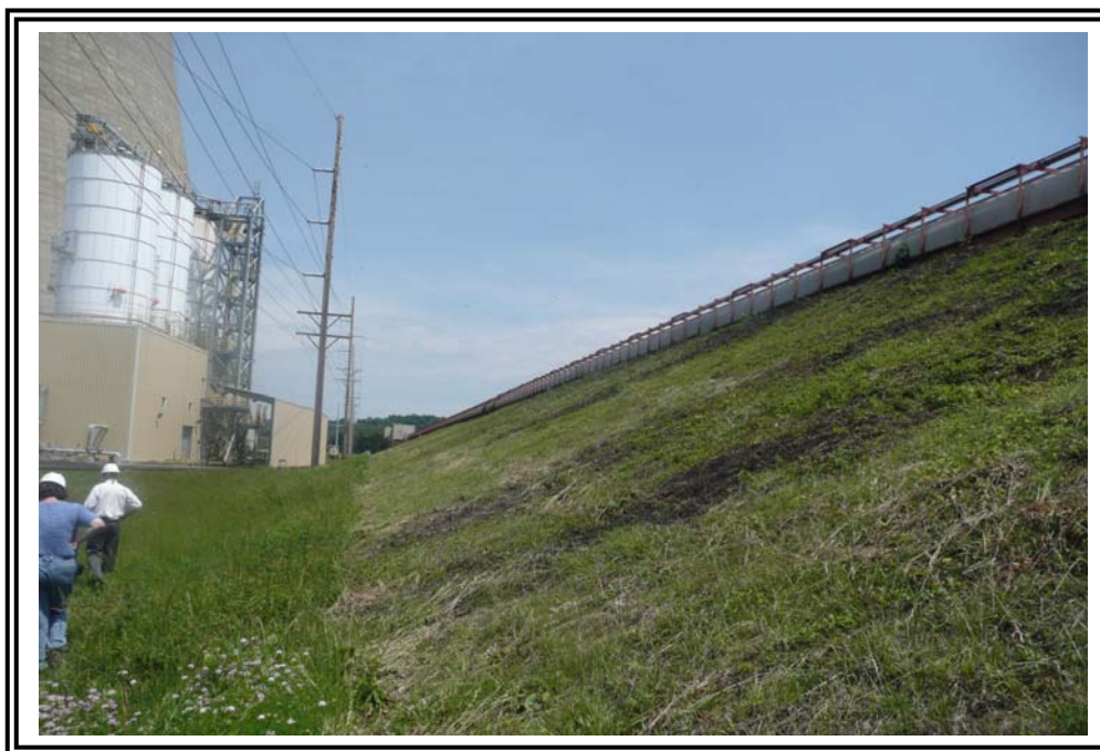
Downstream slope of north dike, looking east. Note dark areas in the grass on the slope are coal residue runoff from flushing the coal conveyor to remove dust buildup.
