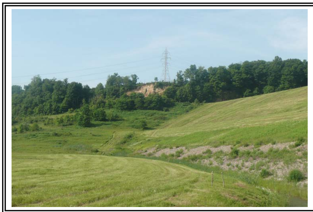
Right (south) downstream abutment contact.
