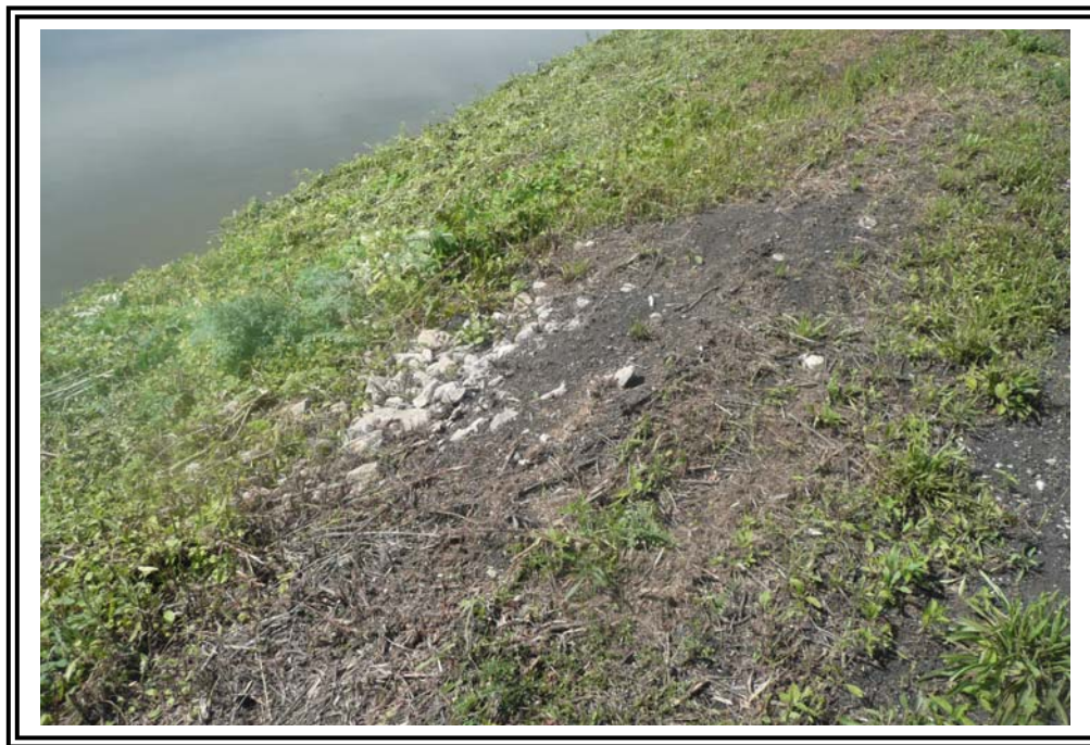
Erosion feature filling on the upstream slope of the west dike.
