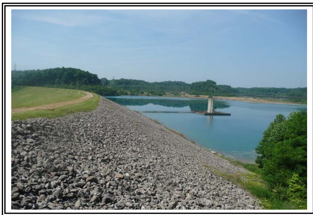
Upstream slope covered with 8-inch diameter rip rap.
