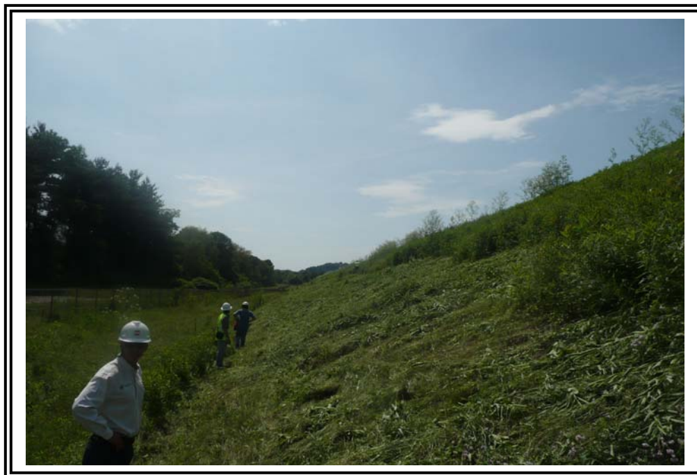
Downstream slope of south dike, looking west.
