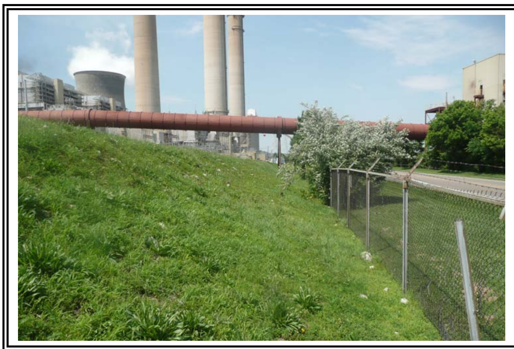
North end of east dike, looking north. This portion of the downstream slope is part of the benched out area for the access road.
