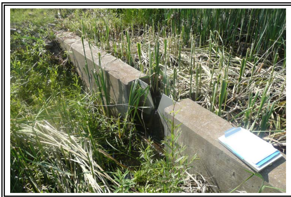
Close-up of Weir 3 near right (south) abutment/toe contact. Note significant difference in flow here compared to that shown in Photo (4) where all toe and groin flow for the whole length of the dam cumulates and discharges at Weir 1.
