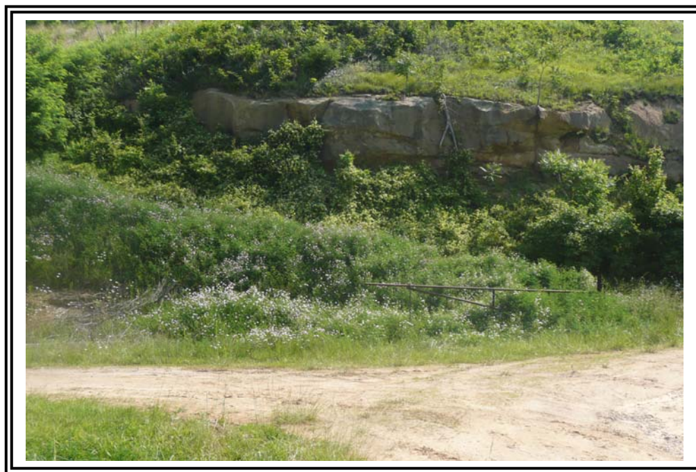
Left (north) abutment.
