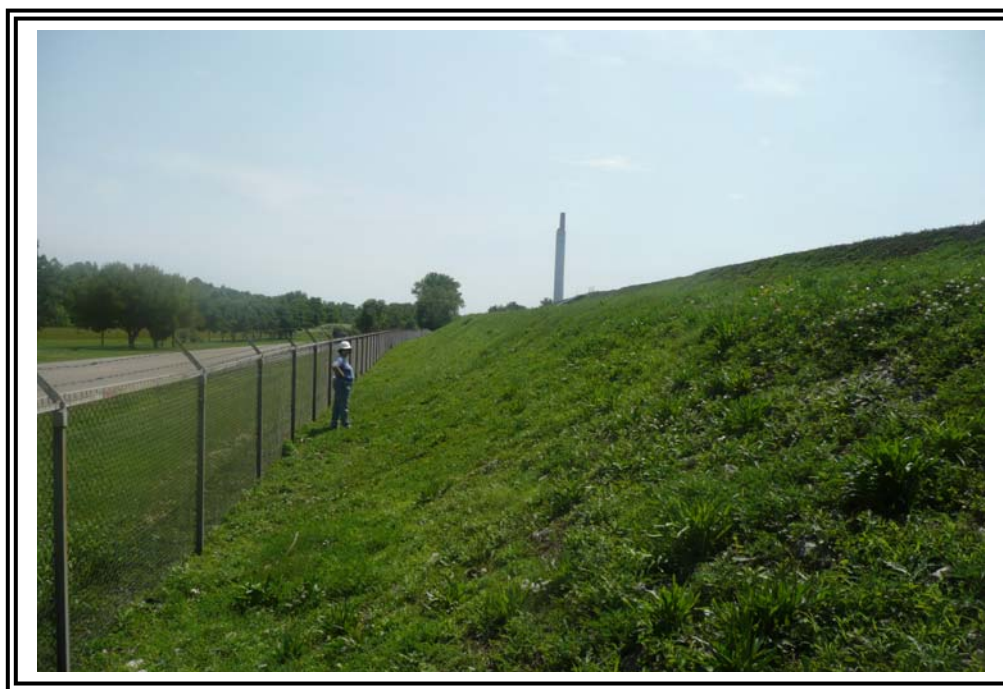
Downstream slope of east dike, looking south.
