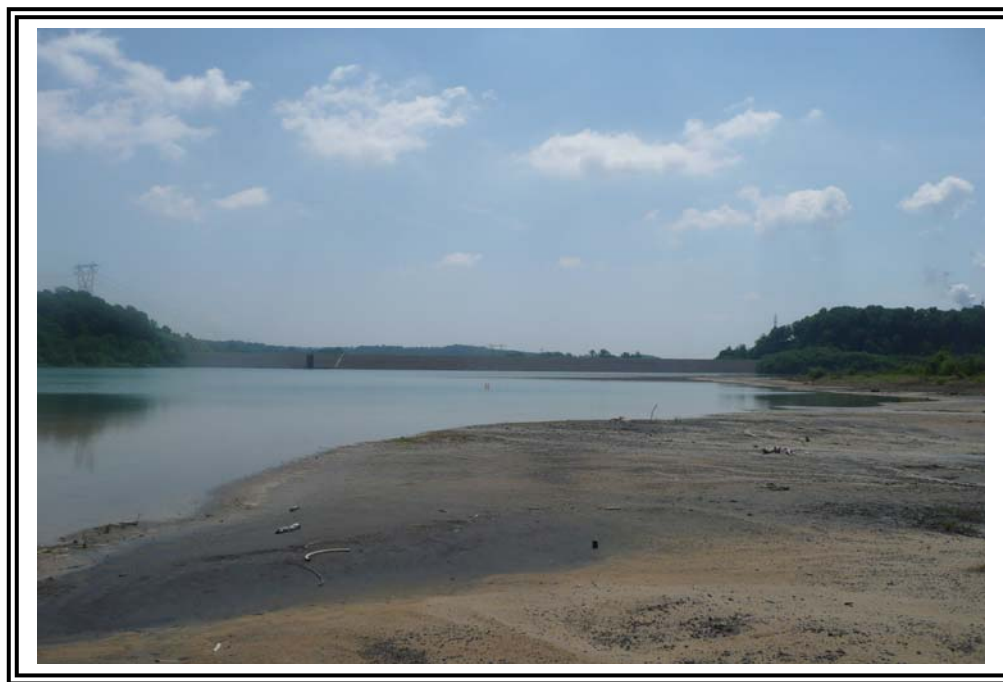
Upstream slope of the dam.
