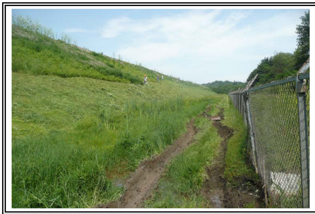
Downstream slope of south dike, looking east. Tractor ruts are in wet area at the toe where drainage backs up. This has been previously reported as a seepage area. Recent regrading to improve surface runoff appears to have dried this area and piezometer readings indicate the water table is below the toe of the dike.
