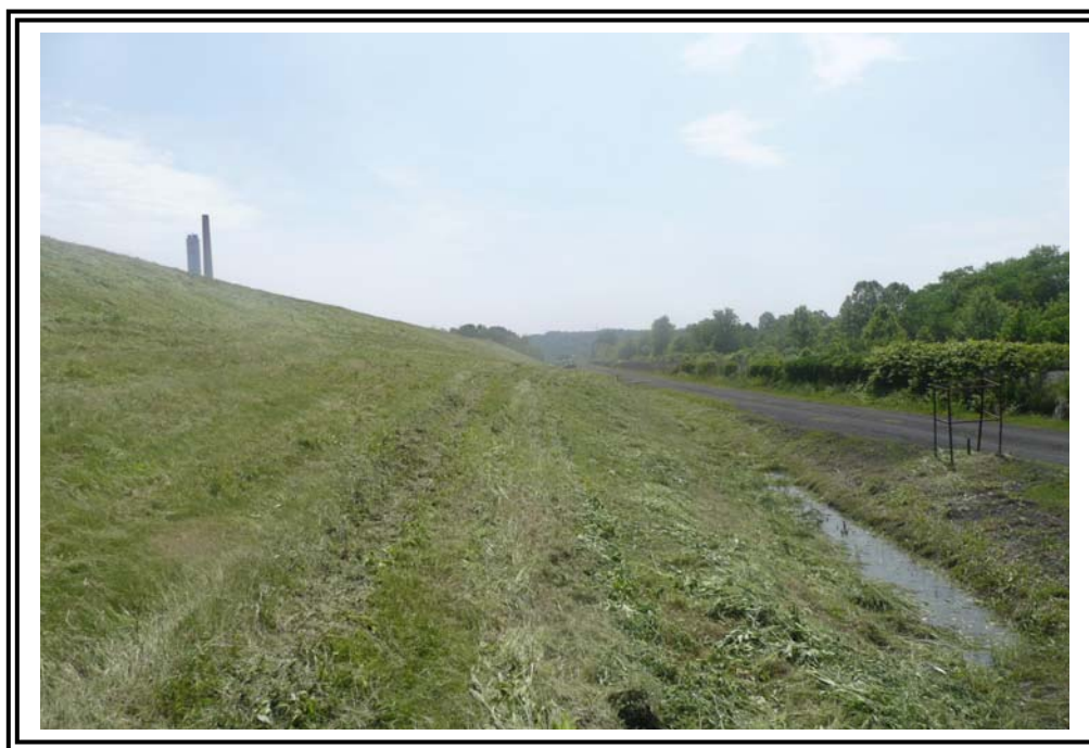
Apparent bulge reported in previous reports along west dike. No signs of current movement.
