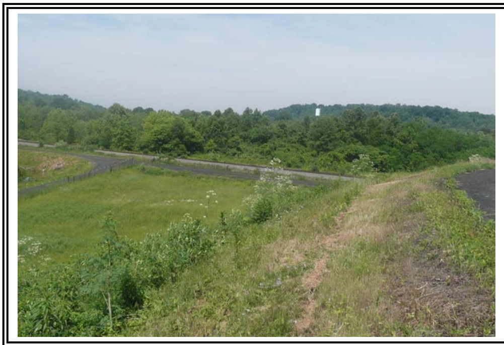
Downstream slope at southwest corner, looking west. Note that weed-whacking was in progress and is reportedly performed twice a year.
