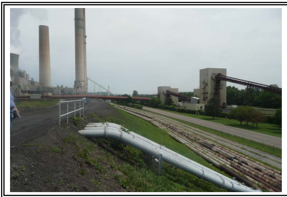
Crest and downstream slope alignment of east dike, looking north. Crest is raised at sluice pipe crossings.
