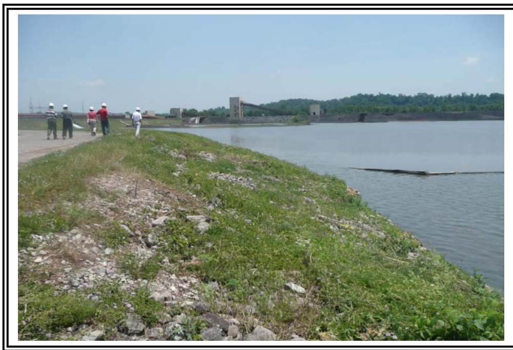
Intermediate dike, looking east.
