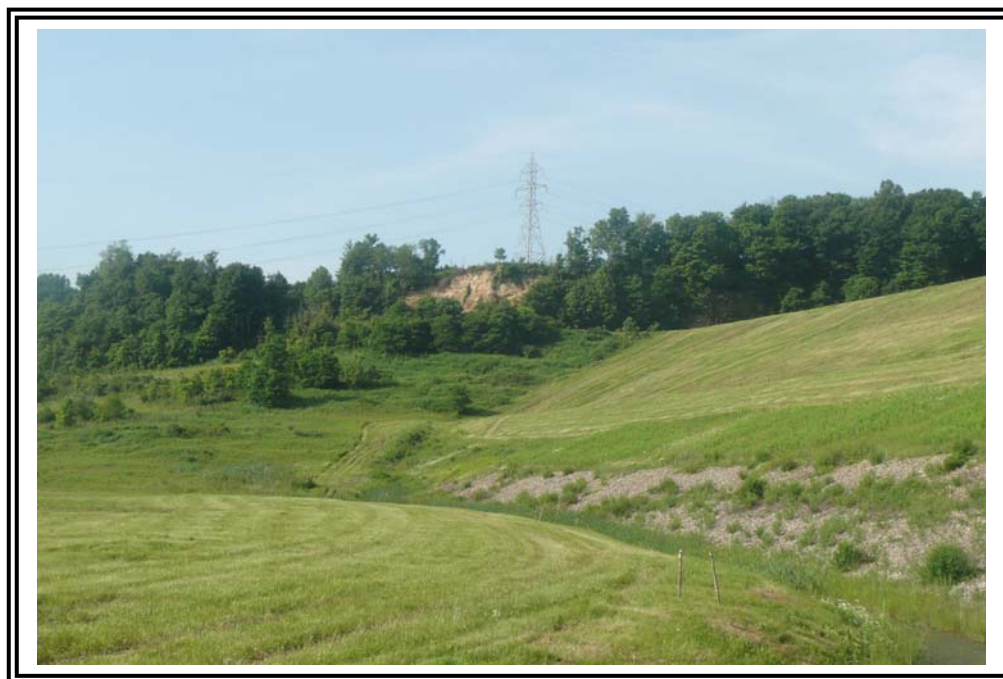
Right (south) downstream abutment contact.
