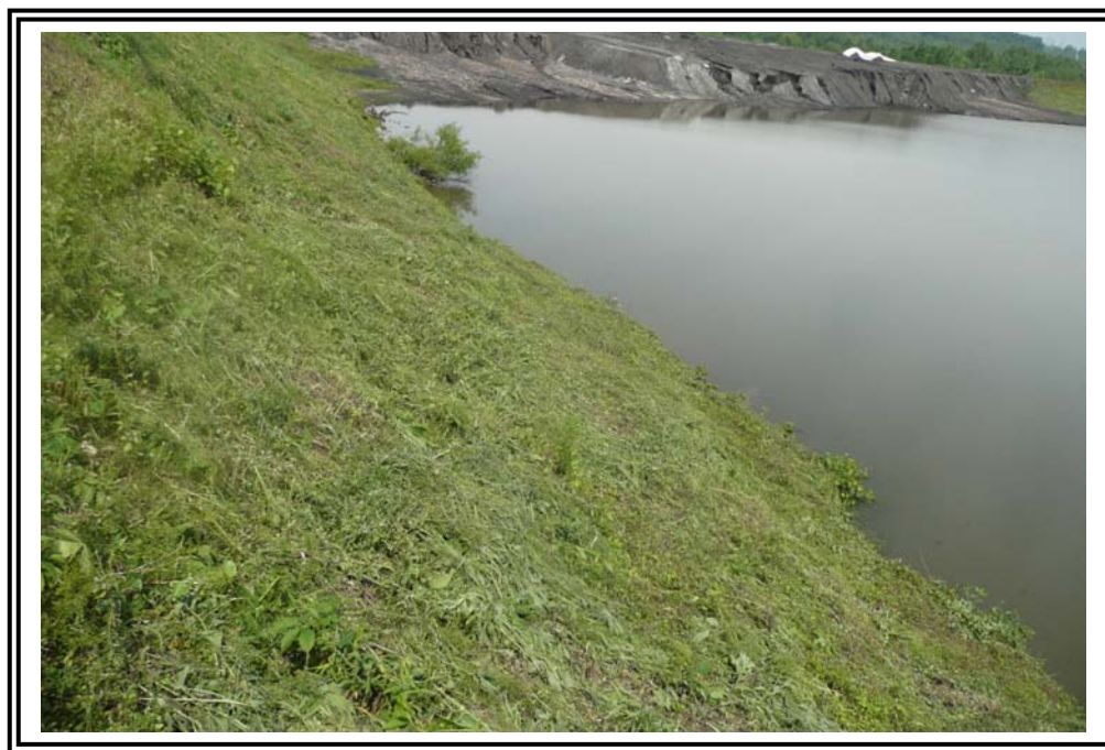
Close up of surficial slough on the upstream slope of the south dike, looking west.
