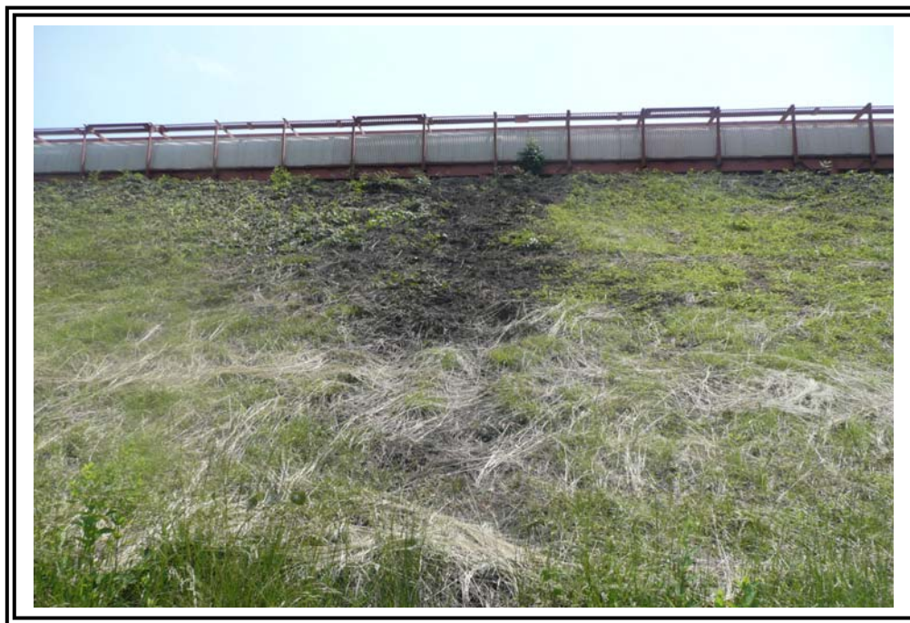
Close-up of one area of coal residue from coal conveyor flushing.
