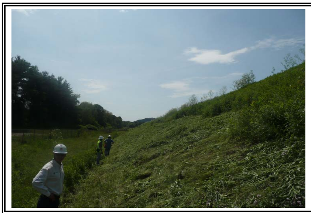
Downstream slope of south dike, looking west.
