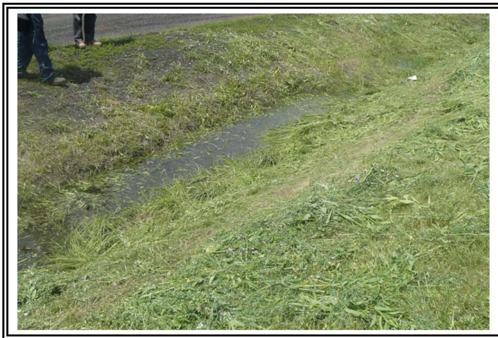
Standing water in drainage swale at toe of west dike. Appears related to surface water runoff. Piezometer readings confirm groundwater is well below the ground surface.
