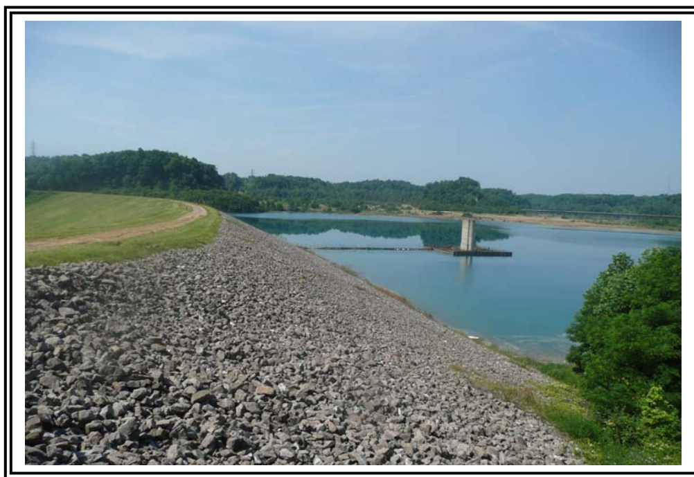
Upstream slope covered with 8-inch diameter rip rap.
