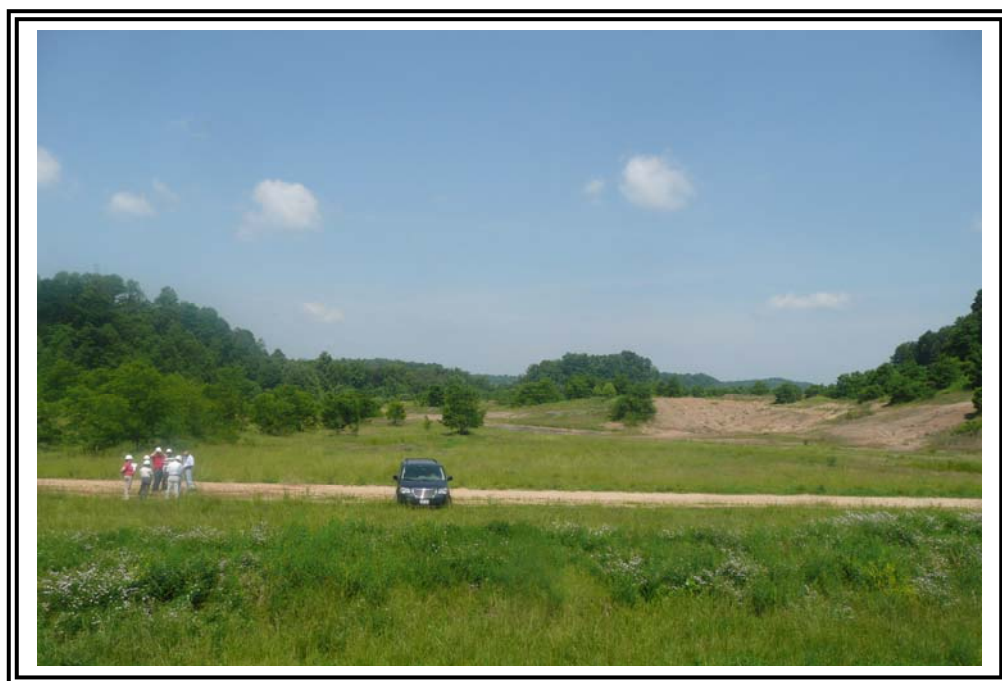
Abandoned emergency spillway looking toward reservoir.
