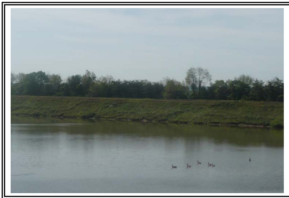
Upstream slope of the south dike, looking south. Note surficial sloughing.
