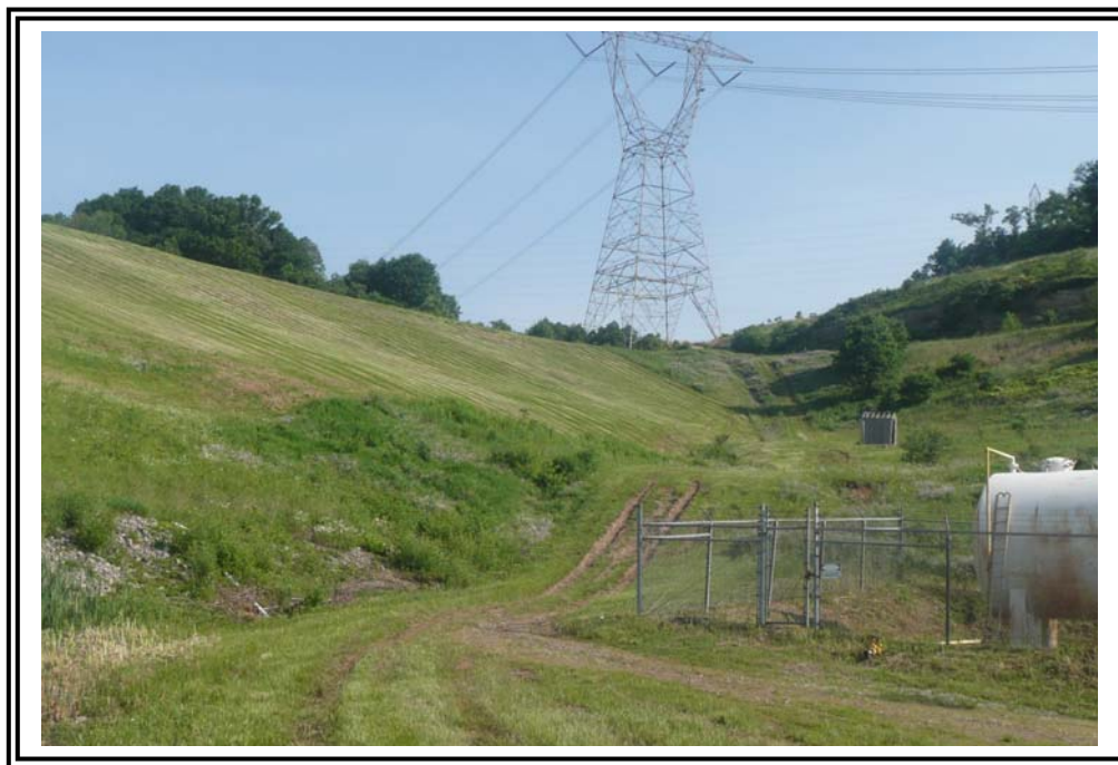
Left (north) downstream abutment contact.
