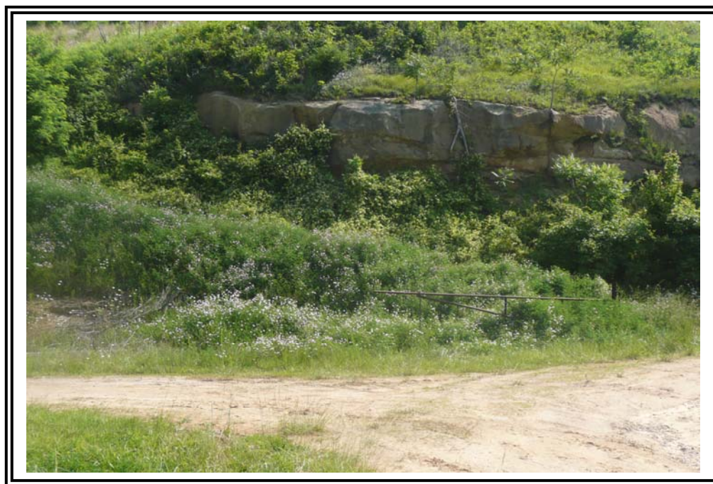
Left (north) abutment.
