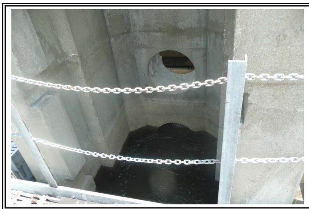
Main intake from primary pond to secondary pond.
