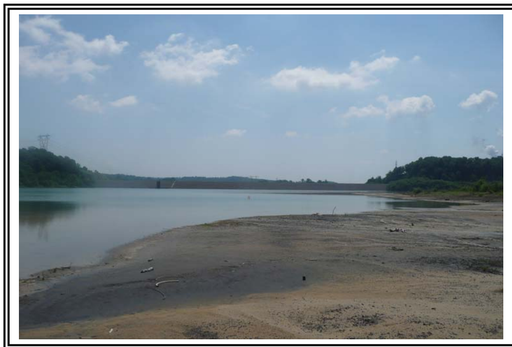
Upstream slope of the dam.
