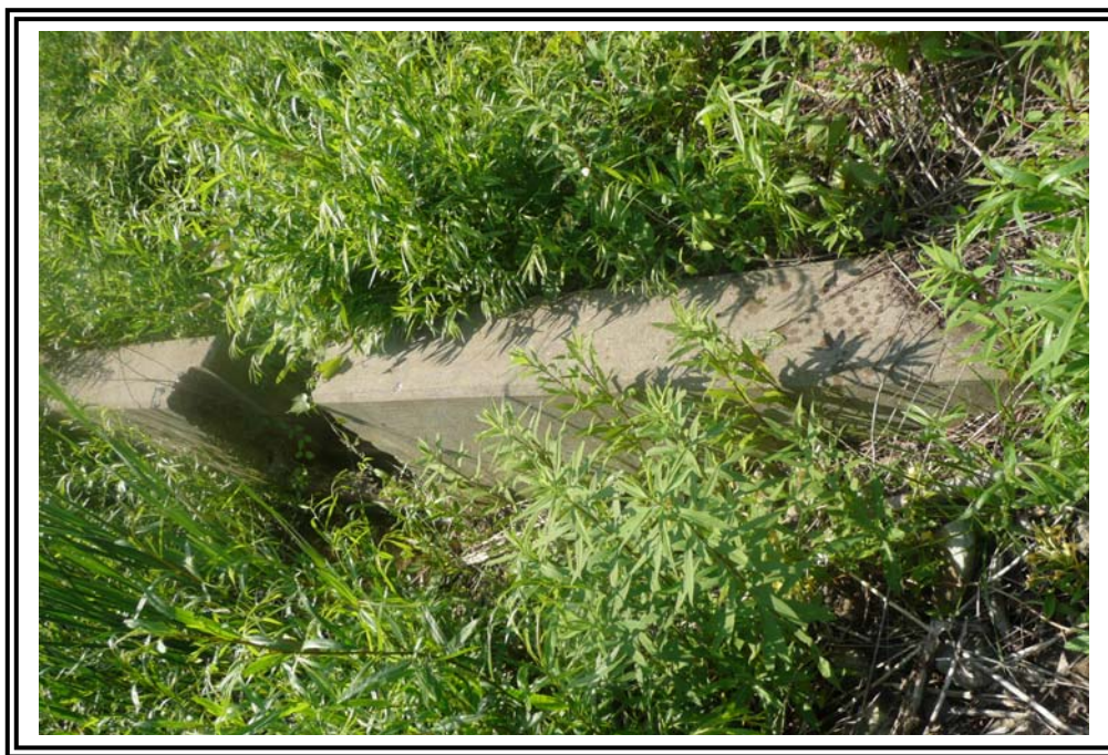
Abandoned weir structure located upstream of Weir 3 (appears weir plate was chipped out of the concrete). AEP staff was not aware when this was abandoned.
