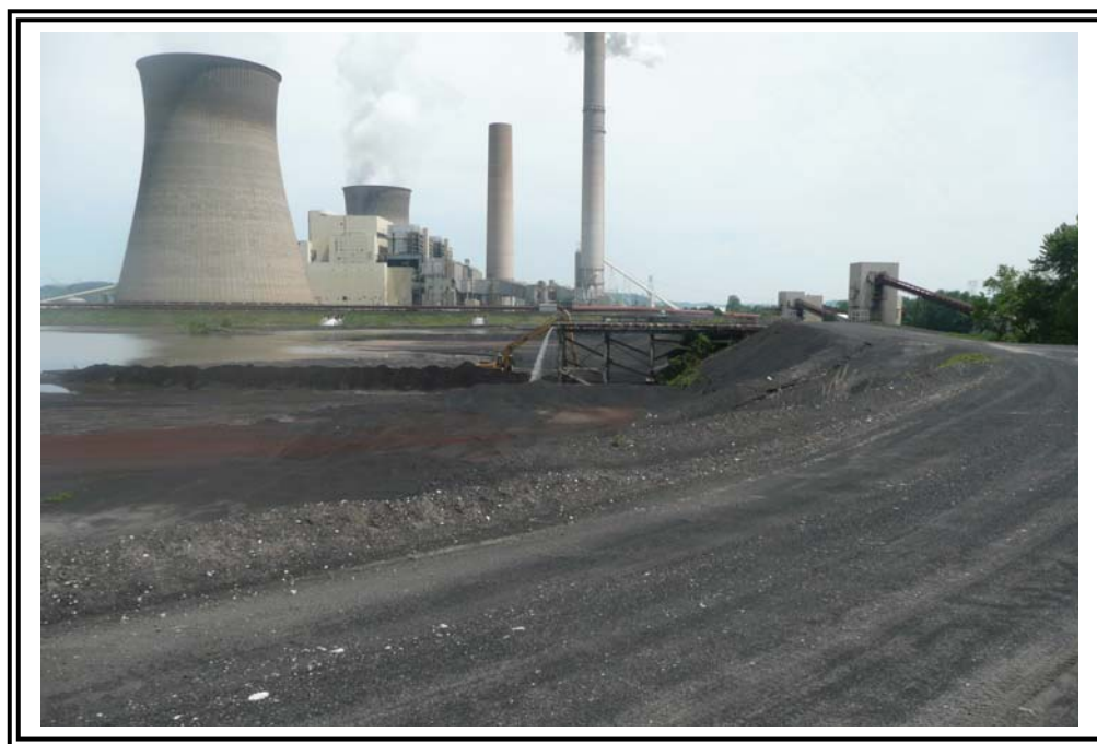
East end of the bottom ash pond. Bottom ash sluicing performed throughout this slope area.
