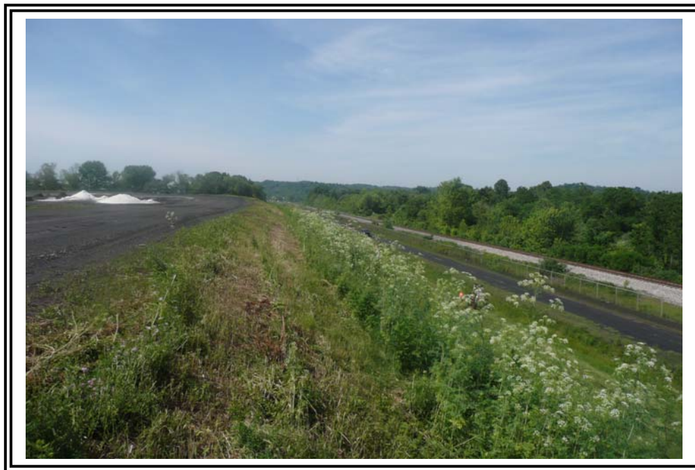
Downstream slope of the west dike, looking south. Note that weed-whacking was in progress and is reportedly performed twice a year.
