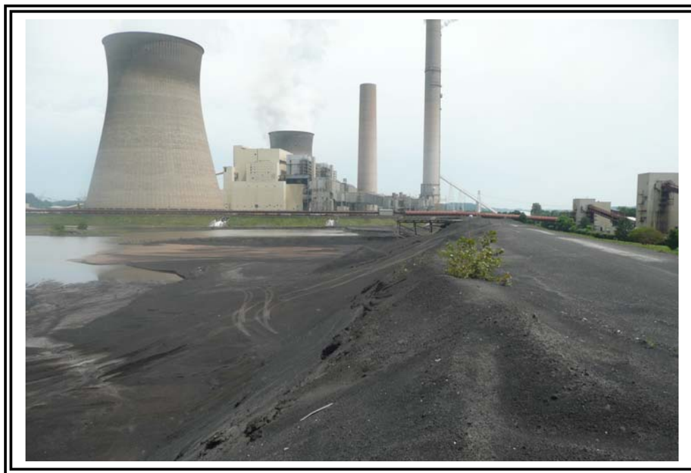
Ash disposal along upstream slope of east dike, looking north.
