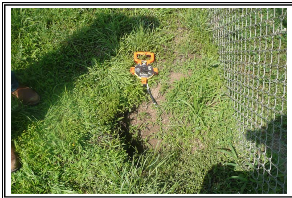
Several rodent holes were noted on the downstream slope of the east dike. Some were plugged from previous AEP efforts to deter rodents and repair holes. Others were unidentifiable as active or abandoned holes.
