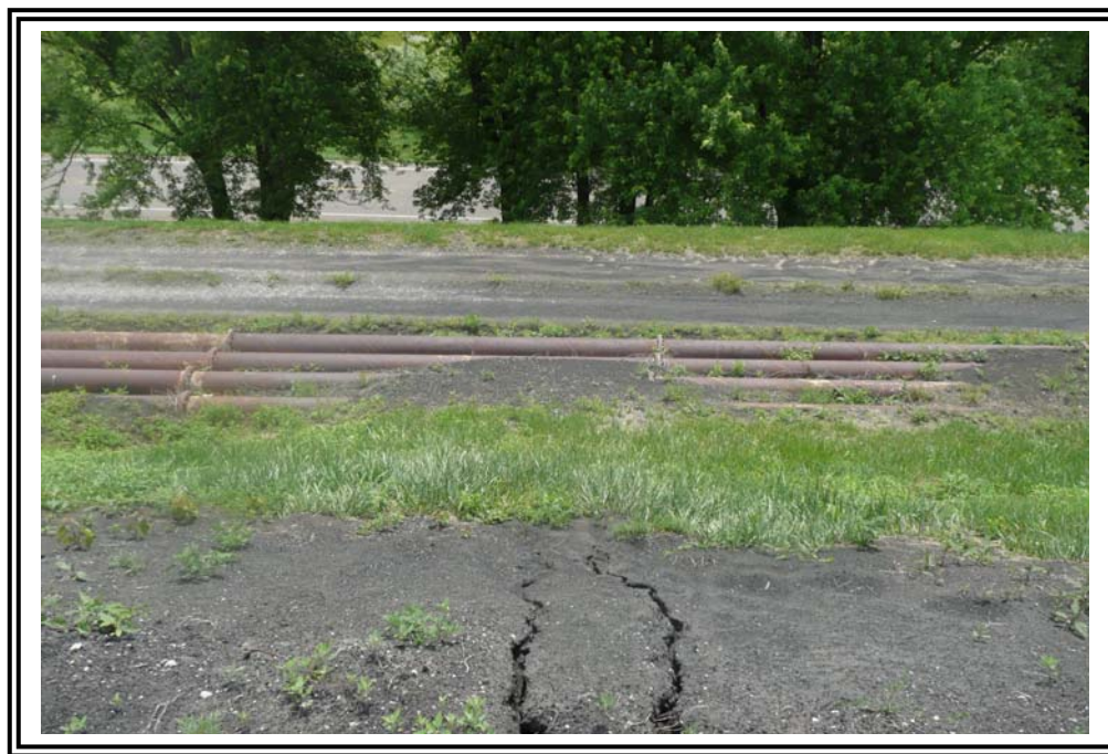
Surface erosion features (typical) along graded ash at east dike upstream slope/crest transition.
