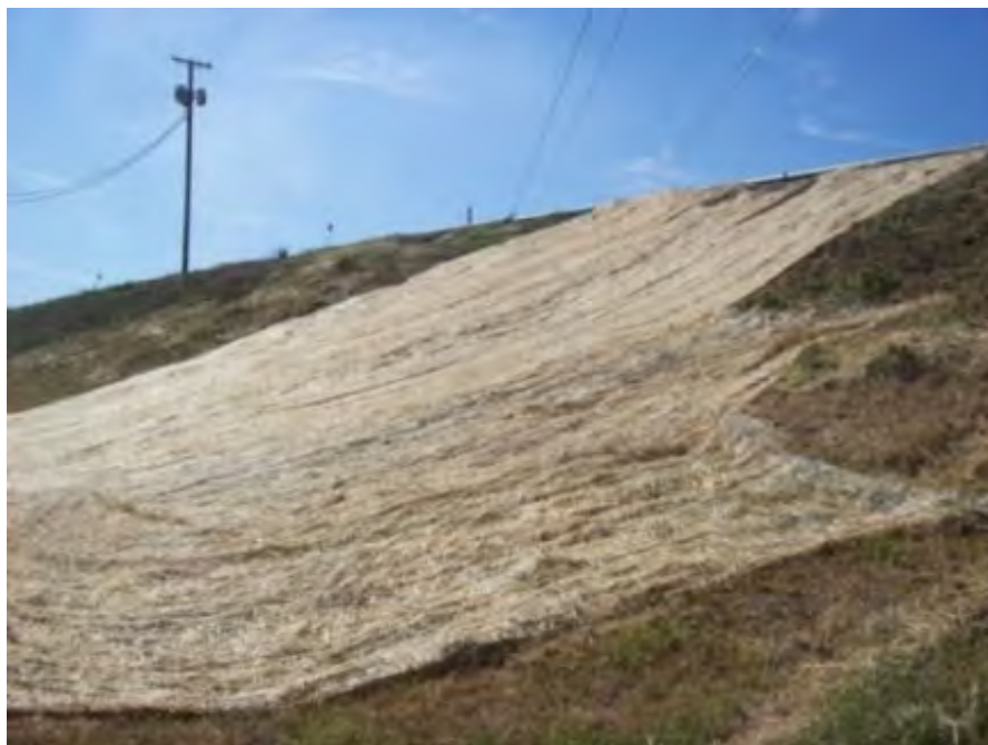
Geotextile for erosion remediation, Downstream Slope, East Dike, Bottom Ash Pond
