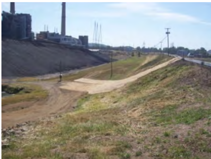
Erosion remediation, Downstream Slope, East Dike, Bottom Ash Pond
