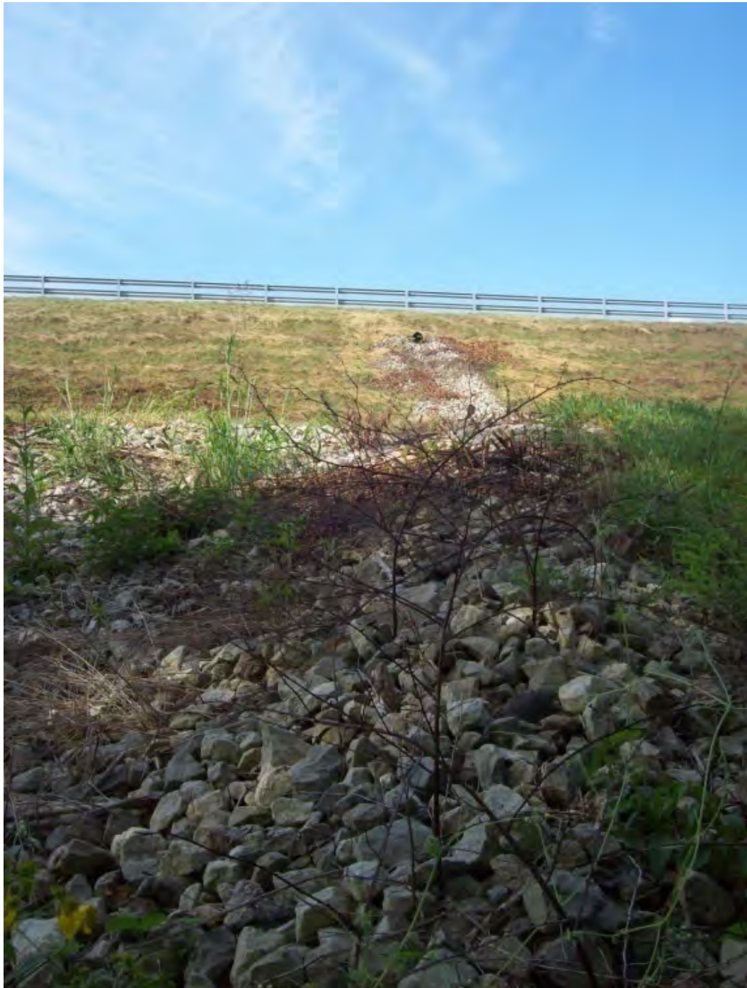
Erosion protection for road runoff, East Dike, Fly Ash Pond
