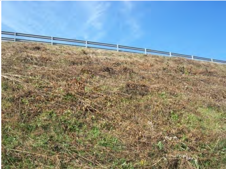
Maintenance for surface sloughing, downstream slope, East Dike, Fly Ash Pond
