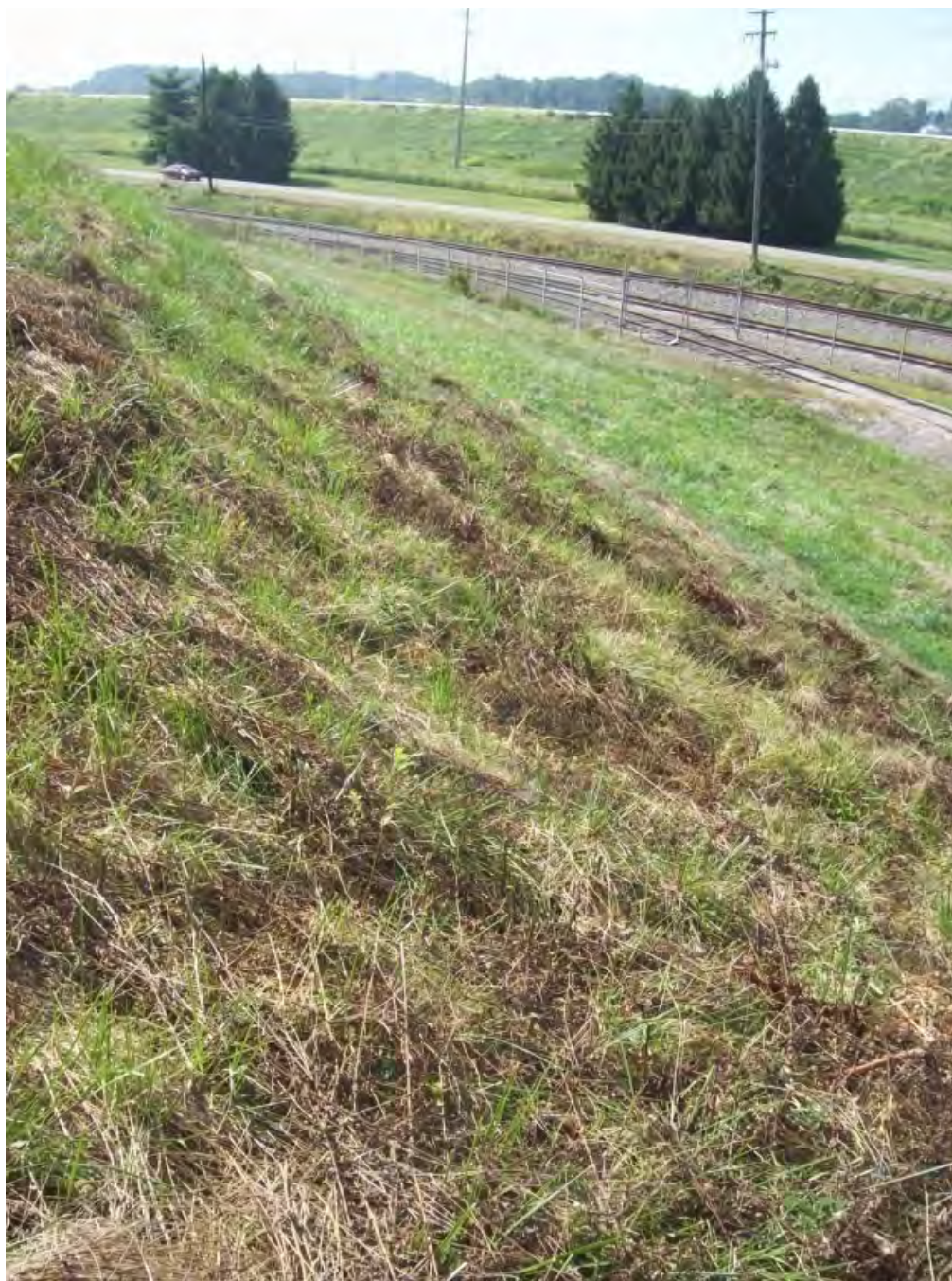
Surface erosion and sloughing on steep slope, Downstream Slope, West Dike, Fly Ash Pond
