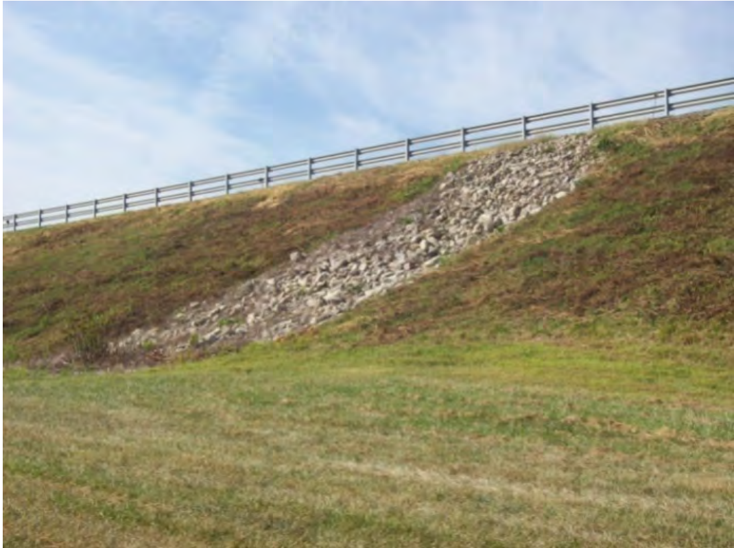
Slope erosion protection rip rap at East Dike, Fly Ash Pond
