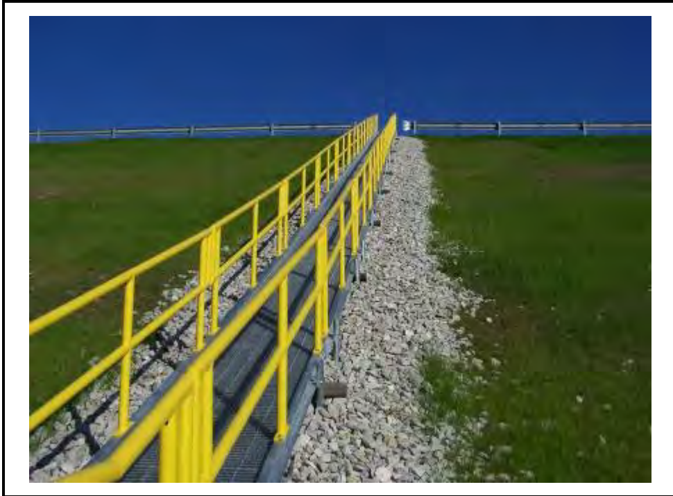
Access ramp to Horseford Creek Dam outlet structure.
