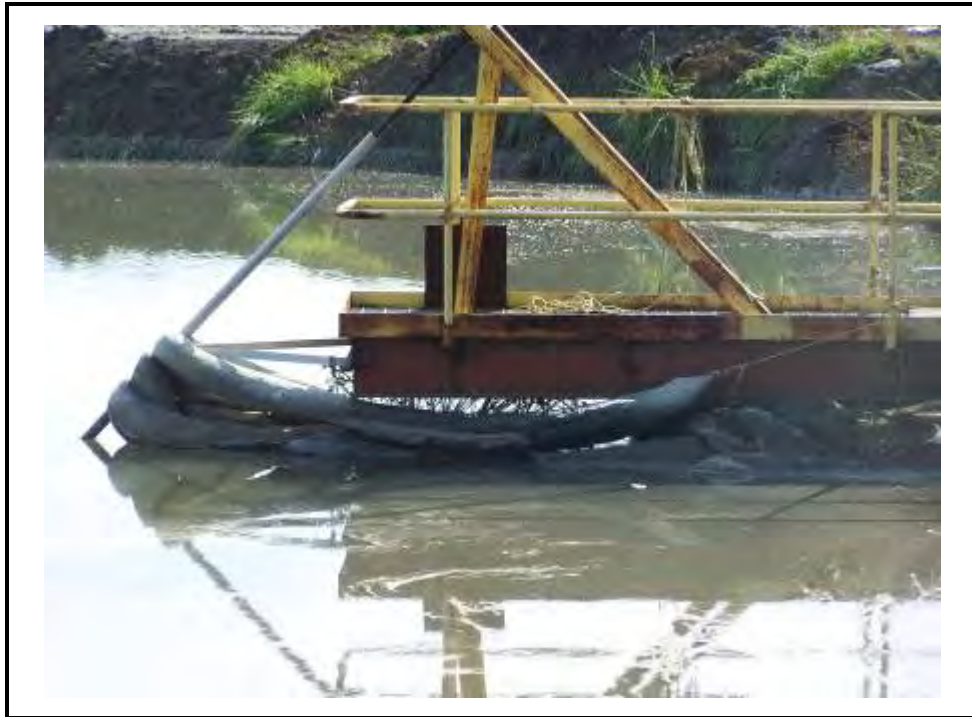
Close-up of decant structure in north Bottom Ash Pond.
