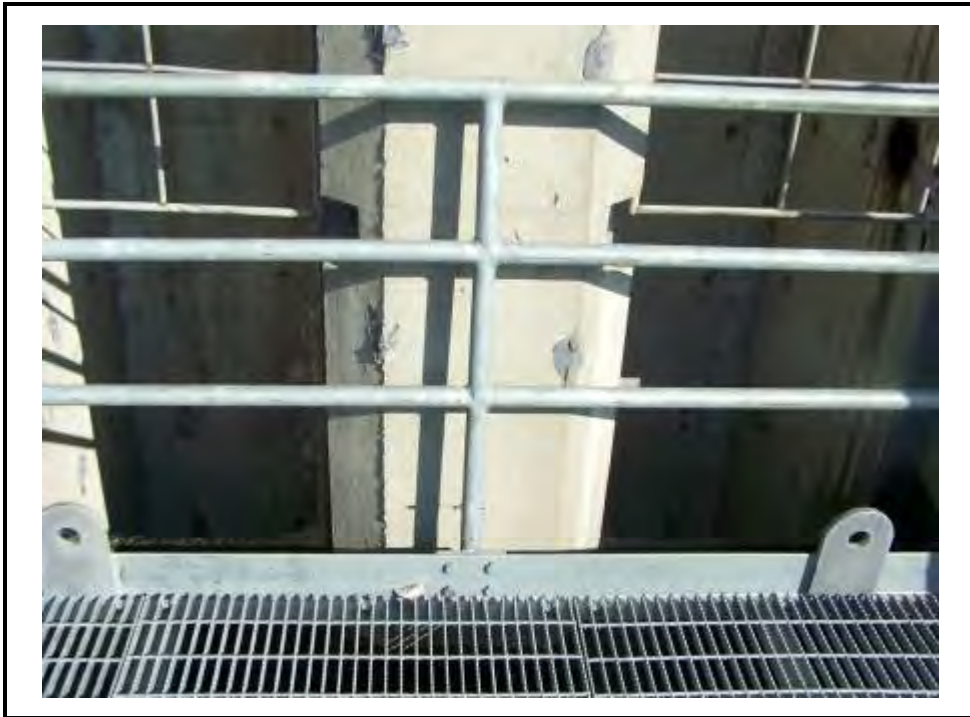
Twin stop log opening at Horseford Creek Dam outlet structure.
