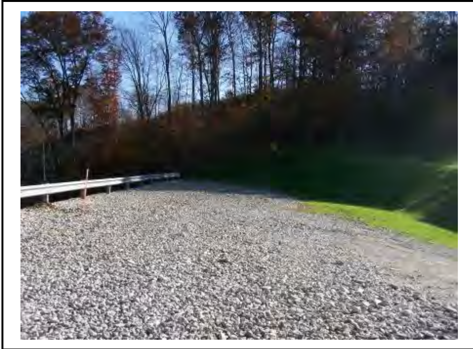
East abutment and crest of Horseford Creek Dam, looking east.
