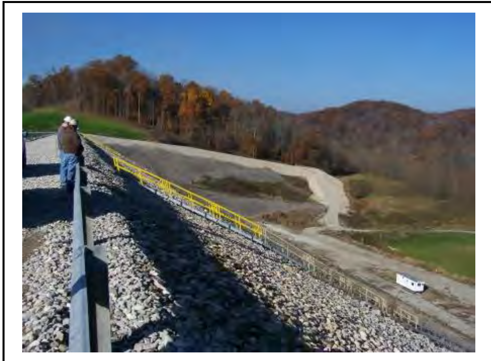
Downstream slope Horseford Creek Dam, looking west.
