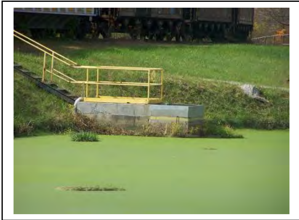
Close-up of non-permitted overflow to the Big Sandy River. Plant Personnel indicated that when water level reaches yellow line on the structure, pumping is initiated to Horseford Reservoir to prevent discharge to the river.
