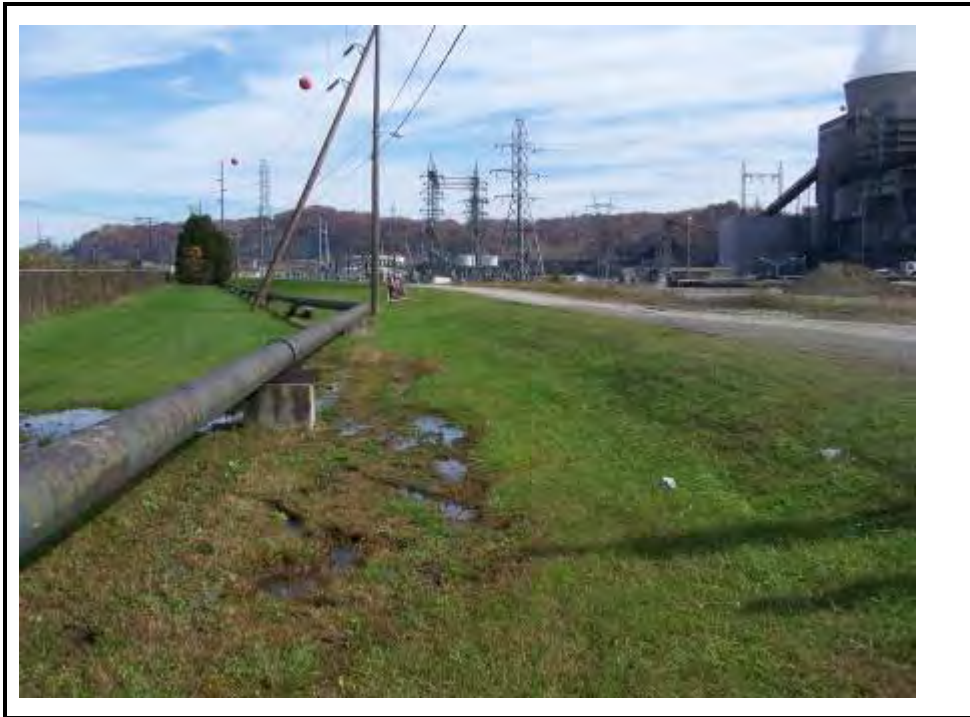
Downstream slope of North Dike and Bottom Ash Complex adjacent to north Bottom Ash Pond, looking east. Note that the north side of the Bottom Ash Complex is largely incised.
