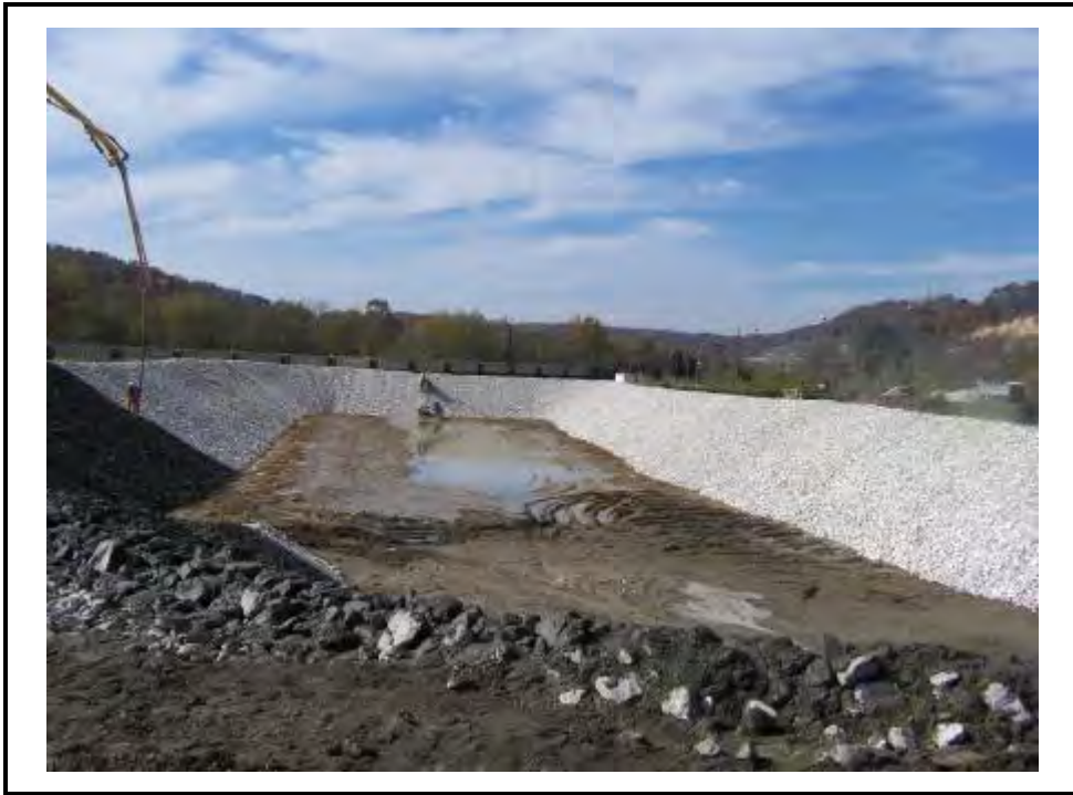
South Bottom Ash Pond looking west. AEP ws installing grouted rip rap on the inside slopes to reduce vegetation and erosion type maintenance.
