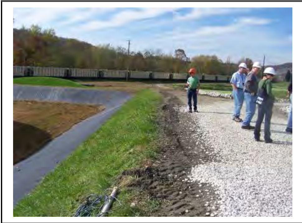
Crest of the South Dike at the Bottom Ash Complex looking west. Note dike crest slopes to about original grade adjacent to the south clear water pond. Liner on downstream slope is part of chemical spill containment berms.
