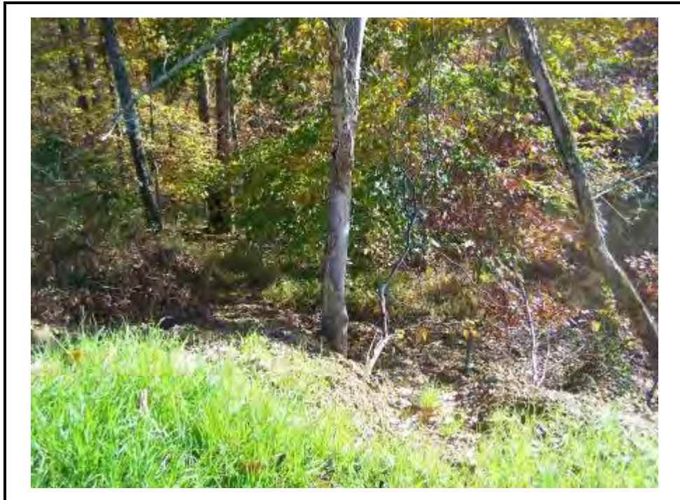
Downstream condition of "new" emergency spillway.
