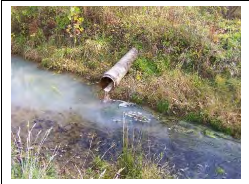
Drain pipe from east abutment area of Horseford Creek Dam. Note calcium deposits in water from limestone formations.
