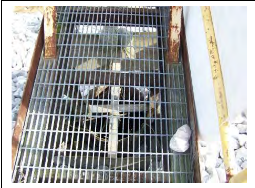
Close-up of south Bottom Ash Pond decant structure.
