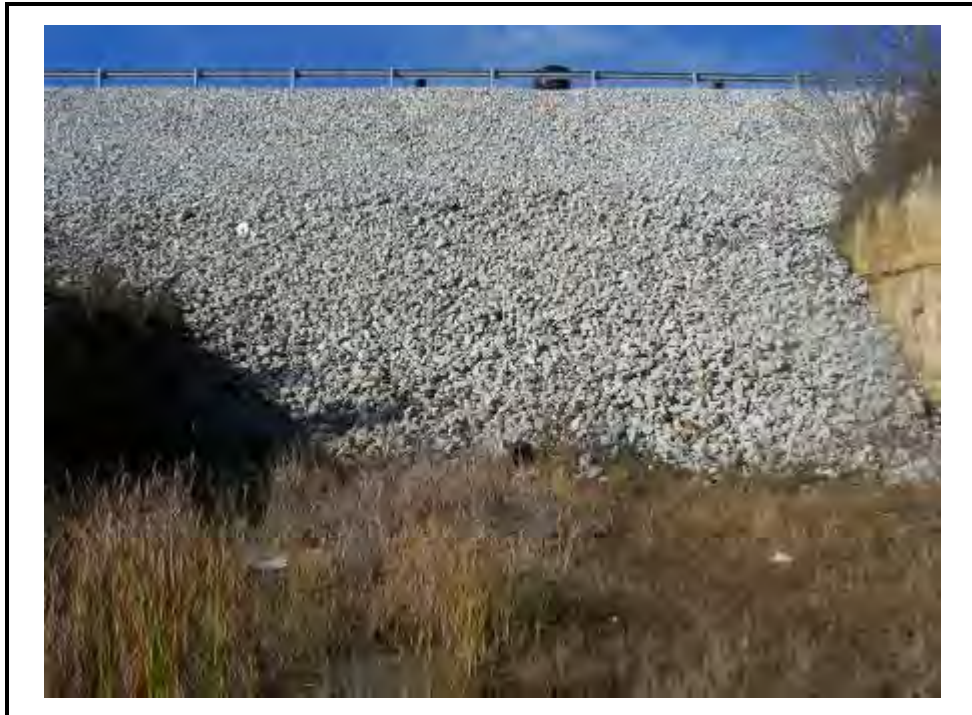
Downstream slope of Saddle Dam filling original emergency spillway.
