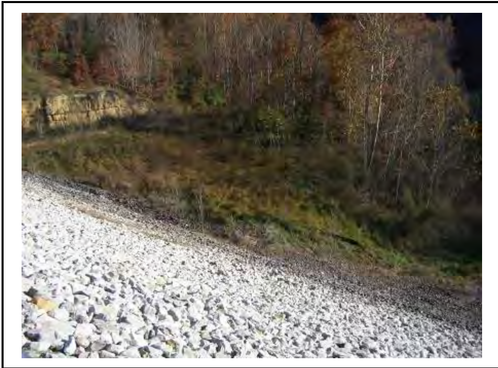
North downstream groin of Saddle Dam looking northeast. Bedrock in upper left is part of original emergency spillway channel which is now plugged. Note small trees in groin have been sprayed with herbicide.
