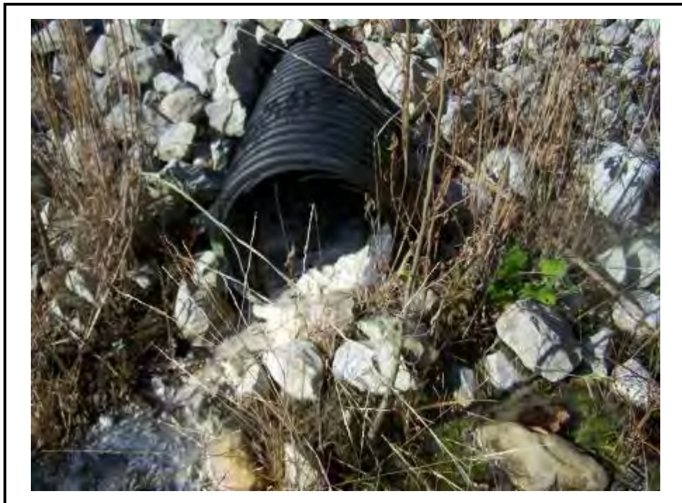
Seepage drain from original emergency spillway plug. Note calcium deposits from granular fill used in filter blanket.
