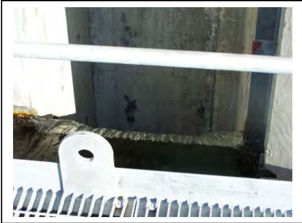
Close-up on one stop log opening at Horseford Creek Dam outlet structure.
