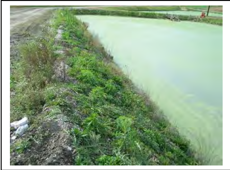
Upstream slope of South Dike of Bottom Ash Complex at south Clearwater Pond, looking west.
