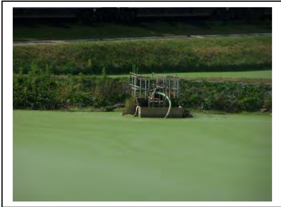
Decant structure from south Clearwater Pond to the Reclaim Pond.
