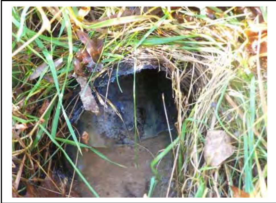
Toe drain outlet after clearing vegetation.
