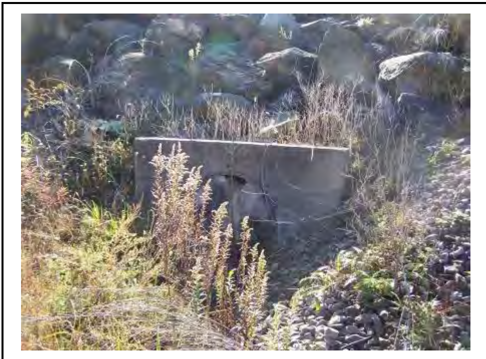
Phase I outlet pipe was abandoned in place.
