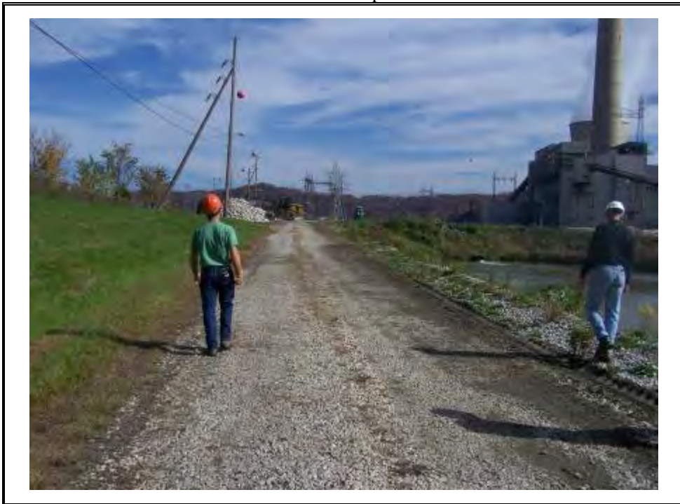
Crest of North Dike of Bottom Ash Complex along north Clearwater Pond where Bottom Ash Complex is incised.
