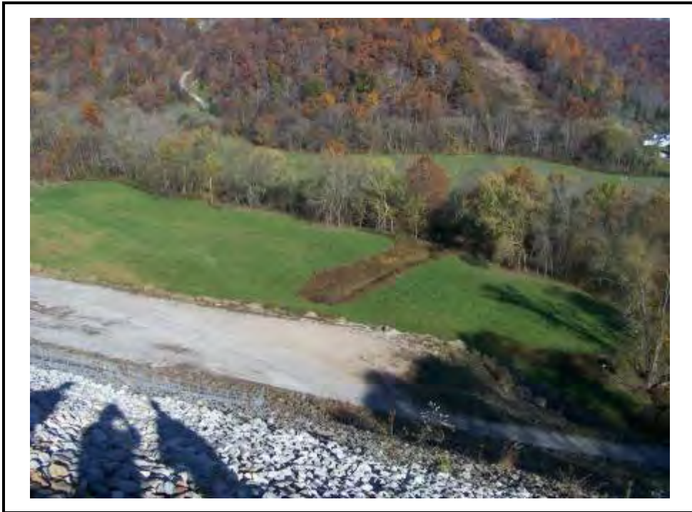
Downstream slope and buttress of Horseford Creek Dam looking north. Channel in field is original discharge channel which is now abandoned.
