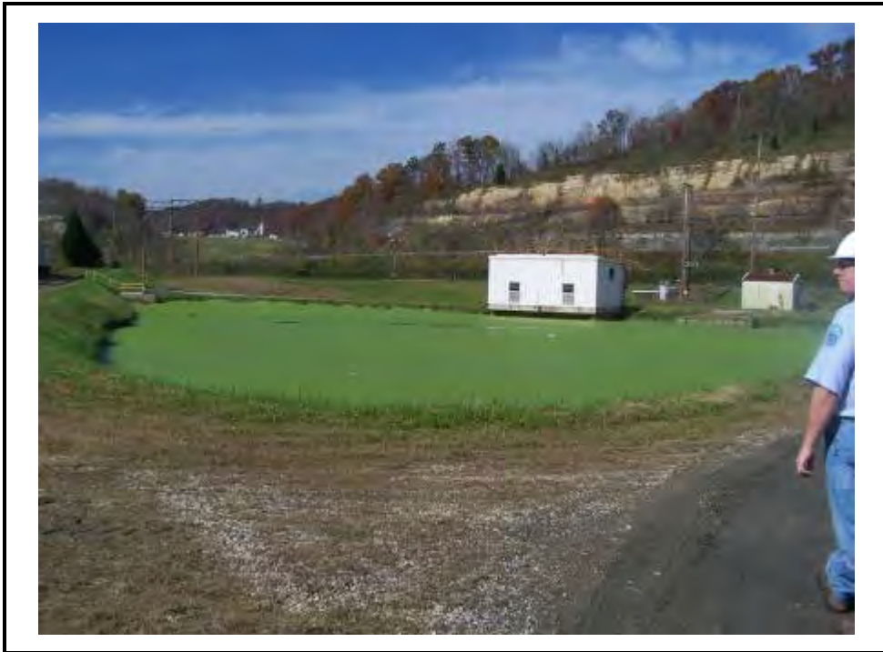
Reclaim Pond (incised) looking west. Building is the pump station which diverts flows back to the plant or to Horseford Reservoir. At west end of pond is a non-permitted overflow to the Big Sandy River.
