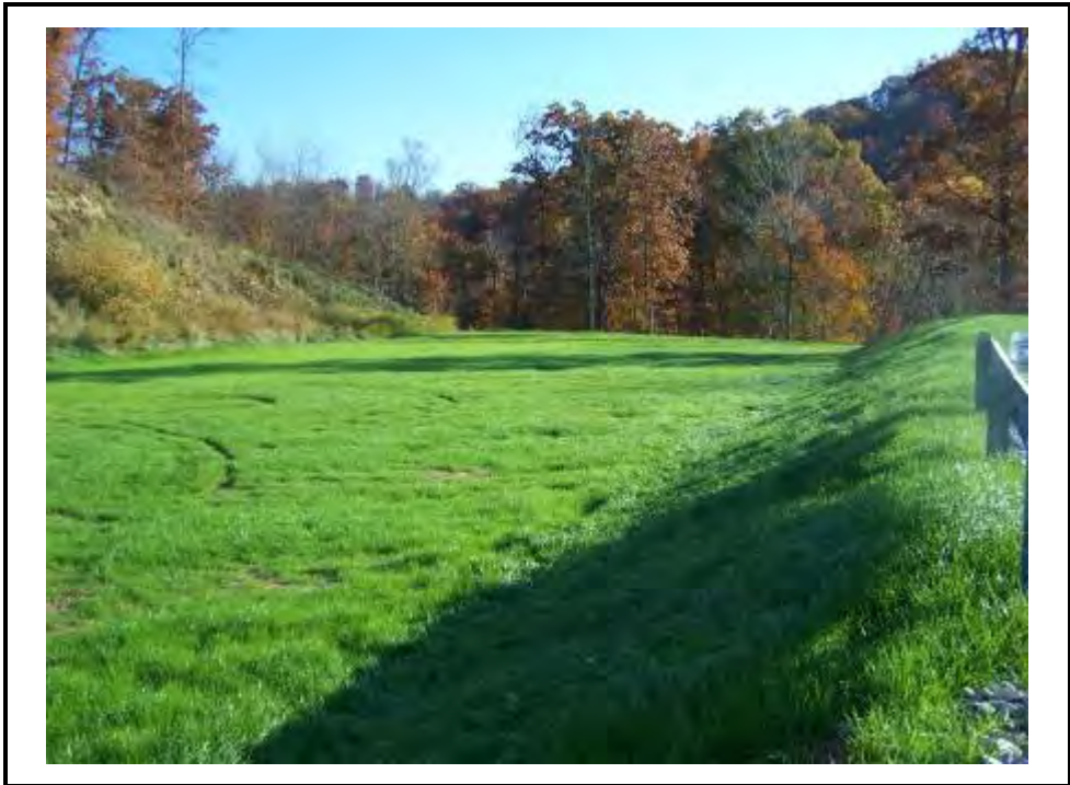
“New” emergency spillway at north abutment of Saddle Dam.
