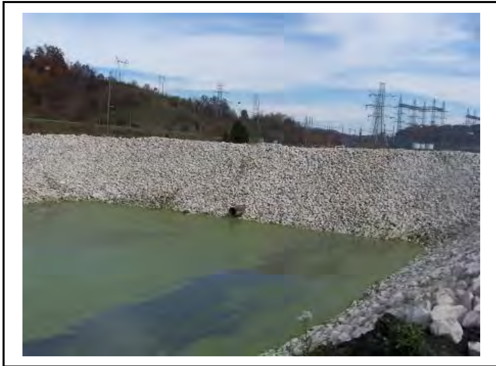
Discharge from South Bottom Ash Pond into South Clearwater Pond.
