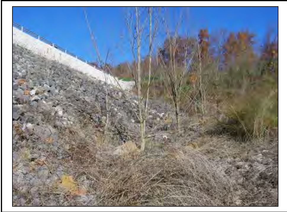
Close-up of trees in north downstream groin.
