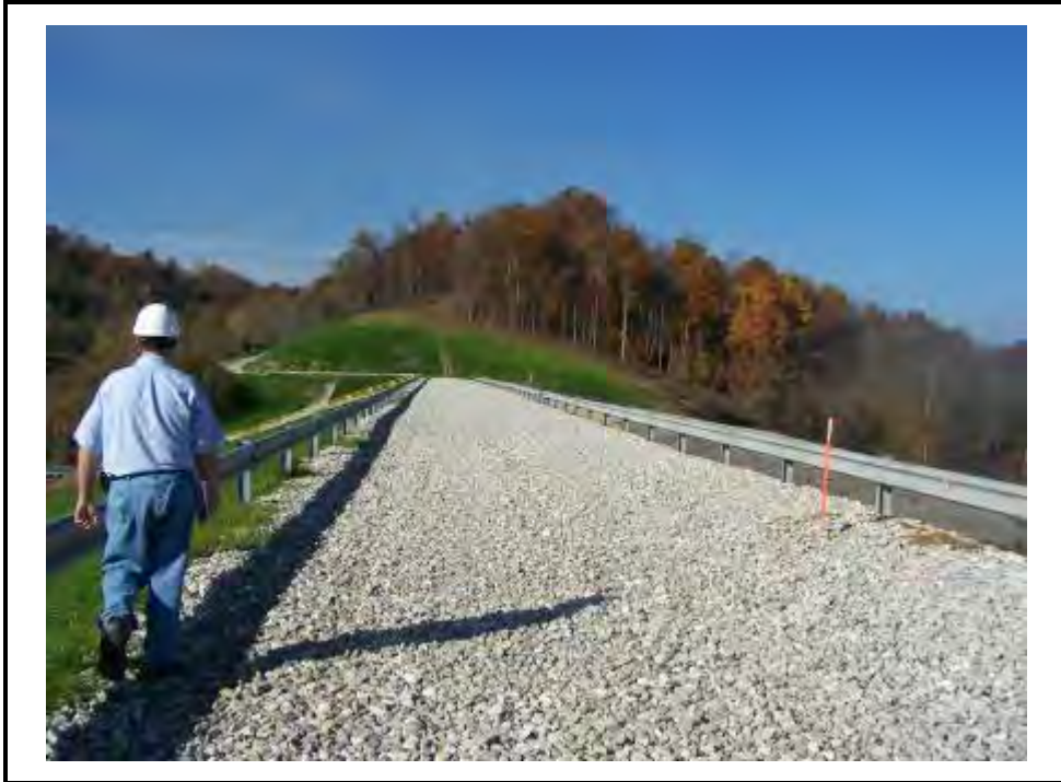
Crest of Horseford Creek Dam, looking east.
