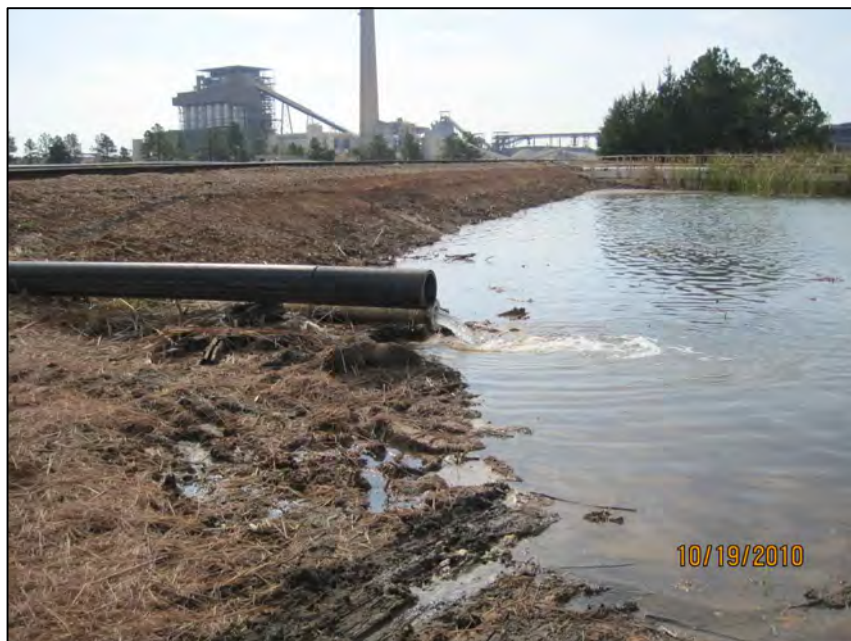
WAP-15 LOOKING SOUTH AT INFLUENT PIPE-NEUTRALIZED WASTE FROM DEMINERALIZER
