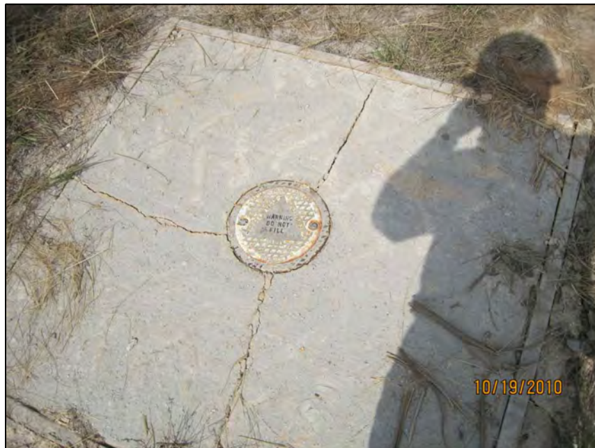
ASP-3 PIEZOMETER ON SOUTHWEST CORNER OF POND EMBANKMENT
