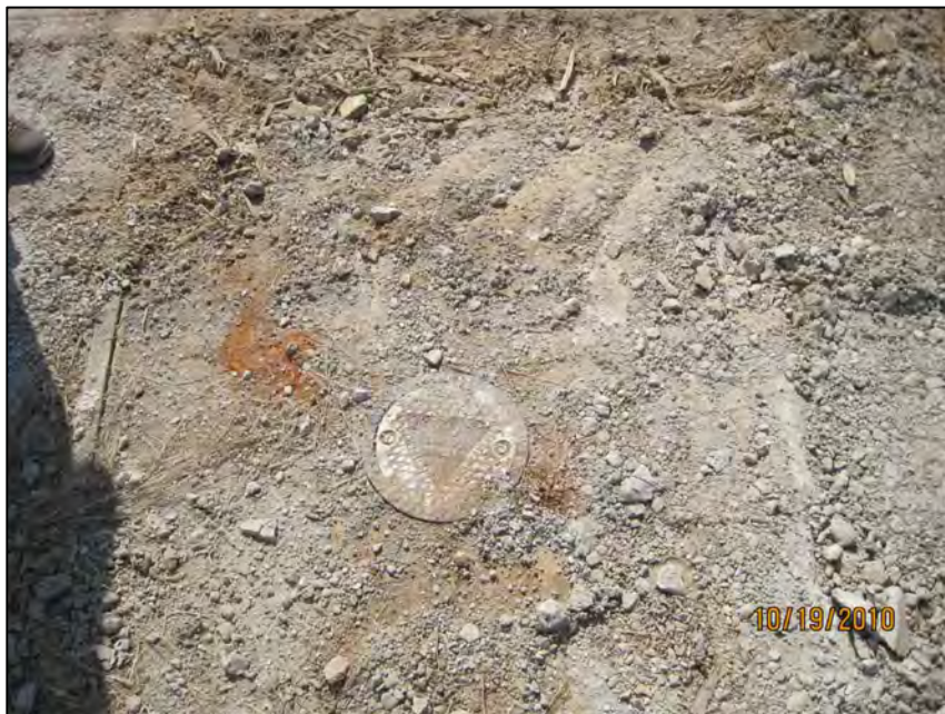
LRP-5 PIEZOMETER ON EMBANKMENT CREST
