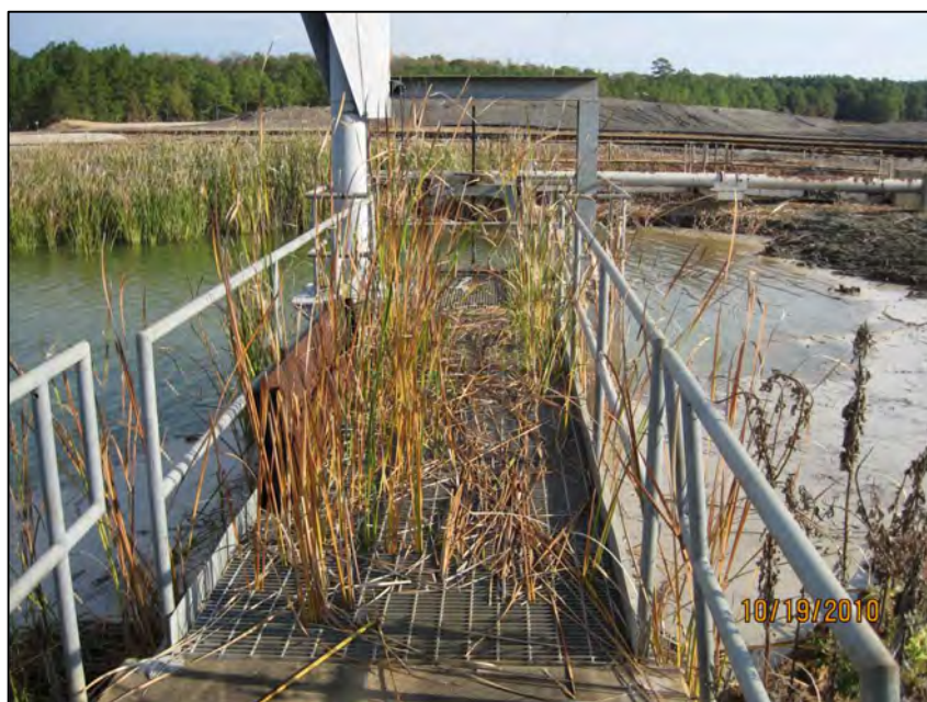
WAP-2 TOP OF DISCHARGE STRUCTURE
