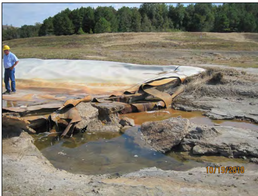
LRP-6 LOOKING EAST AT DOWNSTREAM DISCHARGE OF 60 ML HDPE LINED LANDFILL RUNOFF/LEACHATE CHANNEL
