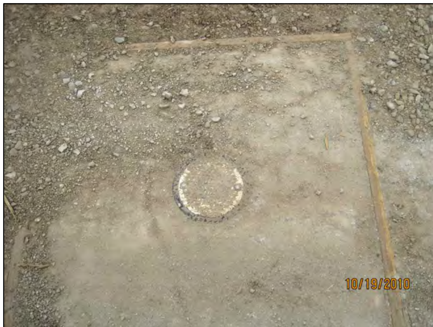
SAP-5 PIEZOMETER AT SOUTHWEST CORNER
