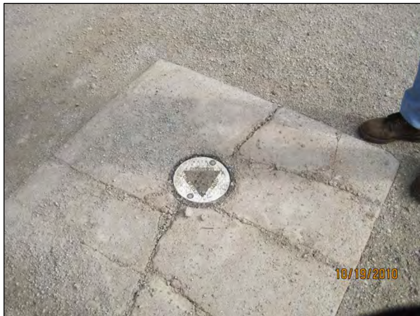
EAP-3 PIEZOMETER ON CREST OF NORTHERN EMBANKMENT
