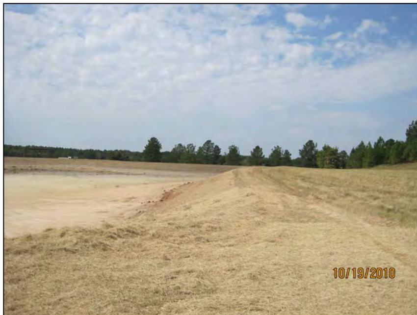
ASP-1 LOOKING WEST FROM NORTHEAST CORNER EMBANKMENT
