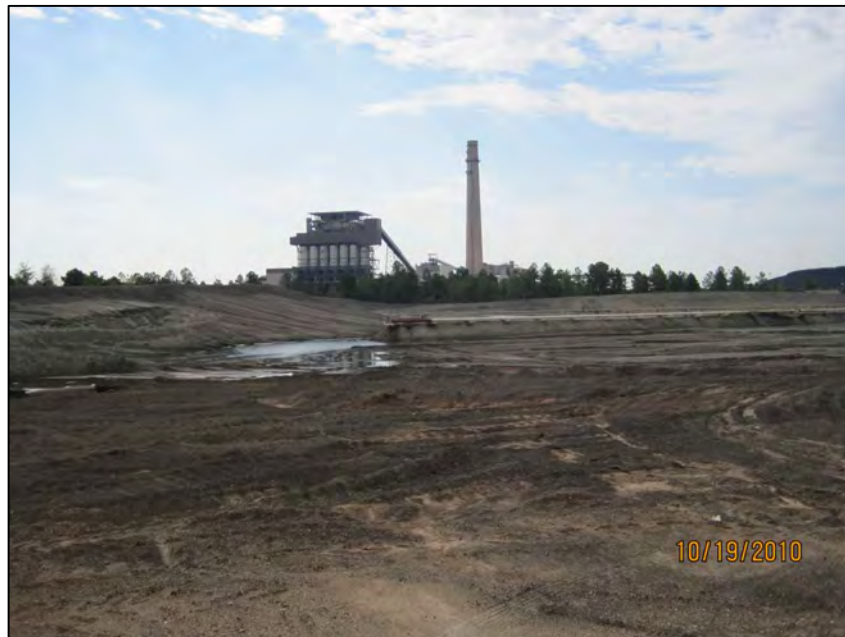
EAP-5 LOOKING SOUTH FROM NORTHERN EMBANKMENT
