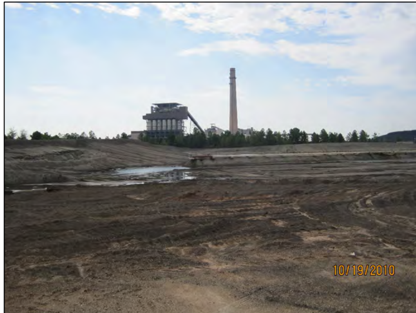
EAP-5 LOOKING SOUTH FROM NORTHERN EMBANKMENT
