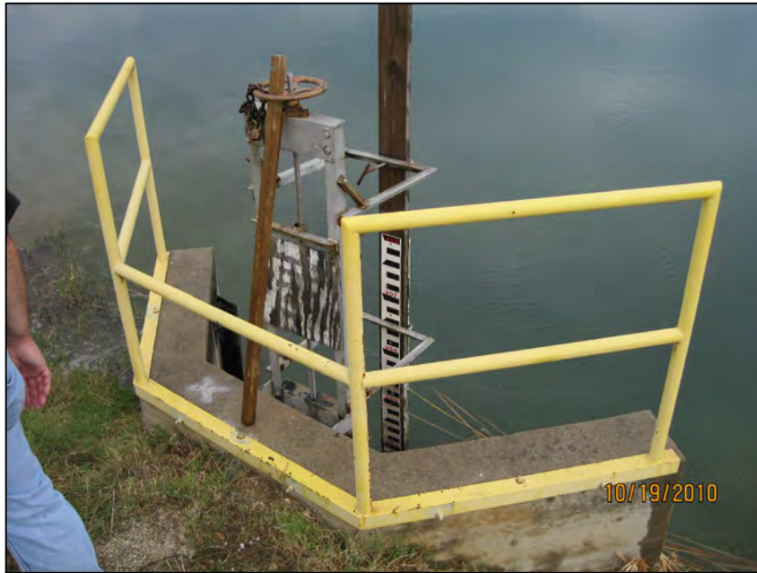
SAP-3 NPDES DISCHARGE OUTFALL 006 AT SOUTHWEST CORNER
