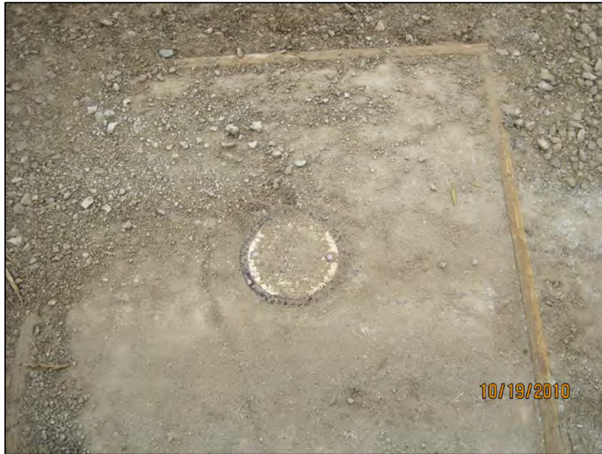
SAP-5 PIEZOMETER AT SOUTHWEST CORNER
