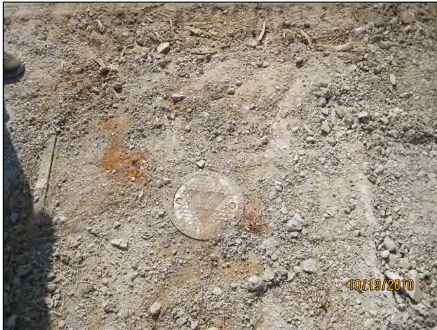
LRP-5 PIEZOMETER ON EMBANKMENT CREST
