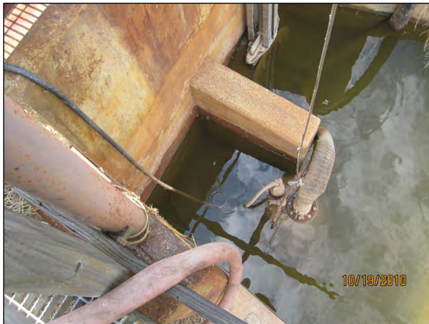
LRP-2 POND DISCHARGE STRUCTURE-NPDES OUTFALL 004
