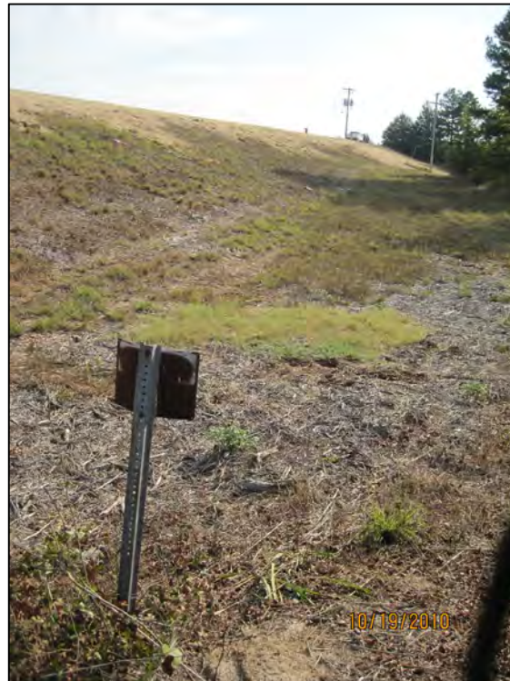
WAP-6 LOOKING EAST ON SOUTH DOWNSTREAM EMBANKMENT
