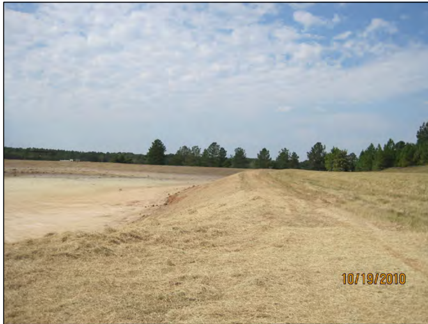
ASP-1 LOOKING WEST FROM NORTHEAST CORNER EMBANKMENT
