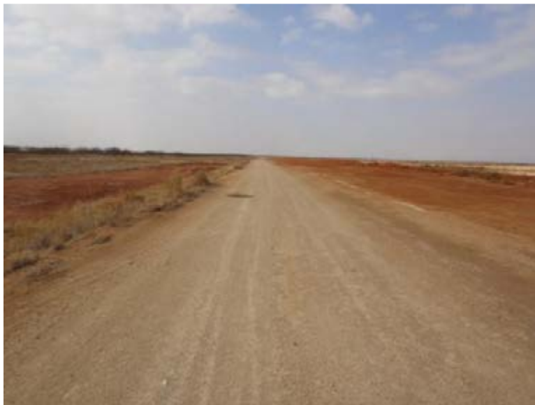
Figure 5.2.1-1. Figure showing the South Embankment crest and outside slope conditions.
