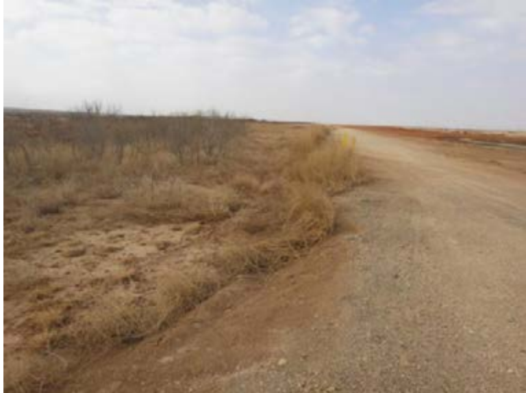
Figure 5.2.3-1 general good condition of the outside slope of the South Embankment.
