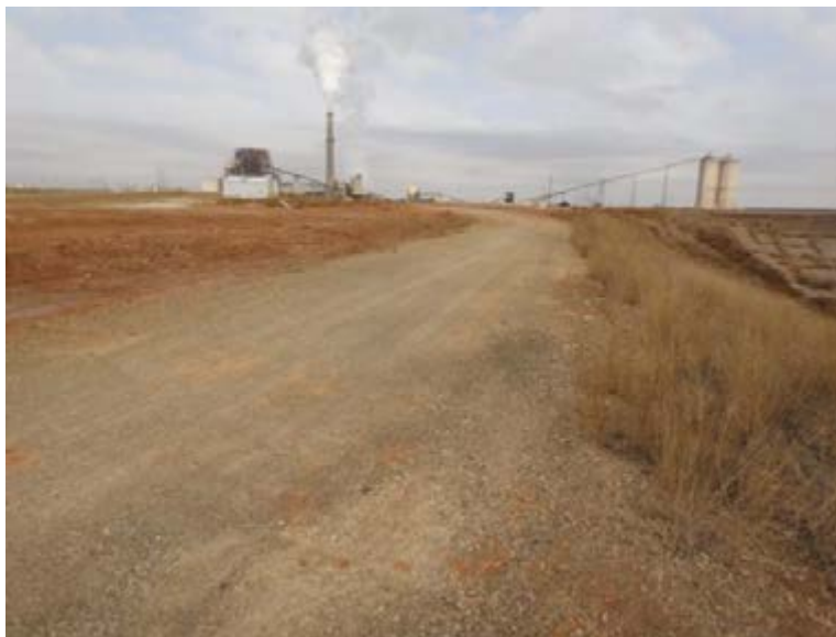
Figure 5.3.1-1. Figure showing the East Embankment crest and outside slope conditions.
