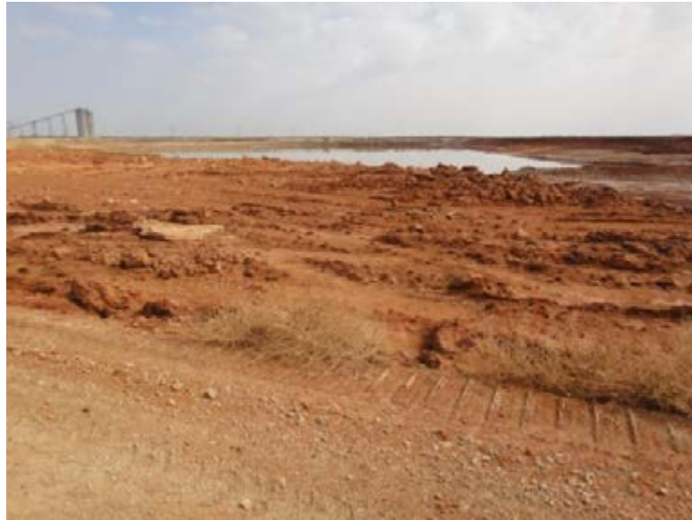
Figure 5.2.2-1. Figure showing the South Embankment lack of inside slope.
