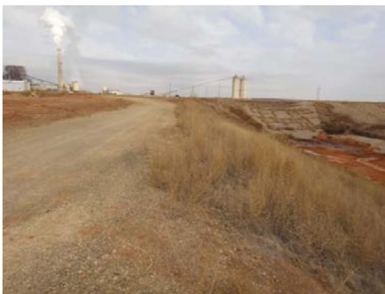
Figure 5.3.3-1. Crest, outside slope and groin of East Embankment.
