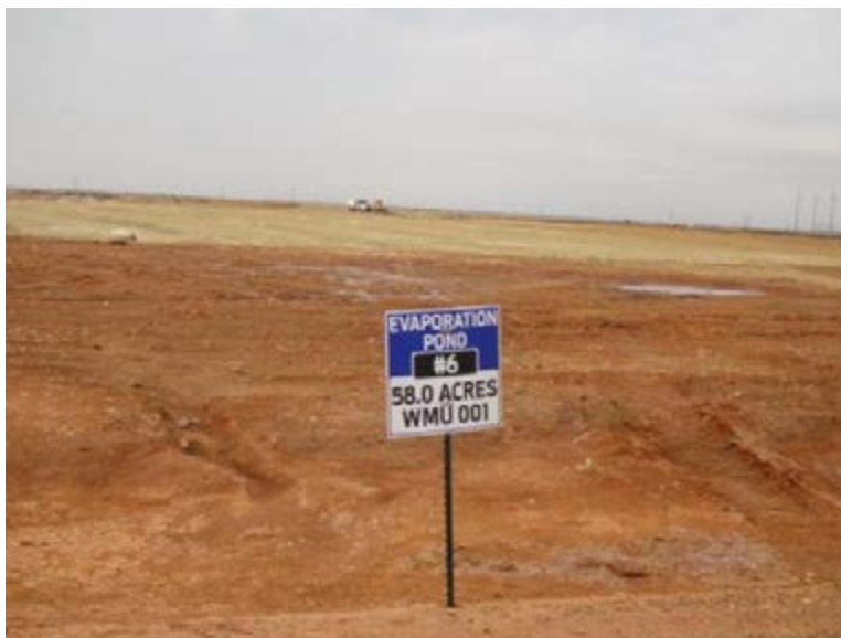
Figure 5.3.2-1. East Embankment, lack of inside slope.
