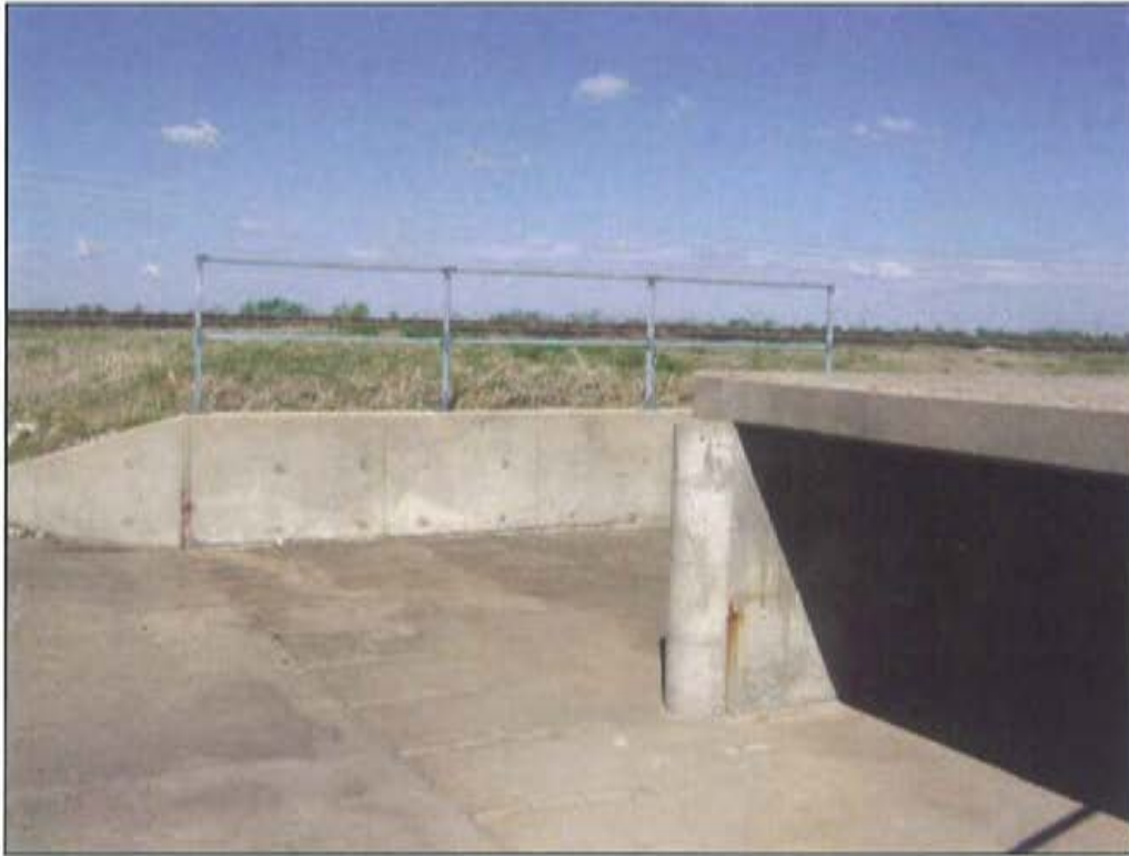
Figure 5 - Bottom Ash Pond Spillway
