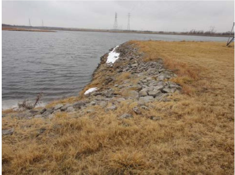
Figure 5.3.2-1. South Embankment inside slope condition.
