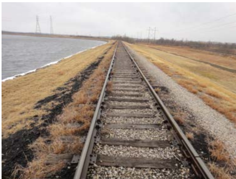
Figure 5.2.1-1. Photo showing railroad on crest and vegetation on the inside slope of West Embankment.
