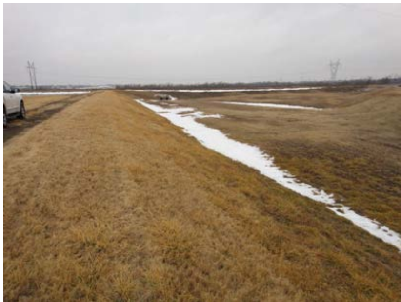
Figure 5.4.3-1. Outside slope of North Embankment.
