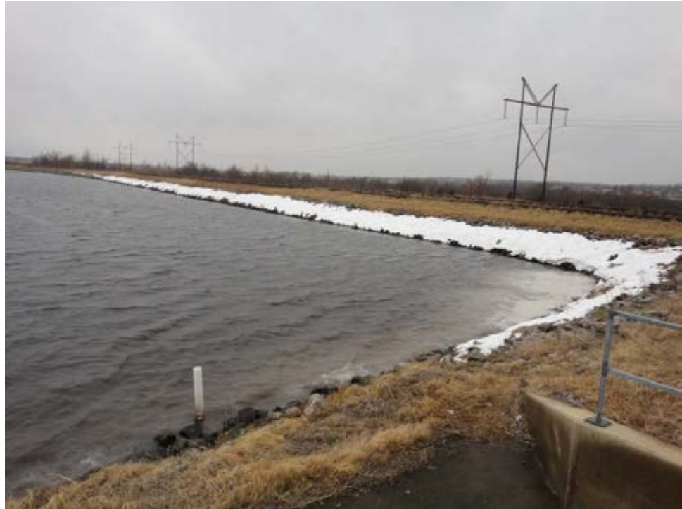
Figure 5.2.2-1. Inside slope grass and riprap
