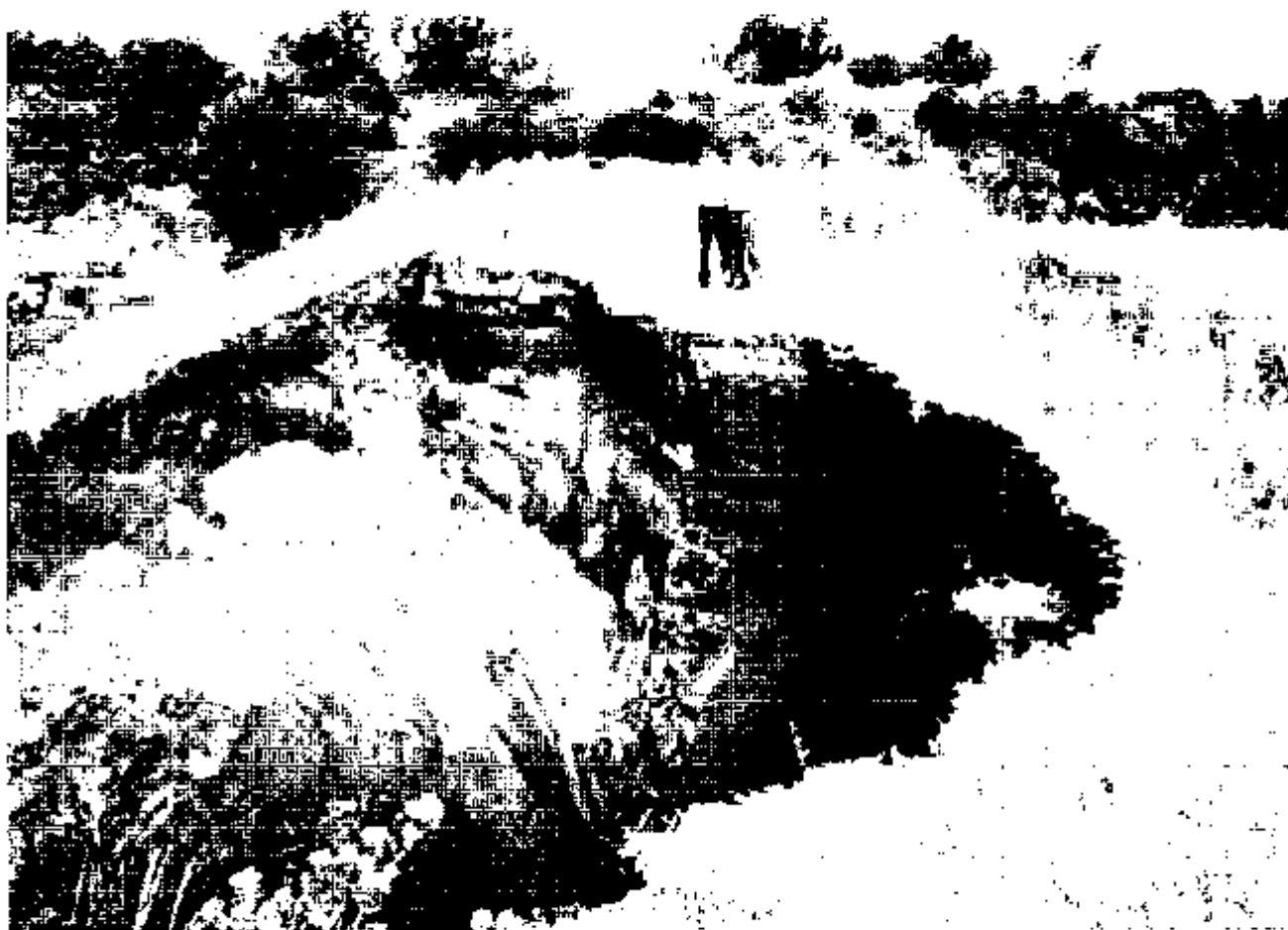
SCS Sugar Creek Site # 44 dam, Caddo Cnty, OK washed out from heavy rains - 2007
