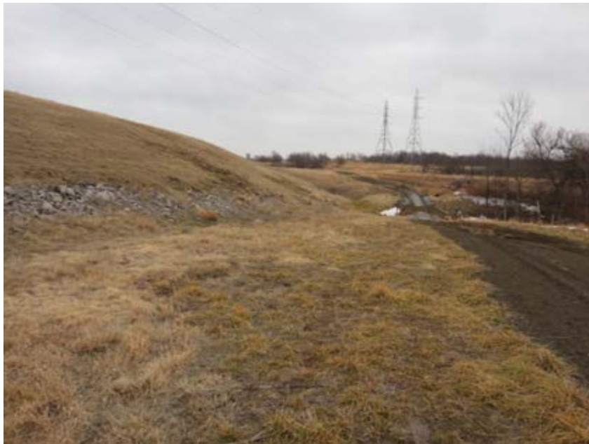
Figure 5.3.3-1. Condition of South Embankment outside slope and toe.
