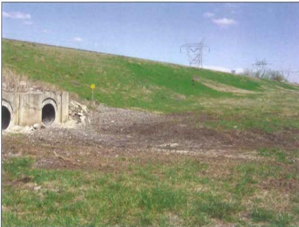
Figure 6 - Downstream Basin with Culverts
