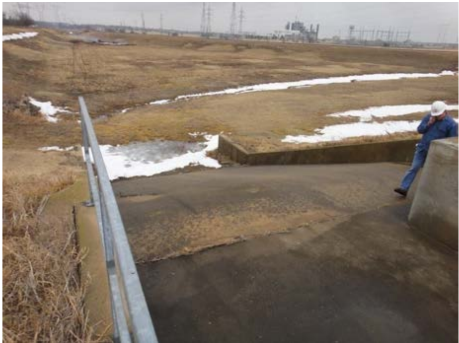
Figure 5.5.1-2. Downstream view of Overflow Structure.
