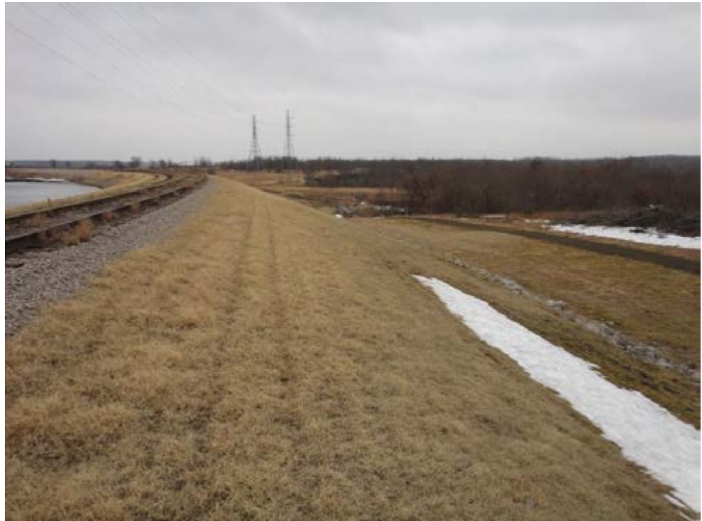
Figure 5.3.1-1. Figure showing the South Embankment crest condition.
