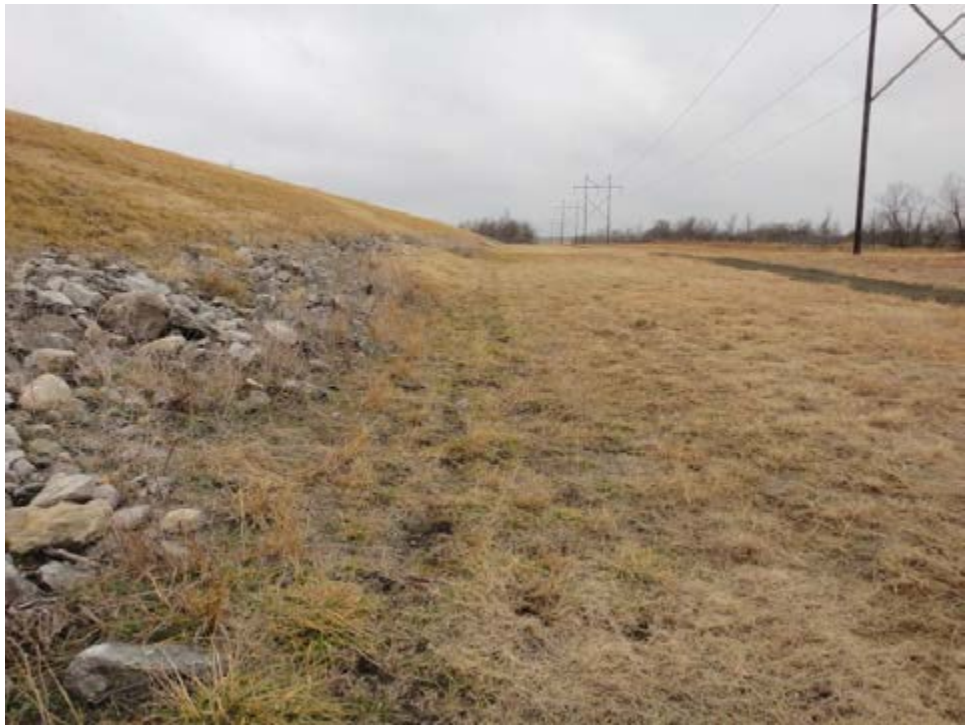
Figure 5.2.3-2. West Embankment toe conditions.
