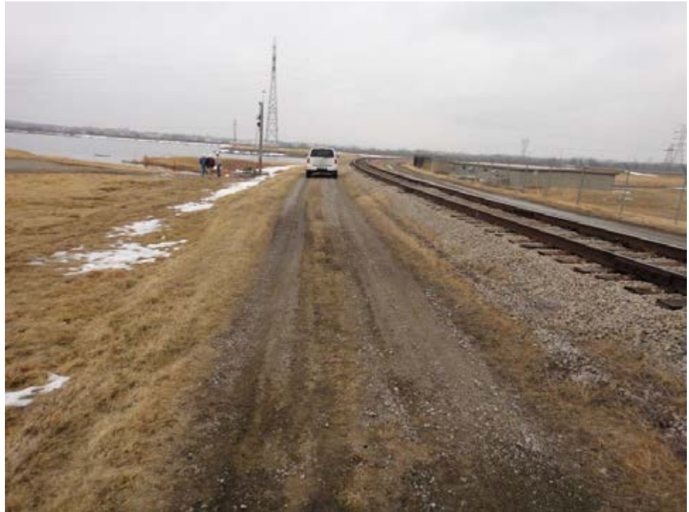
Figure 5.4.1-1. North embankment crest with two access roads and railroad track at the east end
