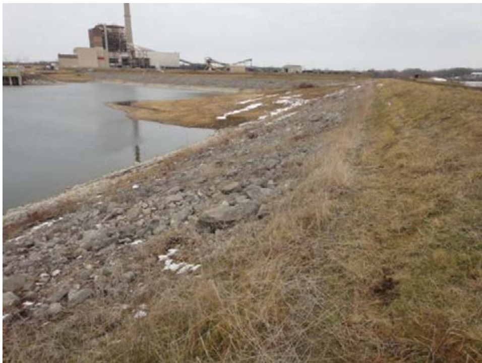
Figure 5.2.3-1: General condition of the west dike outside slope and groin
