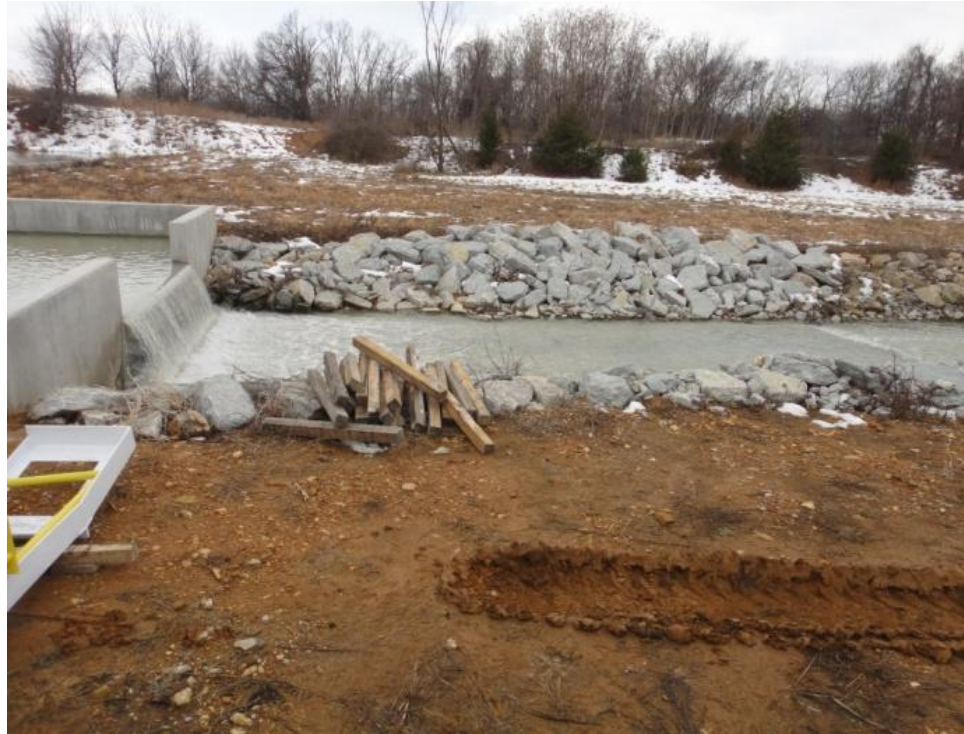
Figure 5.4.2-1. Water discharging from the main spillway outfall
