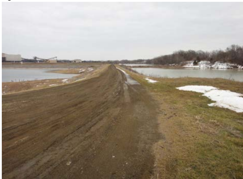
Figure 5.2.1-1: Photo Showing Crest, West Dike
