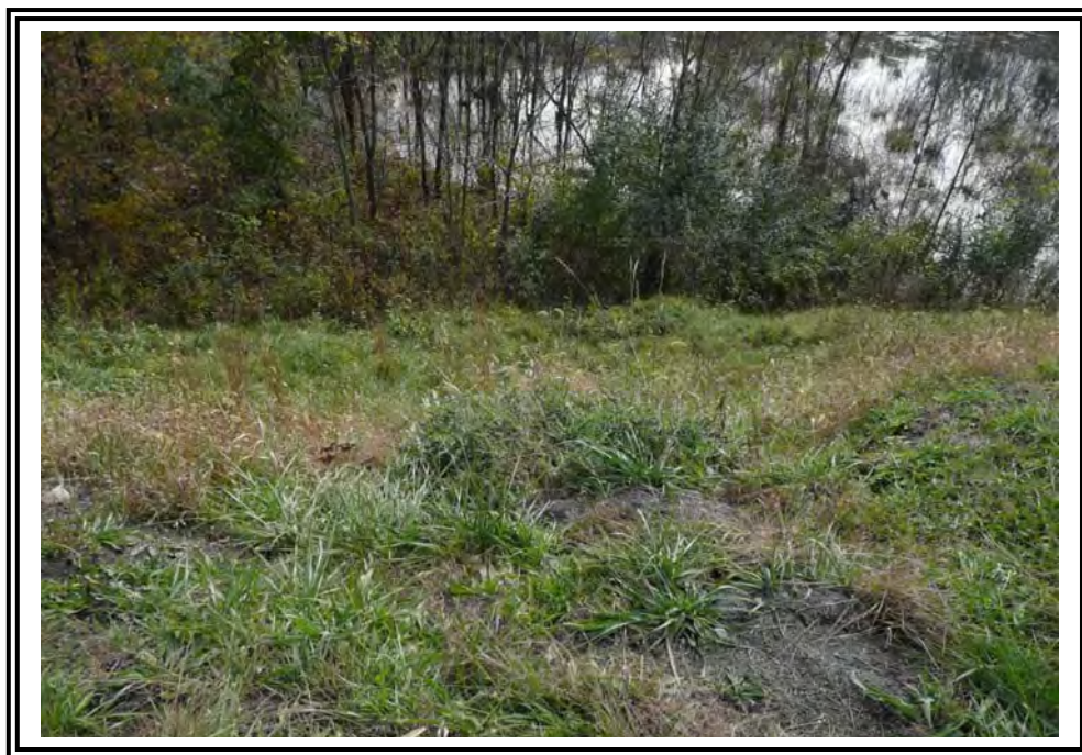
Example of soil and coal dust transport and intermittent grass cover loss near crest of Coal Haul Road Dike.
