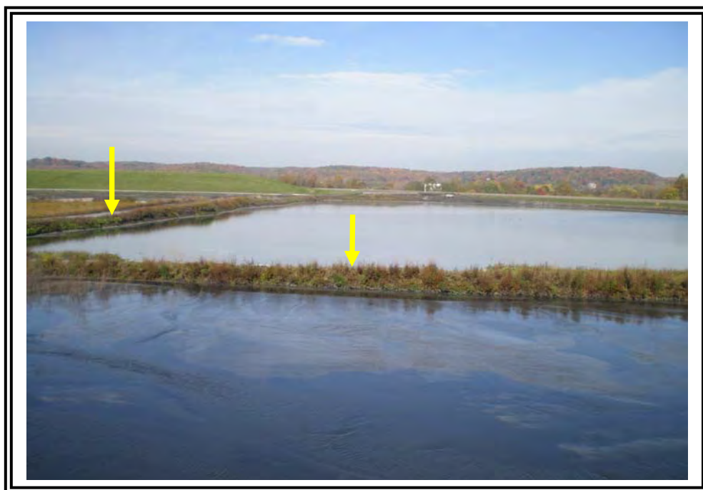
Closer view of interior divider dikes (see arrows) the Fly Ash Storage Area and Central Fly Ash Pond area.
