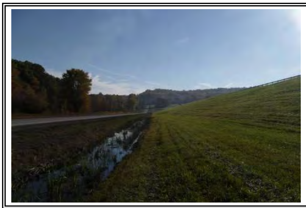
Toe of the North Haul Road Dike, looking east. Standing water in the road ditch along toe can be seen in left of photo.
