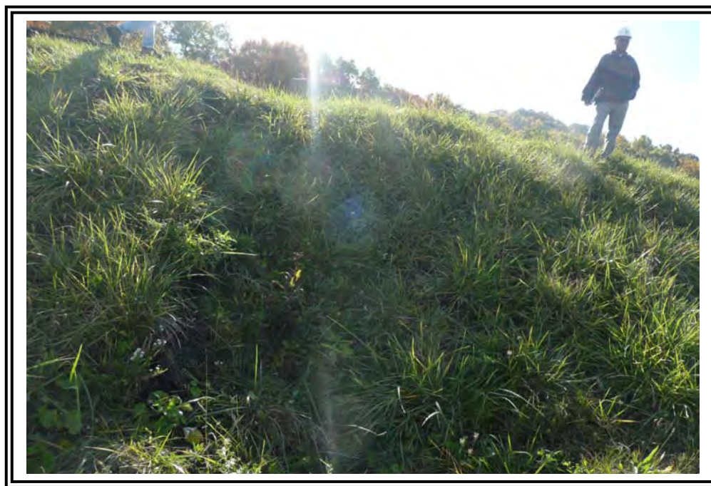
Grassed older erosion rill in upstream slope of Coal Haul Road Dike.
