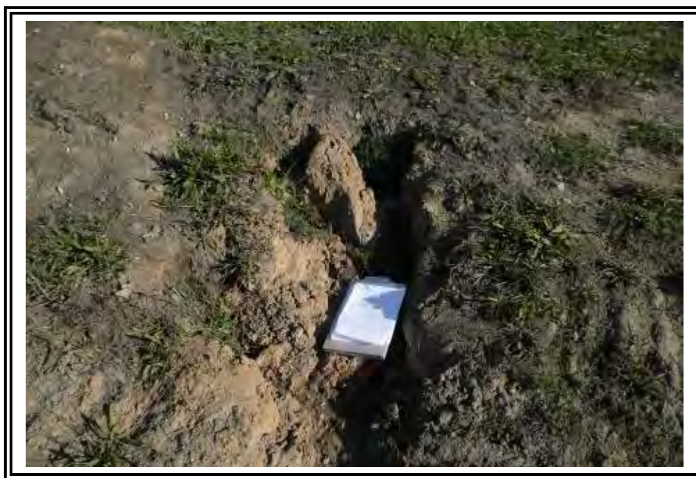
A close up of a large erosion rill and loss of vegetation on the upstream slope of the North Haul Road Dike.
