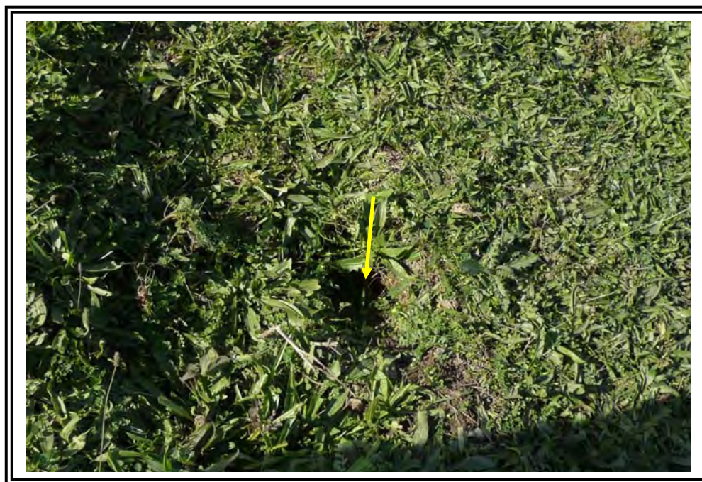
Collapsed, vegetated rodent burrow on upstream slope of Southwest Dike, likely abandoned (See arrow).
