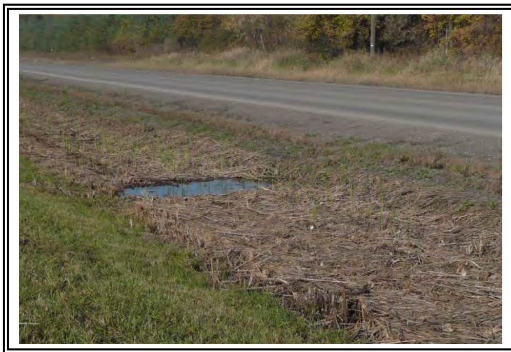
Recently mowed cattail growth in drainage swale at toe of the North Haul Road Dike and County Route 273.
