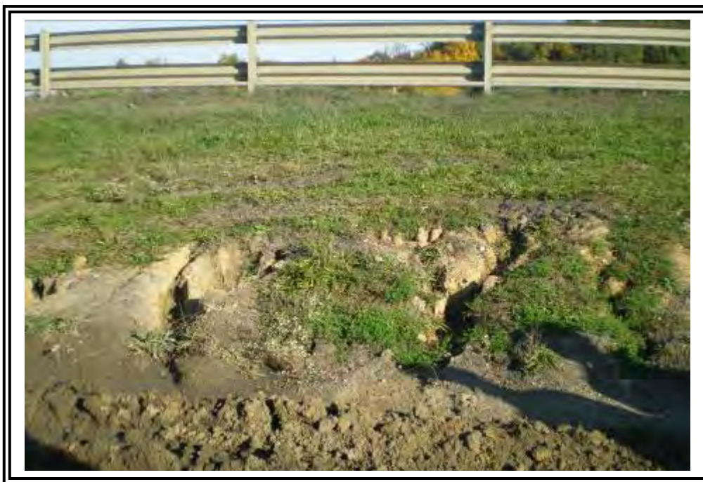
Erosion rills from haul road run off on the upstream slope of the North Haul Road Dike.
