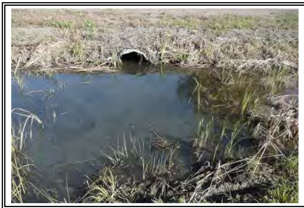
Close up of the half submerged drainage pipe under the county road.
