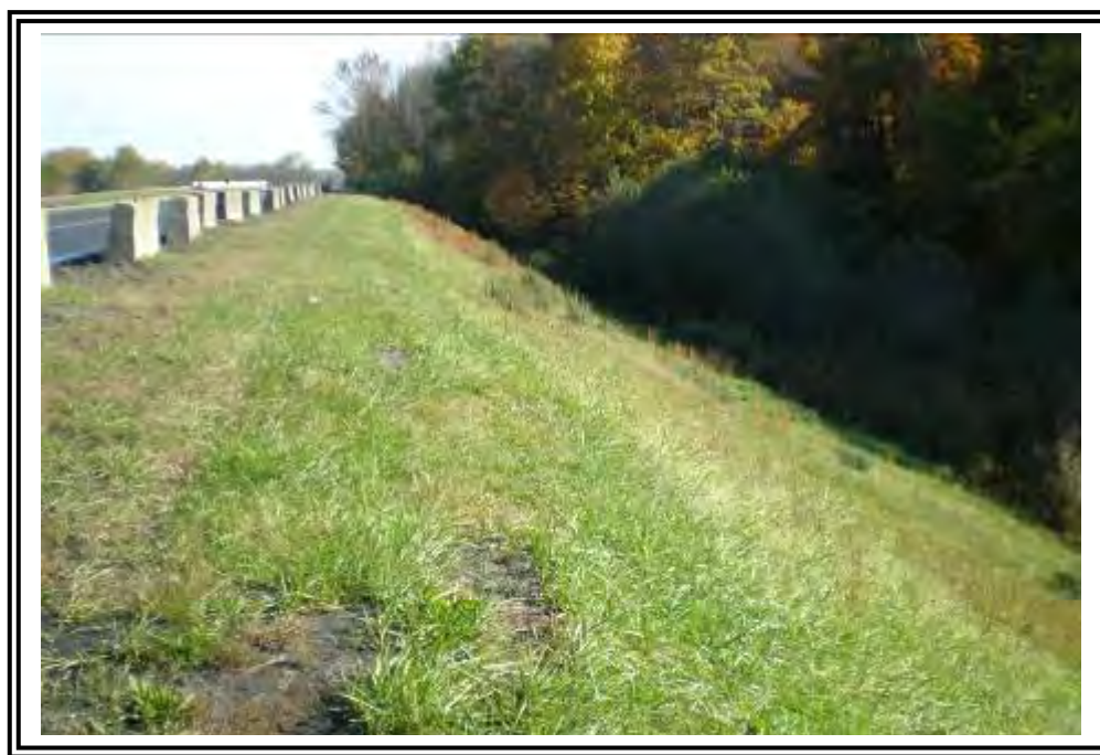
Looking northeast along downstream slope of the Coal Haul Road Dike. Small trees and moderate vegetation lower on the slope can be seen in the shade in the right of the photo.
