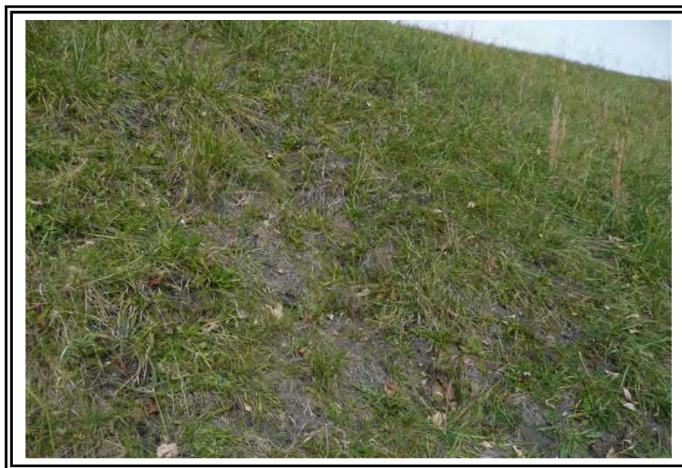
Soil and coal dust transport with intermittent grass cover loss on downstream slope of Coal Haul Road Dike.
