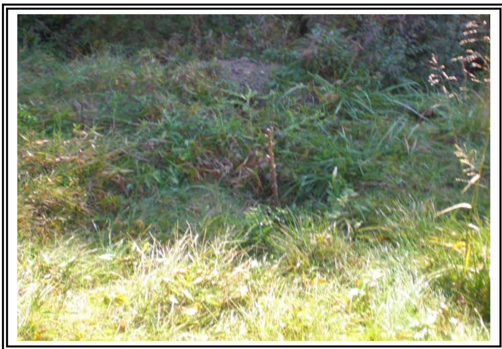
Open rodent burrow in area of older collapsed burrows that have become erosion rills (stick is in burrow) in Coal Haul Road Dike.
