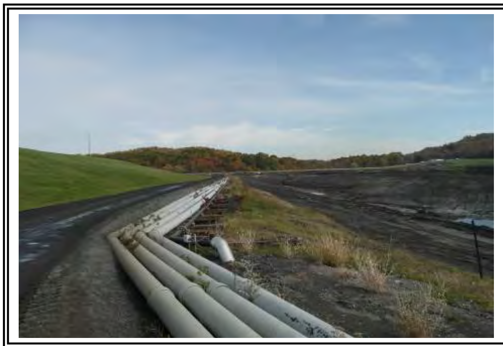
Sluice lines running to the Fly Ash Pond along the western side of the complex.
