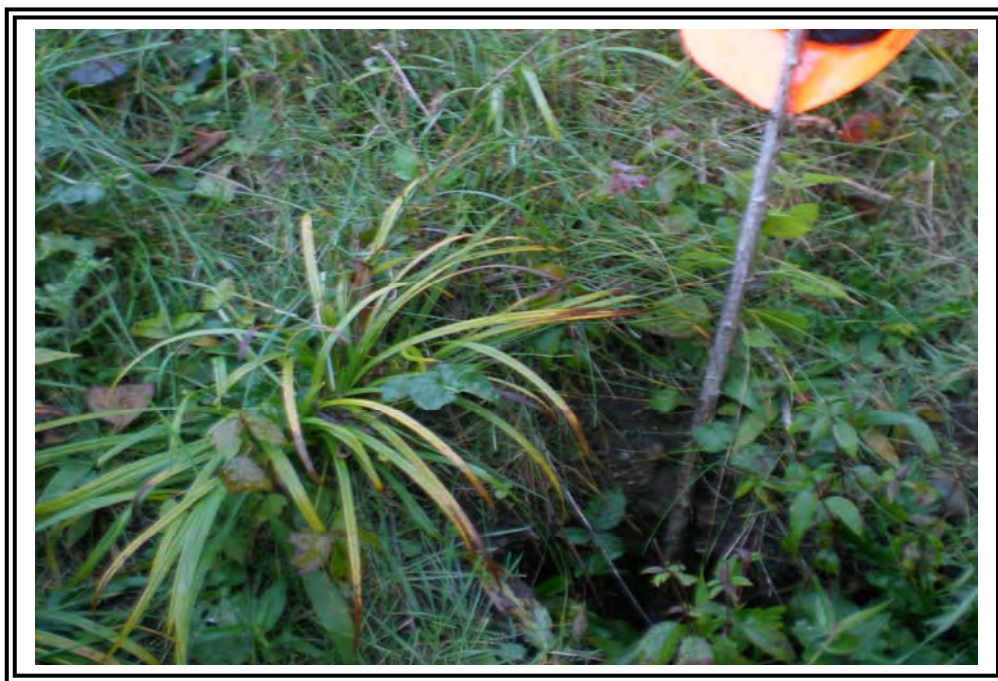
Another rodent burrow on downstream slope of Coal Haul Road Dike.
