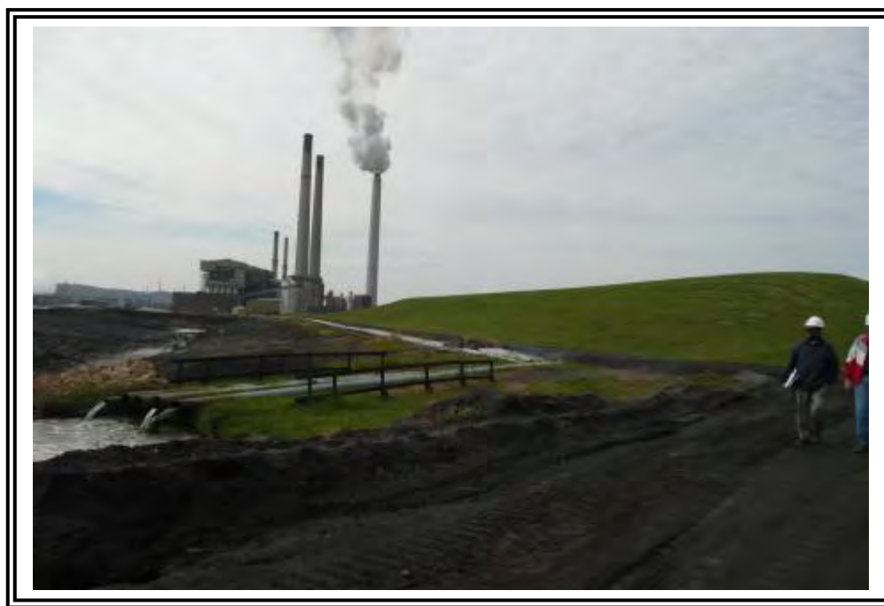
Sluice lines running into the Fly Ash Pond.
