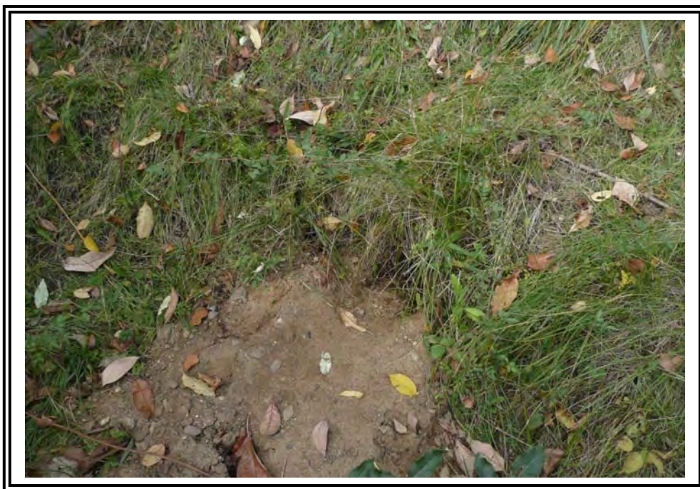
More recent rodent burrow in Coal Haul Road Dike with exposed soil spoil.
