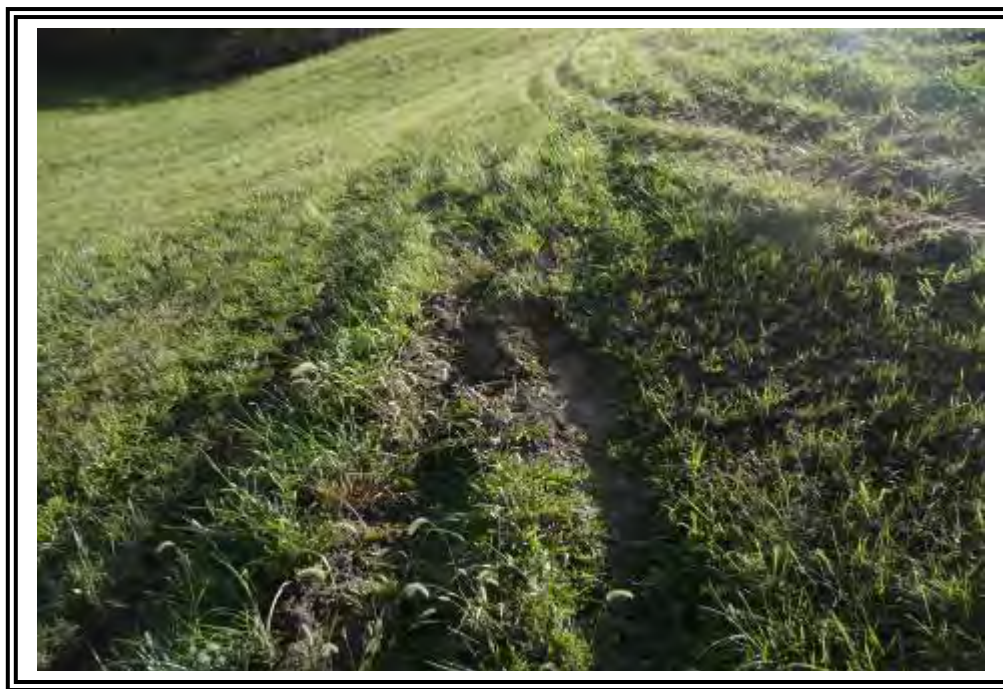
Close up of rutting and loss of vegetation on the downstream slope of the North Haul Road Dike.
