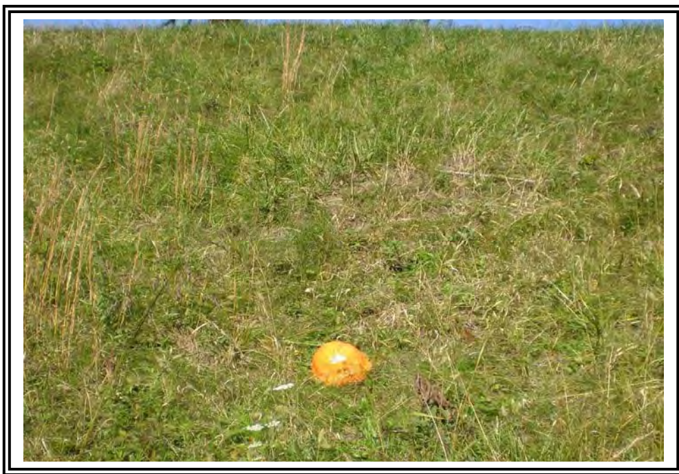
Grassed erosion rill on downstream slope of Coal Haul Road Dike. Hard hat is in bottom of rill.
