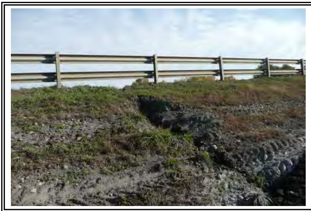
Large erosion rill and rutting on the upstream slope of the North Haul Road Dike.
