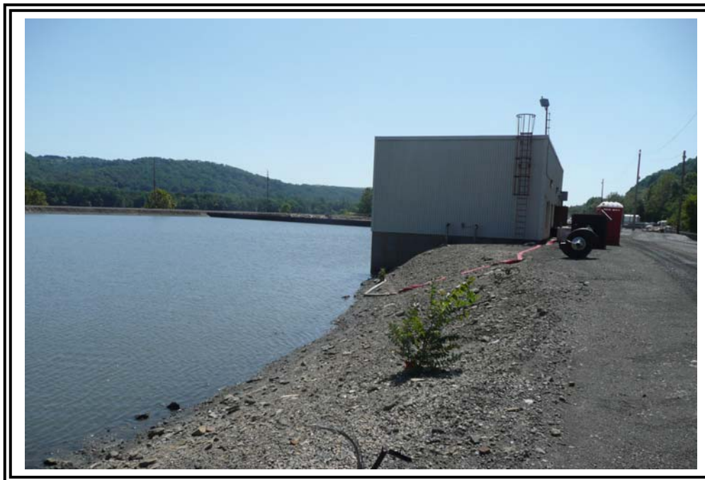
Upstream slope and crest on west dike adjacent to pump house, looking south. Slope is fairly gentle but steepens adjacent to pump house.
