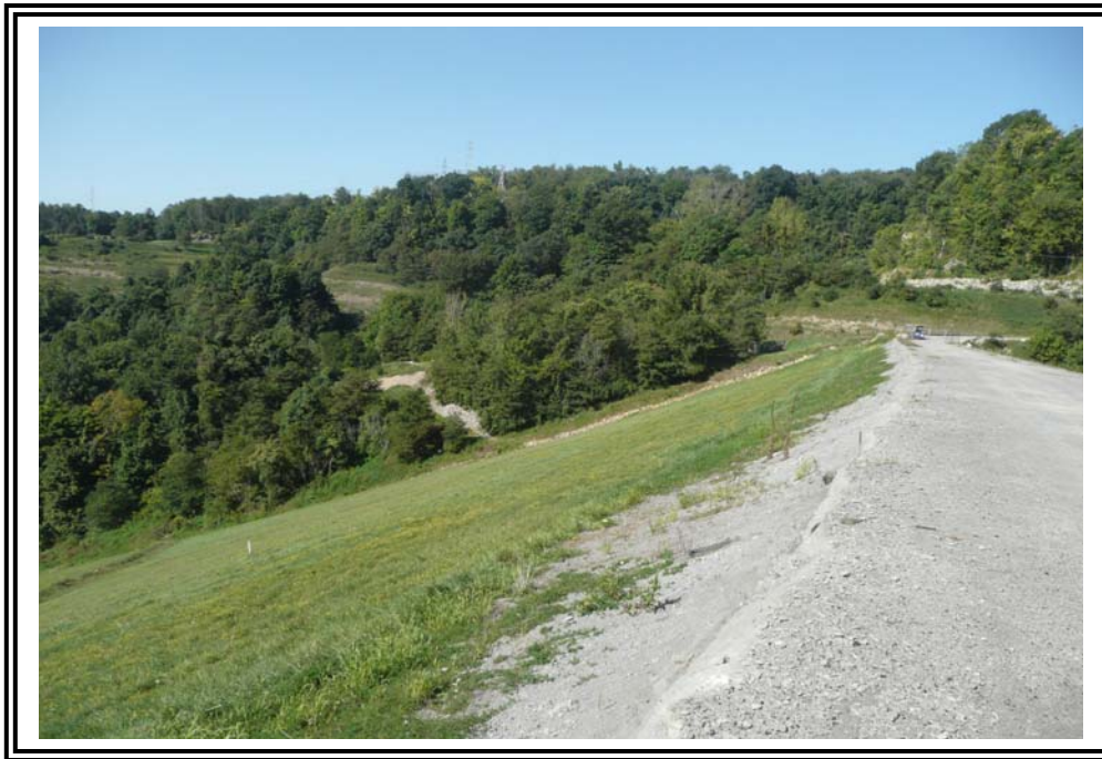
Downstream slope at crest looking west toward right abutment.
