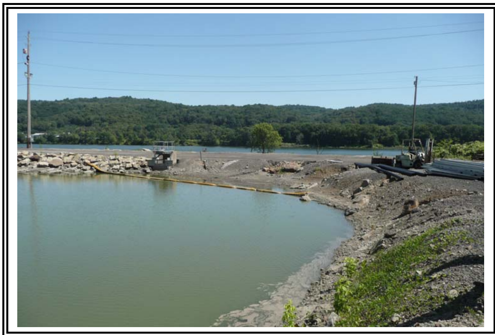
Looking east at upstream face of east dike. Note large armor stone adjacent to outlet structure and large erosion gullies adjacent to equipment at south wall - east dike interface.
