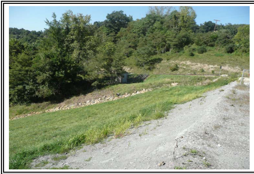
Closer view of rock groin at right (west) abutment hillside contact from crest.
