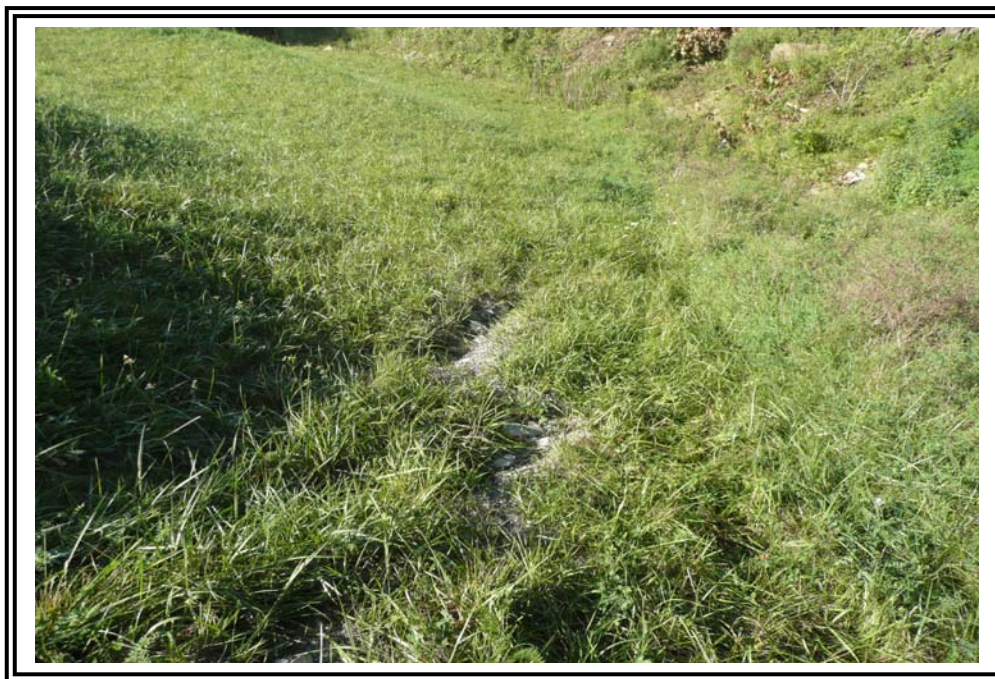
Erosion feature on downstream slope next to west groin at upper bench.
