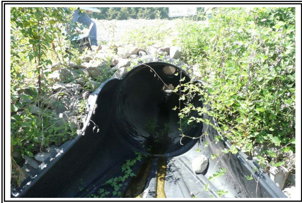
36" diameter Recirculation Pond outfall.
