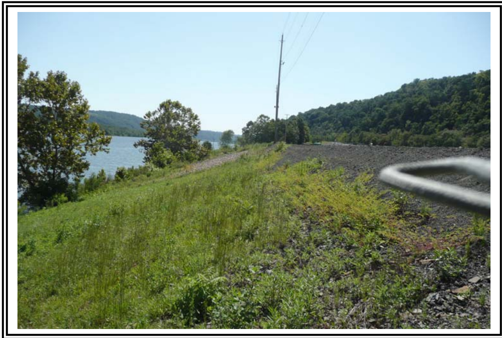
Downstream slope of east dike, looking south showing typical vegetation cover.
