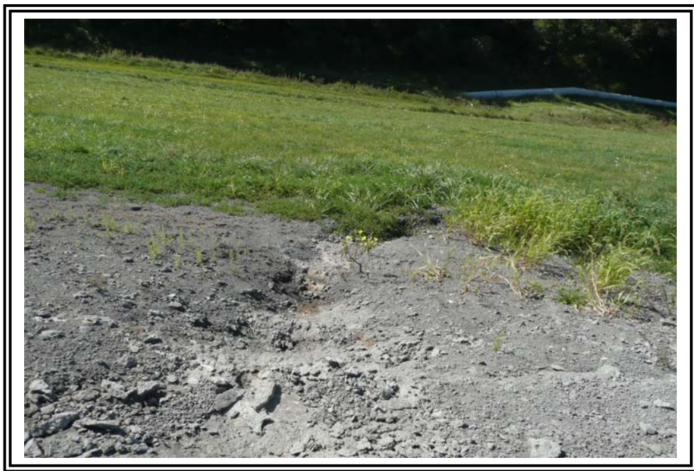
Example of weathering and erosion in RCC material.
