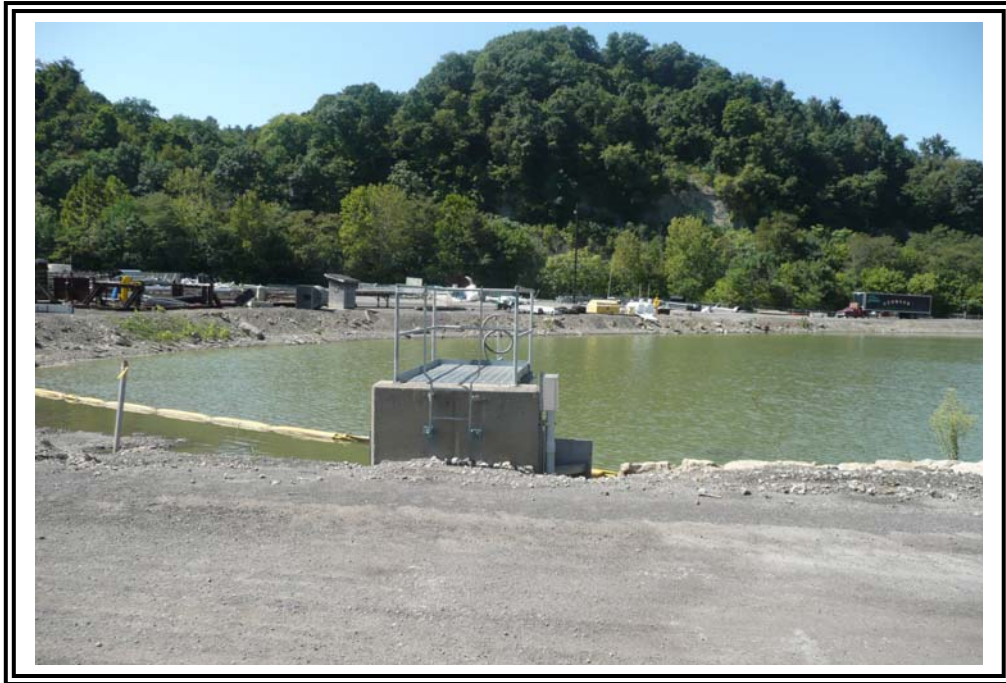
Recirculation pond outlet structure from east dike crest, looking west.
