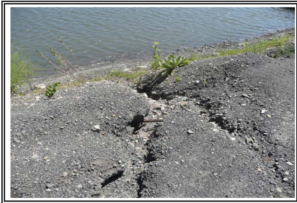
Closer look at erosion feature in Photo #36. Note exposed rebar debris in erosion gully.
