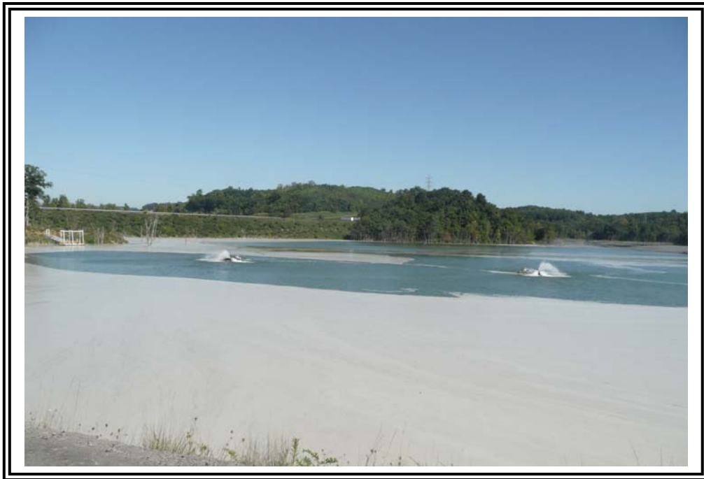
Looking north from crest across the reservoir at Fly Ash Dam No. 1.
