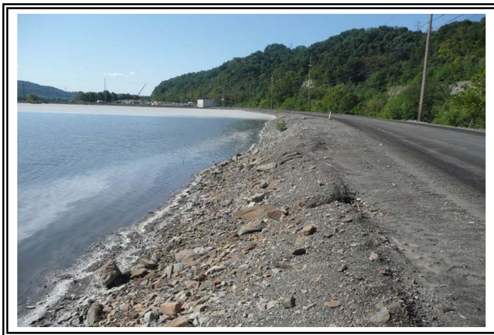
Upstream slope of the west dike, looking south. Note erosion at crest and sparse vegetation in background.
