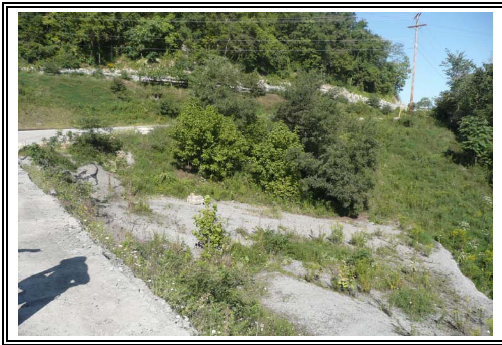
On crest looking west at abutment on upstream side.
