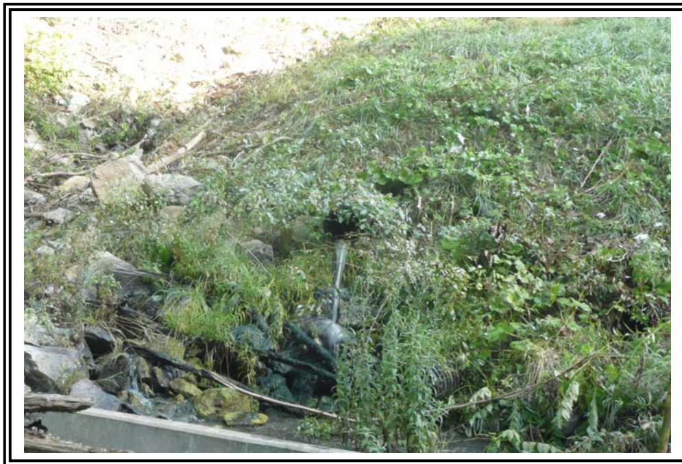
Closer view of seepage discharge.
