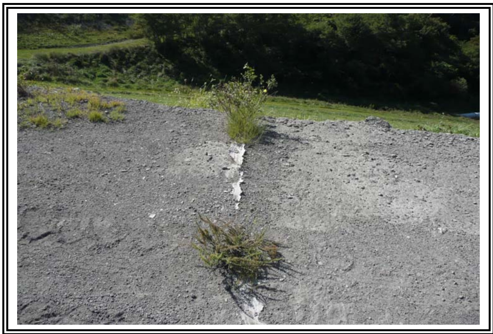
Surface expression of sealed crack at crest in RCC that initiated the diagonal joint in the inclined spillway.
