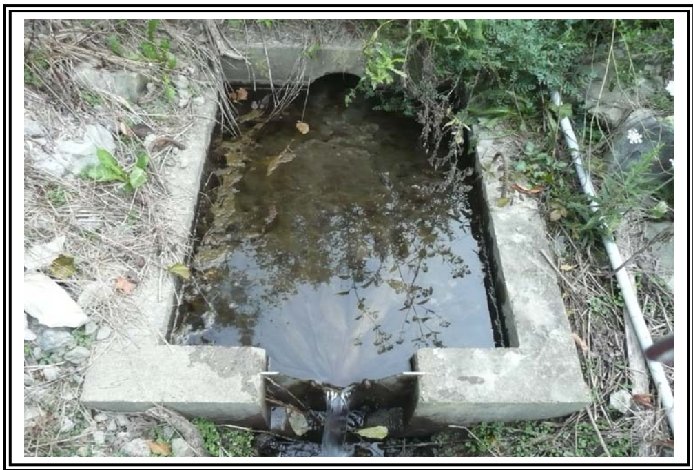
V-notch weir at original (Pre RCC) toe drain.
