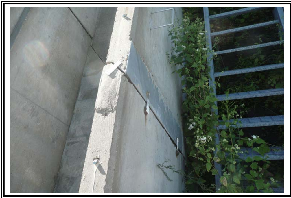
Close-up of crack gauges on inclined spillway diagonal joint.
