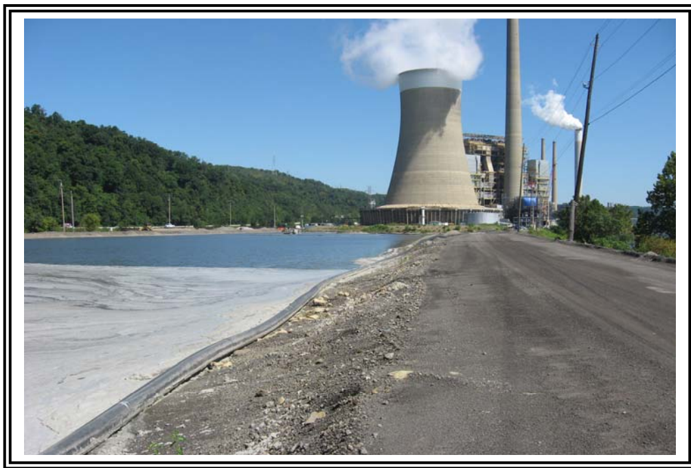
Upstream slope and crest alignment of east dike, looking north.
