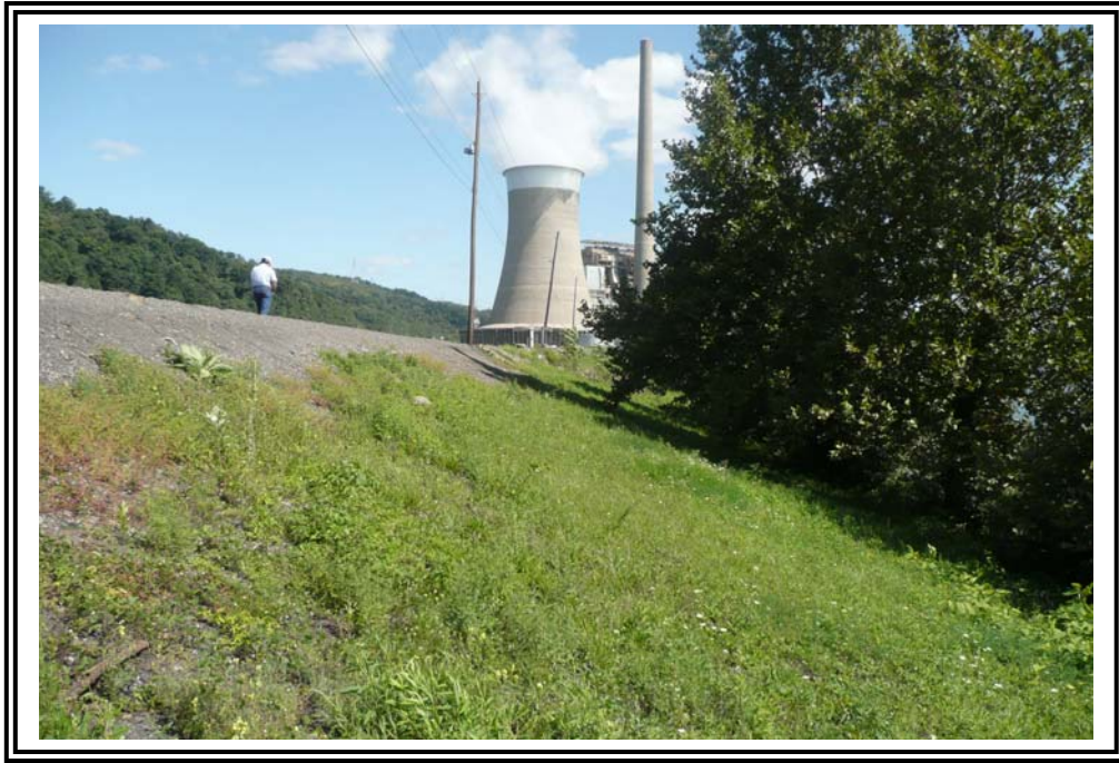
Downstream slope of east dike, looking north, showing effect of routine grading activities at the crest where vegetation is not established.
