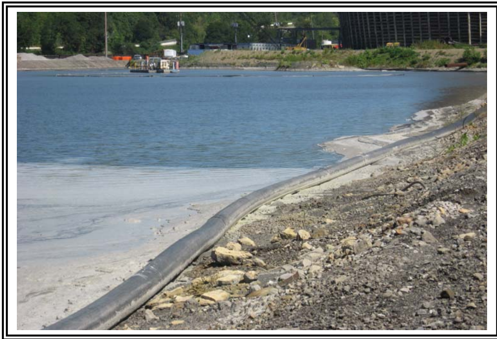
Closer view of upstream slope of east dike, looking north.
