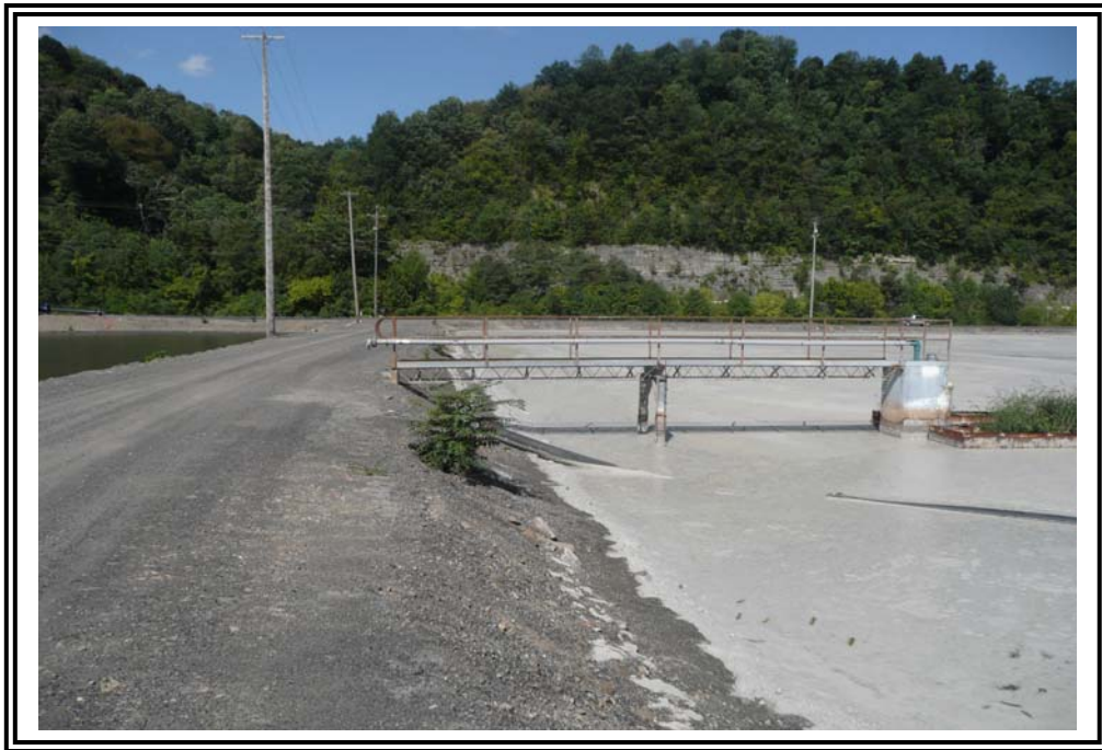
Upstream slope and crest of separator dike, looking west. Note isolated vegetation.
