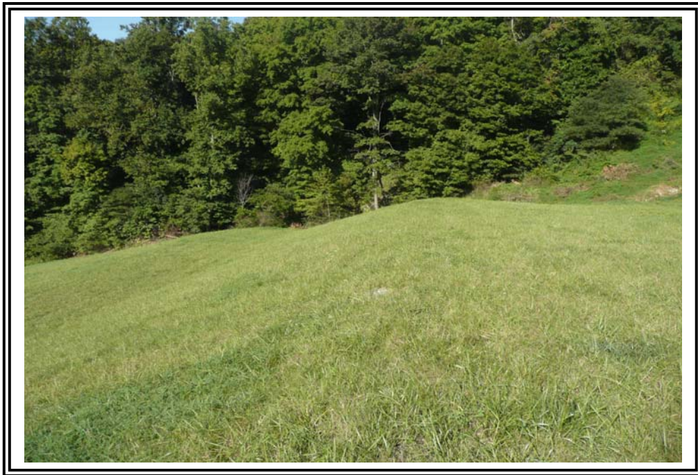
Downstream slope looking west at crest of upper bench.
