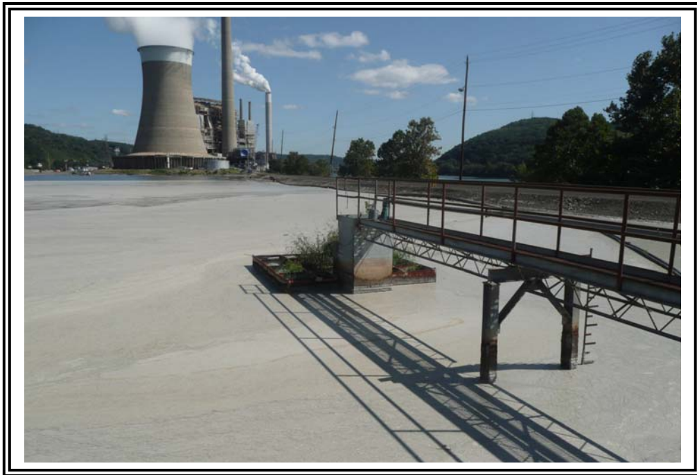
Pond spillway tower looking north.
