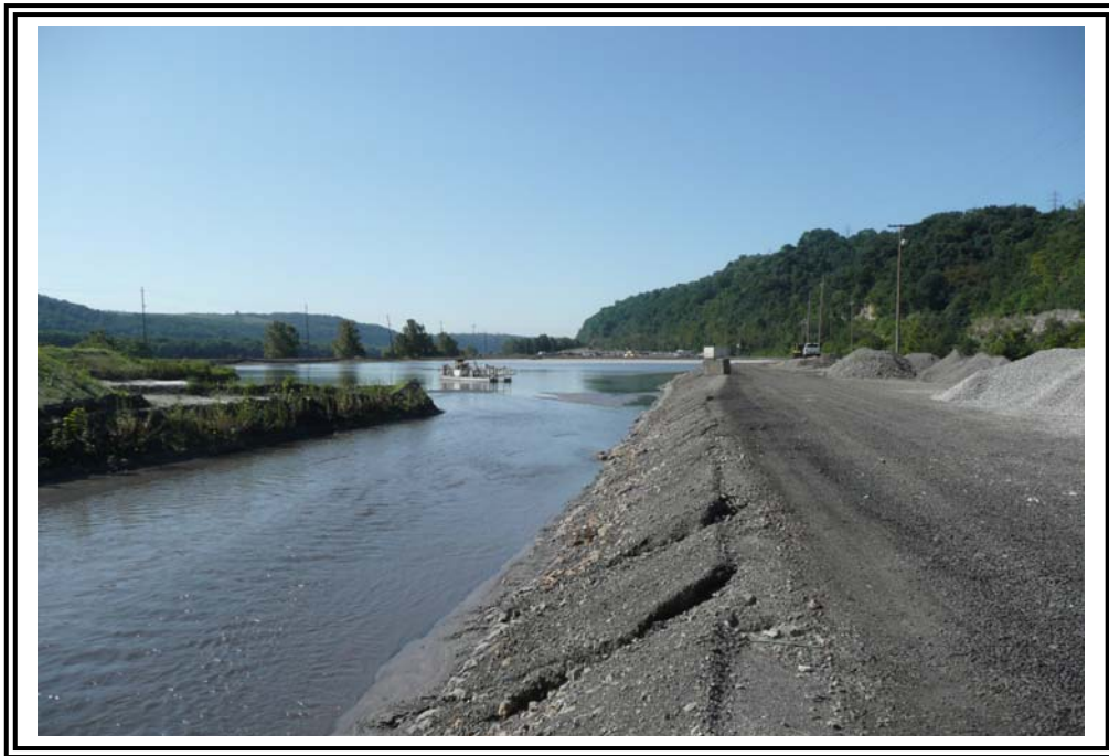
Upstream slope and crest of west dike looking south. Note erosion rills in granular surface
