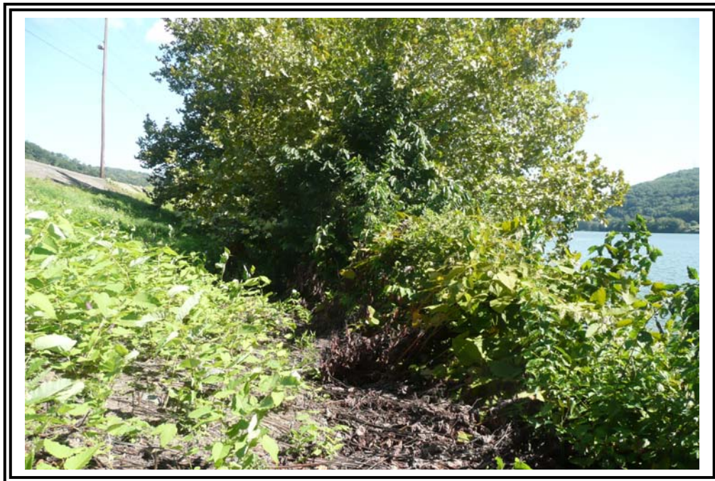
Downstream toe of east dike showing change in vegetation at slope toe-river bank contact.
