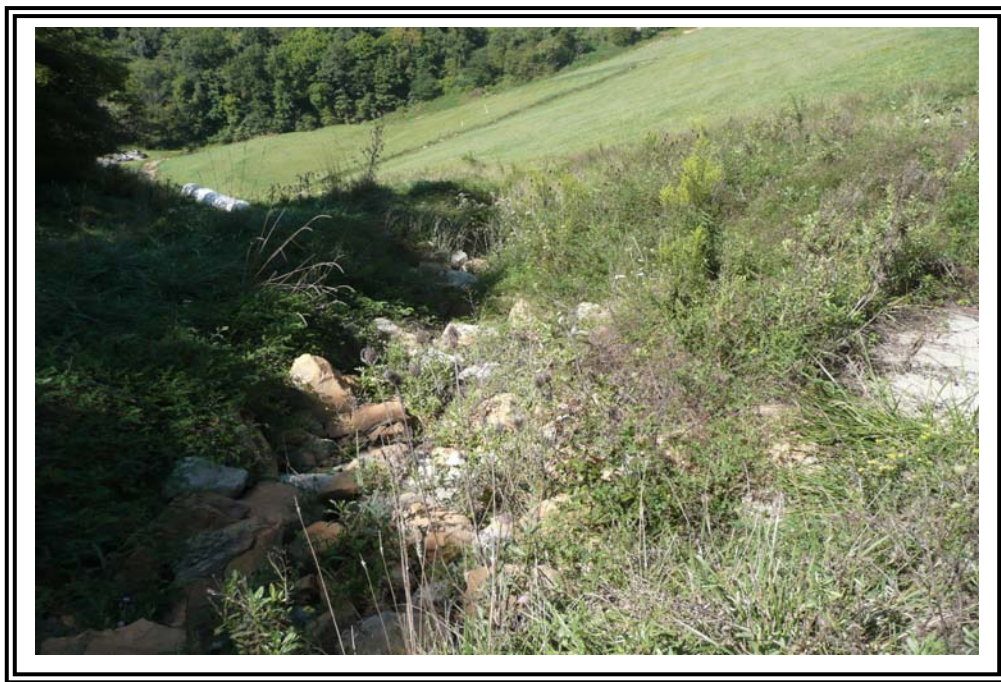
Closer view of rock groin at east abutment where spillway outlet transitions to welded steel pipe.
