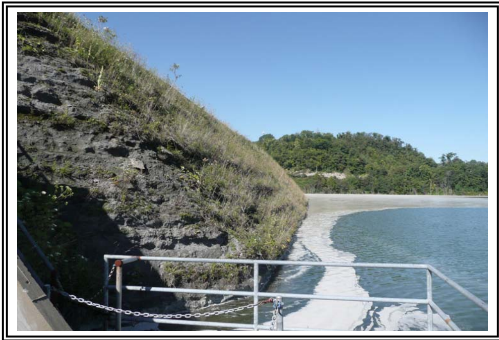
Upstream slope looking west from spillway.
