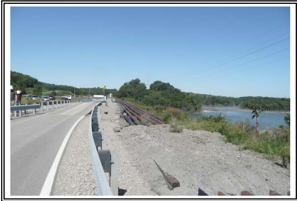
Looking north at crest area showing landfill truck scales and sluice lines to Fly Ash Reservoir No. 2.
