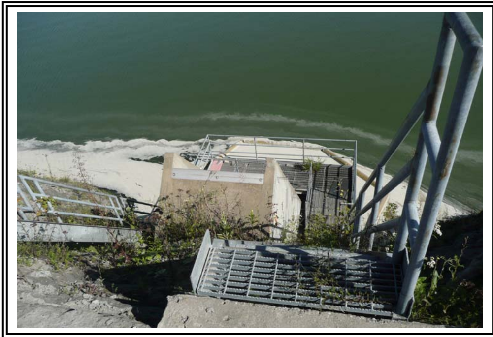
Inclined spillway from crest.
