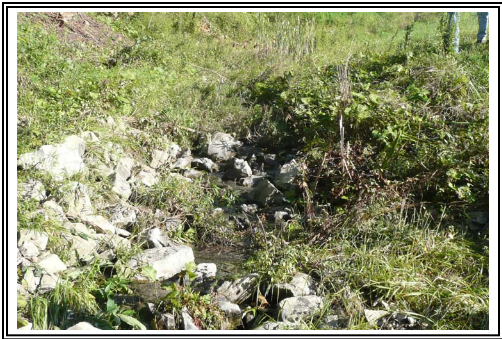
Water in right (west) groin adjacent to lower benches flowing toward toe drain.
