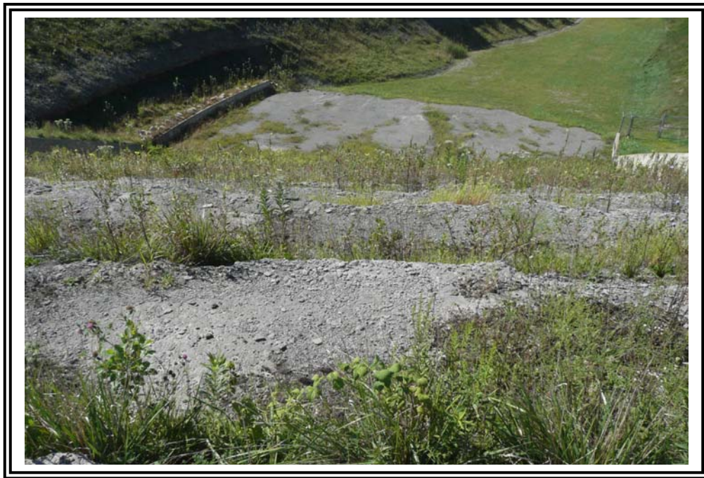
Close-up view of emergency spillway showing RCC steps for energy dissipation, vegetation, and weathering.
