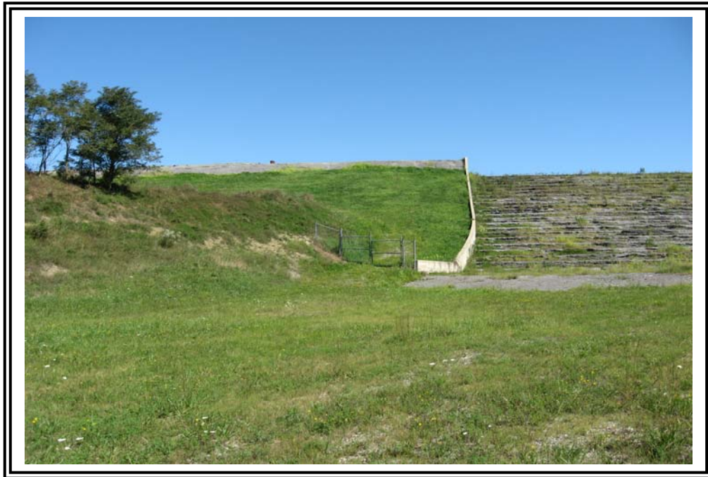
Looking north at dam crest and emergency spillway from downstream channel.
