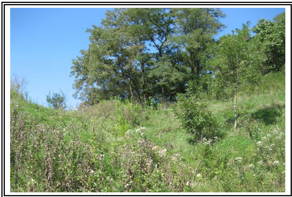
Left (north) abutment rock groin; heavily vegetated.
