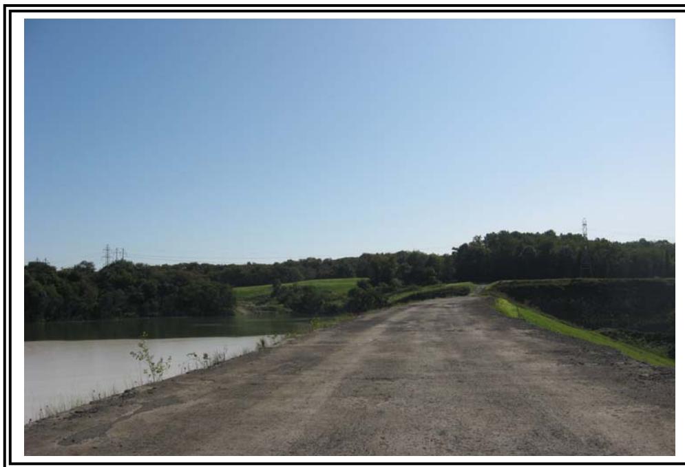
On crest looking east toward left abutment and emergency spillway.
