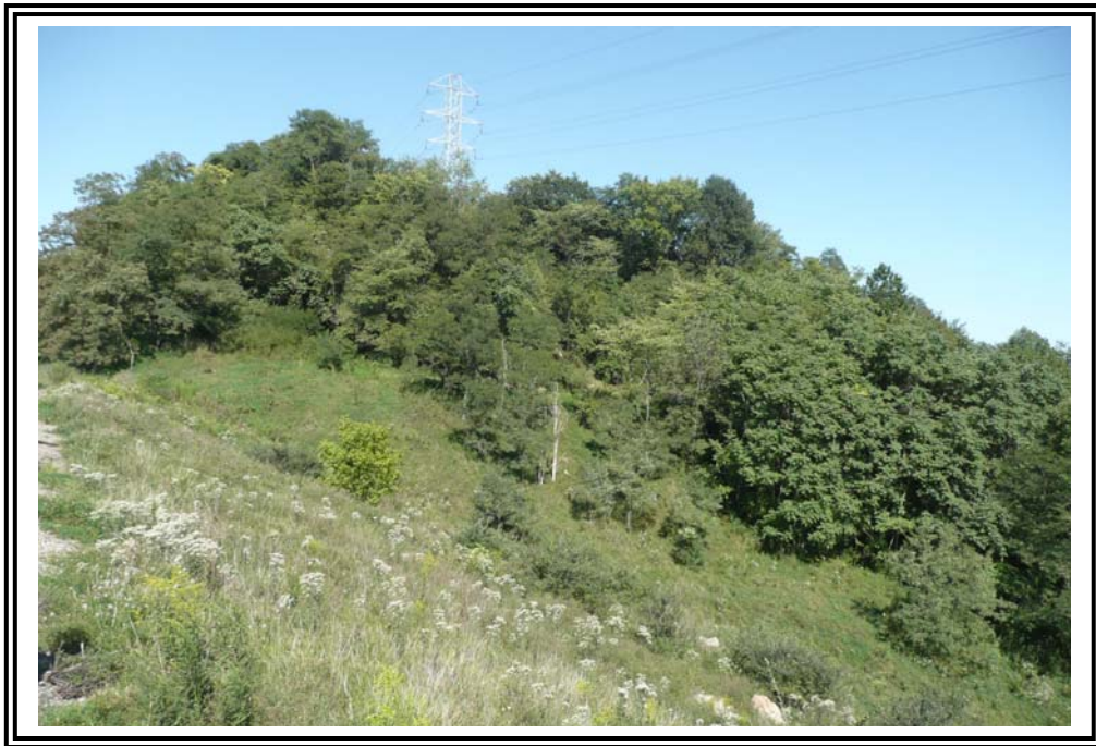
Looking north at downstream slope and left (north) abutment contact.
