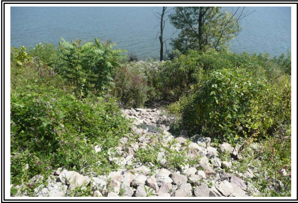
Slope protection below recirculation pond outfall.
