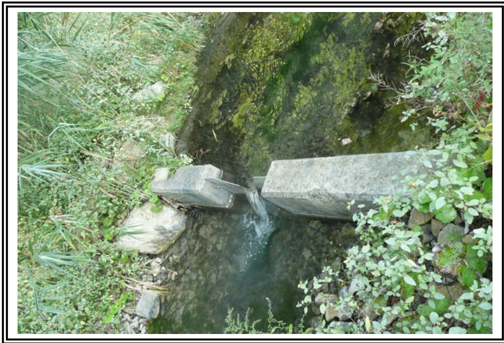
Concrete V-notch weir downstream of seepage collection pool.
