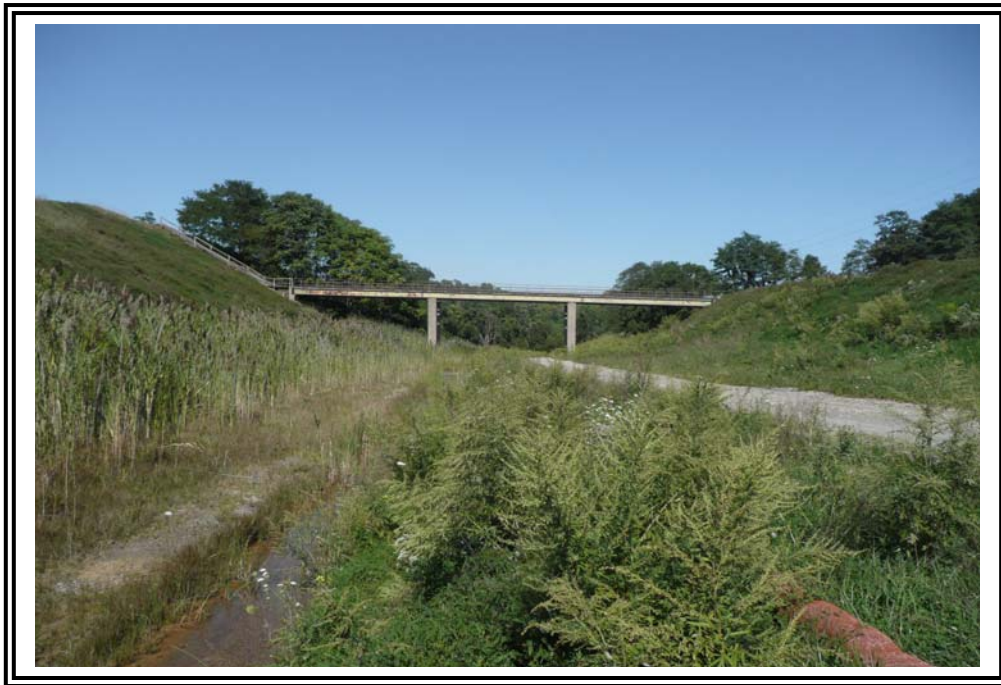
Emergency spillway, looking north from old basin area.
