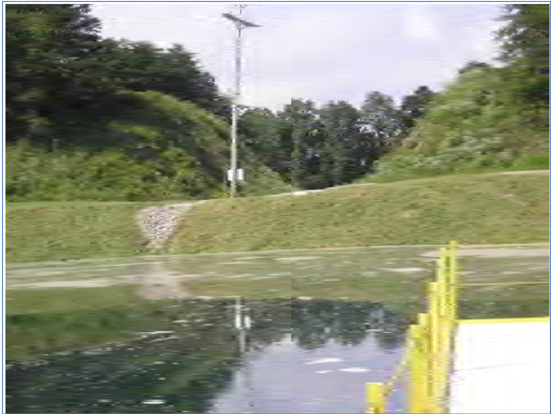
Figure 5.3.3-1. Emergency Spillway at the North end of Dam.
