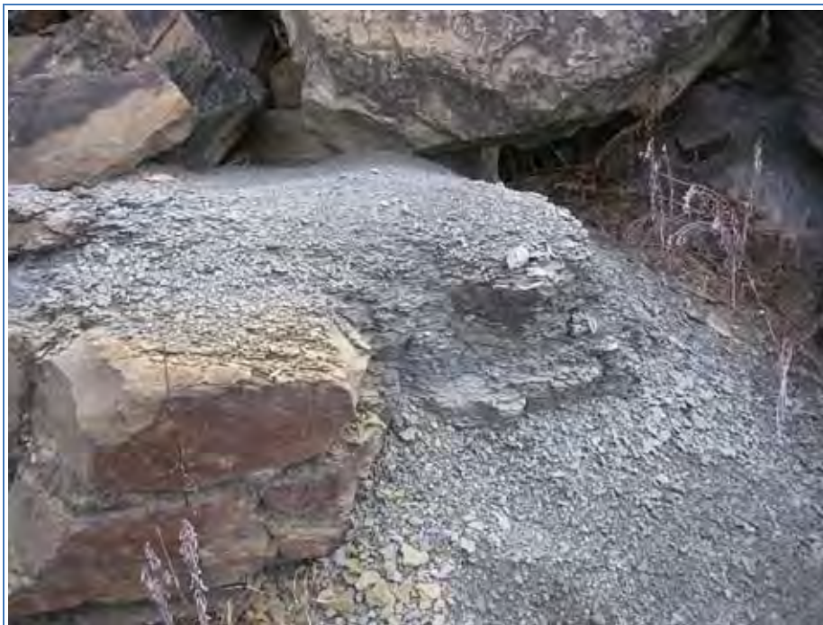
Figure 5.2.3-3. Weathered Rip-Rap at Downstream Slope.
