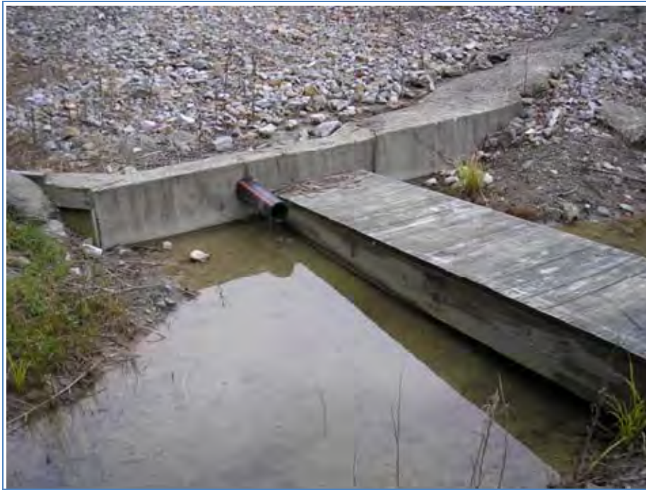
Figure 5.2.3-2. Seepage Collection Basin, Downstream Embankment.
