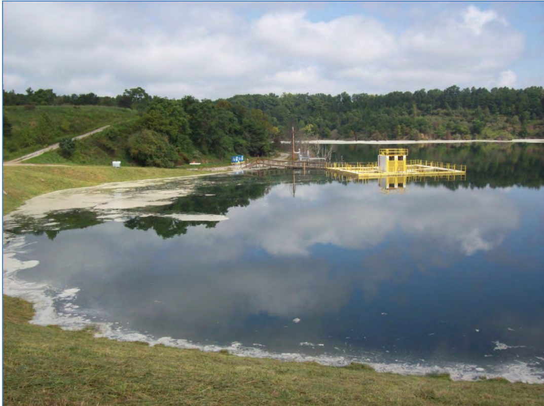
Figure 5.3.1-1. Outlet Structure (Principal Spillway) and the Floating Pier Around it on the Northwest End of Dam.
