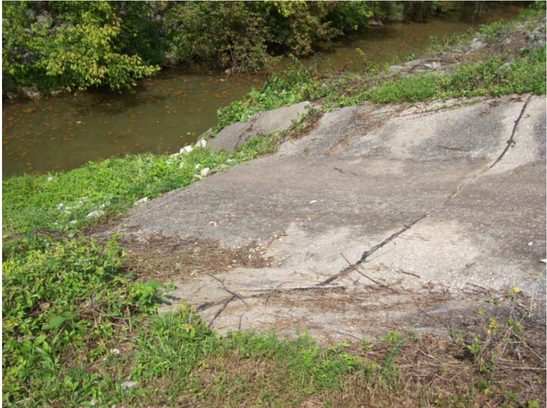
Figure 5.3.3-2. The Downstream View of the Emergency Spillway. The Broken concrete Section Filled with Rip-rap and Covered with Grass is Visible on the Downstream Side.
