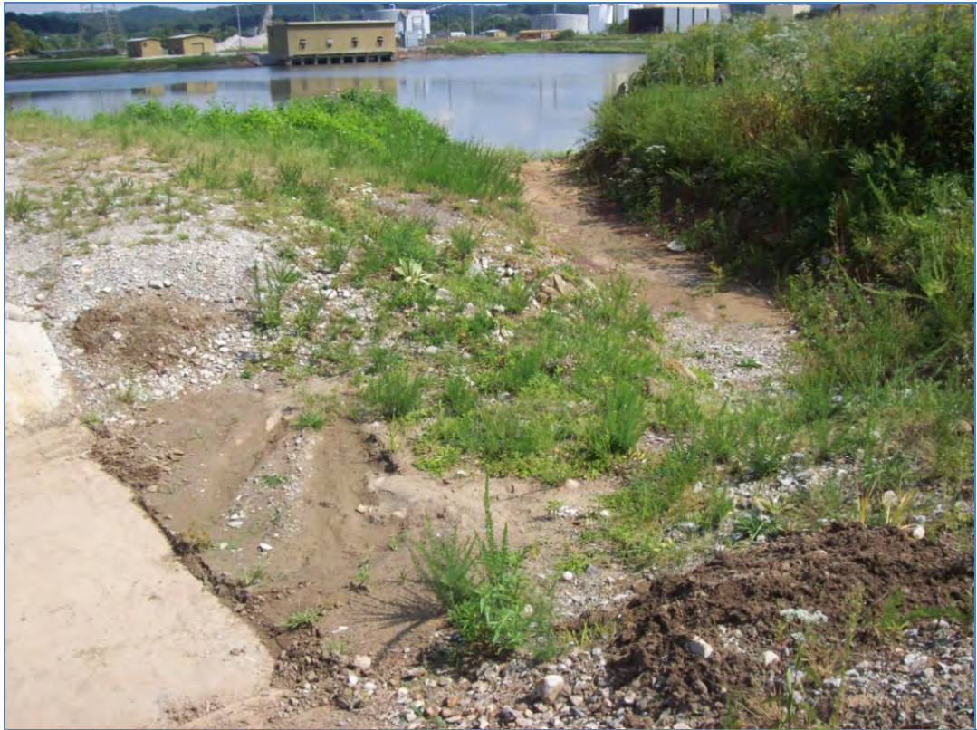
Figure 5.3.3-1. Approach Channel to Emergency Spillway Excavated to on the Main Dam Embankment. The Upstream Side of the Overflow Concrete Spillway is Visible on the Left Side of the Picture.
