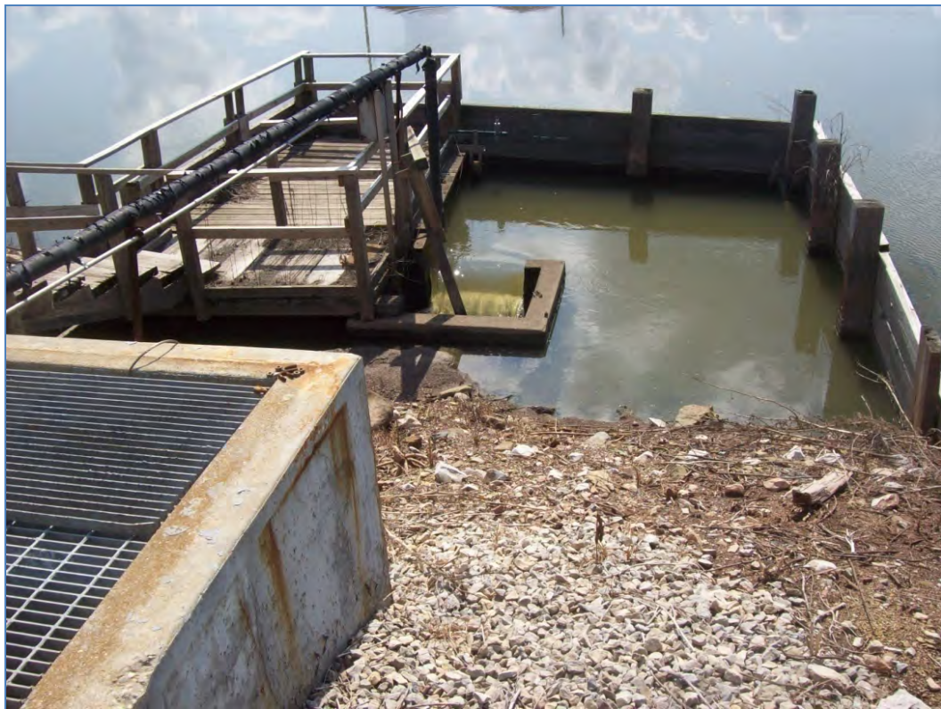
Figure 5.3.1-1. Low Inlet Overflow Outlet Structure at the North Corner of the Treatment basin.
