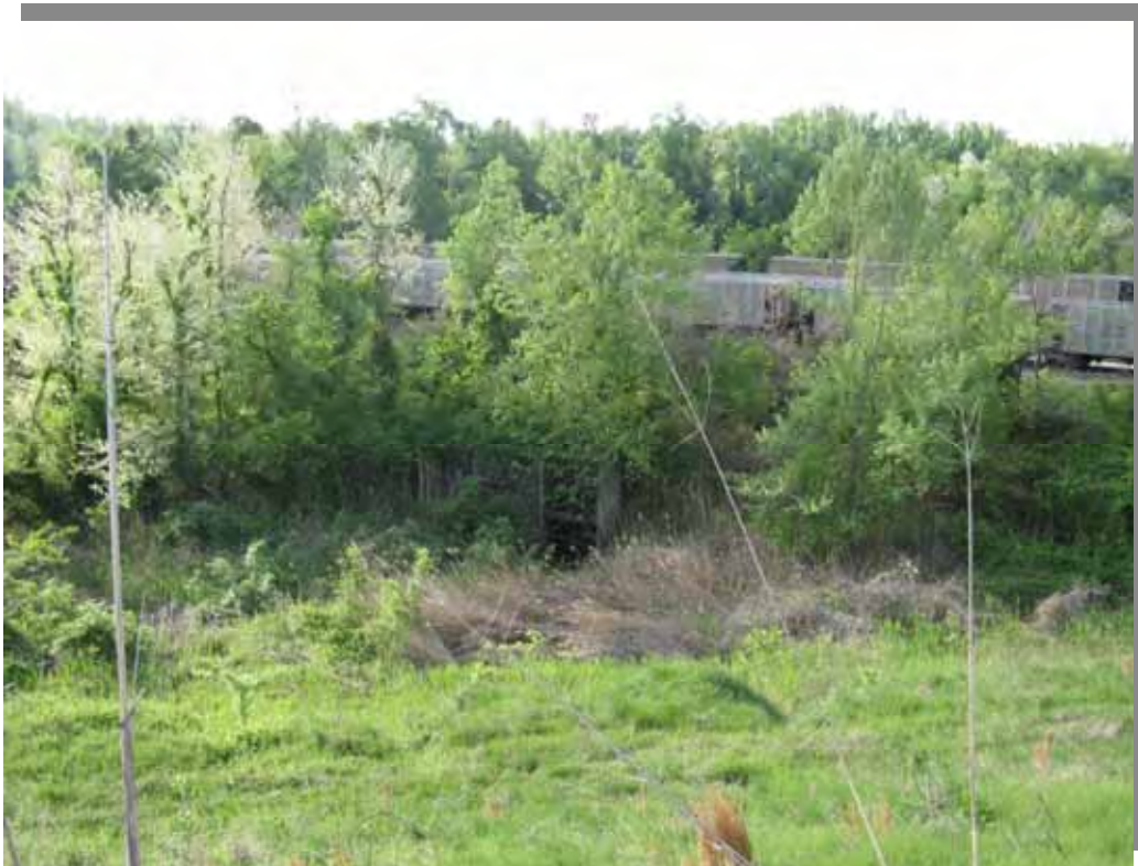
Photo 25 – Ash Pond outlet channel pass-through below EEI railroad siding.
