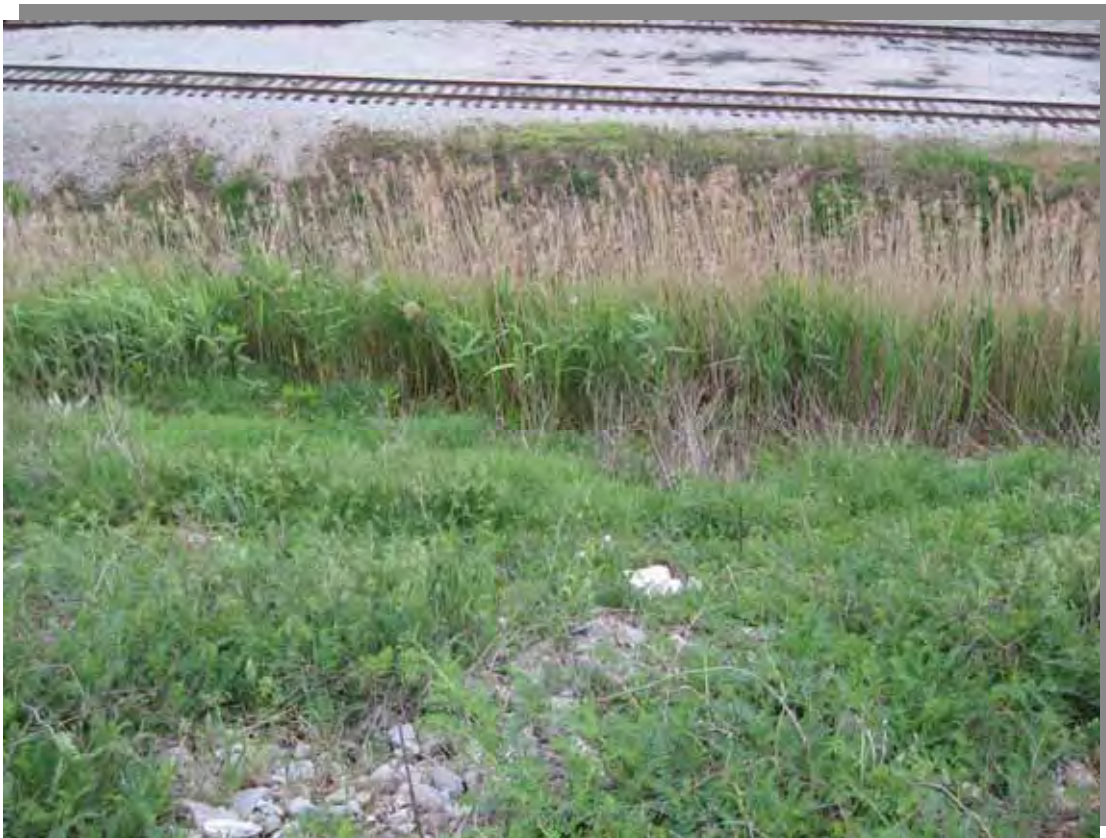
Photo 8 – Outboard slope of Northern Pond near the northern end. Note reedy grasses at toe.
