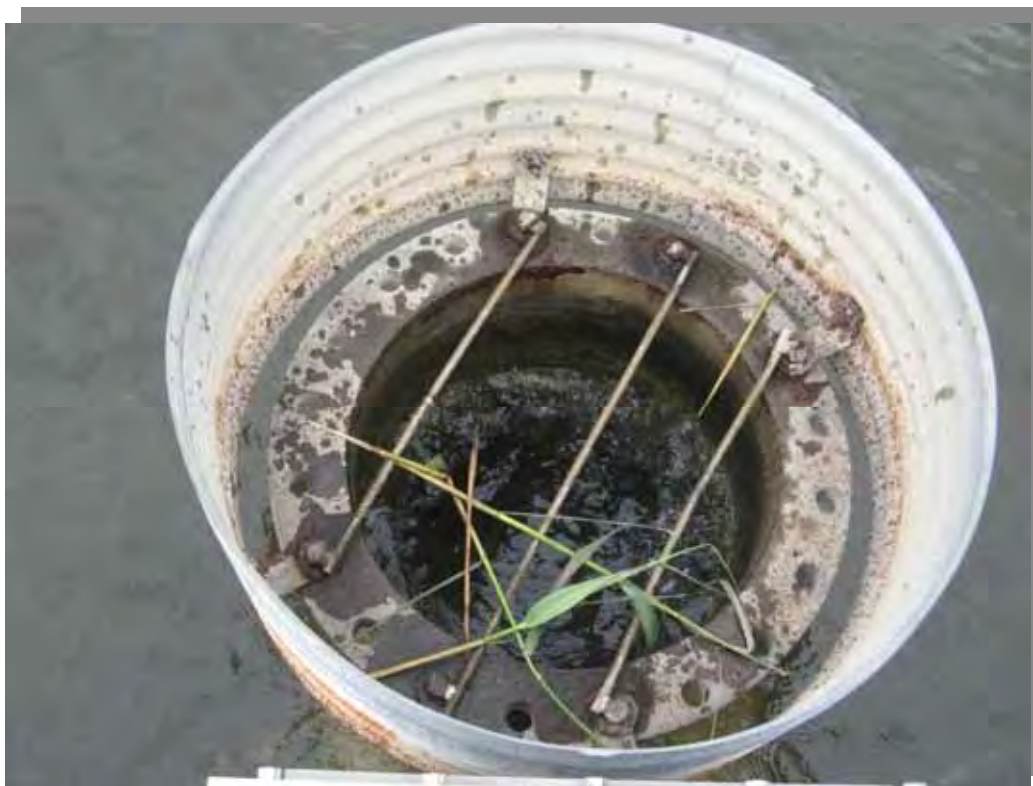
Photo 16 – Interior of Southern Pond primary outlet structure.
