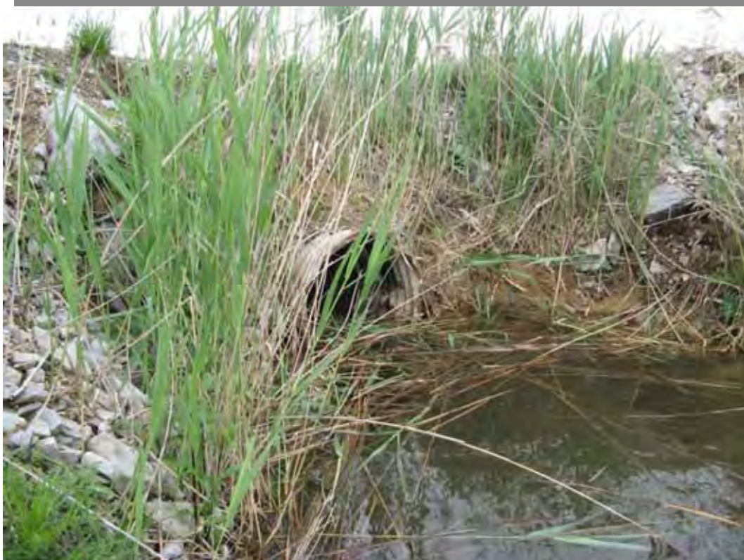
Photo 2 – Central Dike Culvert entrance in Southern Pond. Note water surface elevation in pond in relation to pipe invert.
