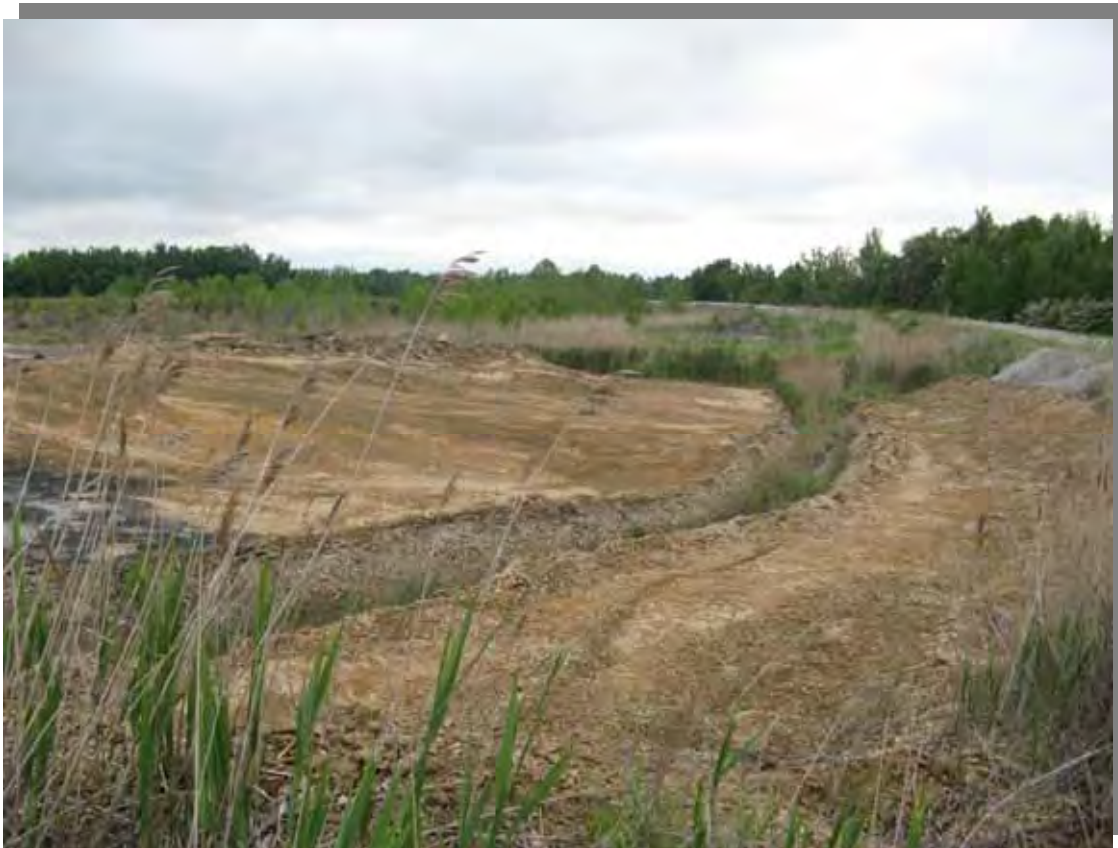
Photo 4 – Interior of Northern Pond, looking north from Central Dike. Channel to direct flow from Culvert to Pond outlet structure.
