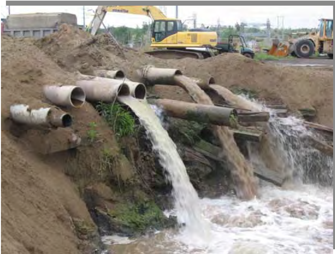
Photo 13 – CCW discharge from Joppa Plant into Ash Pond at southwestern corner of Southern Pond..
