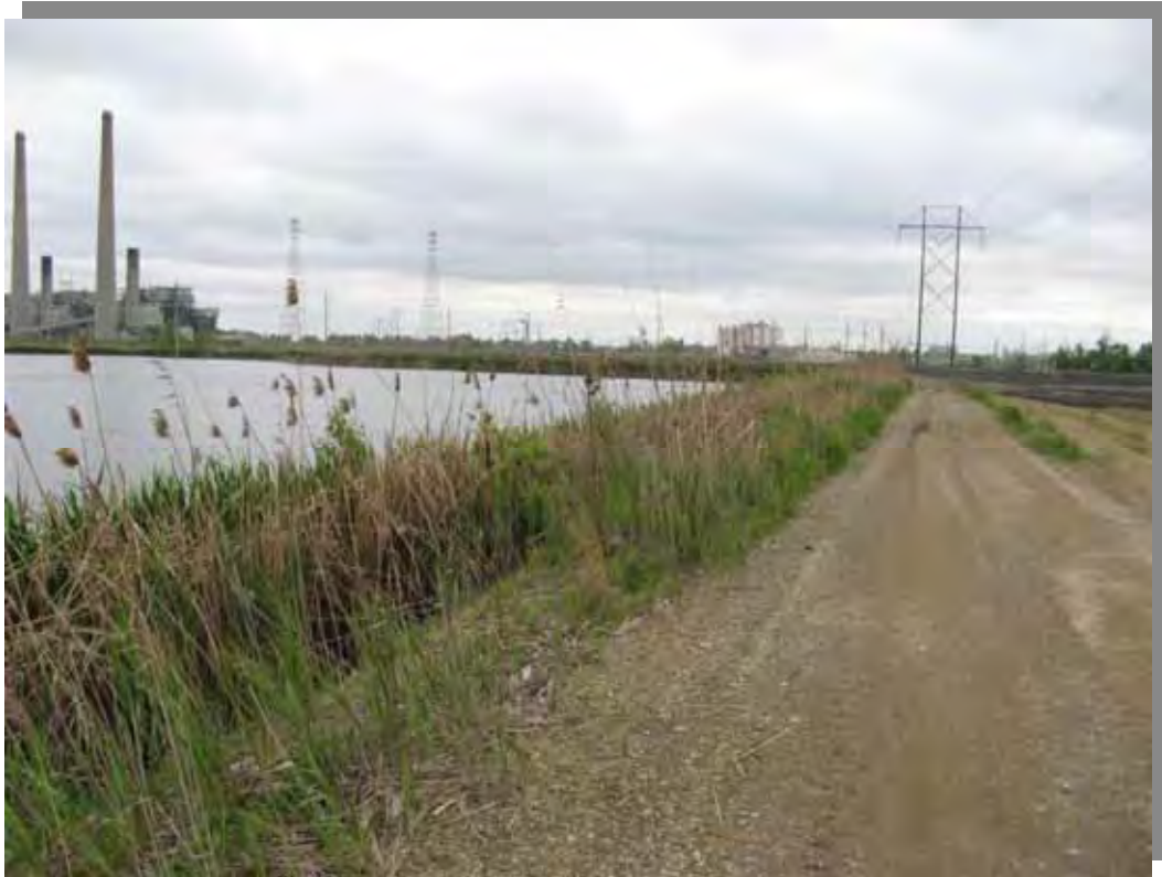
Photo 1 – Central Dike, looking west. Note vegetative growth on inboard slope of Southern Pond.
