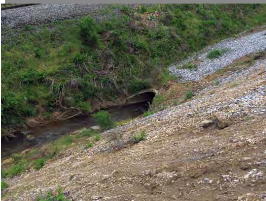
Photo 11 – Ash Pond outlet channel transitioning from open channel to underground culvert.
