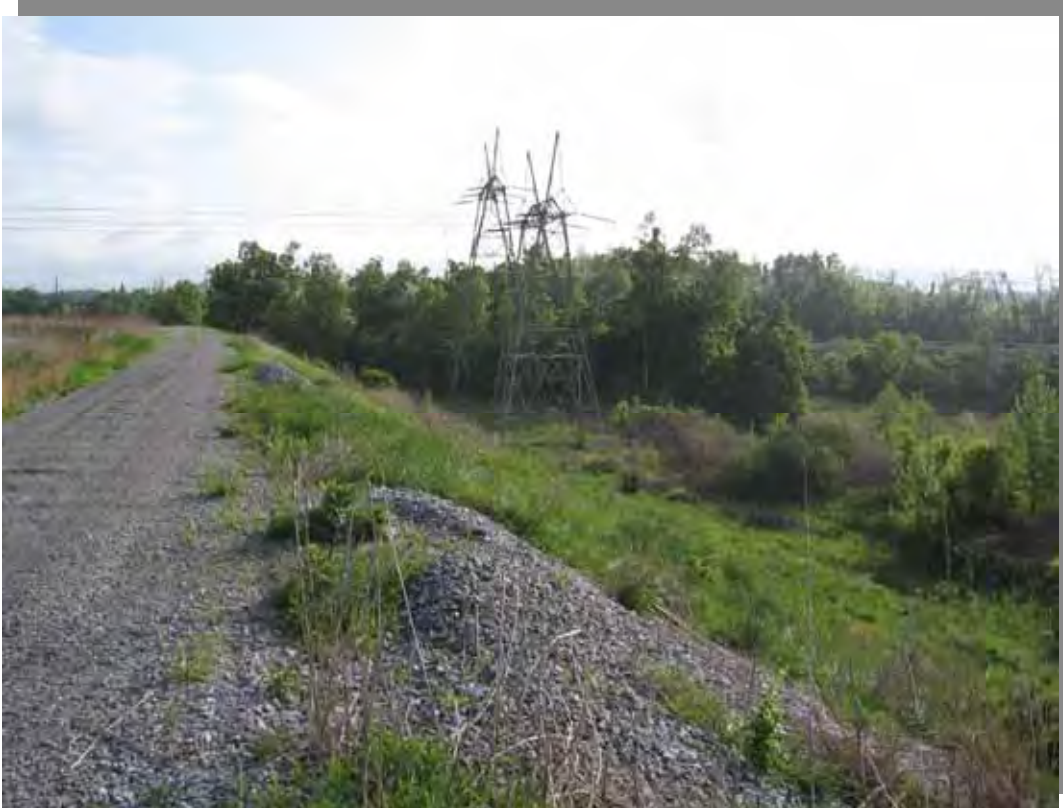
Photo 20 – Outboard slope of Southern Pond near power lines.
