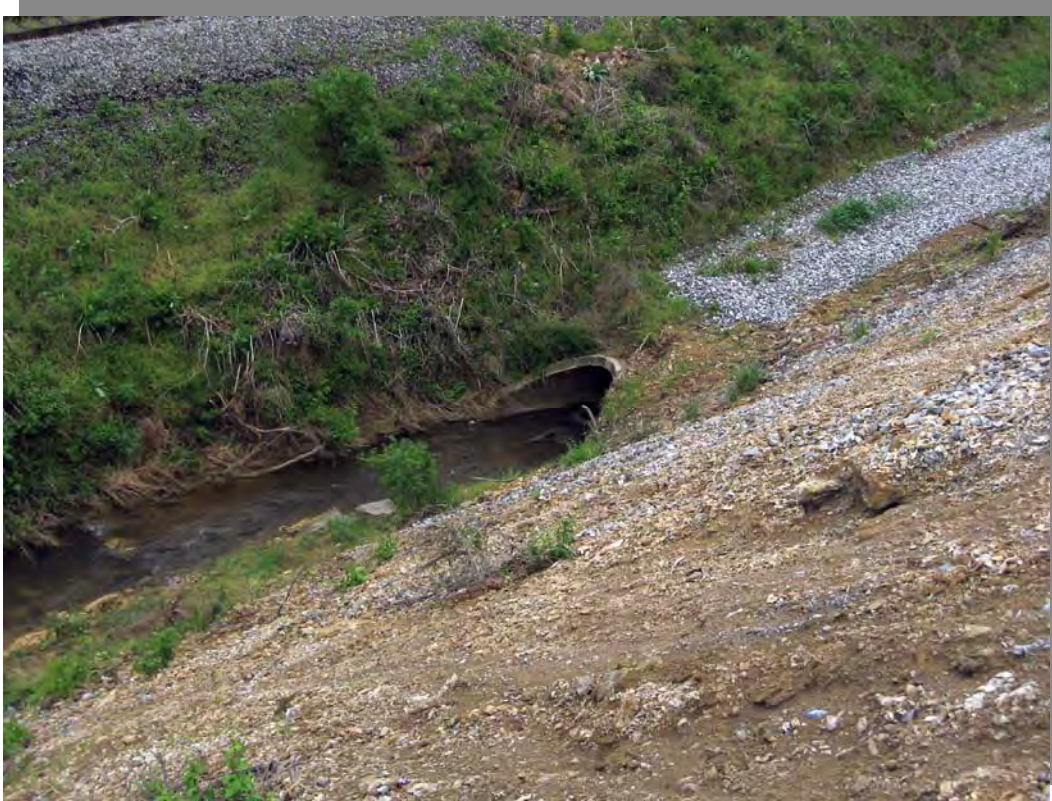
Photo 11 – Ash Pond outlet channel transitioning from open channel to underground culvert.
