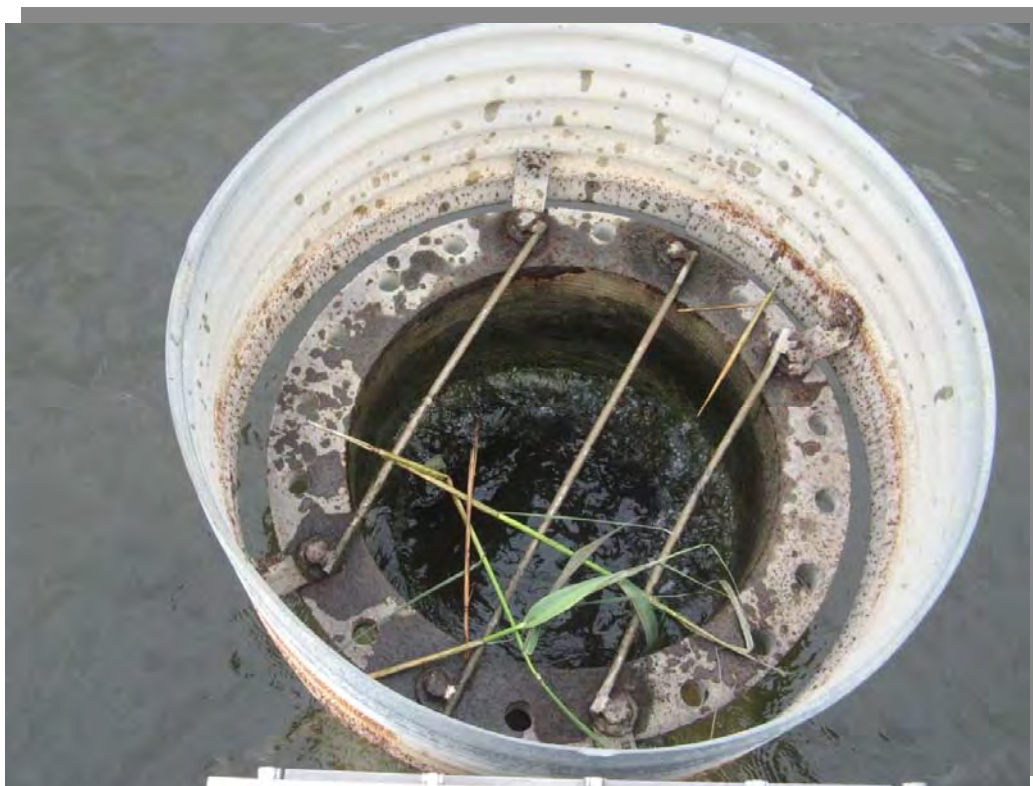
Photo 16 – Interior of Southern Pond primary outlet structure.
