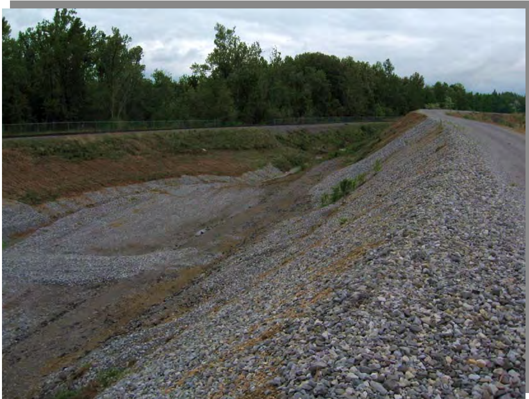
Photo 5 – Interior of Northern Pond, looking south from northern corner. Note vegetative growth on inboard slope..
