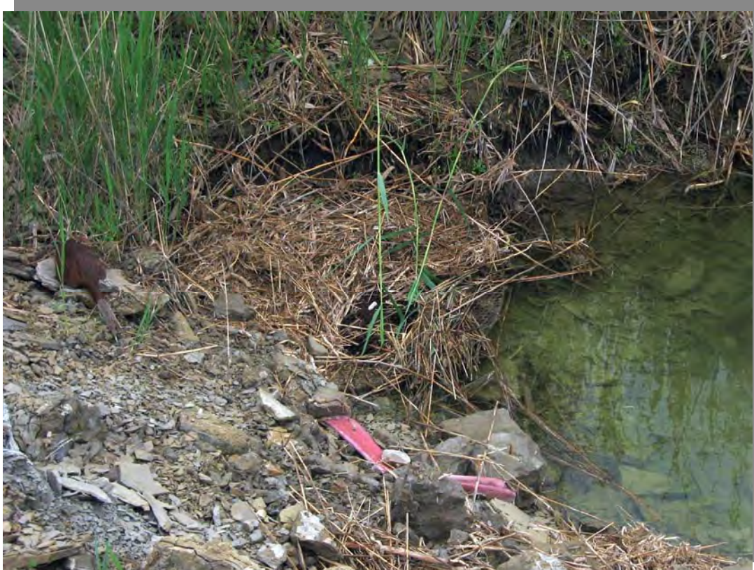
Photo 12 – Northern Pond outlet structure, located at northern end of impoundment.
