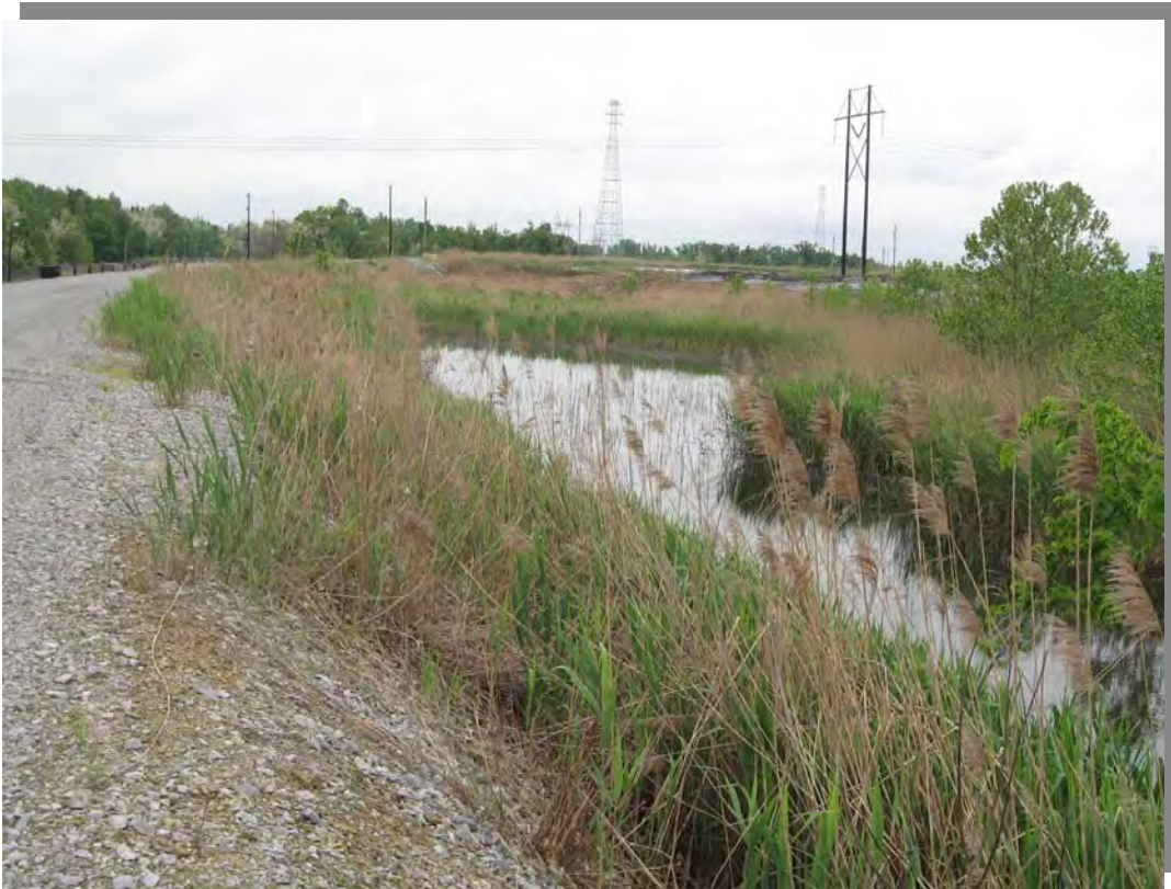
Photo 5 – Interior of Northern Pond, looking south from northern corner. Note vegetative growth on inboard slope..
