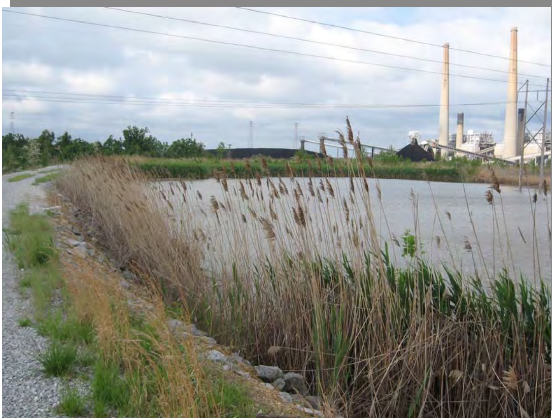
Photo 17 – Interior of Southern Pond, looking south from primary outlet structure.
