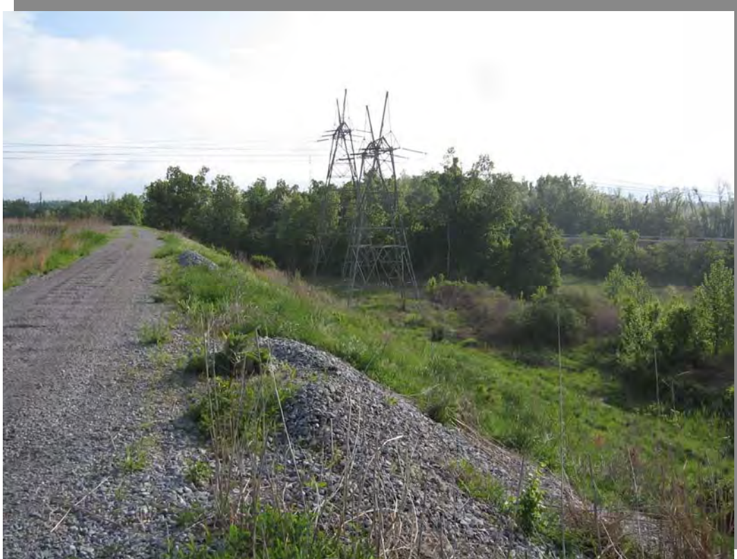
Photo 20 – Outboard slope of Southern Pond near power lines.
