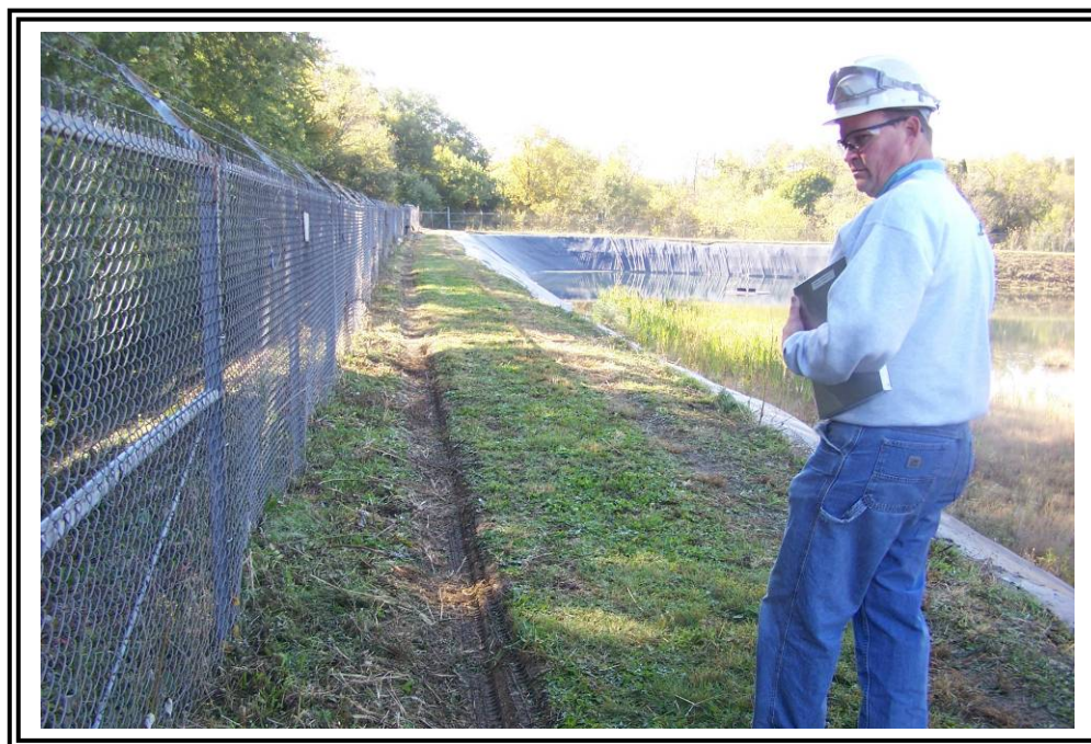
Crest of east dike at Pond #4, looking south.
