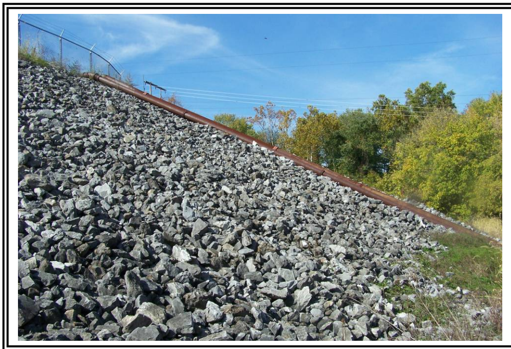
Sluice lines from R Paul Smith Station at northeast corner of Pond #3 service both Pond #3 and Pond #4. Hardened steel line to dike crest and are replaced approximately every 15 years as routine maintenance.
