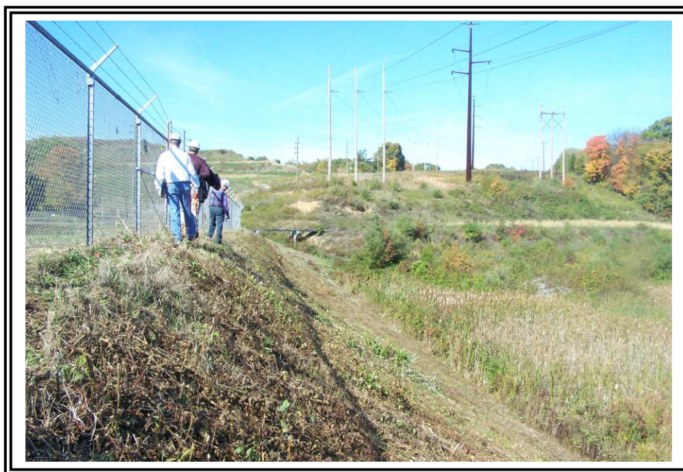
Downstream slope of north dike at Pond #4, looking north.
