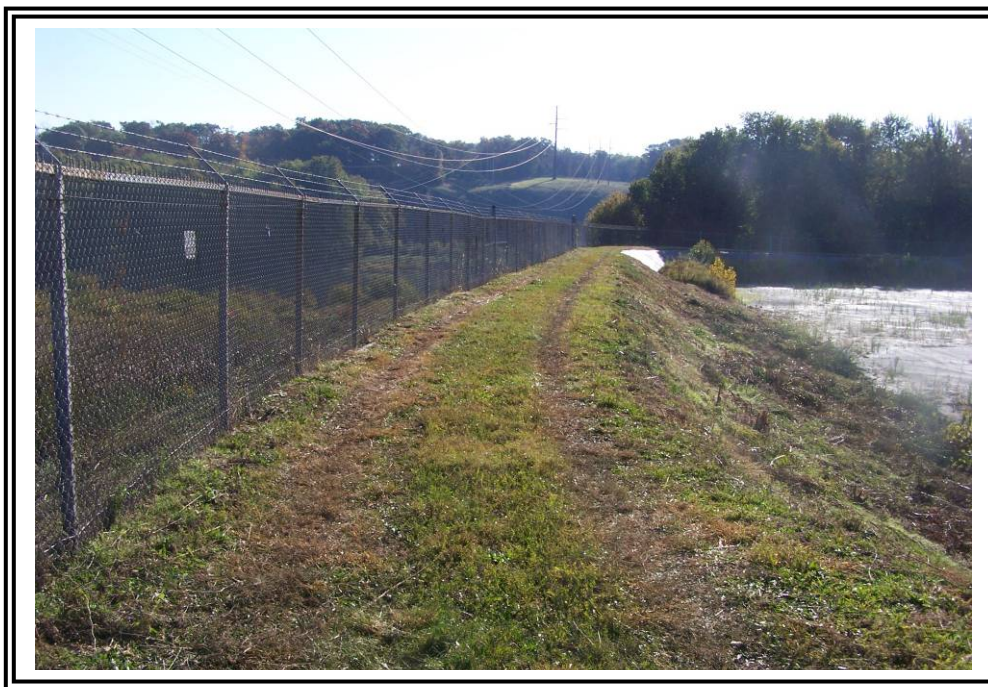
Crest of the north dike at Pond #4, looking east.
