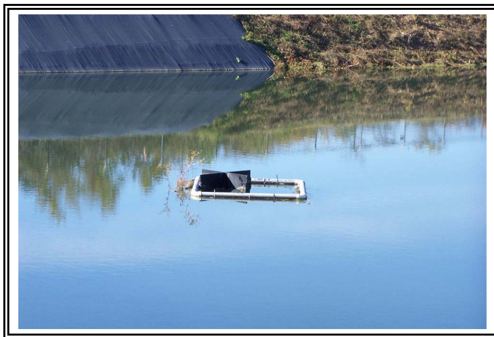
Decant structure in the southeast corner of Pond #4.
