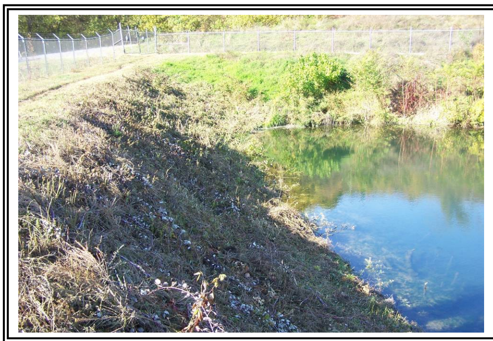
Upstream slope of the south dike at Pond #4, looking west toward the south abutment.
