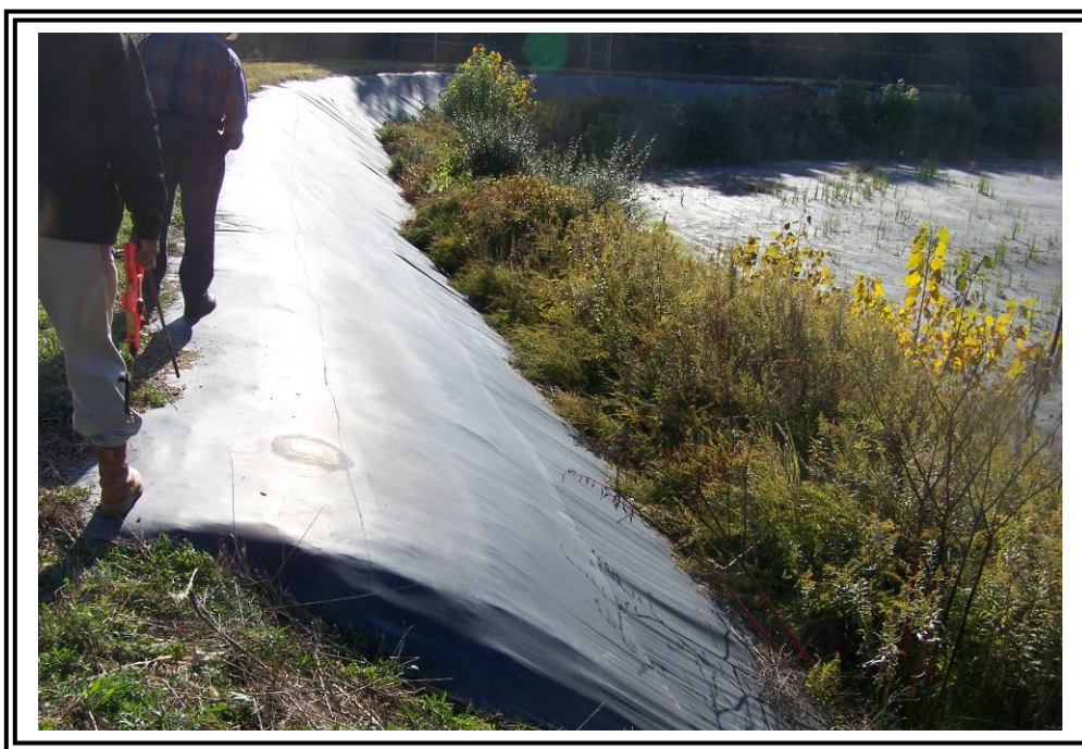
Hypalon liner on the upstream slope of the north dike at Pond #4.
