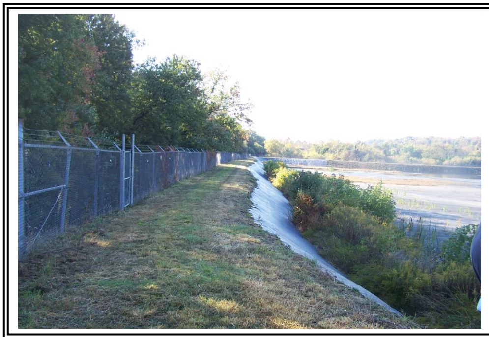
Crest of east dike at Pond #4, looking south.
