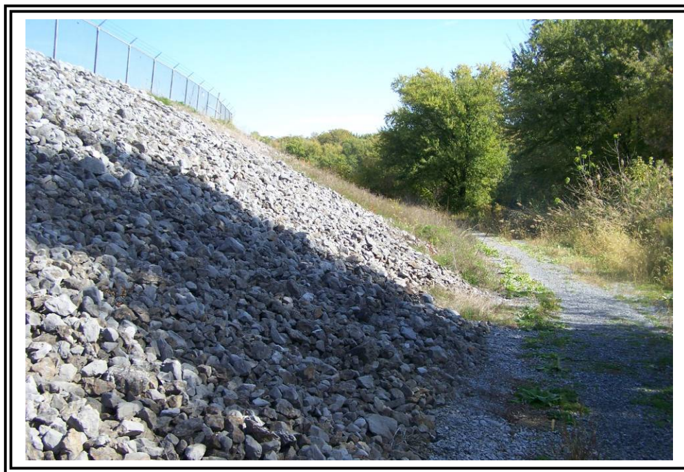
Downstream slope of south dike of Pond #3, looking east.
