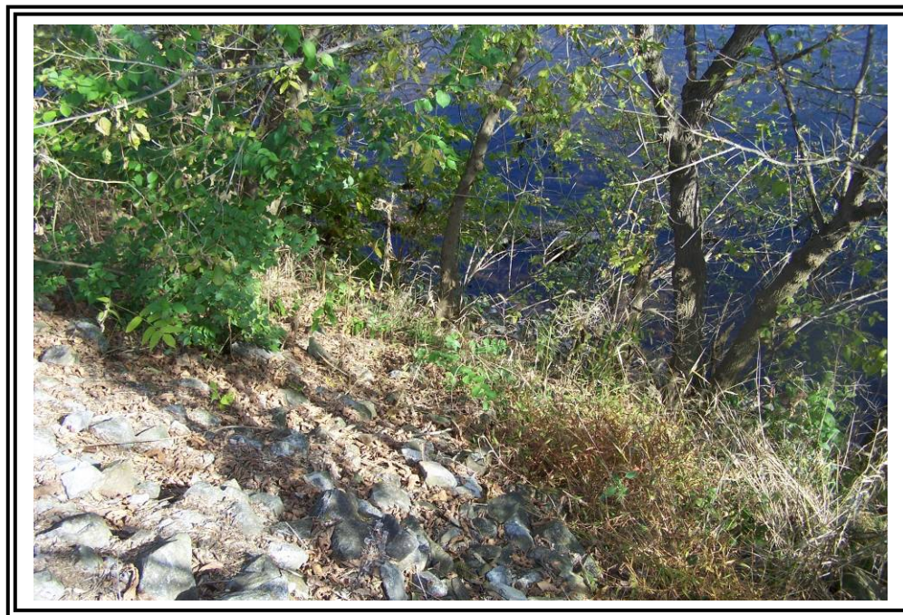
Stone buttress on east dike of Pond #3 extends to the edge of the Potomac River.
