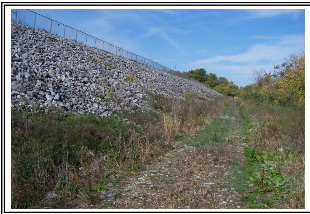
Downstream slope of east dike at Pond #3, looking north.
