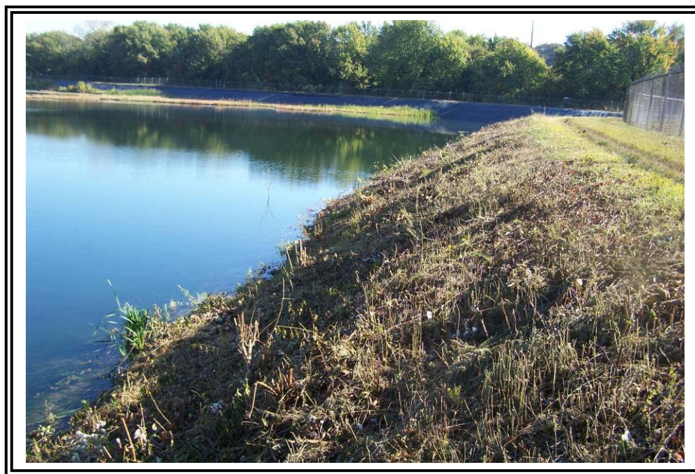
Upstream slope of south dike at Pond #4, looking east.
