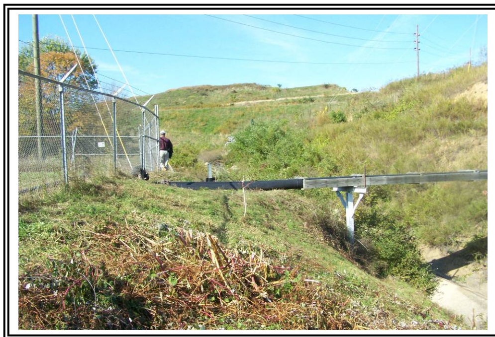
Sluice lines at north abutment.
