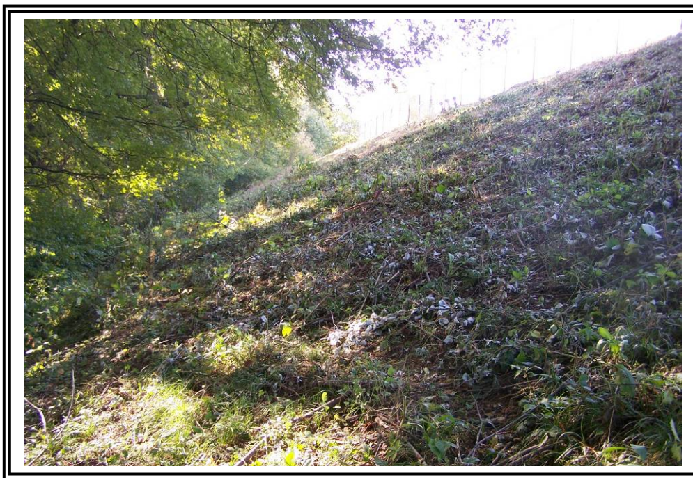
Downstream slope of east dike at Pond #4, looking south.
