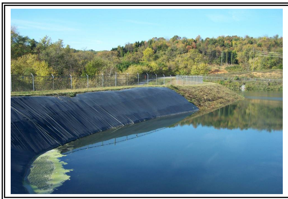
Upstream slope of south dike at Pond #4, looking southwest.
