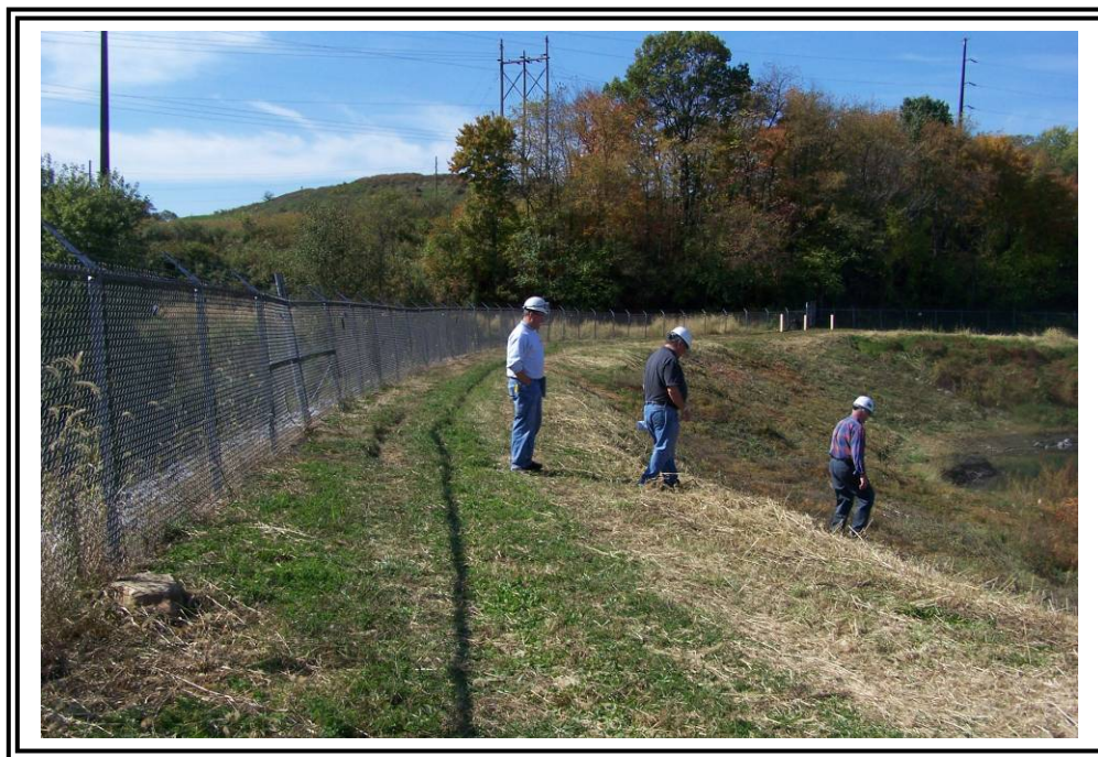
Crest of south dike at Pond #3, looking west toward south abutment.
