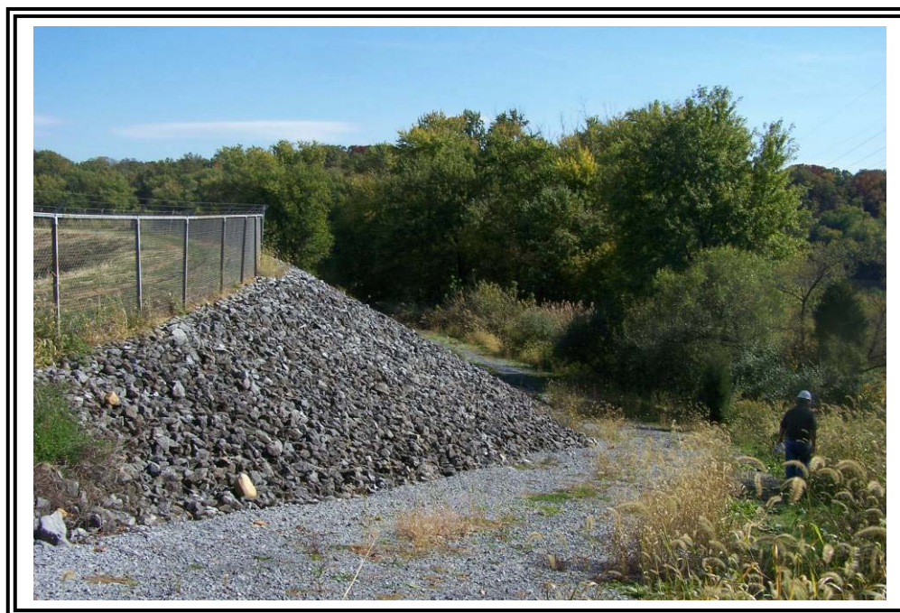
Downstream slope of south dike of Pond #3, looking east.
