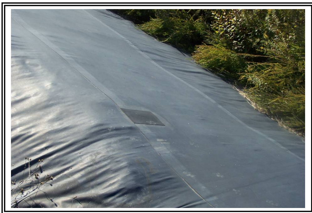
Routine maintenance includes patching holes on the hypalon liner created by animals walking on the liner.
