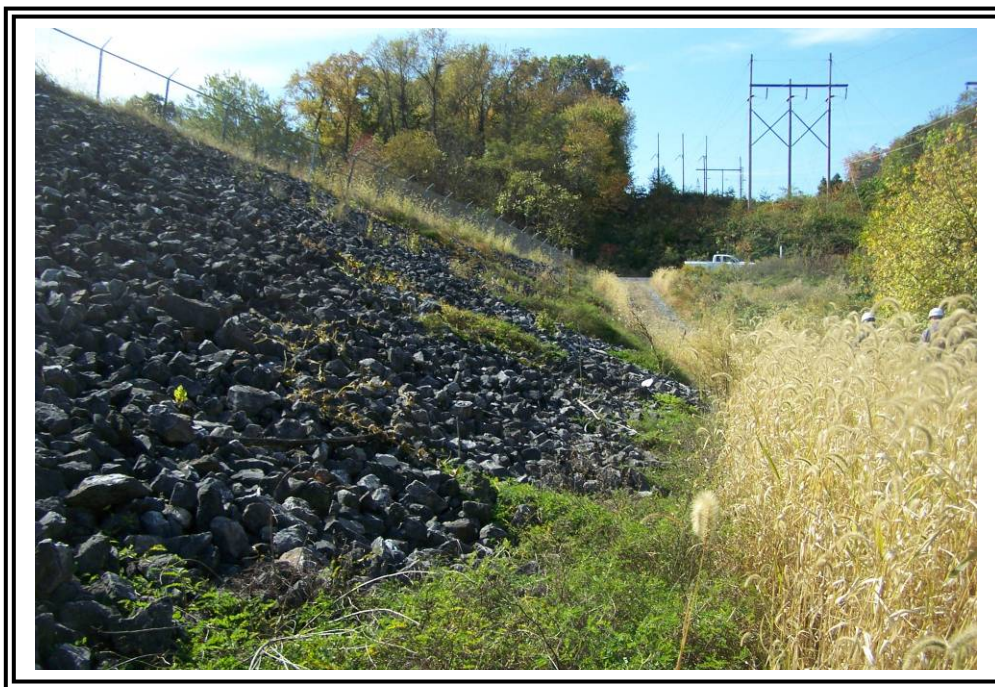
Downstream slope of north dike at Pond #3, looking west towards north abutment.
