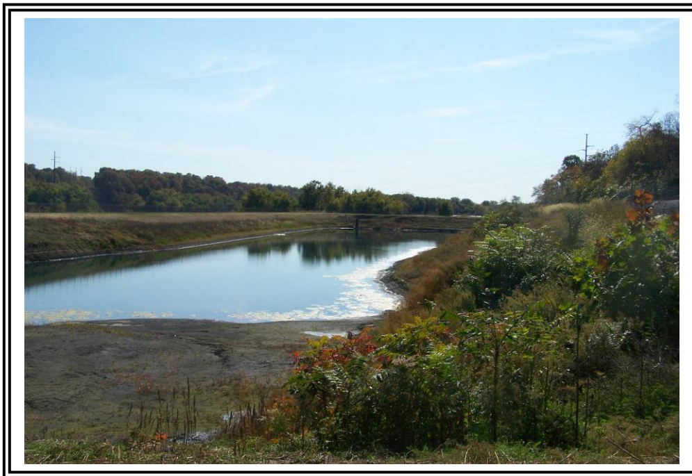
Pond #3, looking southeast from the north abutment. West side of pond (right side of photo) is in natural ground.
