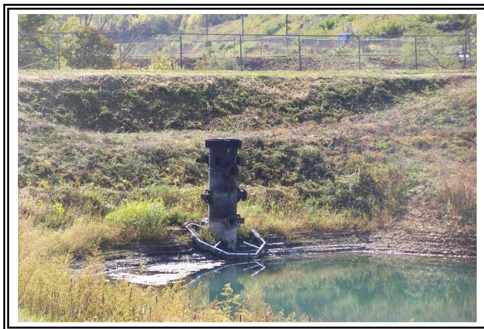
Upstream slope of south dike of Pond #3 looking south and decant structure. Bench is remnant of an access road built when the decant structure was replaced in 1997.
