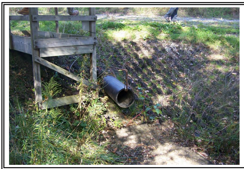
Outlet pipe from the decant structure. Pond currently dewatered/dredged below the decant elevation.
