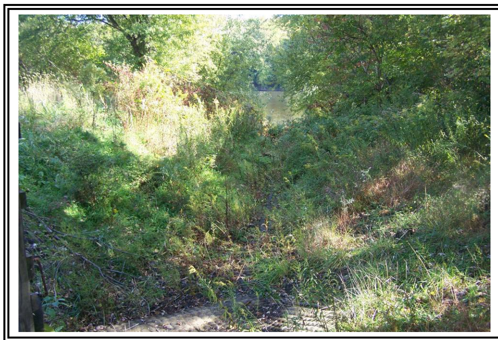
Fabriform lined discharge channel from Pond #3 to the Potomac River.
