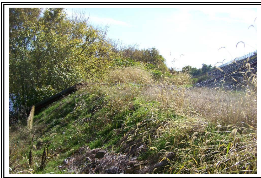
Stone buttress at looking south from northeast corner of Pond #3.
