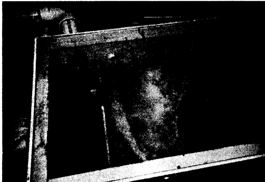
FIGURE 10. SEDIMENTATION TANK FOR LIQUID EFFLUENT FROM MECHANICAL/CHEMICAL TREATMENT SYSTEM
