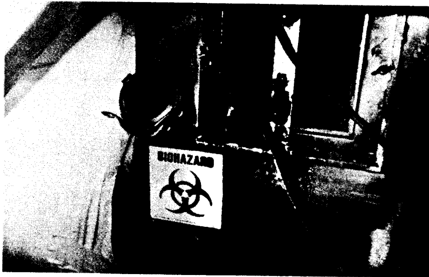
FIGURE 4. MICROWAVE UNIT ACCESS PORT TO UNTREATED WASTE TRANSPORT AUGER
