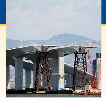
over 30 concrete mix designs in the new bridge, some containing more than 50% fly ash. In addition, ground granulated blast furnace slag was used in pier columns to improve durability and workability and reduce bleeding. In 2006, Caltrans received an award for Innovation from EPA's Coal Combustion Products Partnership (C<sup>2</sup>P<sup>2</sup>), in part based on its work on the new Bay Bridge.
