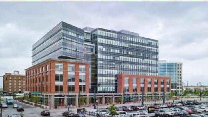
EPA's Region 8 headquarters in Denver has earned a Leadership in Energy and Environmental Design (LEED®) Gold rating and contains recycled industrial materials throughout the structure. For more information, visit: www.epa.gov/region8/building/index.html .
