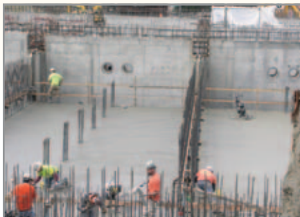
Construction workers pour concrete containing fly ash
