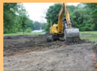
Heavy equipment removes lead tainted dirt from nearby park. Photo courtesy of Reading Eagle.
