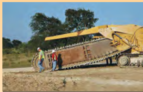
Trenching machine used in biowall construction.
