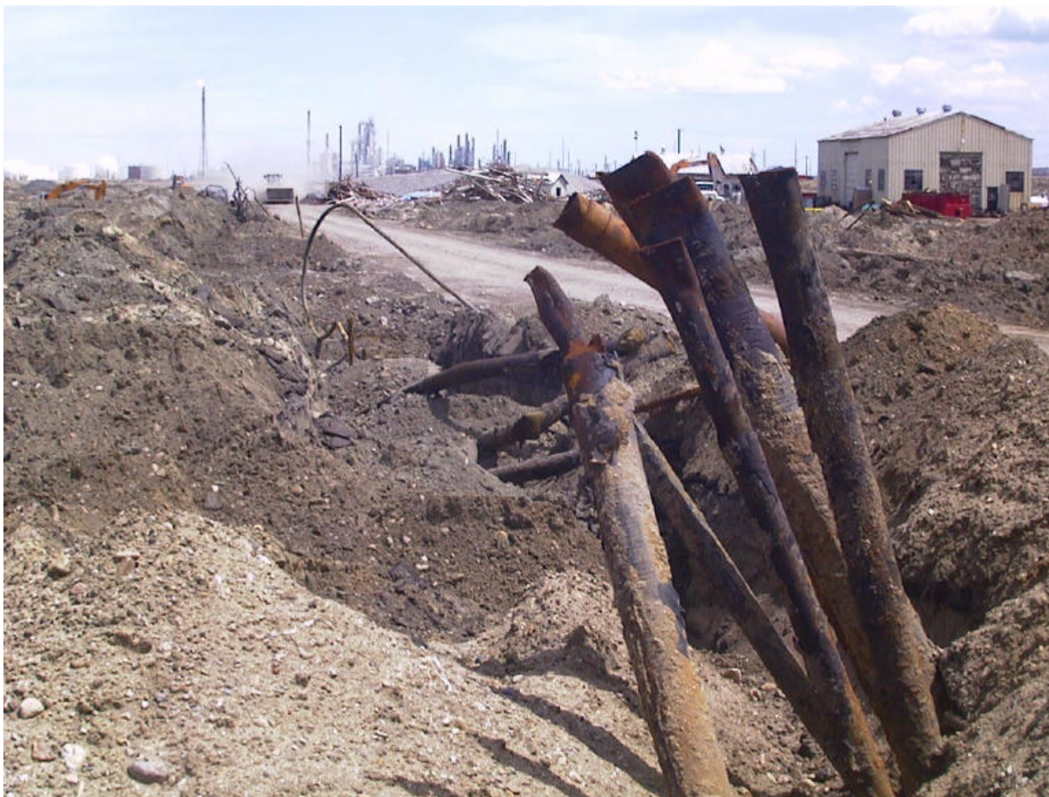
Underground piping removal in progress, Former Texaco Casper Refinery
