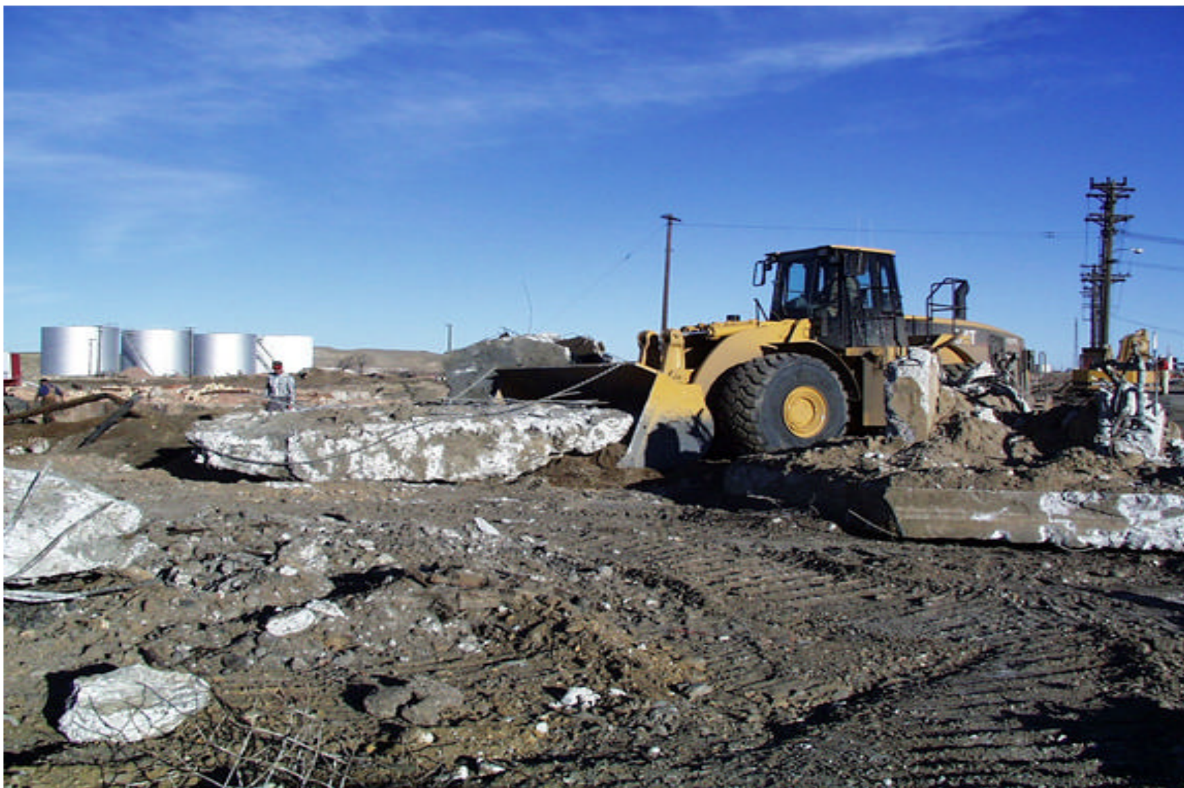
Excavation and removal of subsurface footings and foundations in progress, Former Texaco Casper Refinery
