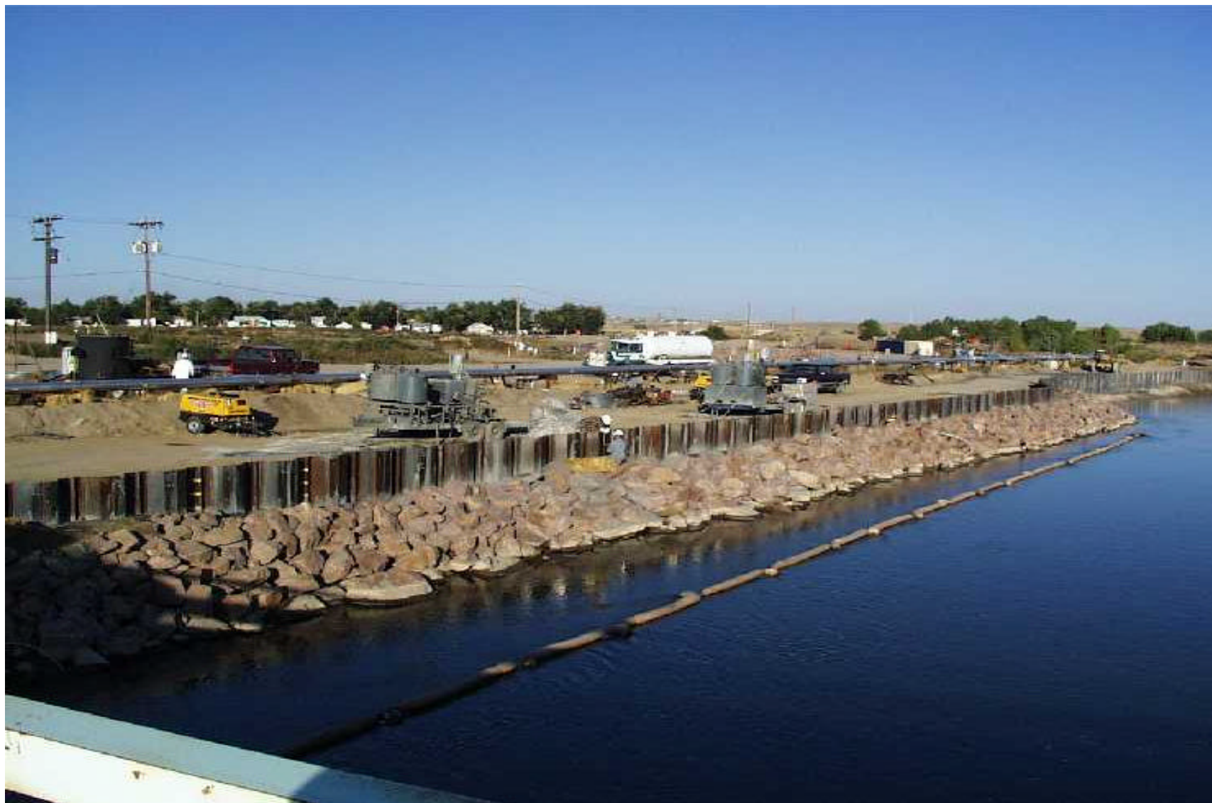
Grouting and sealing operation in progress for sealed joint piling barrier, Former Texaco Casper Refinery
