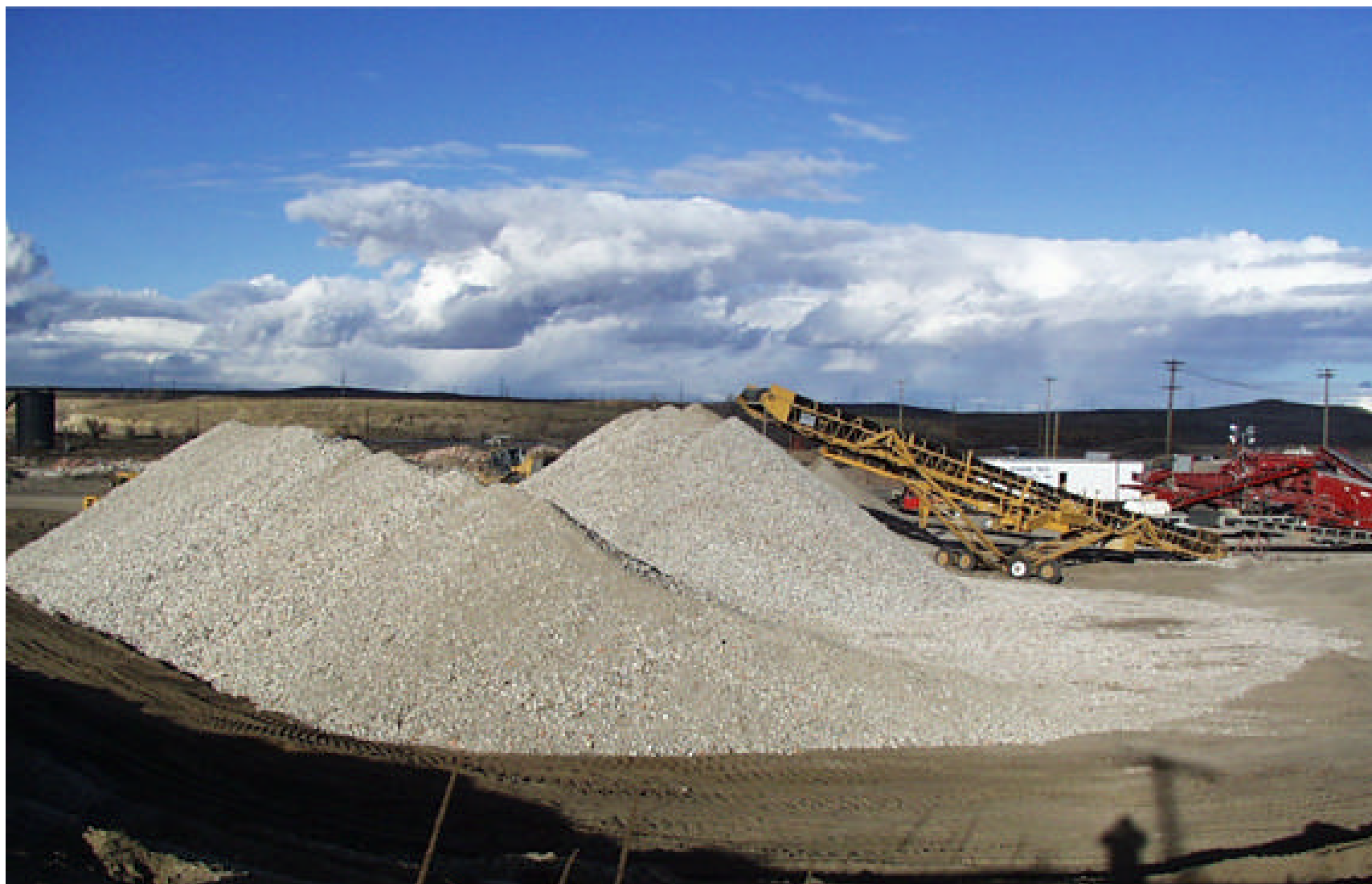
Concrete crushing operation in progress, Former Texaco Casper Refinery
