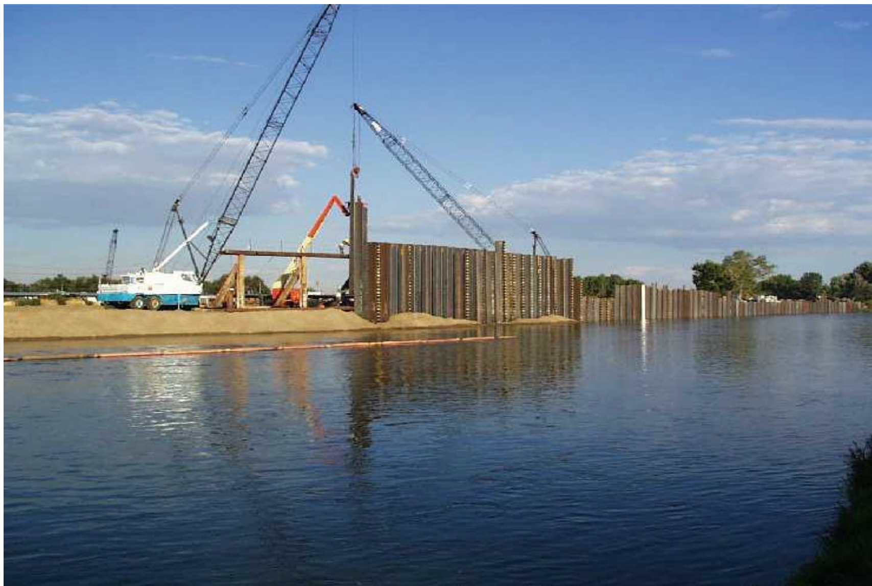
Construction of Sealed-Joint Piling Barrier along south bank of the North Platte River, Former Texaco Casper Refinery
