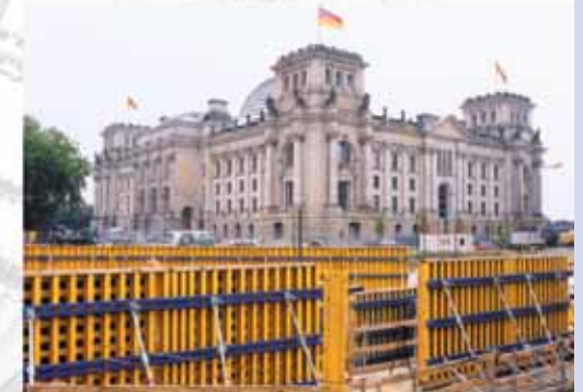
SAS Micro piles in the foundations of Berlin government buildings
