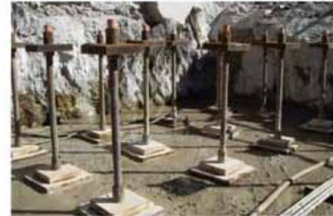
SAS Micro piles for the Foundation of new World Trade Center in New York
