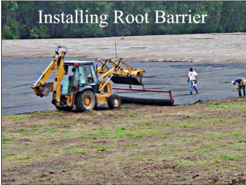
Installing Root Barrier
