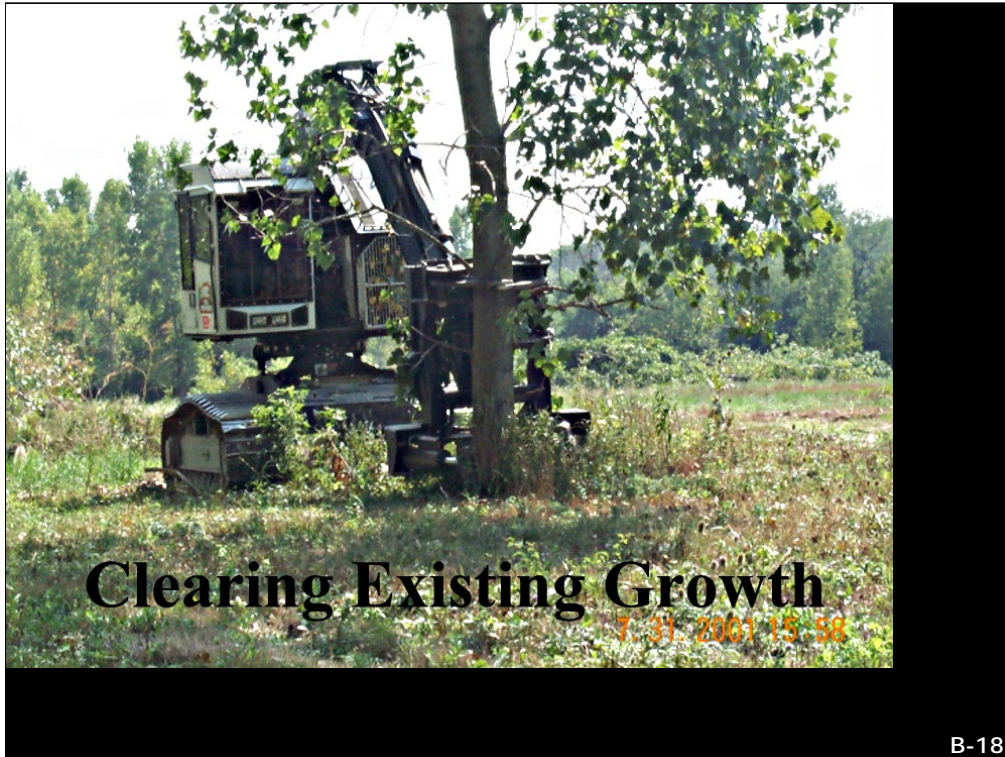
Clearing Existing Growth
