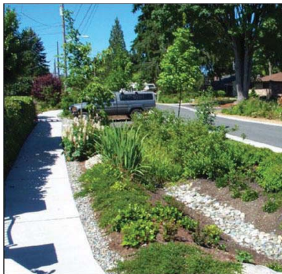
Figure 12 and 13: Parking and streets make up a large percentage of impervious land area within a city. Incorporating green infrastructure into street and parking lot standards could improve water quality from as much as 20 - 30% of the paved surface. (Source: Nevue Ngan Associates for both figures)
