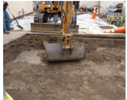
Colorado Smelter cleanup crews excavate contaminated soil from a residential property in Pueblo, Colorado
