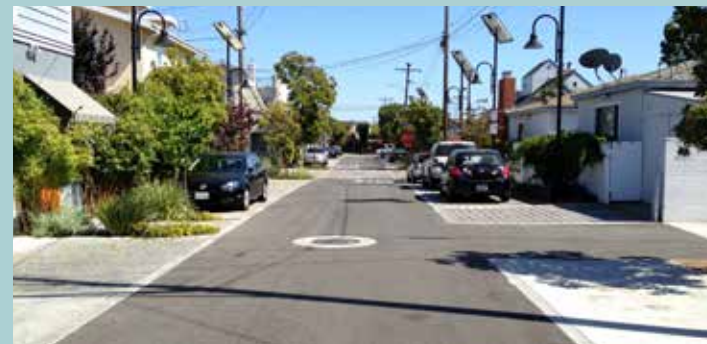
Figure 8. Longfellow Street in Santa Monica, CA is curbless and has no sidewalks. The entire street can be shared by all users. Permeable pavers and landscape planters define parking areas and visually narrow the drive aisle. Cross street intersections are depressed, continuing the curbless street and paver treatments for a uniform appearance and function. Image source: Sherwood Design Engineers
