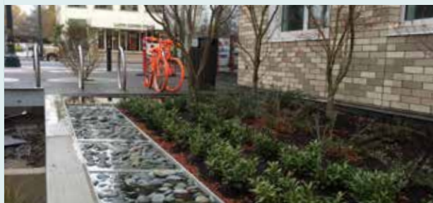
Figure 43. Water features are fed by water harvested from a green roof, and provide a complementary and aesthetically pleasing background of wetland plants and cascading water in the midst of the urban development. Image source: Biohabitats, Inc.
