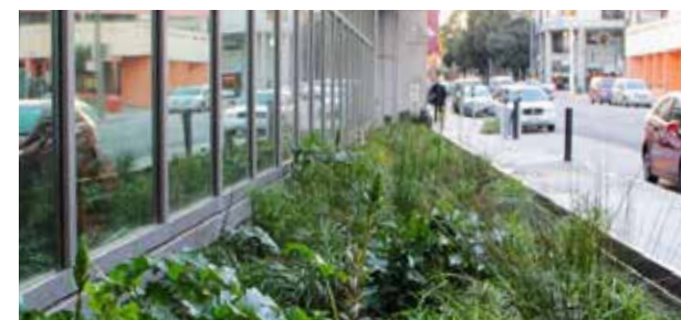
Figure 44. The constructed wetland technology is coined "The Living Machine." The wetlands are in raised planters located between the sidewalk and building. Image source: Biohabitats, Inc.
