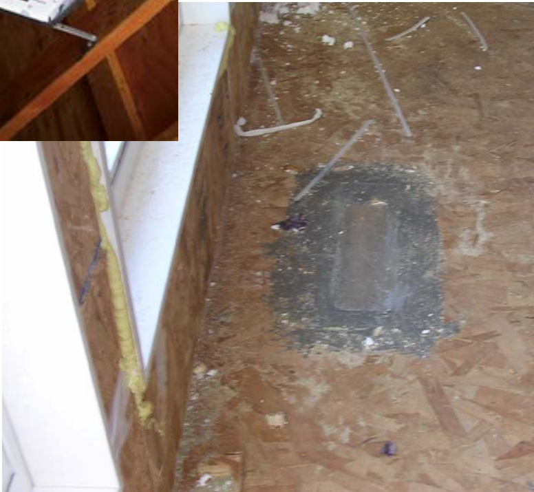
COVERING DUCT OPENINGS DURING CONSTRUCTION
