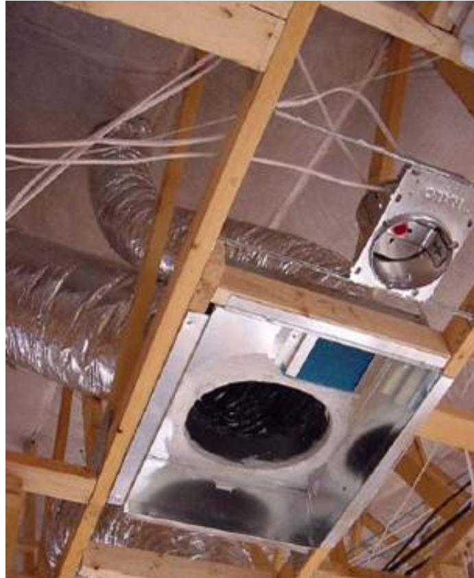
DUCTED FRESH AIR SUPPLY
