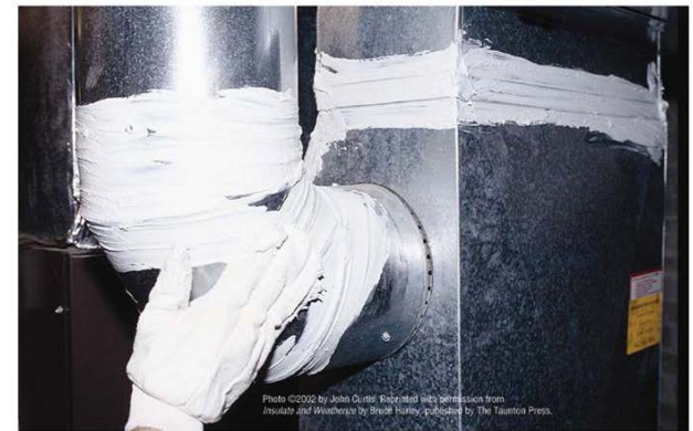
SEALING WITH MASTIC
