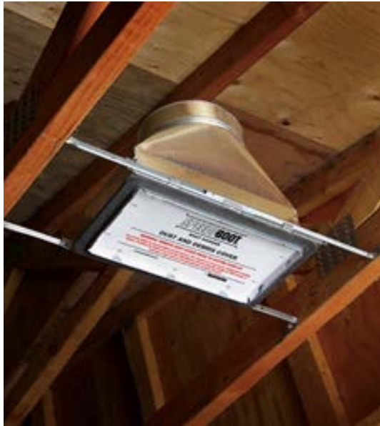
COVERING DUCT OPENINGS DURING CONSTRUCTION
