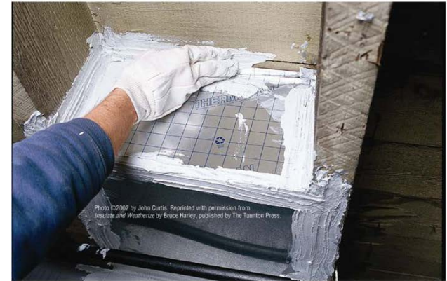
SEALING WITH MASTIC
