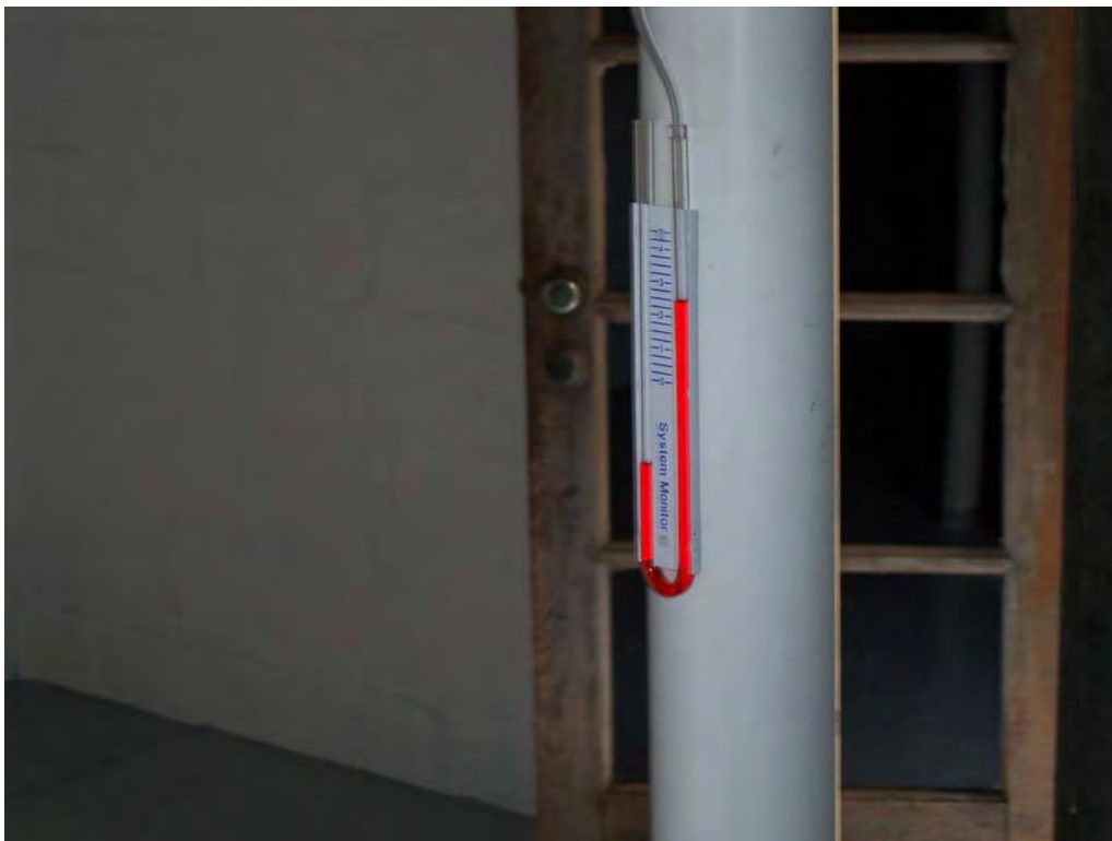
Photo 6 – VM system manometer mounted on vertical extraction pipe in west room of basement
