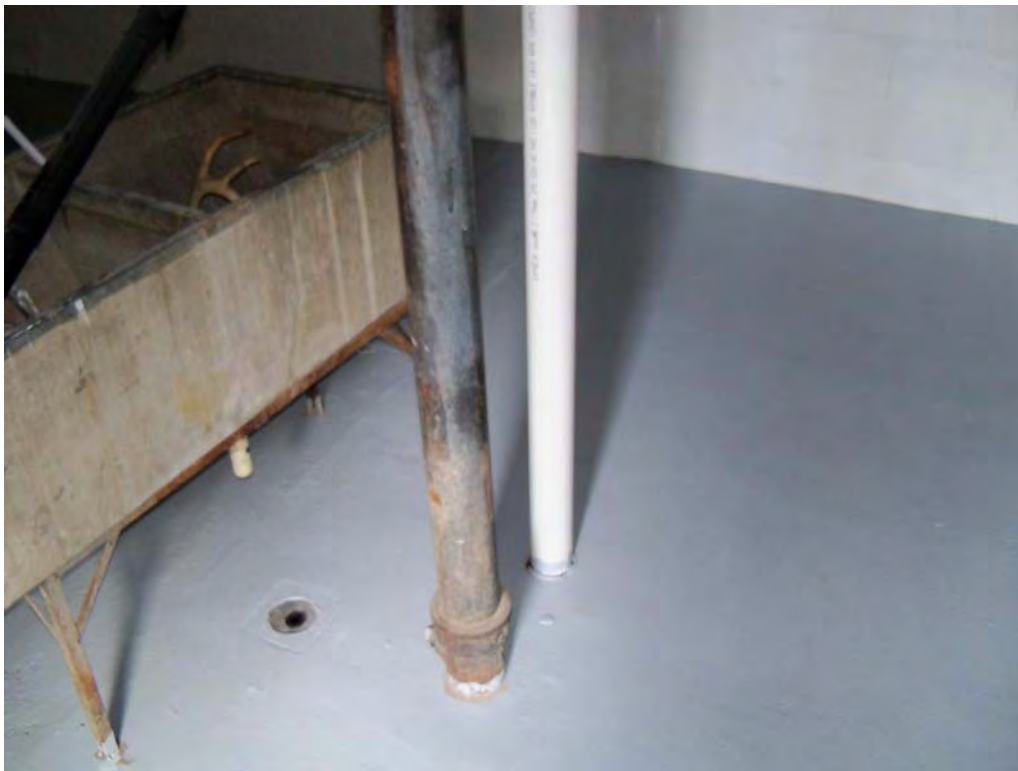
Photo 3 – VM extraction point and trapped drain in center of west basement room
