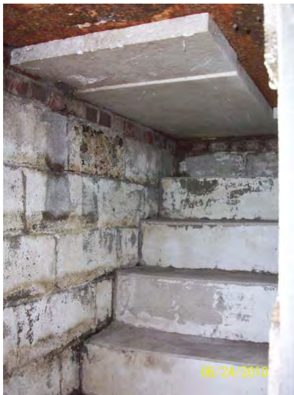
Photo 8 – Former exterior entrance stairs and concrete slab above
