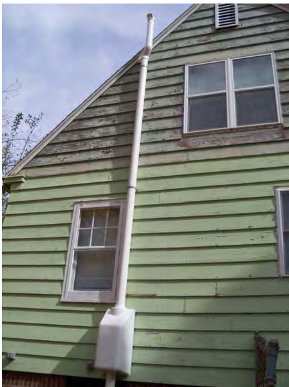
Photo 12 – West wall of residence, looking east, showing VM system fan housing and discharge piping
