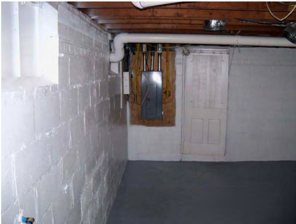
Photo 1 – West wall of basement, looking north, showing wall sealant, breaker box, doorway to former outside entrance and VM system header pipe exiting residence
