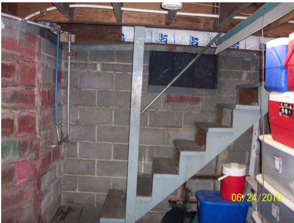
Photo 1 – Basement stairs and typical block wall construction
