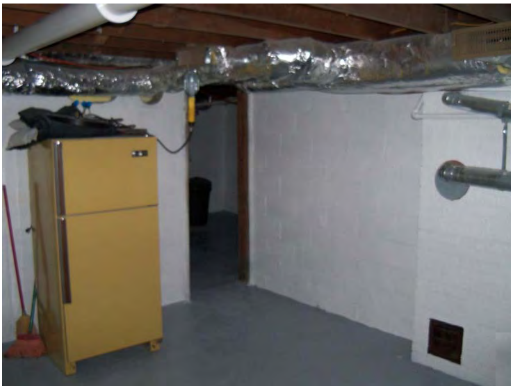
Photo 8 – South wall of center basement room, looking southeast, showing wall and floor sealant
