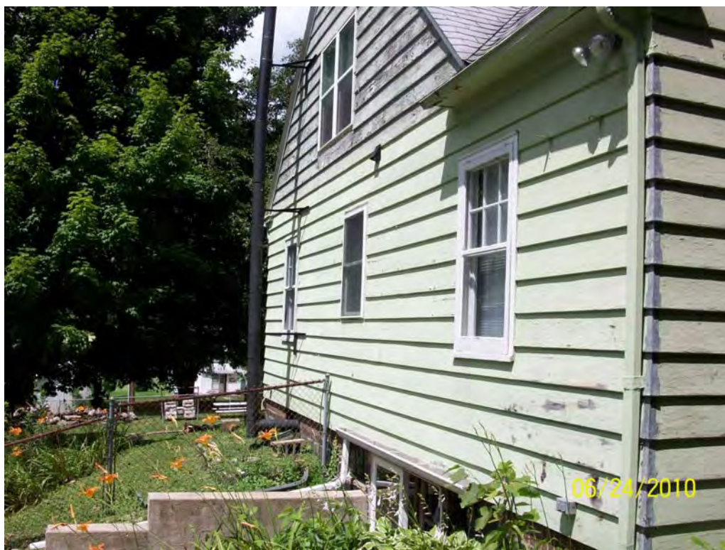
Photo 10 – Wood burning heater vent stack and proposed location of vent fan
