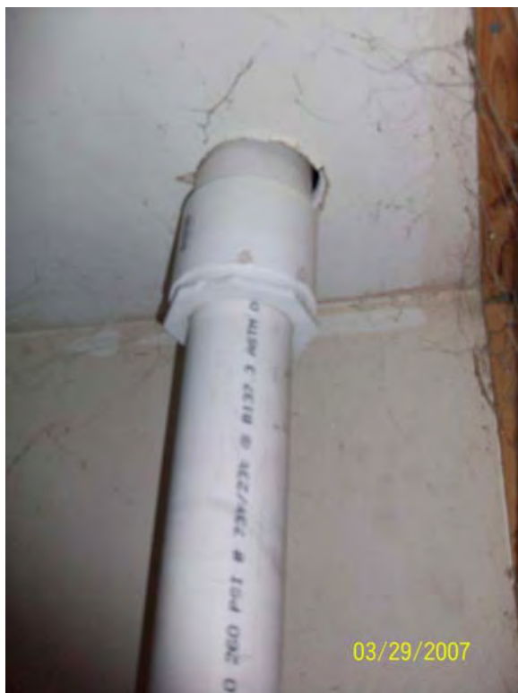
Photo 3 – VM system extraction pipe penetration through ceiling
