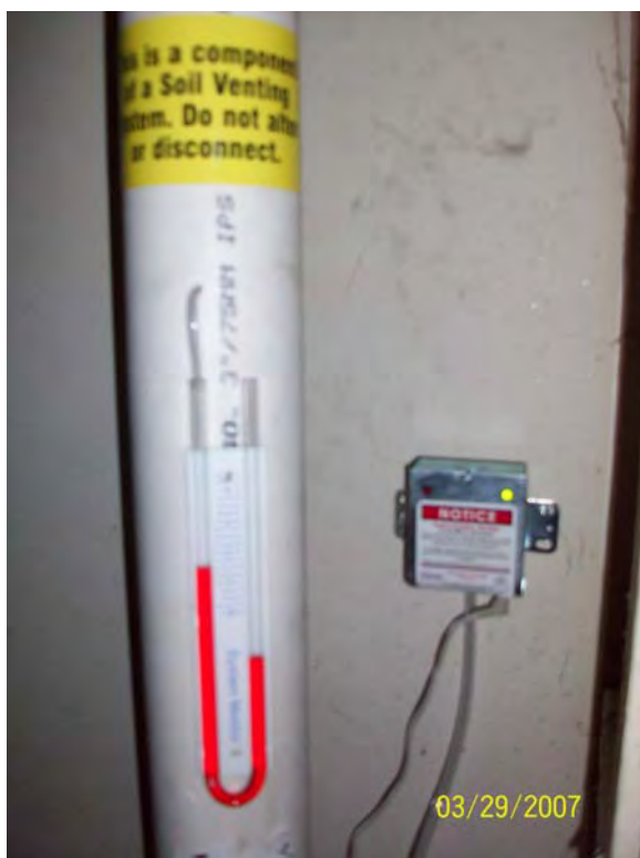
Photo 1 – VM system showing manometer, label and alarm
