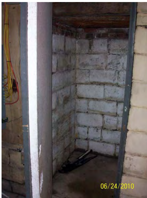
Photo 7 – Former exterior entrance - concrete slab currently seals entrance
