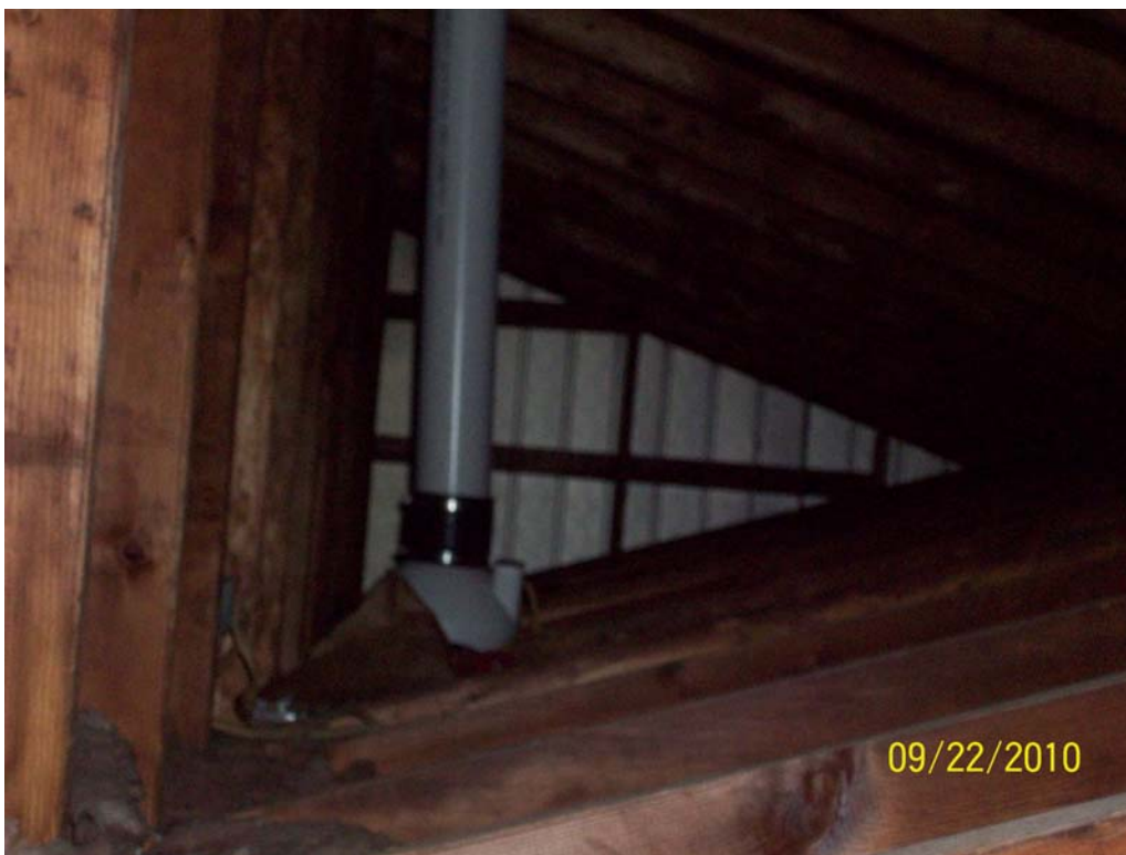
Photo 5 – VM system fan mounted in attic
