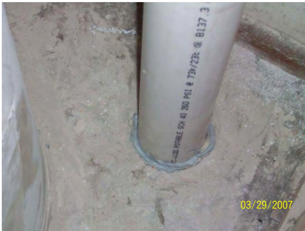
Photo 2 – VM system extraction point
