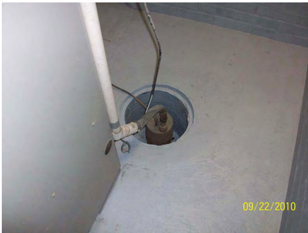
Photo 3 – Sealed sump next to furnace
