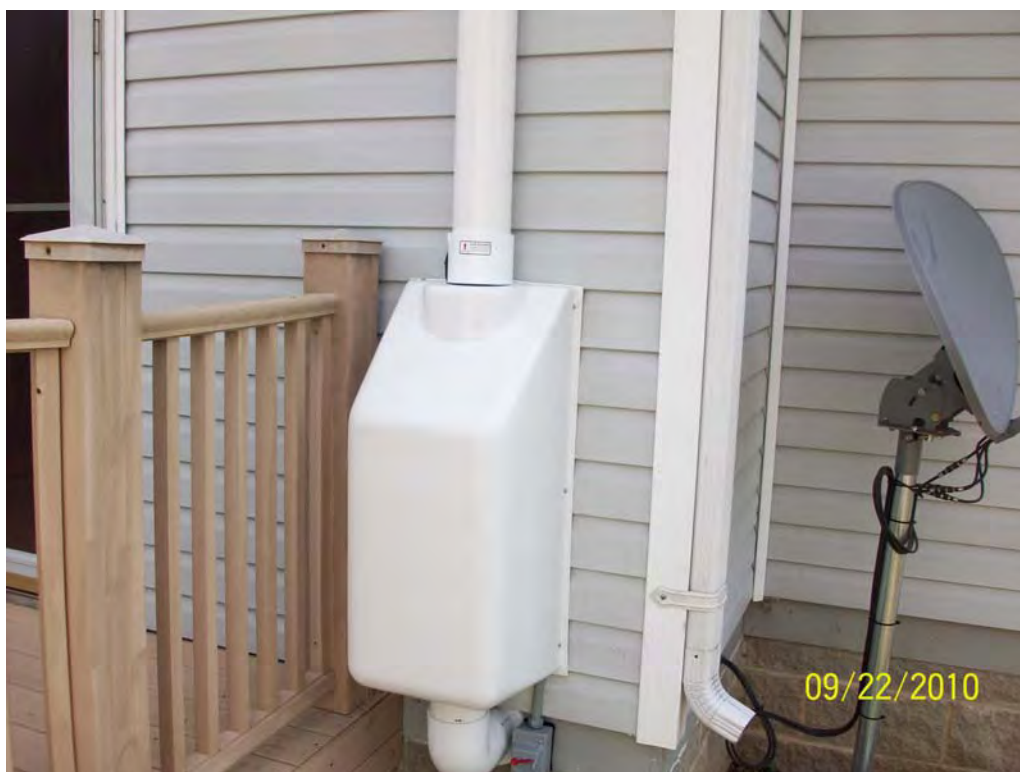
Photo 9 – VM fan and housing on west wall of residence
