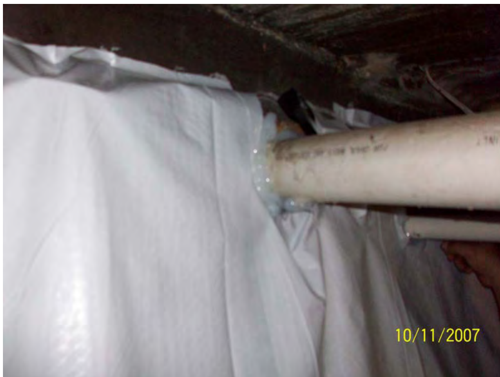
Photo 11 – Sealed utility penetration in north wall
