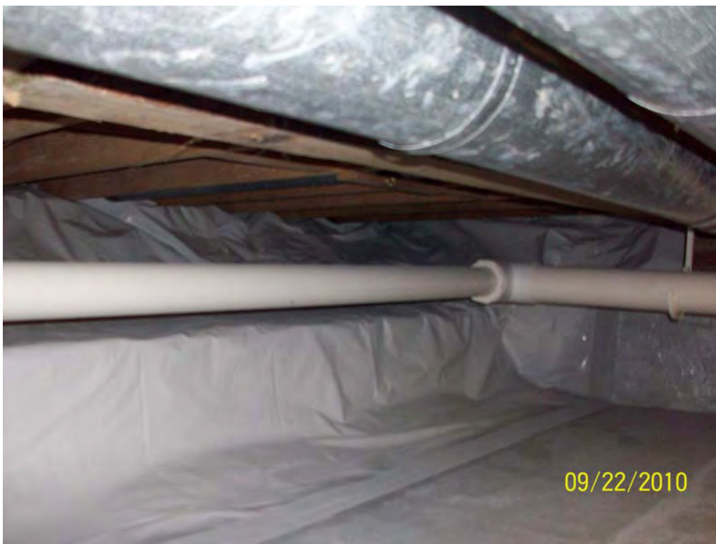
Photo 5 – VM header pipe in east crawlspace
