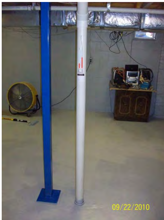
Photo 2 – VM system extraction point in center of basement
