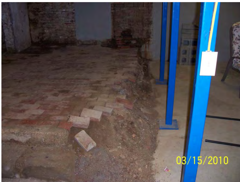
Photo 3 - Floor elevation/construction type difference in middle of basement
