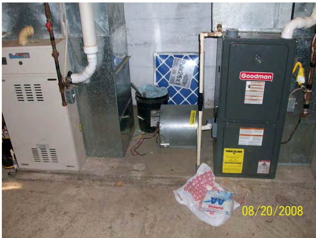
Photo 4 – Furnaces in basement
