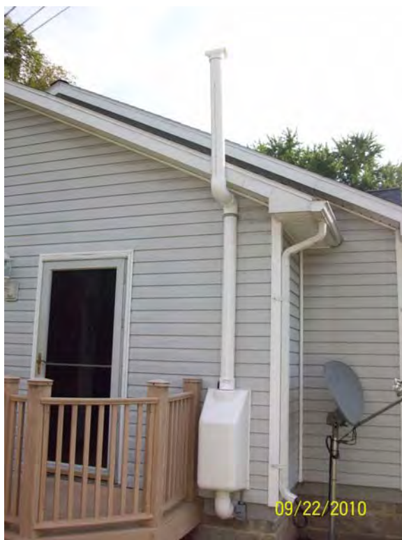
Photo 10 – Exterior portion of VM system
