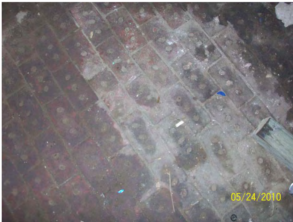
Photo 10 - Brick floor construction – partial coverage in basement
