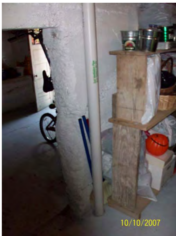
Photo 8 – VM extraction point just outside of the south room
