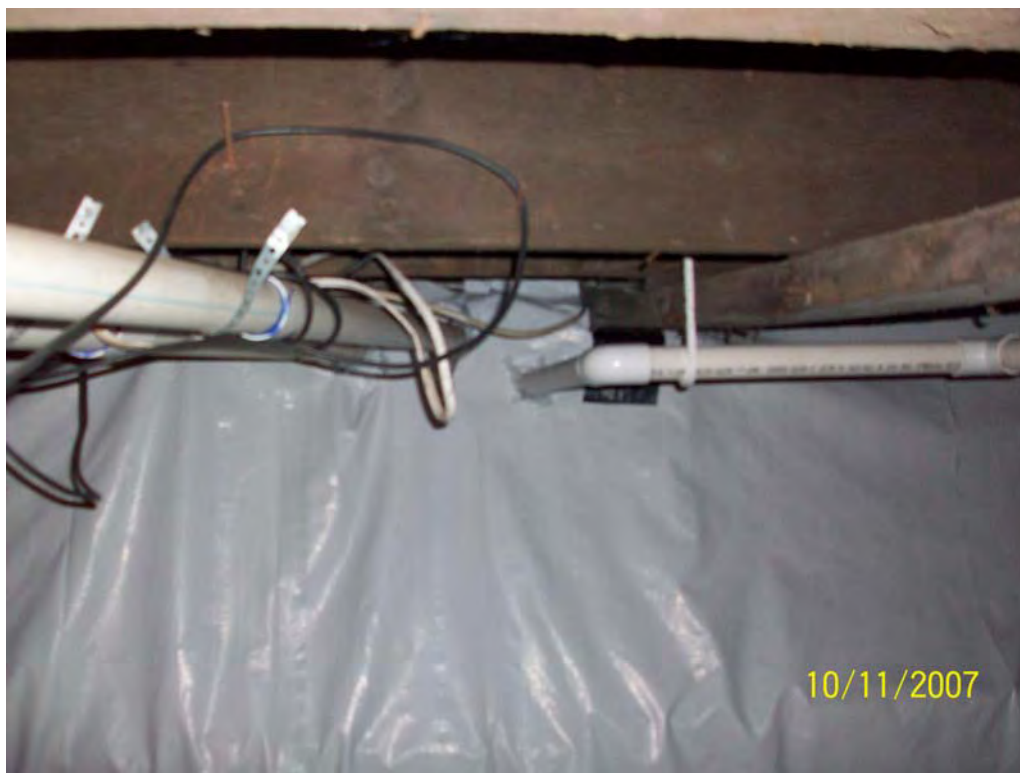
Photo 9 – Sump discharge pipe penetrating east wall of basement
