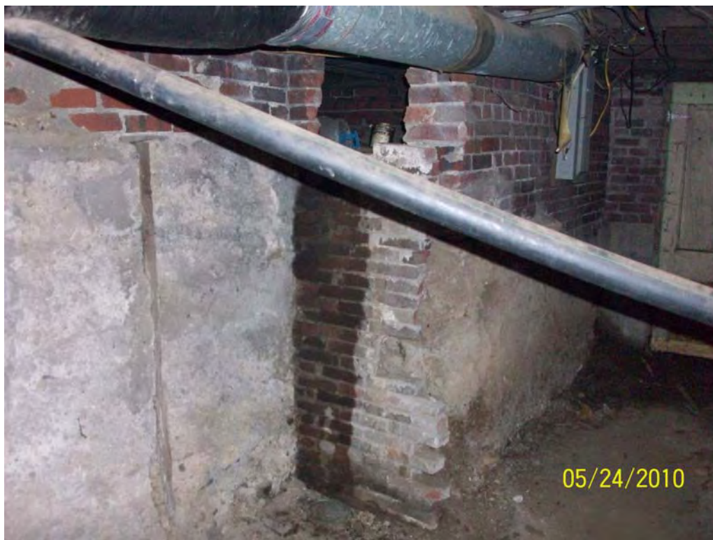
Photo 5 – Entrance to southwest crawlspace; water intrusion staining
