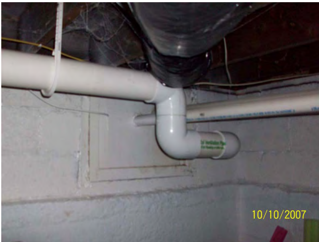
Photo 4 – VM system manifold pipe penetration through north wall of basement
