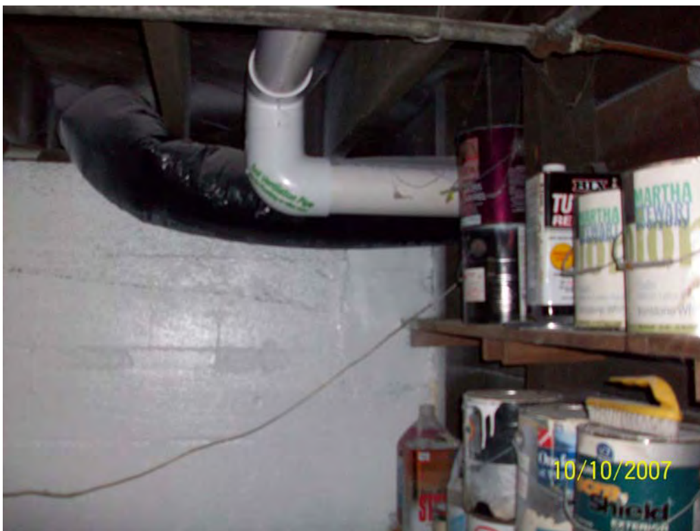
Photo 3 – VM system manifold piping showing labeling
