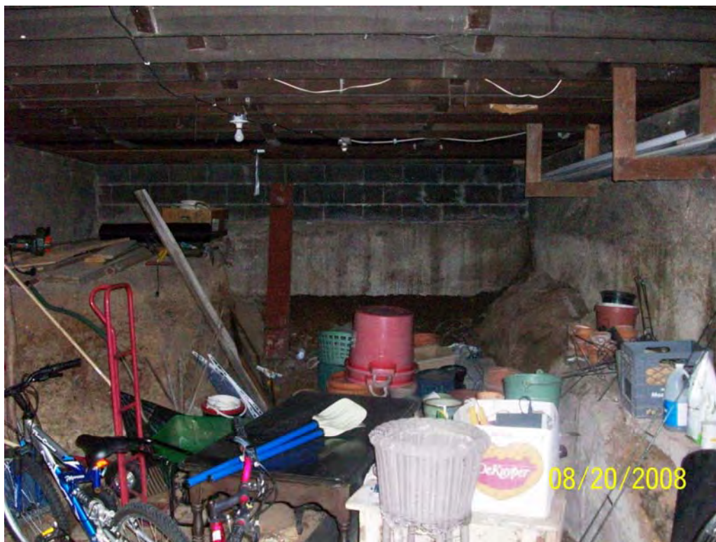
Photo 2 – South room of basement showing damaged wall and exposed soil
