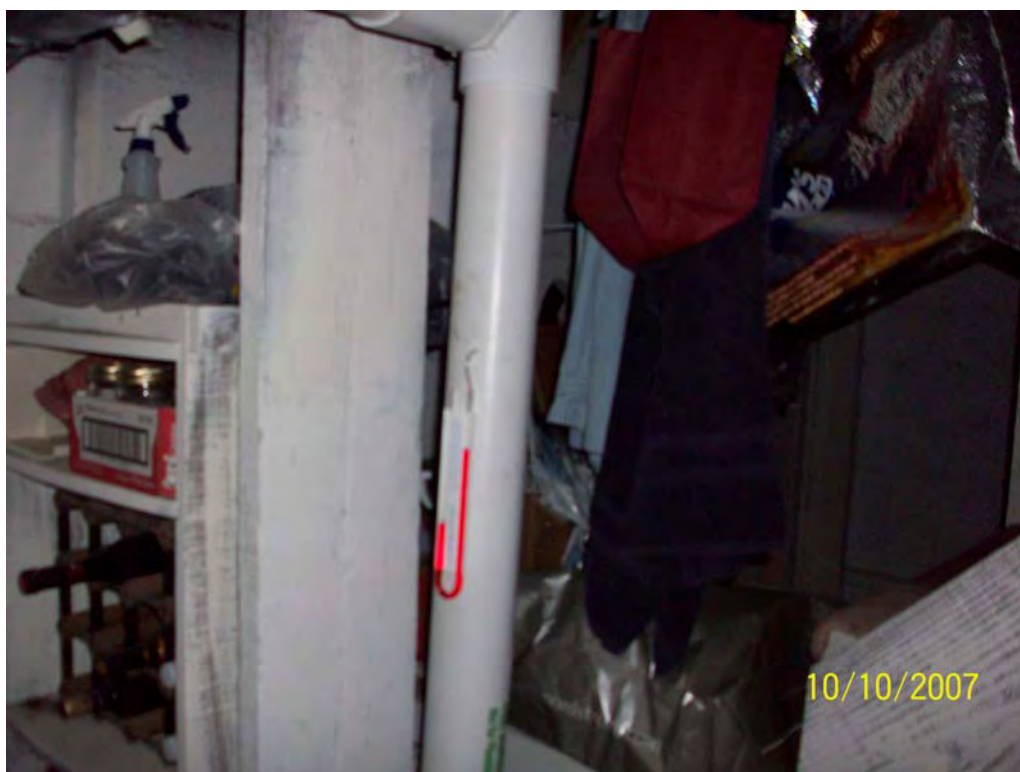
Photo 7 – VM system manometer
