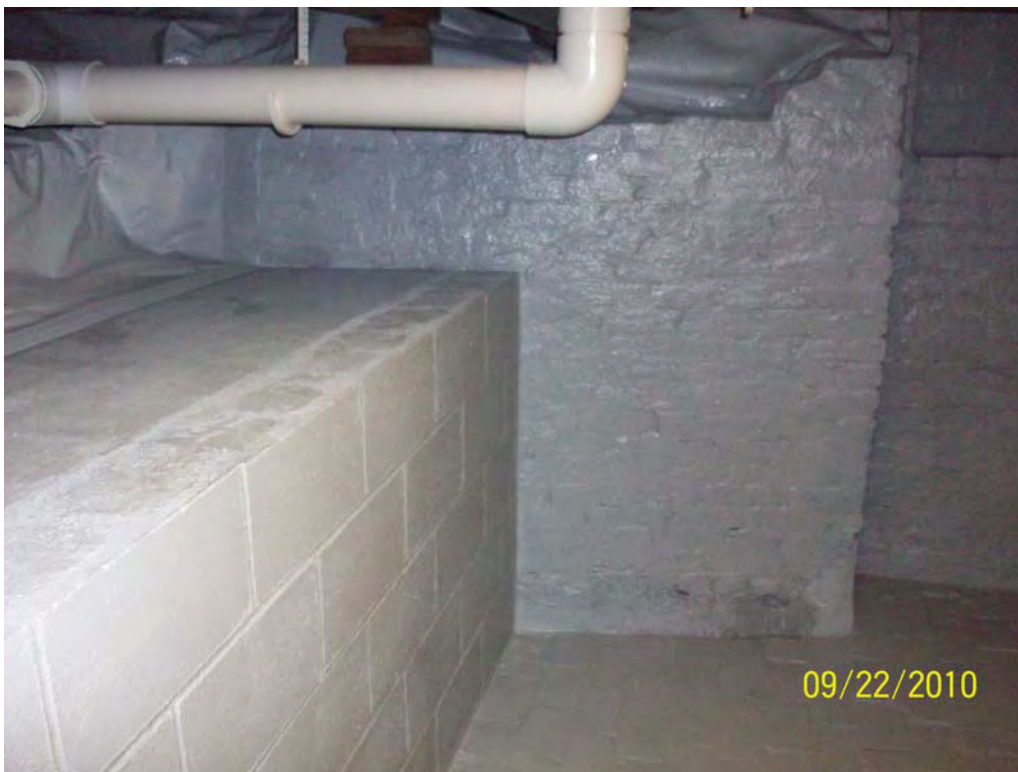
Photo 6 – Southeast corner of basement showing VM header pipe and sealing of walls and floor
