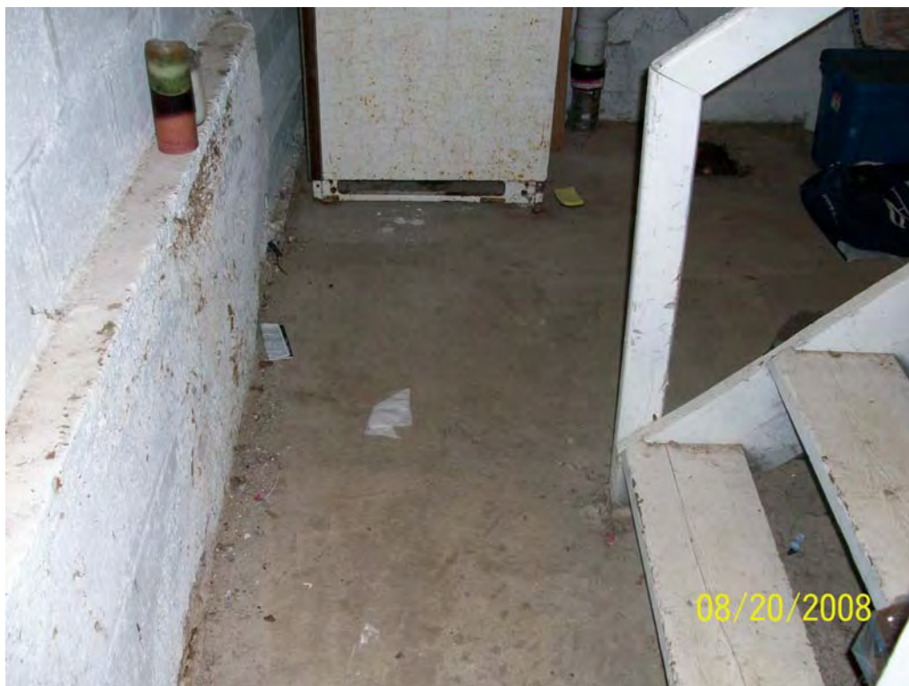
Photo 6 – Basic wall construction is cinder block and poured concrete; concrete floor slab
