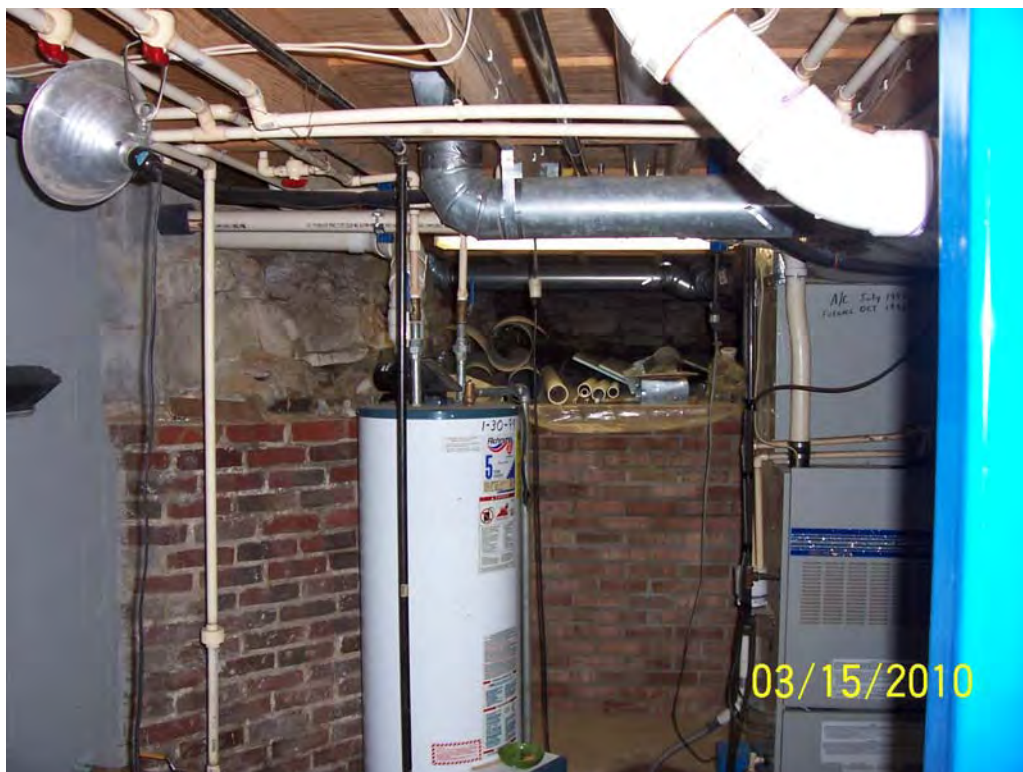
Photo 4 - Brick, block, and stone wall construction near furnace and water heater on concrete slab
