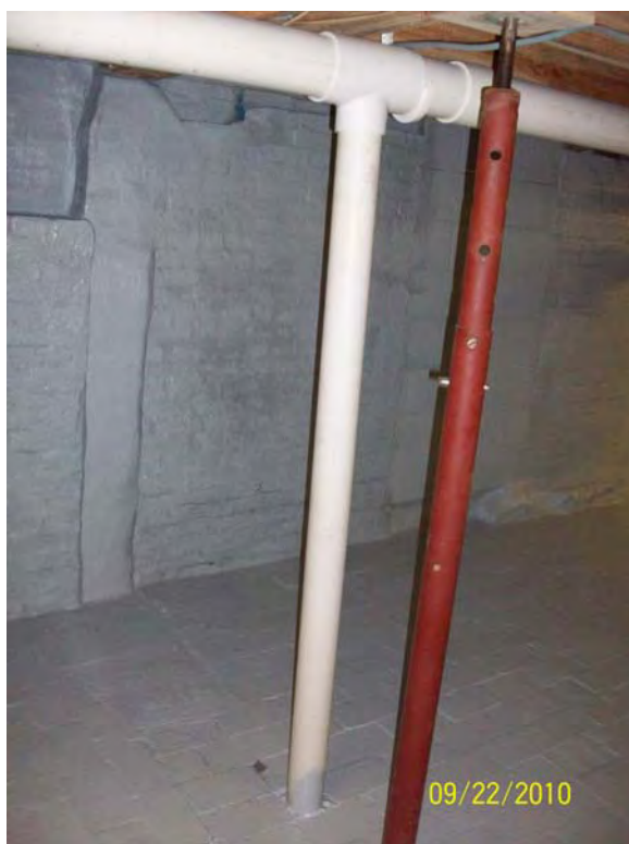
Photo 7 – VM extraction point along south wall of basement
