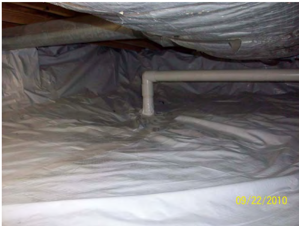
Photo 4 – Membrane in east crawlspace and submembrane extraction point
