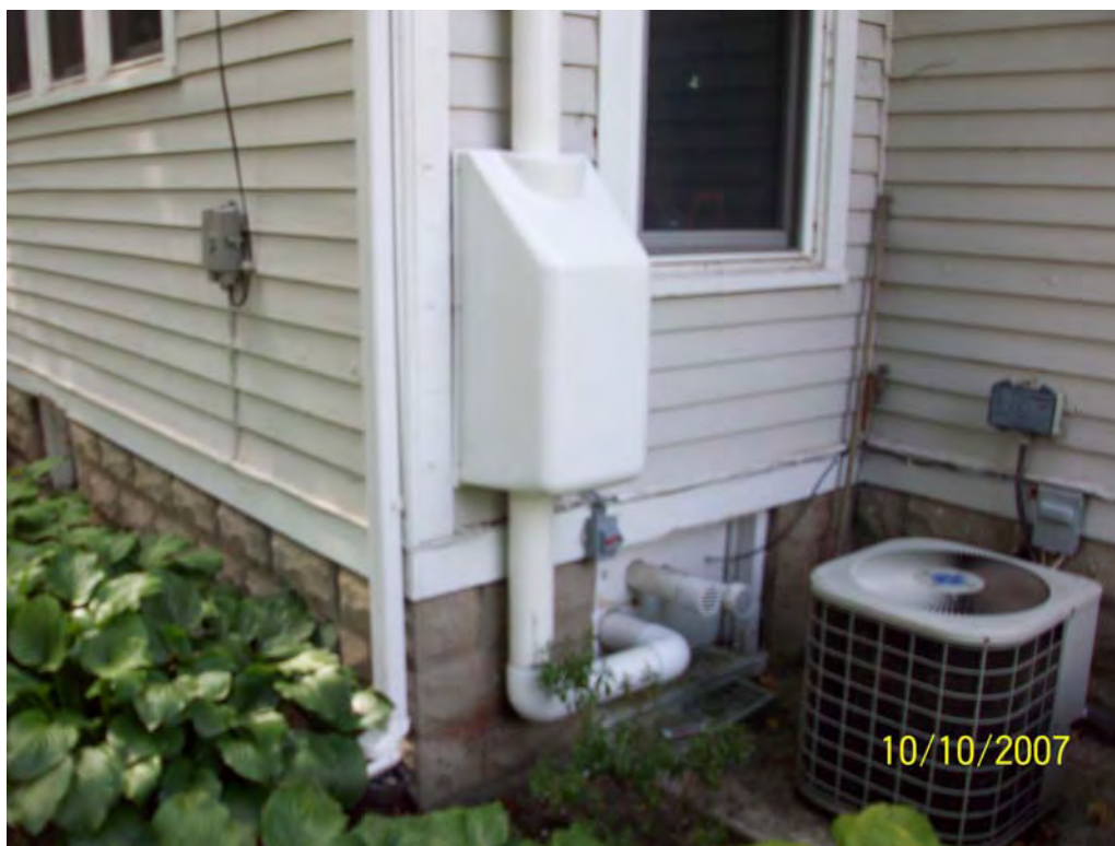
Photo 10 – System fan and cover on north wall of residence
