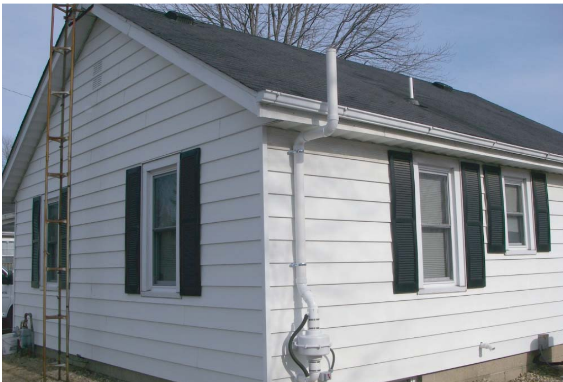
PHOTOGRAPH 1: Mitigation system fan and discharge. The fan creates a vacuum under the concrete floor slab or crawlspace. The vacuum draws vapors from under your home into a PVC pipe system that is vented above the structure. The fan must be "on" and running 24 hours a day to ensure the system is operating effectively. The vent pipe must be clear of obstructions at all times. This includes caps and covers.
