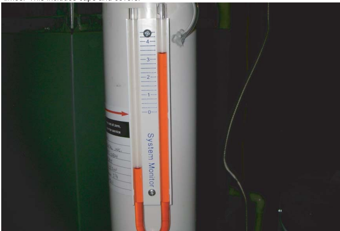
PHOTOGRAPH 2: Manometer (vacuum pressure gauge) to monitor system performance; the "u-tube" will display a reading greater than zero (the system is designed to operate between 1-4 inches of water column) on the side where the small poly tubing is located when the system is operating effectively.
