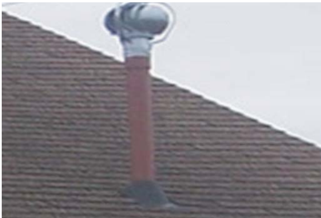
PHOTOGRAPH 10: A wind turbine is used for a passive mitigation system. The turbine should spin freely at times to ensure the system is effective. Any roof penetration is sealed using roof flashing when required.
