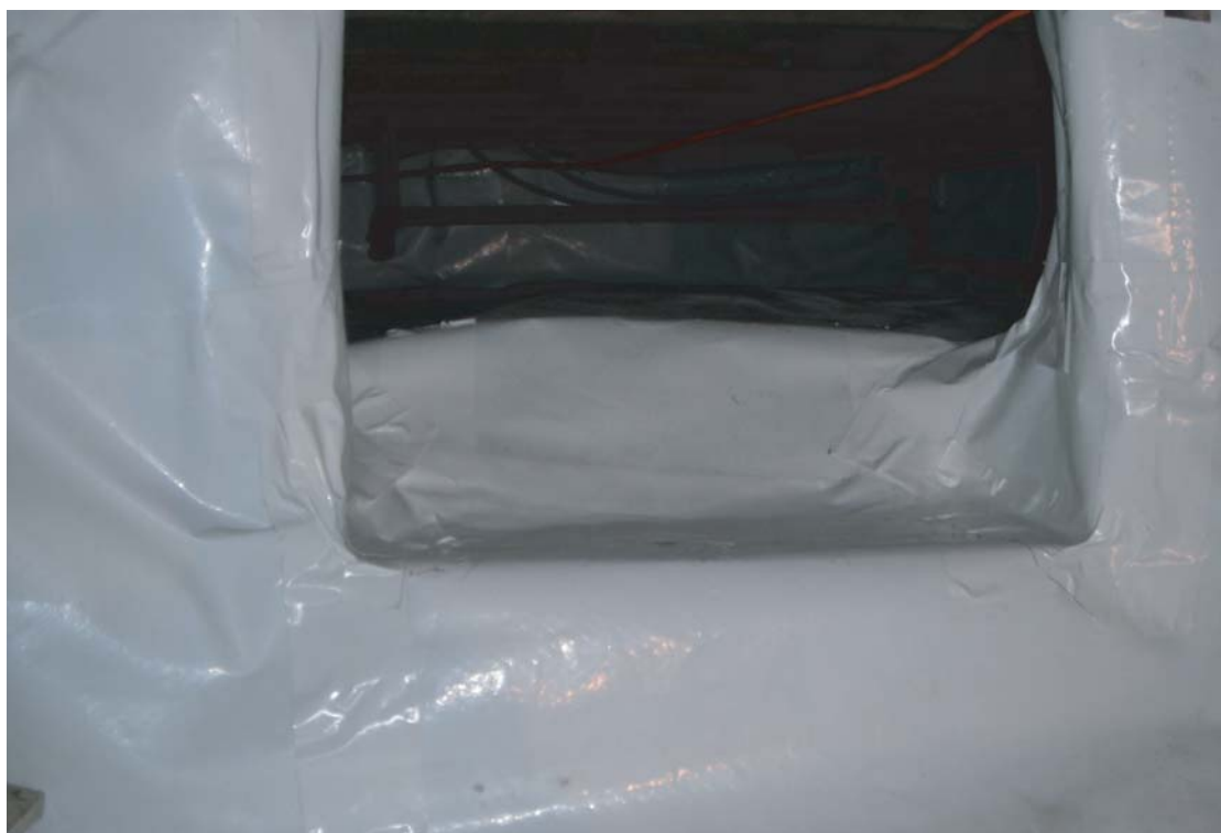
PHOTOGRAPH 8: Crawlspace sealed using polyethylene sheeting. Sheeting is sealed at the perimeter of the crawlspace and around any protrusions. Polyethylene sheeting installed in areas accessible to foot traffic or used for storage are protected using foam padding and untreated plywood.
