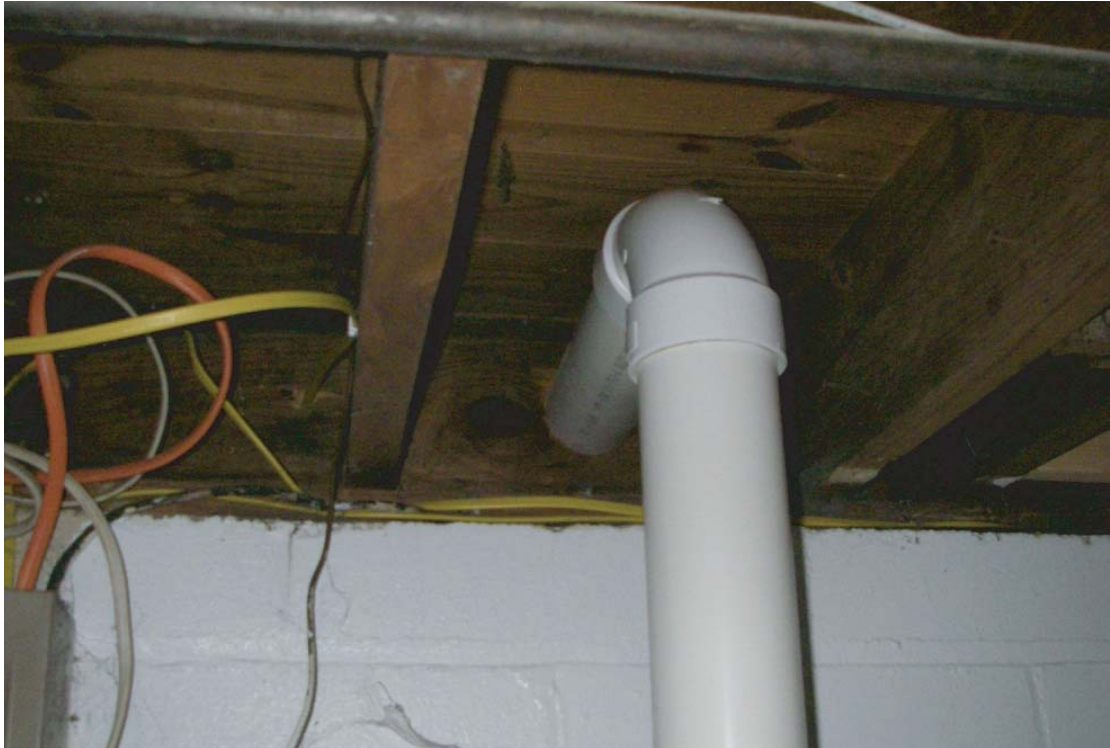
PHOTOGRAPH 4: Overhead extraction piping to exterior fan or turbine. Horizontal piping is installed at a 1% slope back the extraction point. Pipe is supported every 8 feet on vertical piping, every 6 feet on horizontal piping, and near the discharge.
