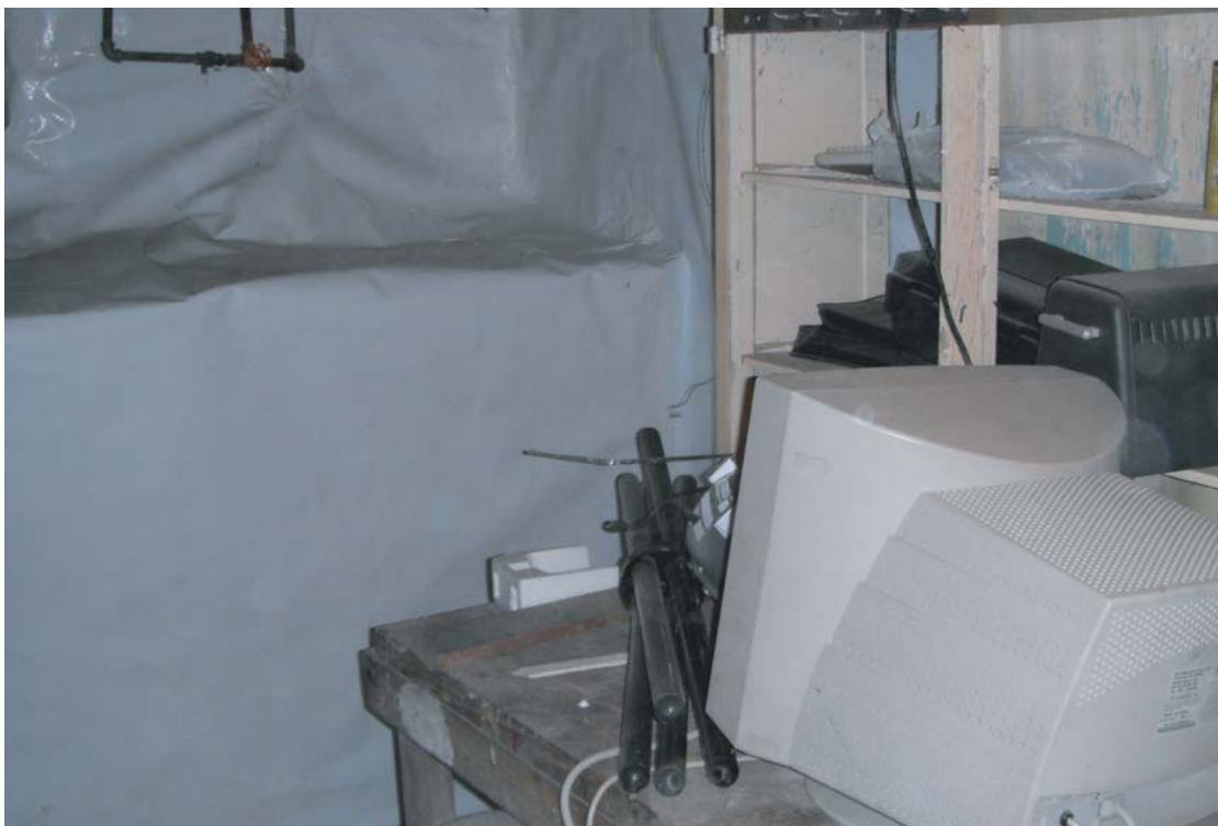
PHOTOGRAPH 6: Liner used to seal damaged wall. Liner should be maintained to ensure vapors are captured by the mitigation system.
