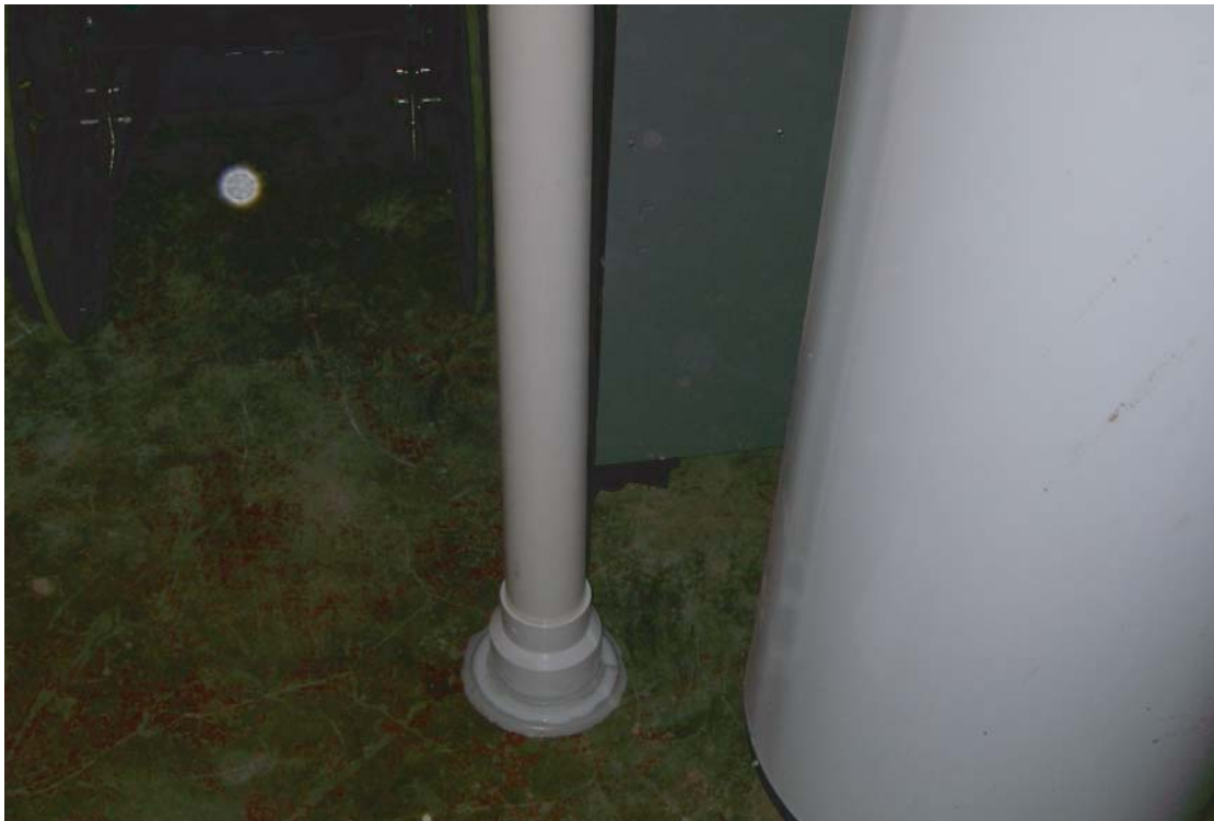
PHOTOGRAPH 3: Extraction point. PVC piping extends through the concrete slab floor or crawl-space liner. PVC pipe extends upward to an overhead piping system routed to an "in-line" fan or turbine used to vent the sub-slab space.
