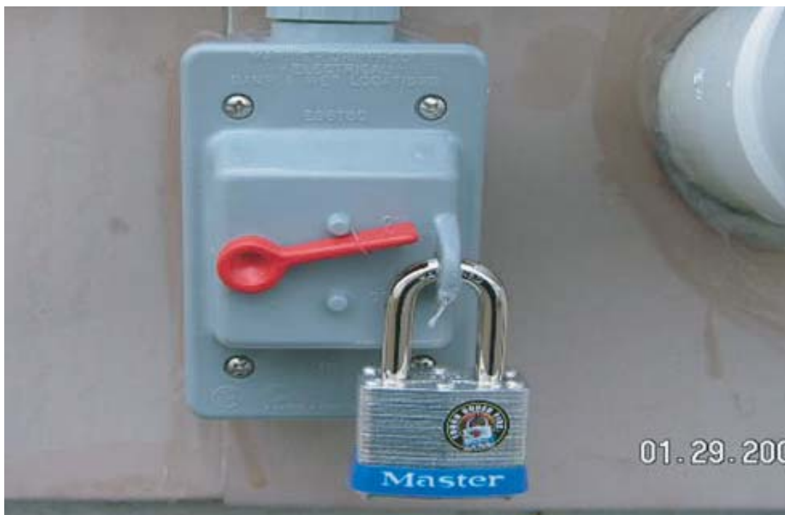
PHOTOGRAPH 9: Padlock located on the “on/off” switch located on the exterior of your structure. This system is designed to run in the “on” position at all times to ensure it is effective.
