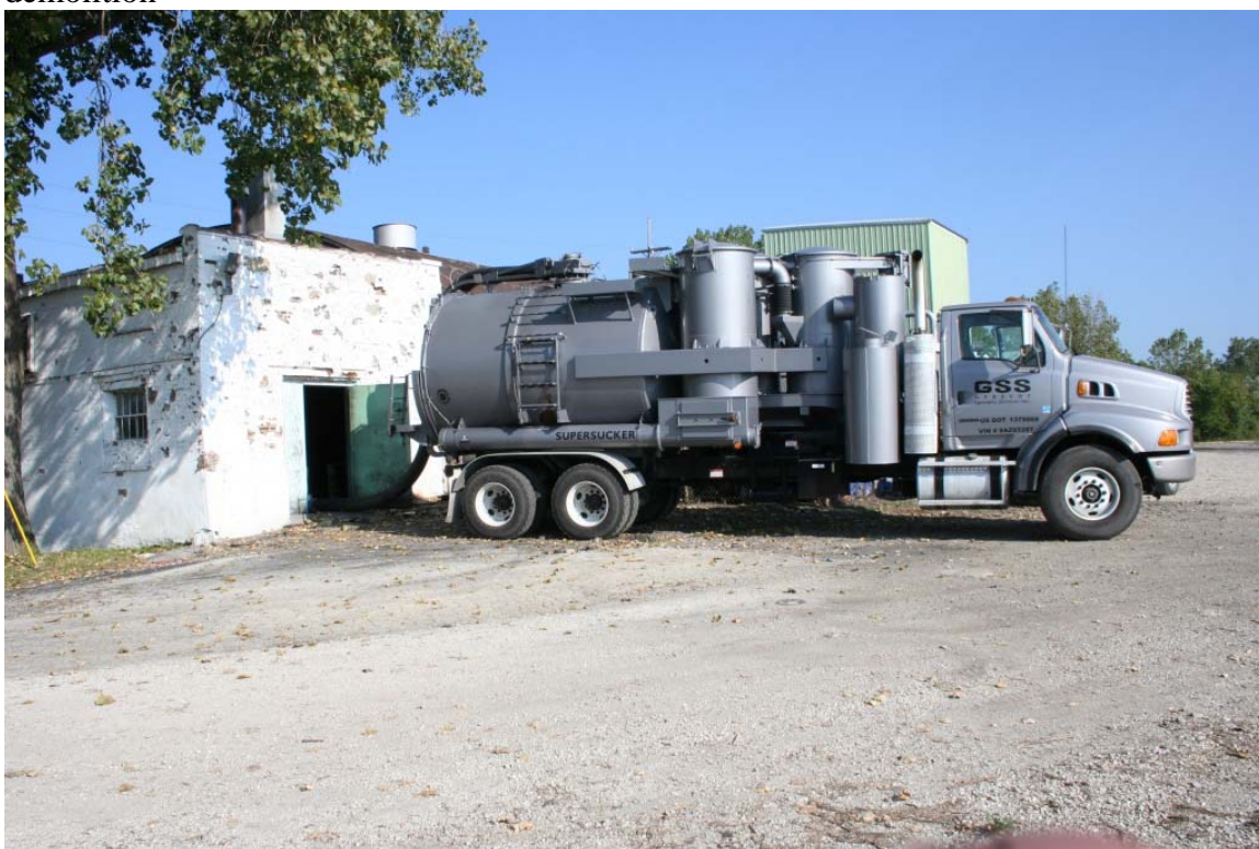
Photo 4 – Hazmat contractor vacuum truck removing foundry sand/dust residues for disposal prior to demolition
