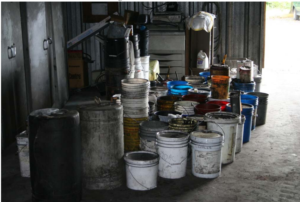
Photo 1 – Staging of petroleum/chemical containers awaiting decanting/removal prior to demolition
