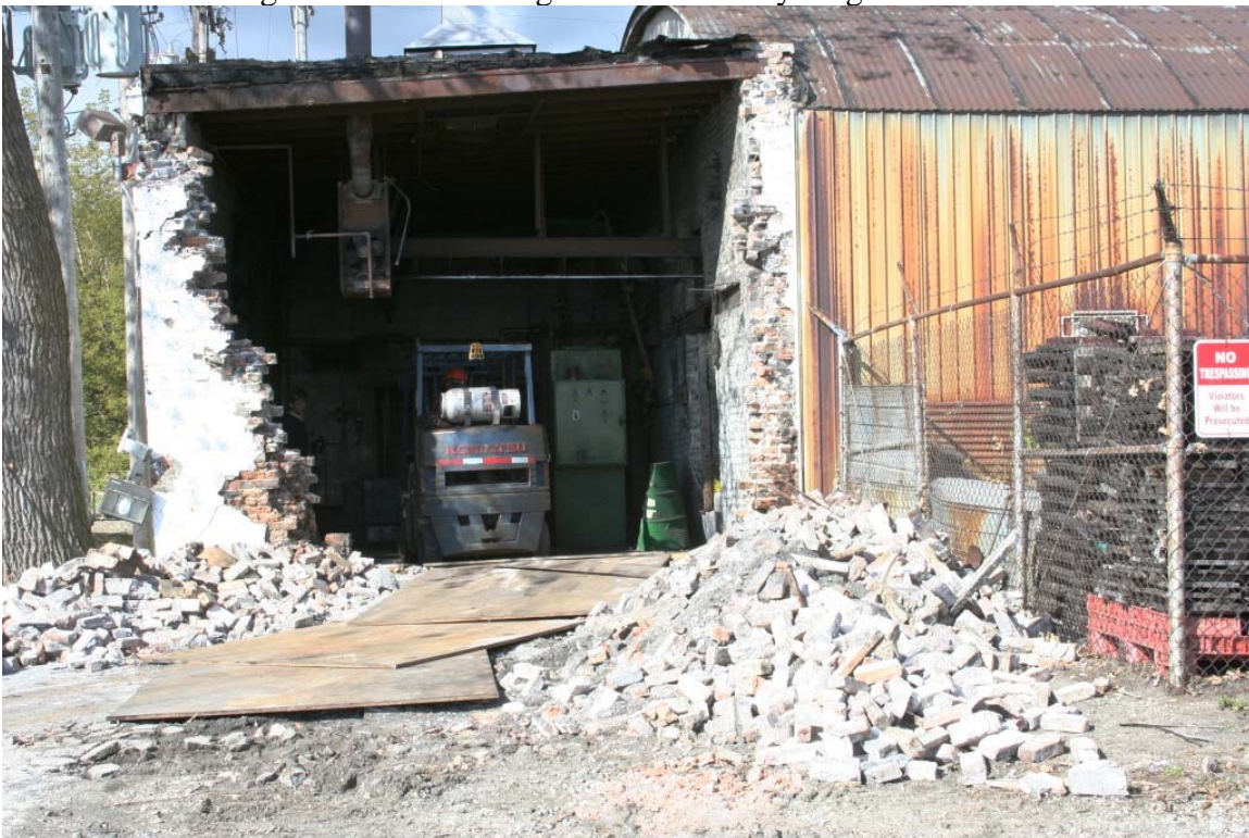
Photo 14– Partial demolition of southeast wall for access to foundry equipment
