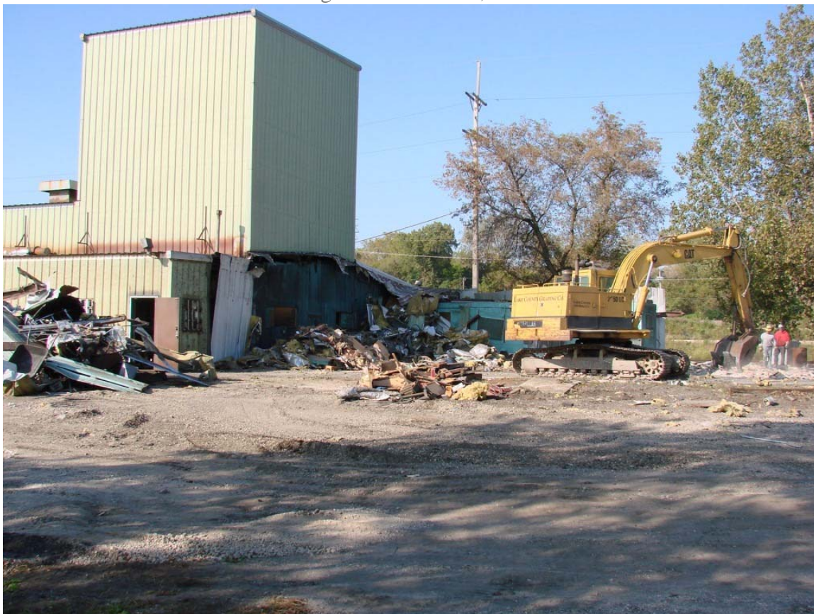
Photo 11 – Separation and sorting of building material for recycling
