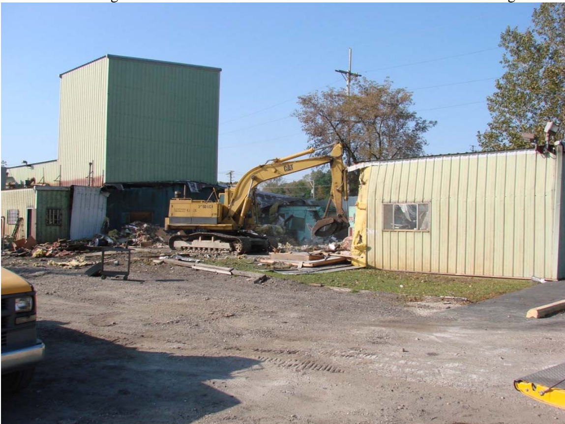
Photo 10 – Continuing demolition of north building and recycling of building materials
