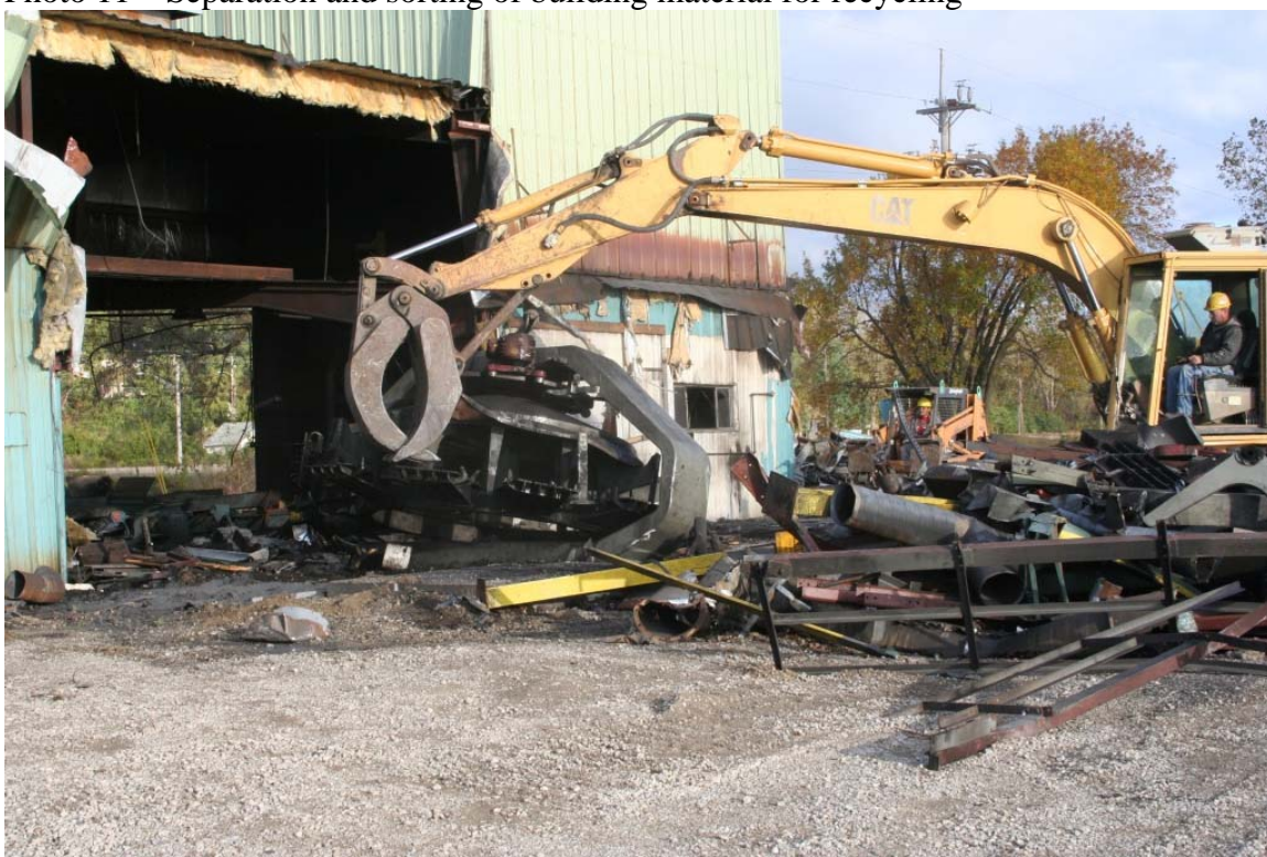
Photo 12 – Removal of foundry equipment for recycling/salvage
