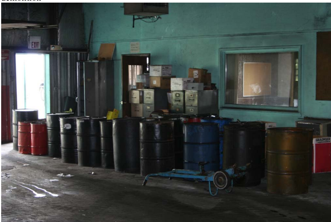
Photo 2 – Staging of petroleum containers awaiting decanting/removal prior to demolition
