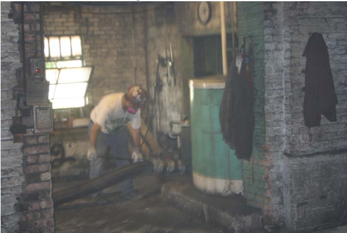
Photo 5 – Hazmat contractor removing interior foundry sand via vacuum methods
