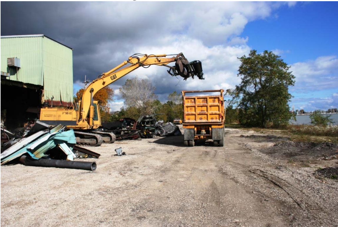
Photo 13 – Loading truck with building material for recycling
