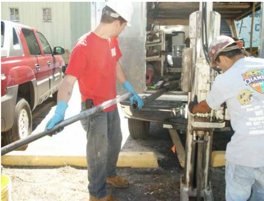
Photo 5 – View of soil core sample being removed from tooling.
