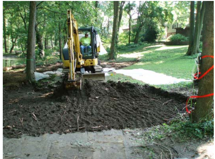
Above: Where grids were excavated, care was taken to protect high quality trees. Consideration was provided to the proximity of excavation as well as compaction of soil with over-sized equipment. For that reason, much of the equipment used was relatively small. Although the smaller equipment required additional time, countless trees were saved.
