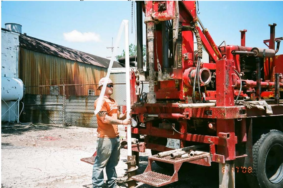
Photo 4 – View of monitoring well installation at LSF-MW-02.
