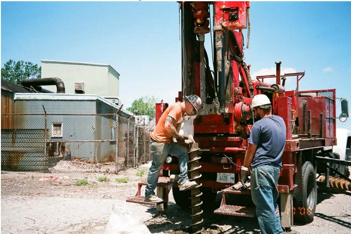
Photo 5 – View of installation of artificial sand pack at LSF-MW-02.
