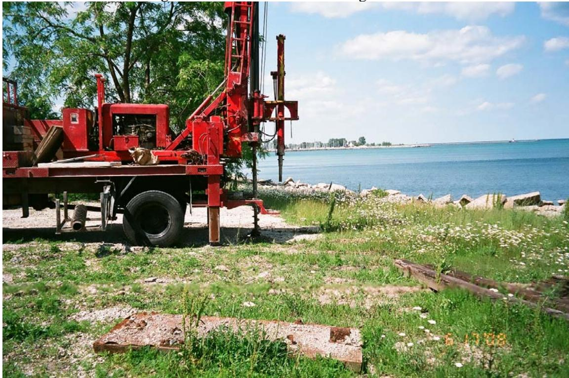
Photo 2 – View of drilling methods with solid stem augurs at LSF-MW-03 offset.
