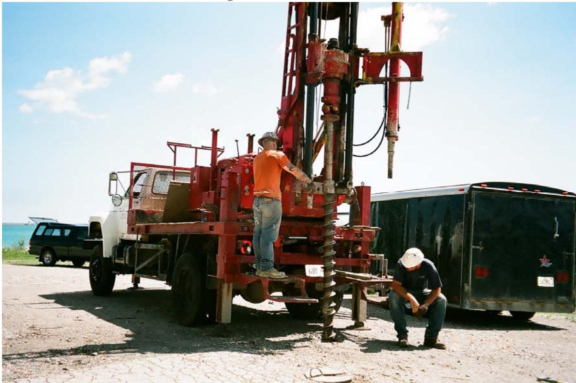
Photo 3 – View of drilling methods using hollow stem augurs at LSF-MW-02.
