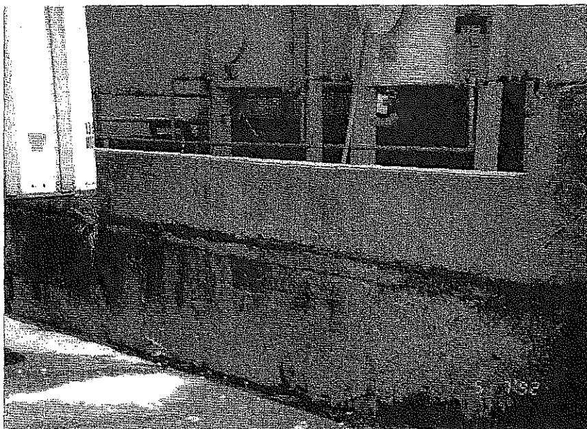
Photograph No. 10 Orientation: West Description: The dike surrounding the Solvent Blending Tanks. Note the deterioration of the unit.
