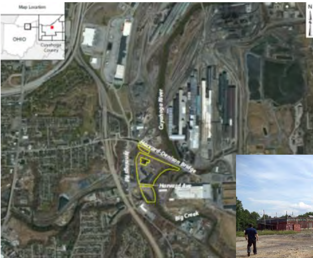
Left – Aerial map shows BASF site at 1000 Harvard Ave. outlined in yellow.
