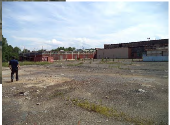
Below – Photo shows some of the buildings on the BASF site in Cleveland.
