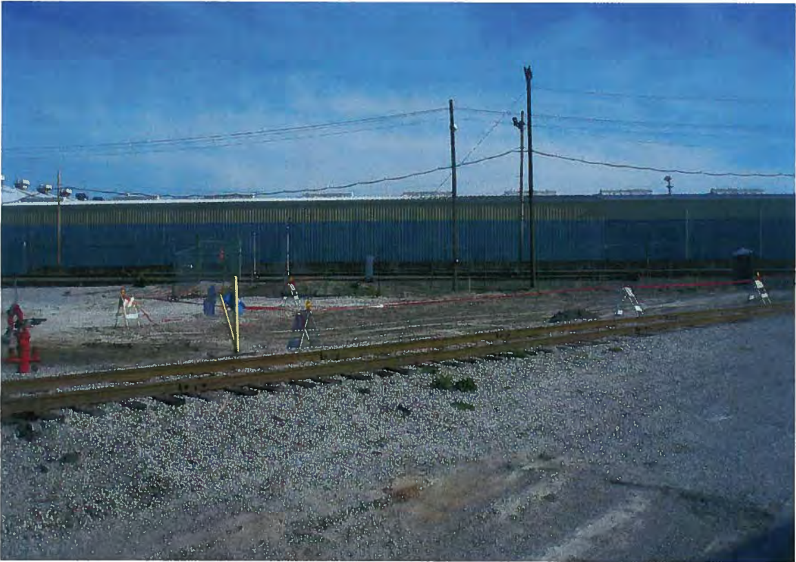
Photo # 30 Backfill of S0609 (borings B-61/B-67/B-78)
