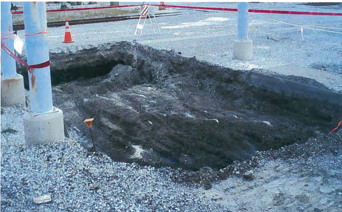
Photo # 2 Former PCB Warehouse excavation.
