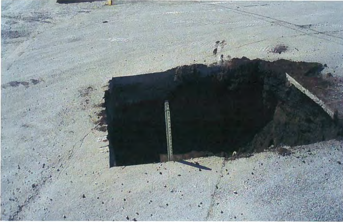
Photo # 9 S0607 excavation (boring B-49)
