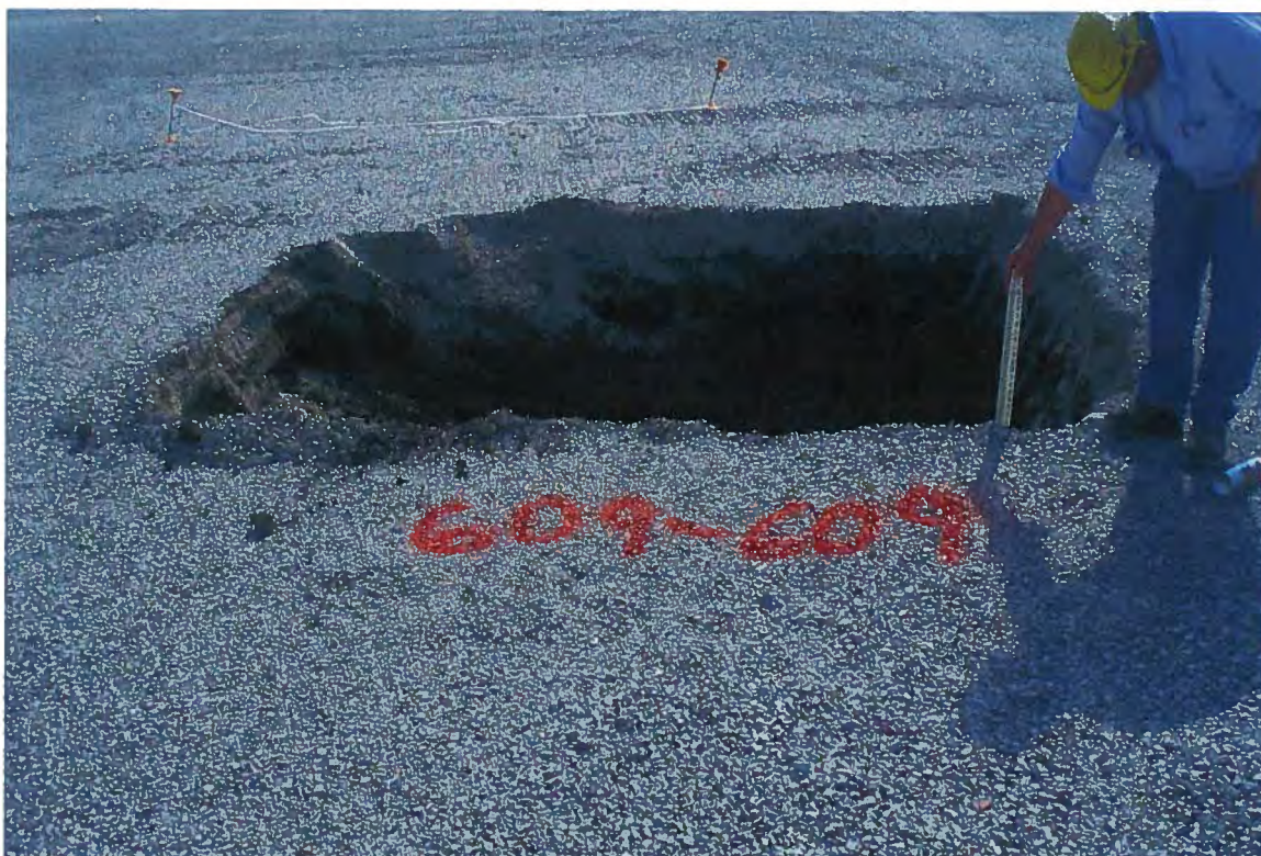
Photo # 43 S0609 excavation (boring B-609).
