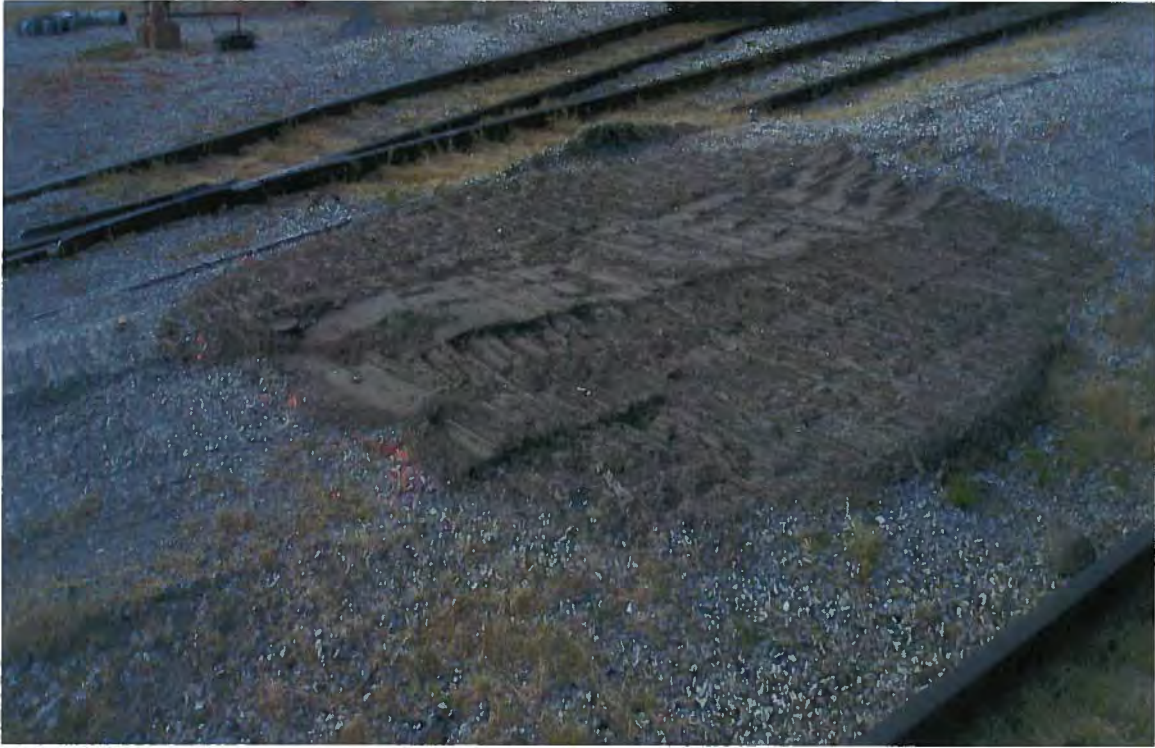
Photo # 25 Backfill of S0608/CT-1 (boring B-36).
