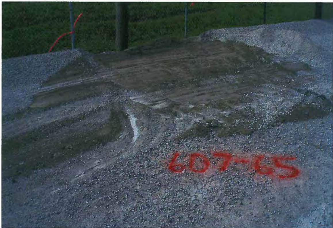
Photo # 16 Backfill of S0607 (boring B-65)
