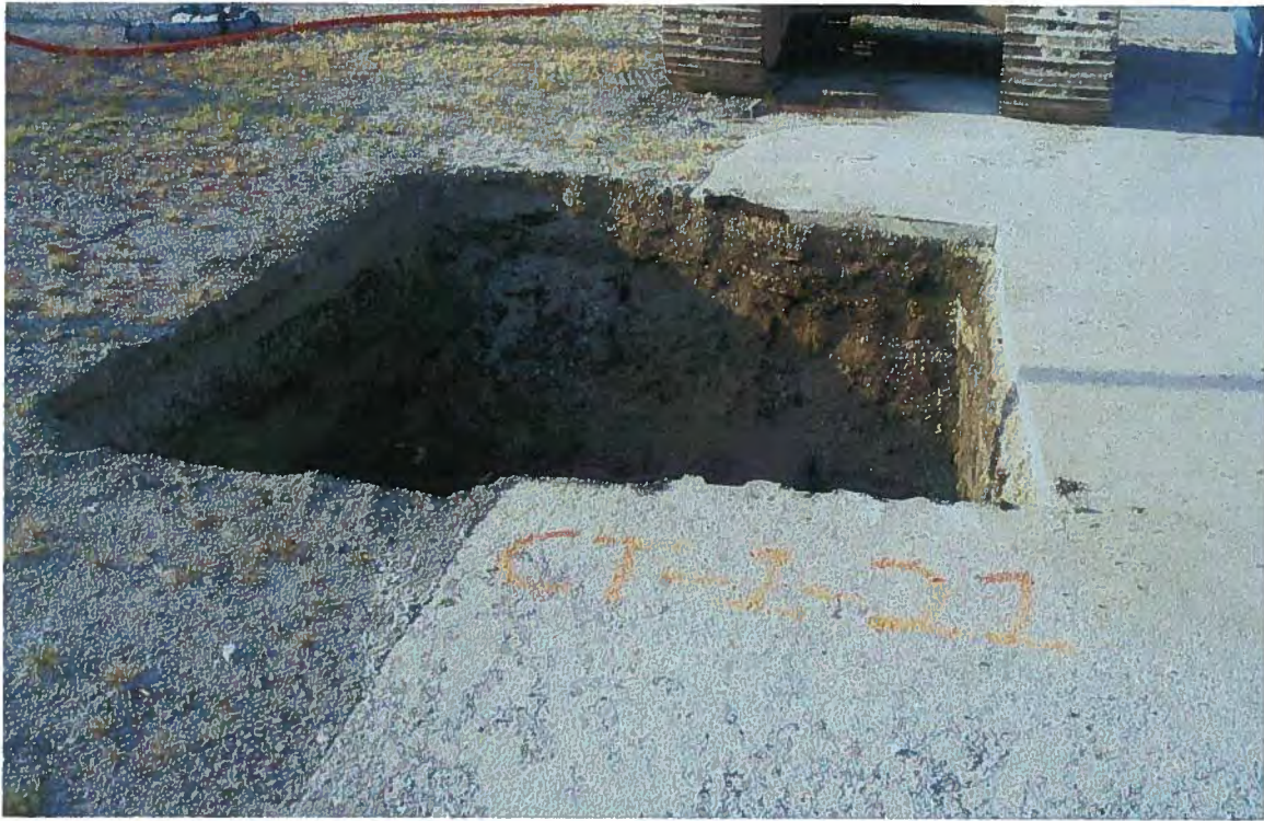
Photo # 17 S0608/CT-1 excavation (boring CT-1-21).
