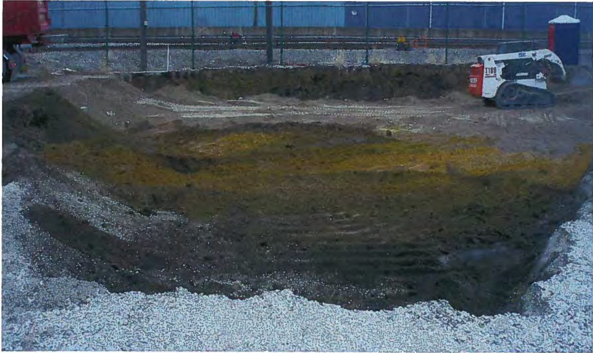
Photo # 29 S0609 excavation (borings B-61/B-67/B-78).
