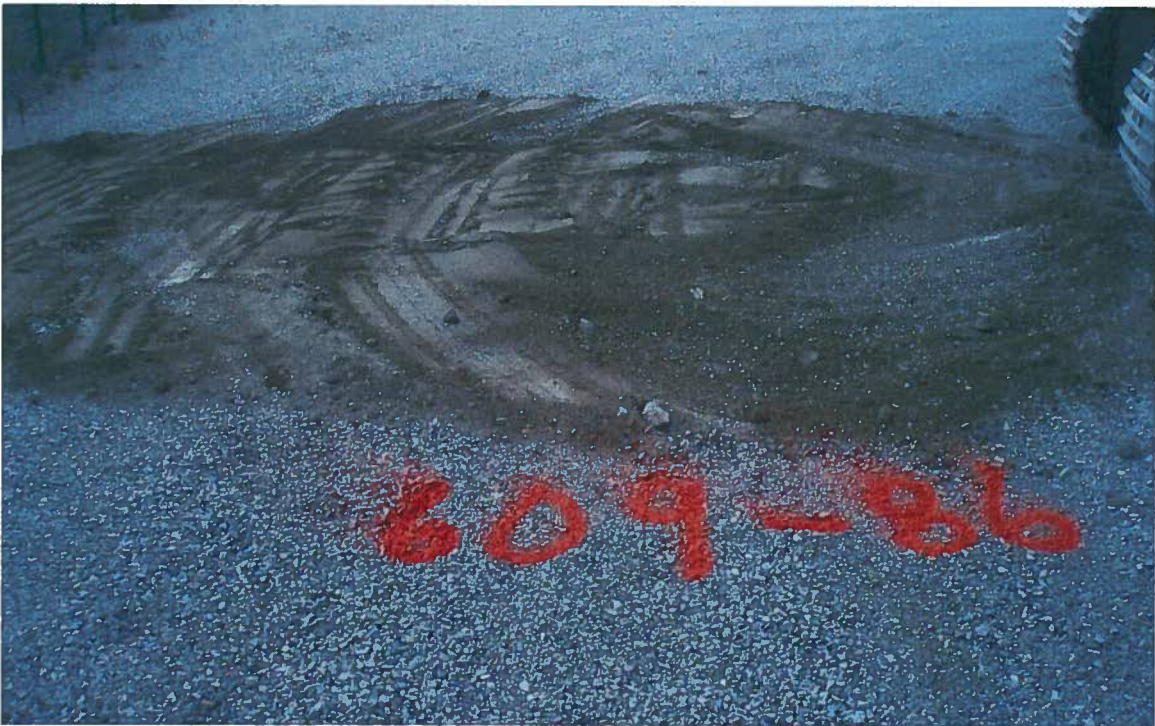
Photo # 42 Backfill of S0609 (boring B-86).
