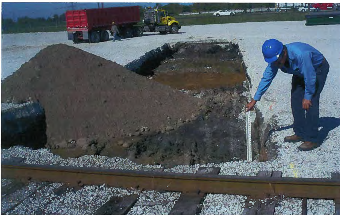
Photo # 35 S0609 excavation (borings B-18/B-28/B-36/B-44).
