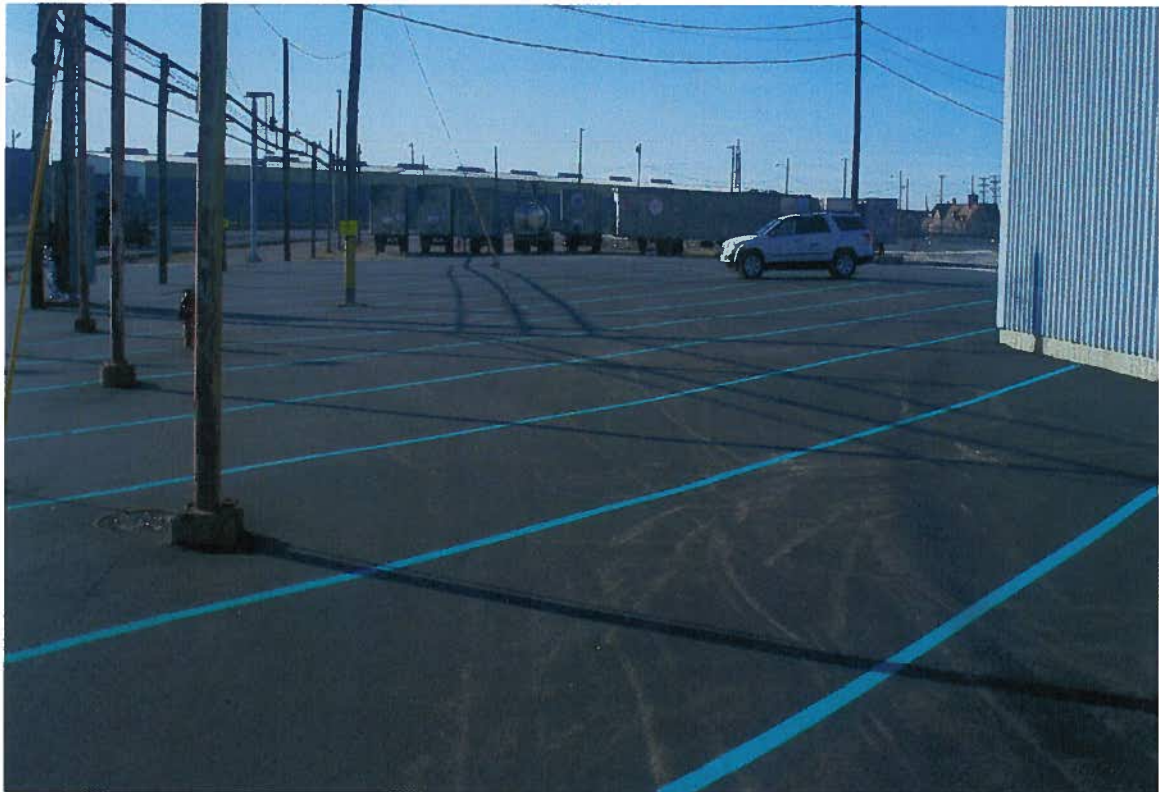
Photo # 28 S0608/CT-1 area following paving activities.
