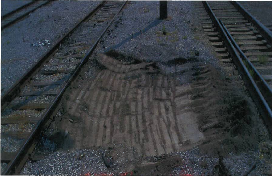
Photo # 27 Backfill of S0608/CT-1 (boring B-45).
