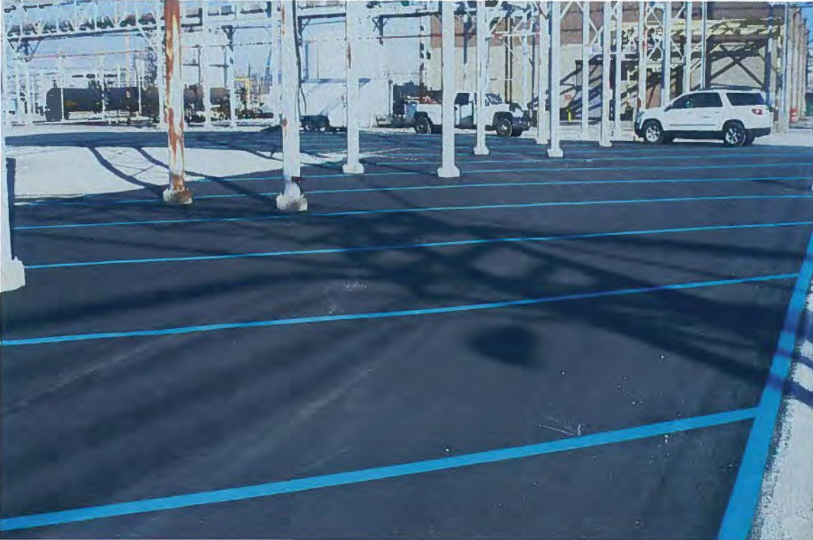
Photo # 4 Former PCB Warehouse area following paving activities.
