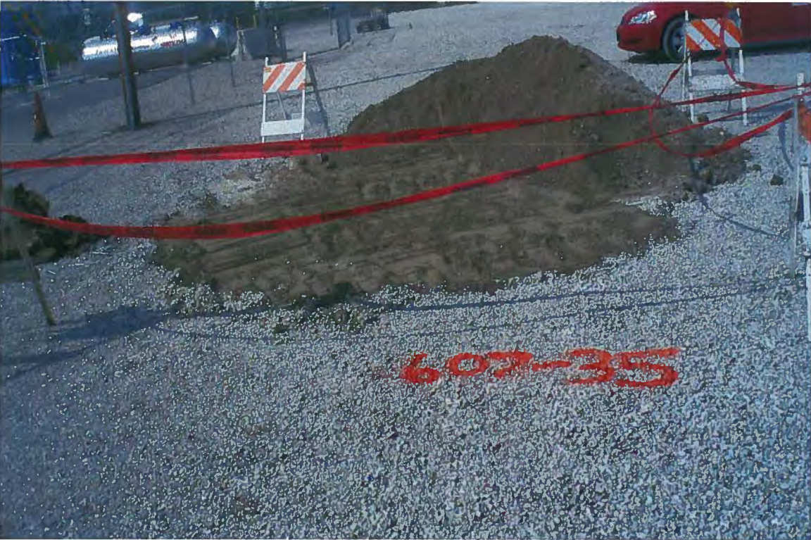
Photo # 8 Backfill of S0607 excavation (boring B-35)
