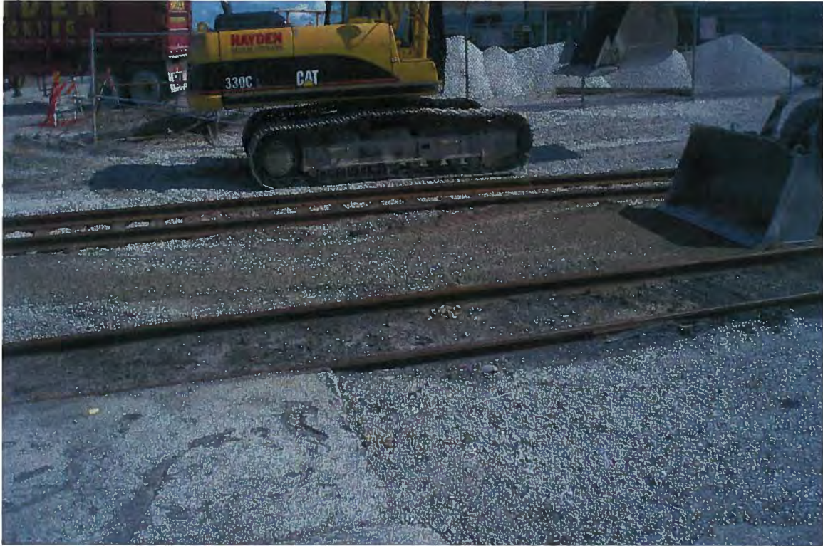
Photo # 47 Backfill of S0715 (boring B-47).
