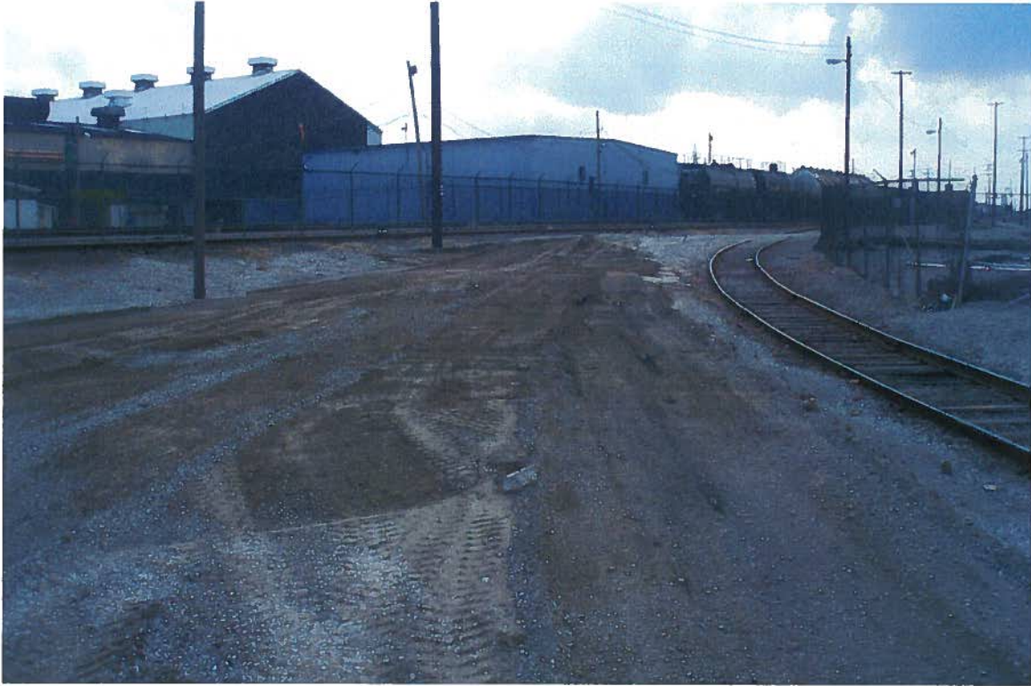
Photo # 49 Backfill of S0715 (borings B-9/B-20/B-25/B-66).
