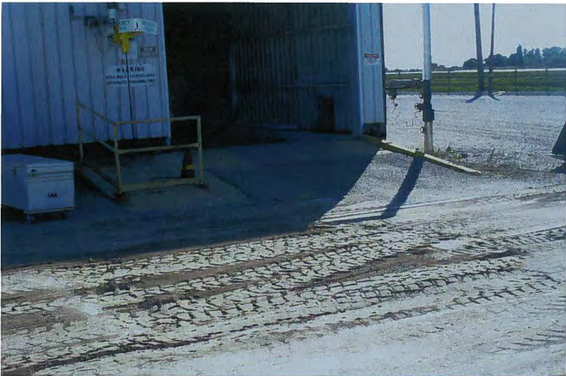
Photo # 12 Backfill of S0607 (boring B-51)
