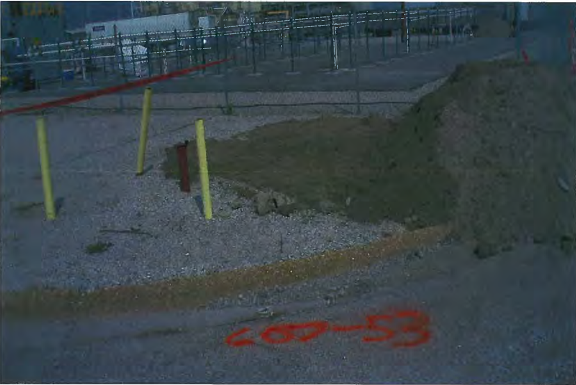
Photo # 14 Backfill of S0607 (boring B-53).
