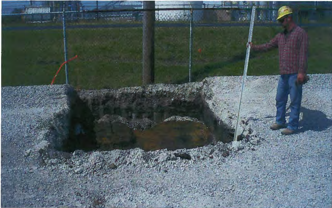
Photo # 15 S0607 excavation (boring B-65)
