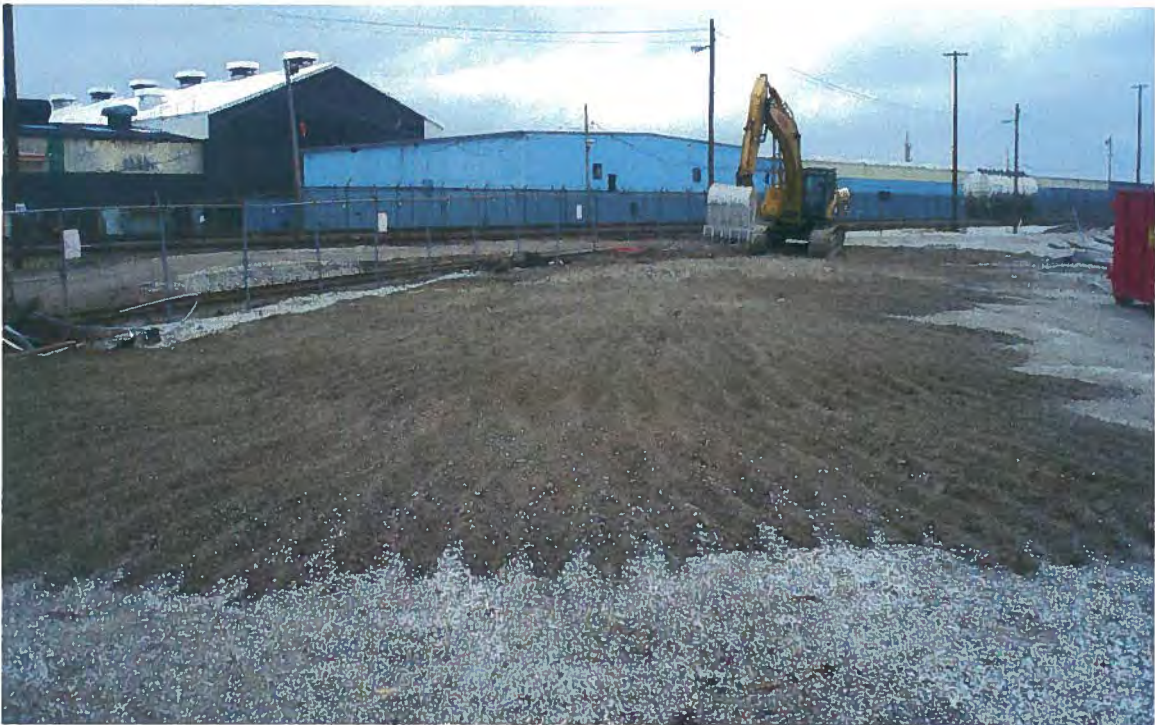
Photo # 52 Backfill of S0715 excavation (borings B-53/B-24/B-62).
