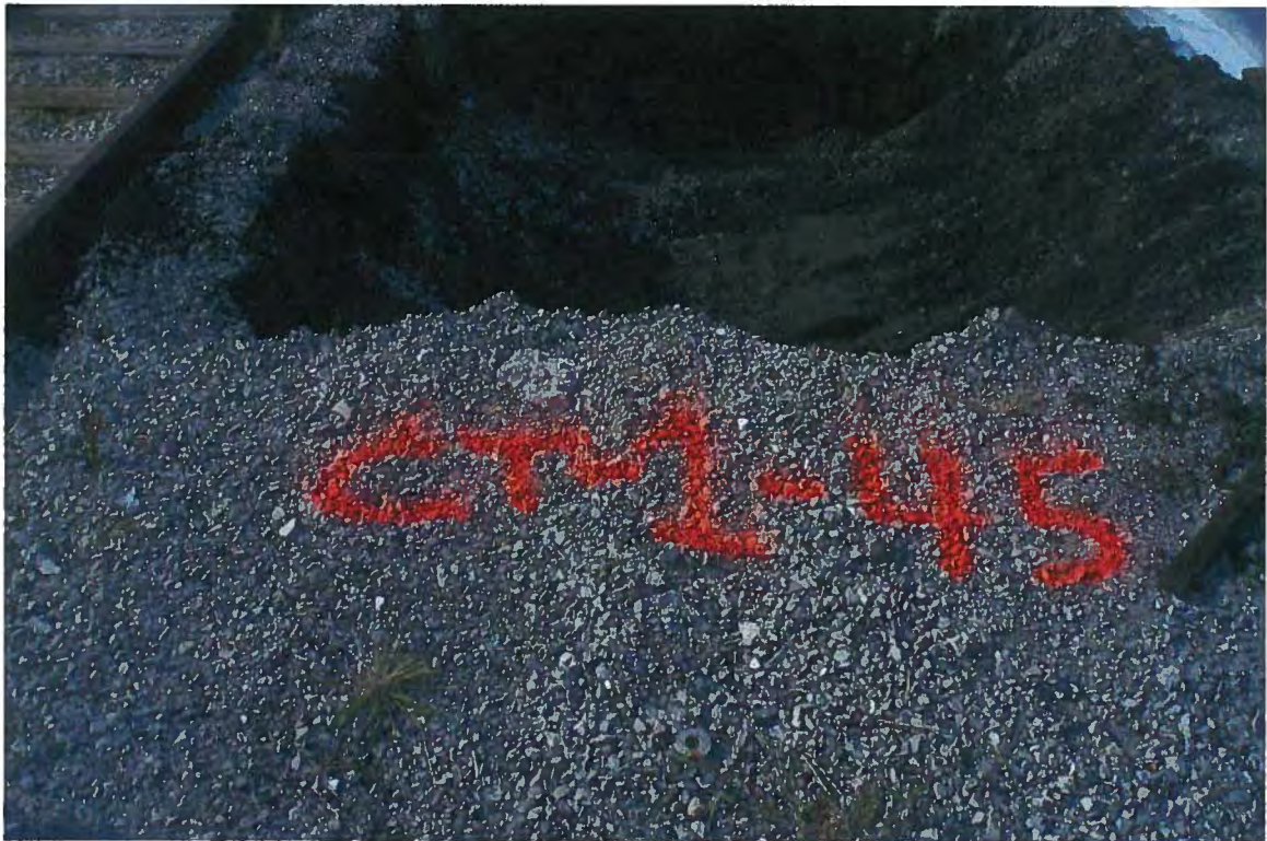
Photo # 26 S0608/CT-1 excavation (boring B-45).
