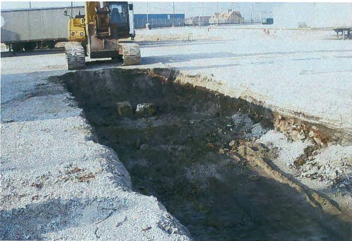
Photo # 22 S0608/CT-1 excavation (borings B-33/B-37).
