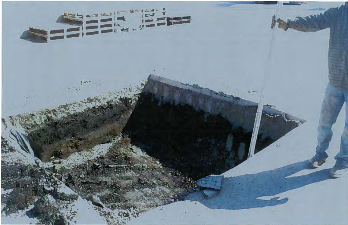
Photo # 11 S0607 excavation (boring B-51)
