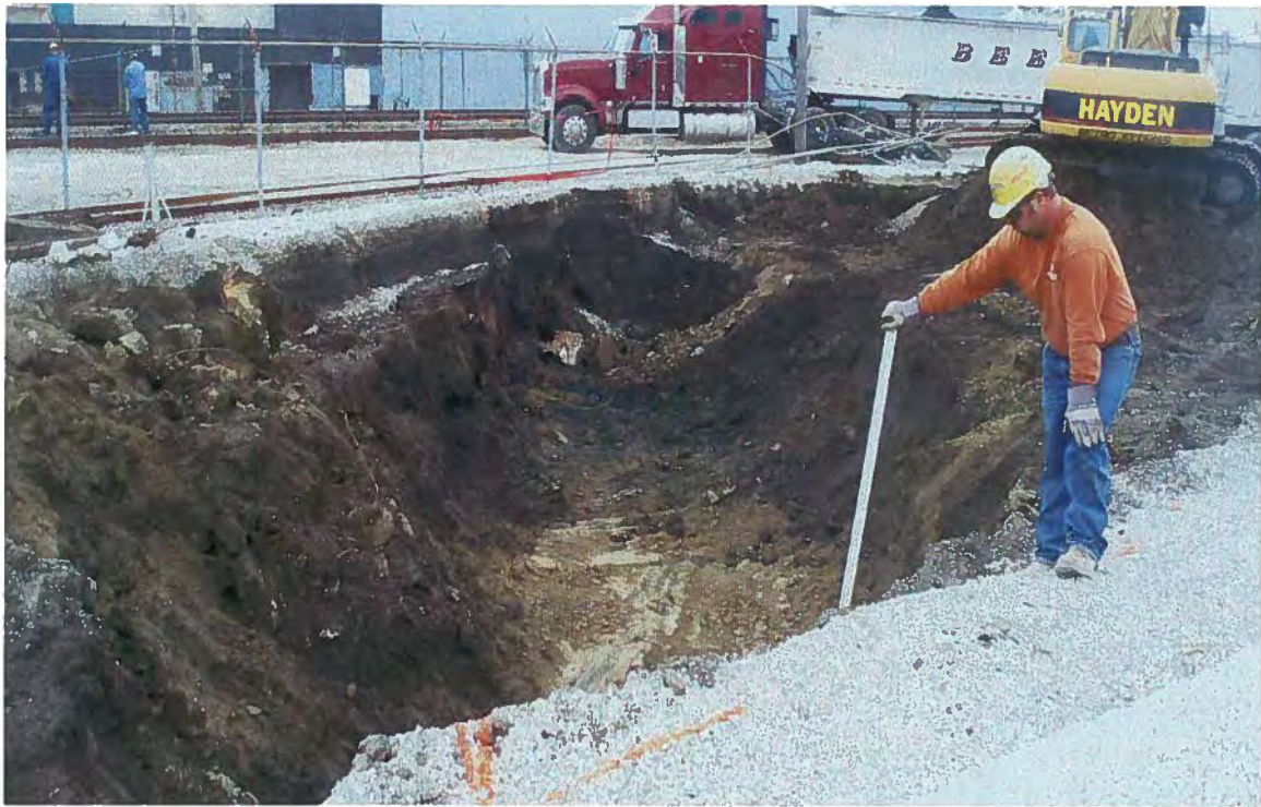
Photo # 51 S0715 excavation (10 ft deep excavation).
