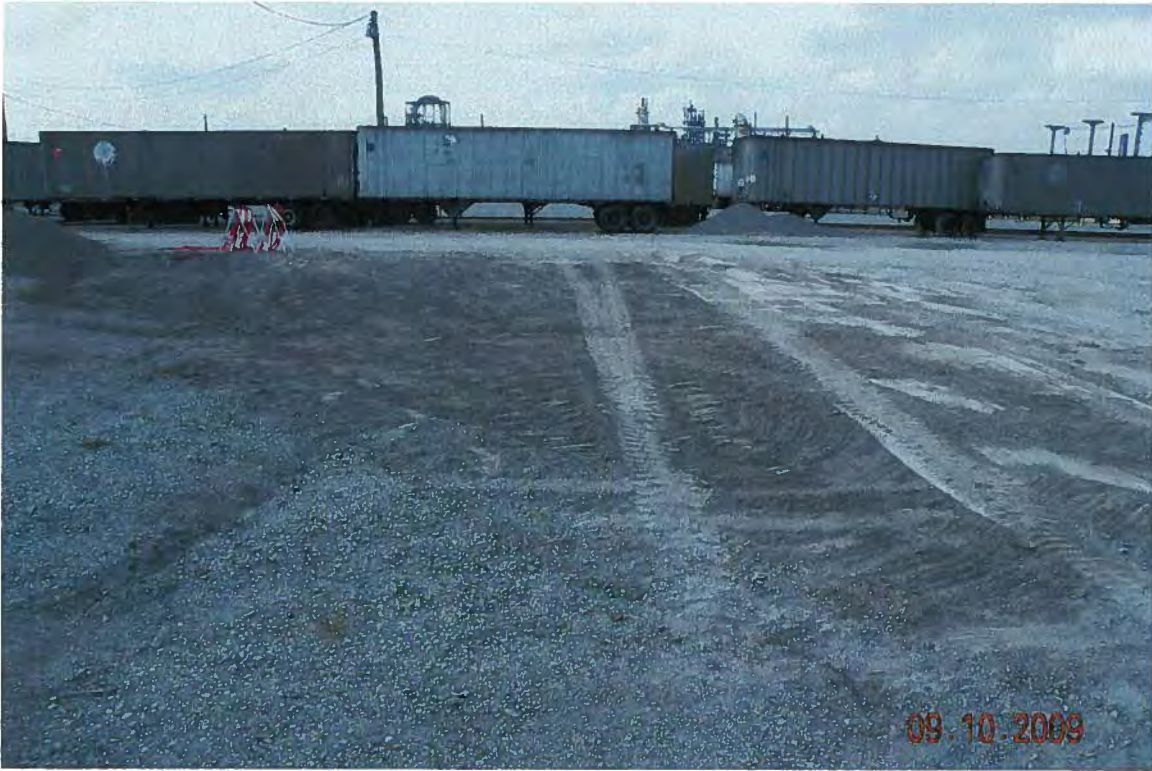
Photo # 23 Backfill of S0608/CT-1 (borings B-33/B-37).
