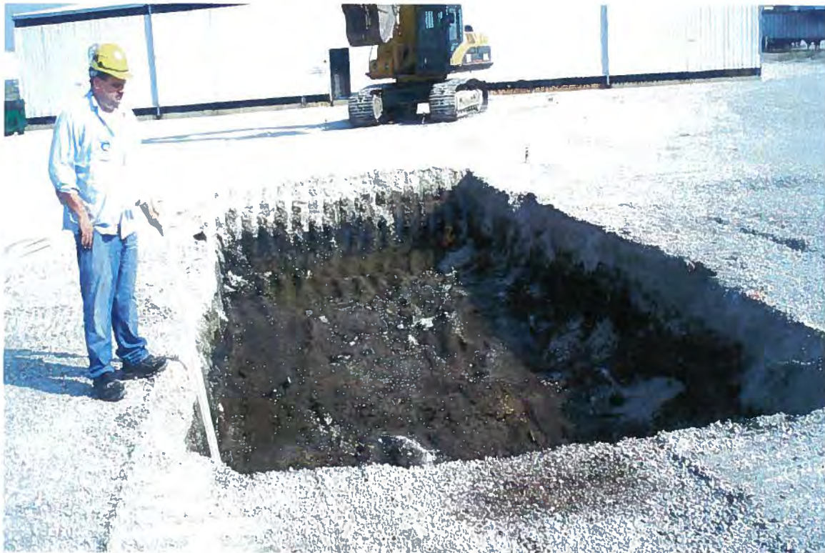
Photo # 33 S0609 excavation (borings B-32/B-40).
