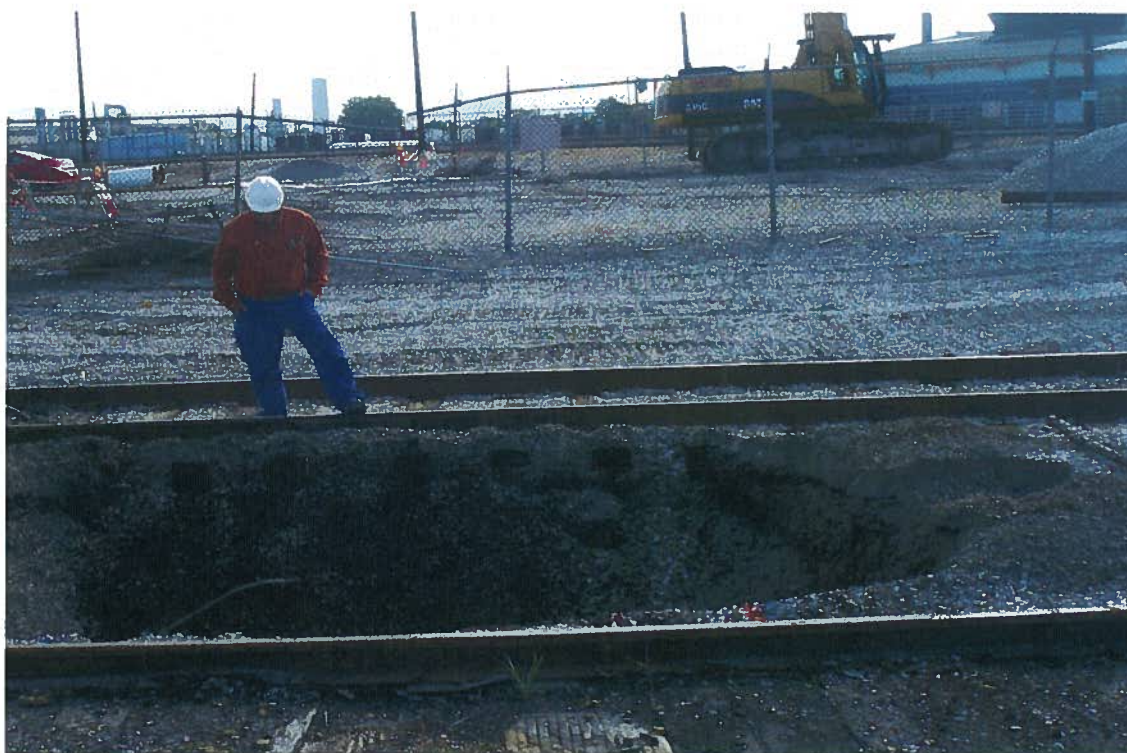
Photo # 46 S0715 excavation (boring B-47).
