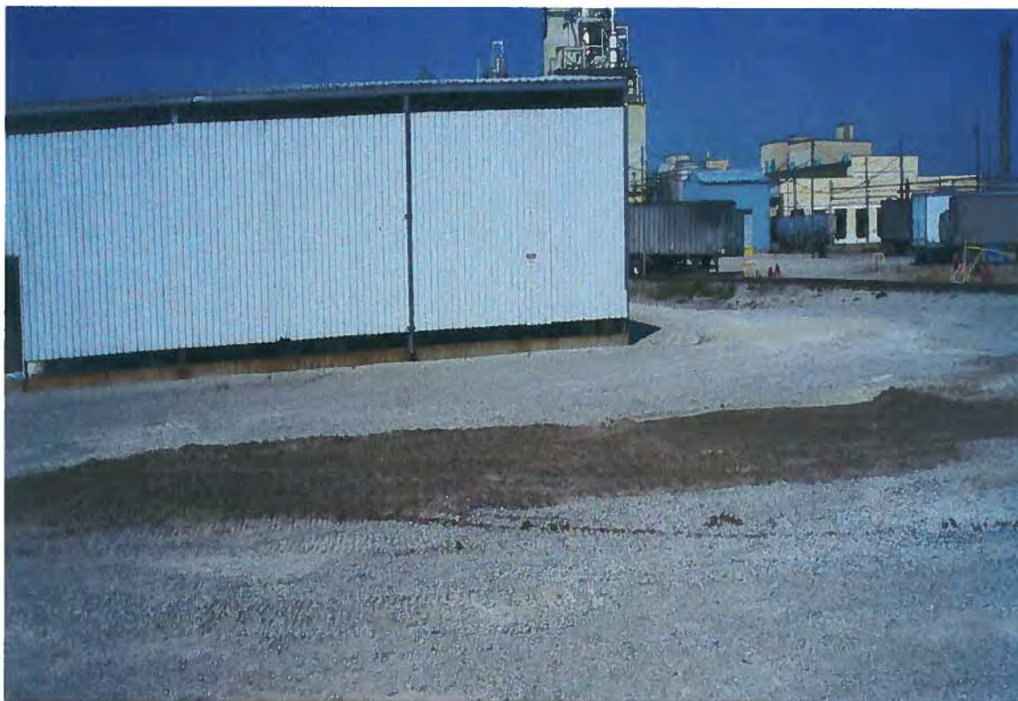
Photo #36 Backfill of S0609 (borings B-18/B-28/B-36/B-44)
