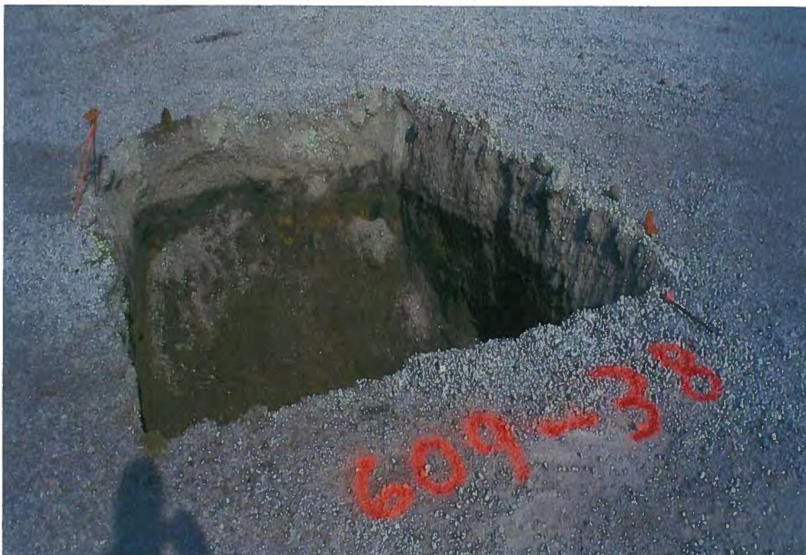
Photo # 37 S0609 excavation (boring B-38).
