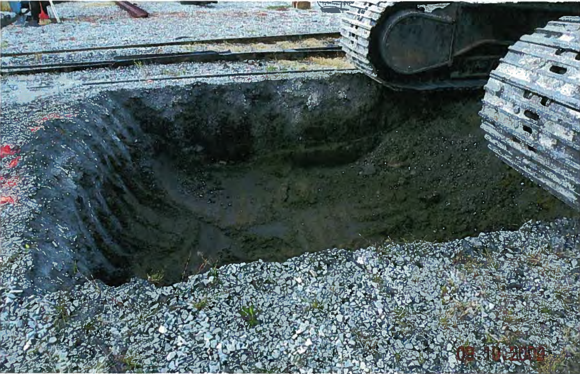
Photo # 24 S0608/CT-1 excavation (boring B-36).
