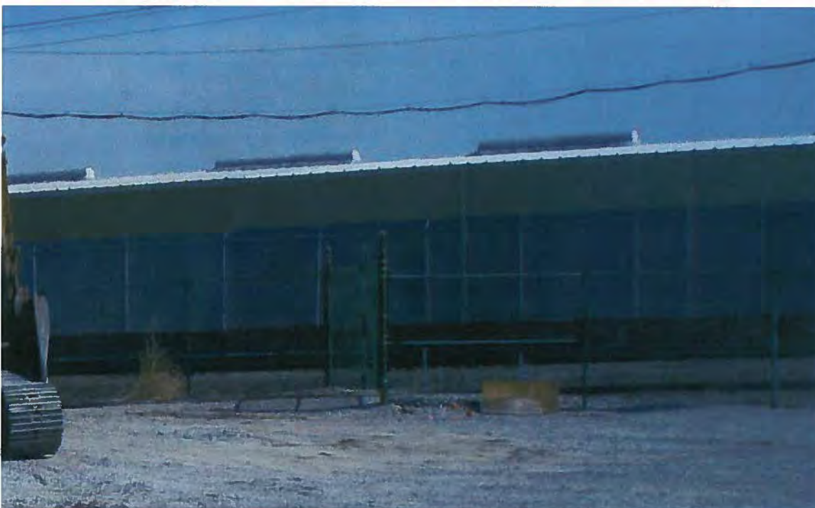
Photo # 38 Backfill of S0609 (boring B-38).
