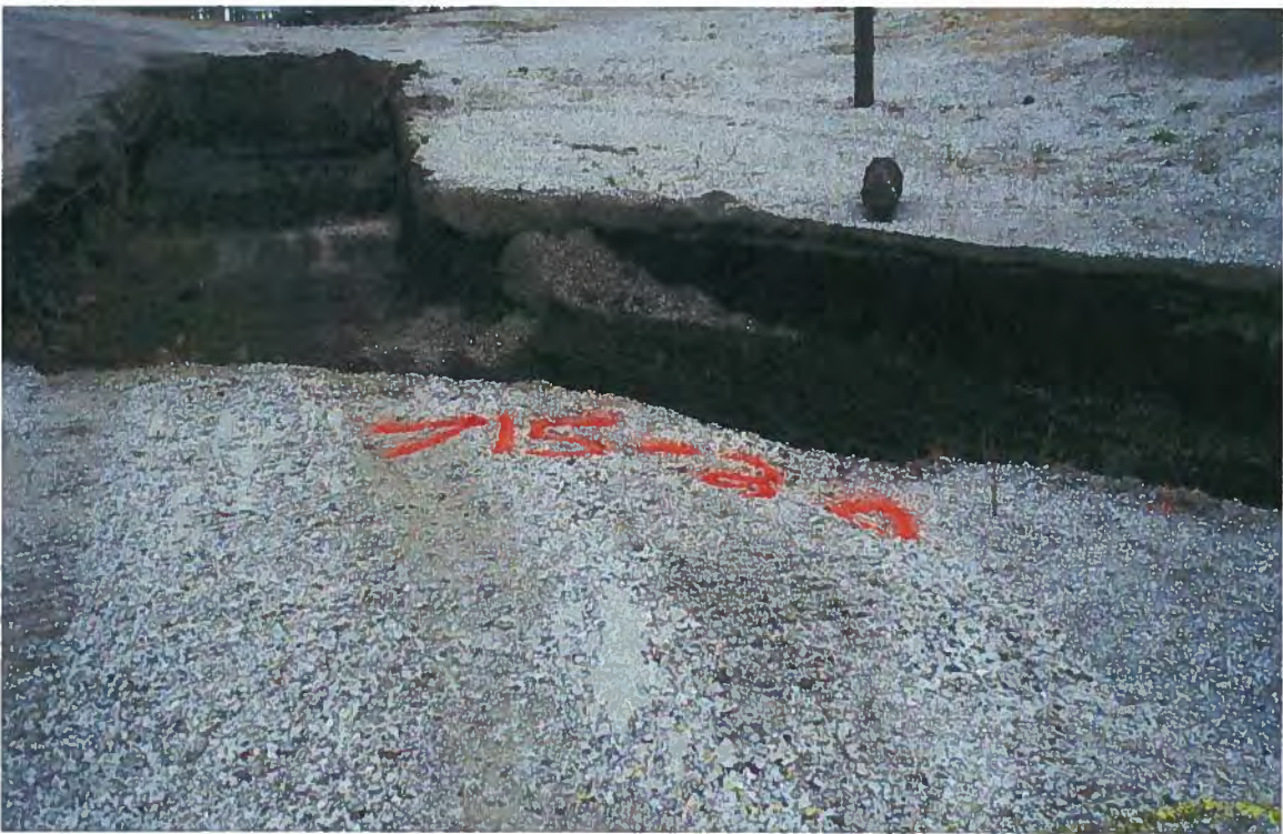
Photo # 48 S0715 excavation (borings B-9/B-20/B-25/B-66).
