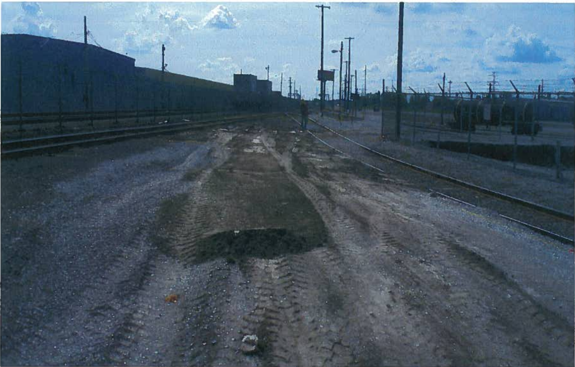
Photo # 50 Backfill of S0715 (borings B-21/B-28/B-36/B-67).
