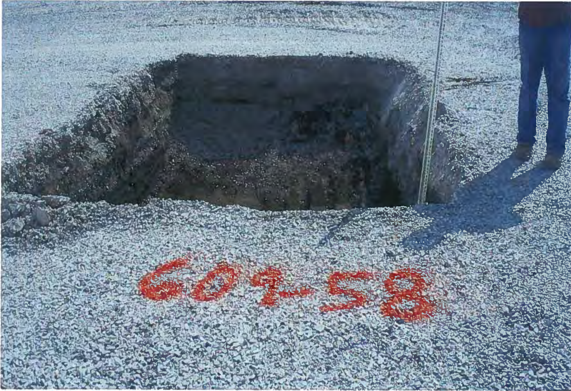
Photo # 39 S0609 excavation (boring B-58).
