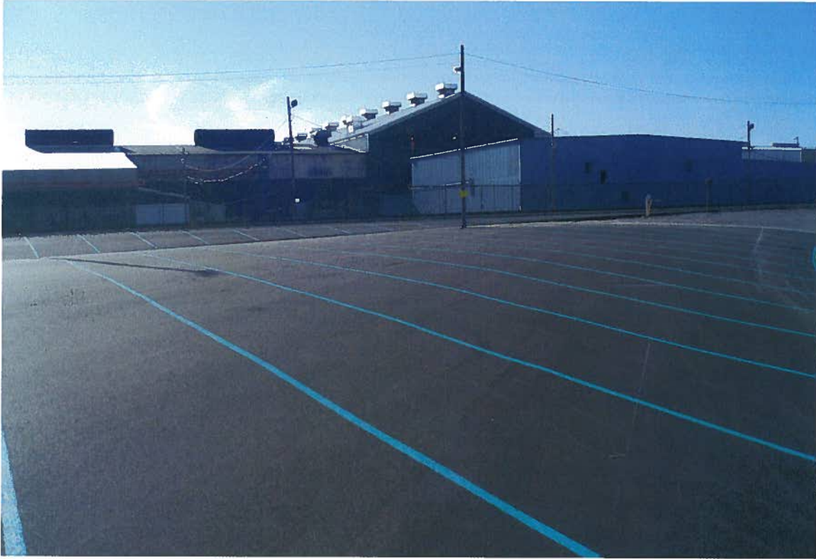
Photo # 53 S0715 area following paving activities.
