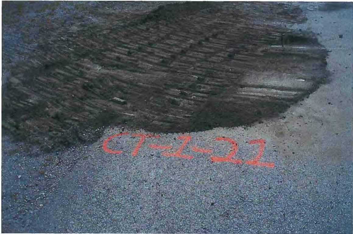
Photo # 18 Backfill of S0608/CT-1 (boring CT-1-21).
