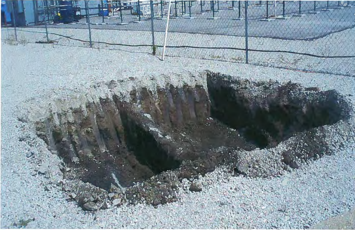
Photo # 13 S0607 excavation (boring B-53).
