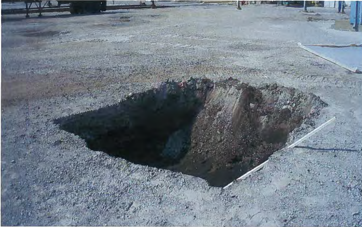
Photo # 19 S0608/CT-1 excavation (boring S0608-B-21).
