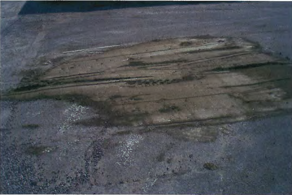
Photo # 10 Backfill of S0607 excavation (boring B-49)
