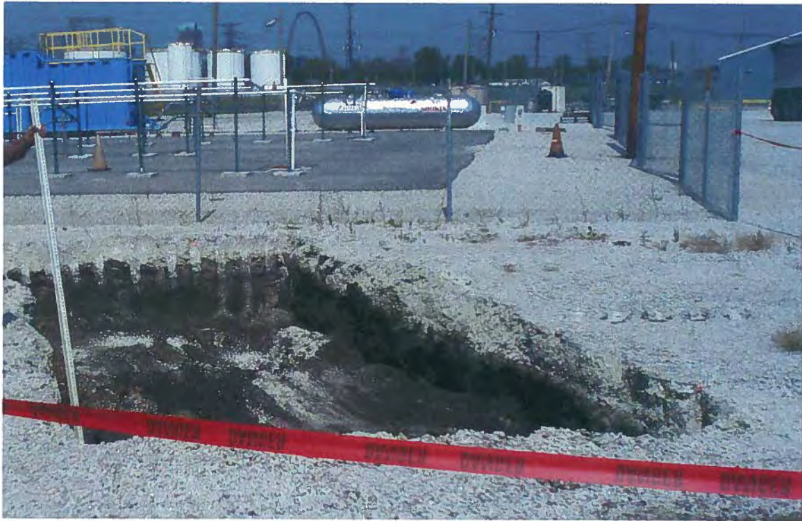
Photo # 5 S0607 excavation (borings B-26/B-34)
