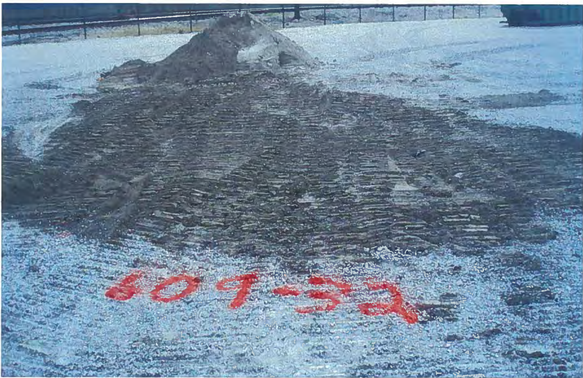
Photo # 34 Backfill of S0609 (borings B-32/B-40)
