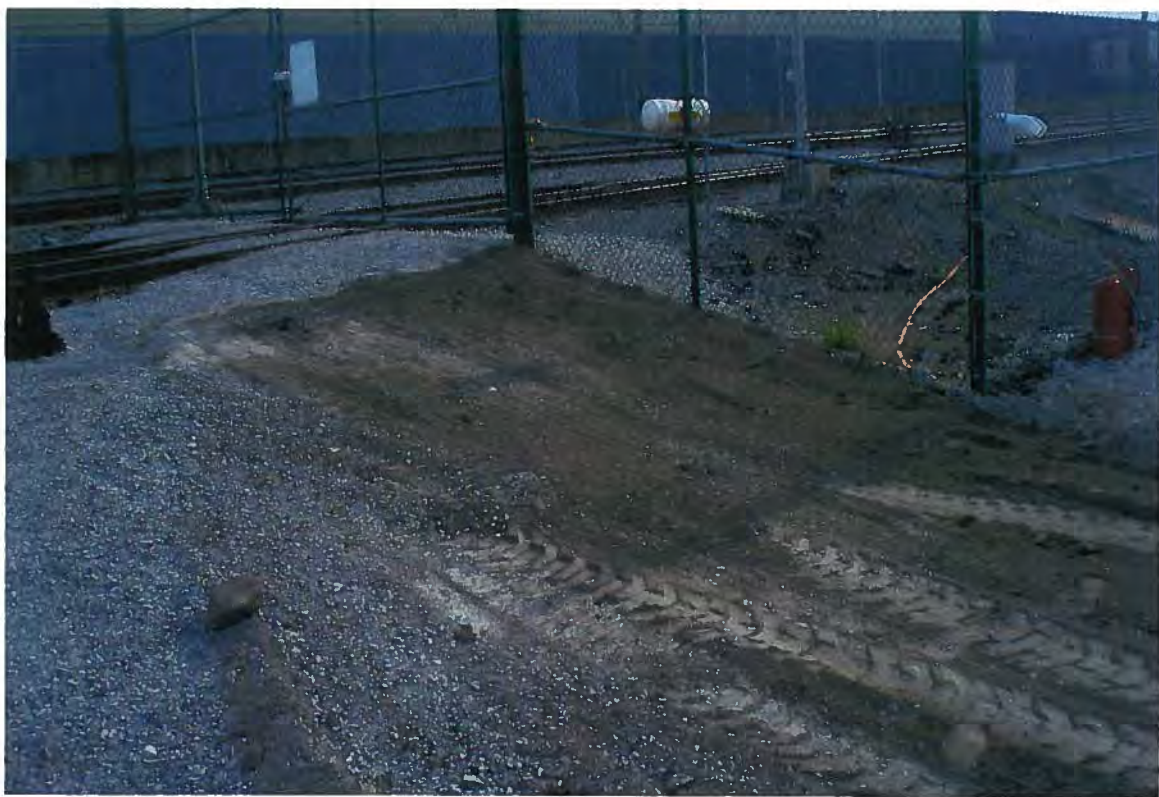
Photo # 32 Backfill of S0609 (boring B-115).
