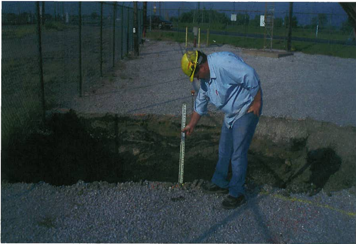
Photo # 41 S0609 excavation (boring B-86).
