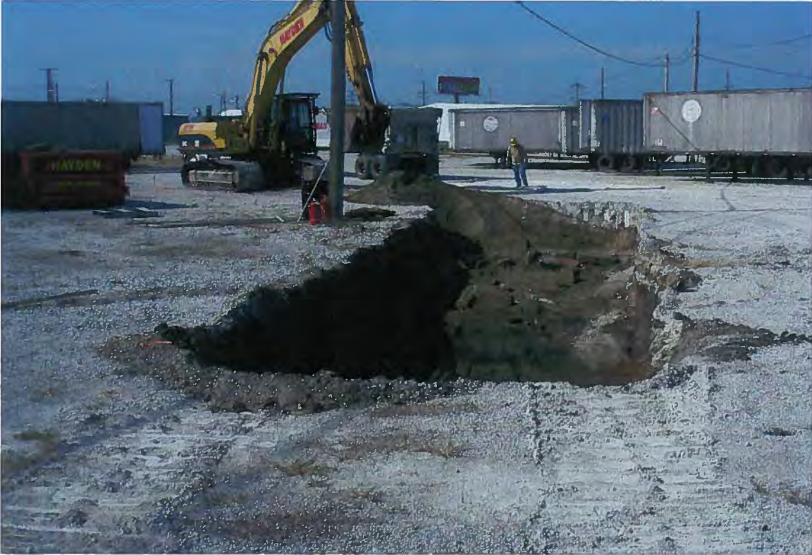
Photo # 20 S0608/CT-1 excavation (borings B-19/B-33).
