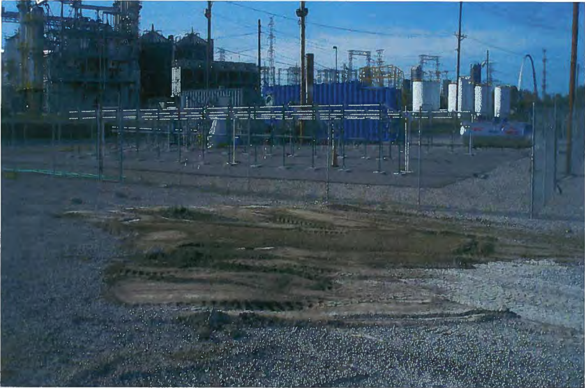
Photo # 6 Backfill of S0607 excavation (borings B-26/B-34)
