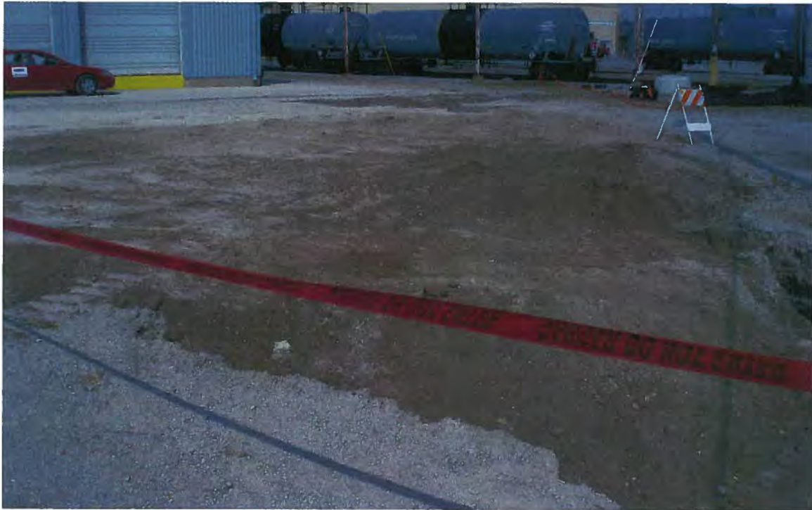
Photo # 21 Backfill of S0608/CT-1 (borings S0608-B-21 and B-19/B-33).
