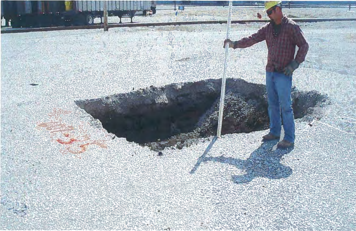
Photo # 7 S0607 excavation (boring B-35)
