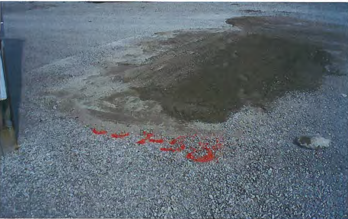
Photo # 40 Backfill of S0609 (boring B-58).
