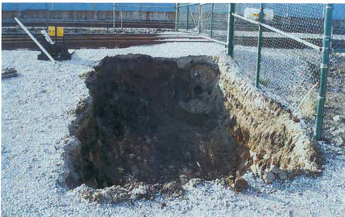
Photo # 31 S0609 excavation (boring B-115).
