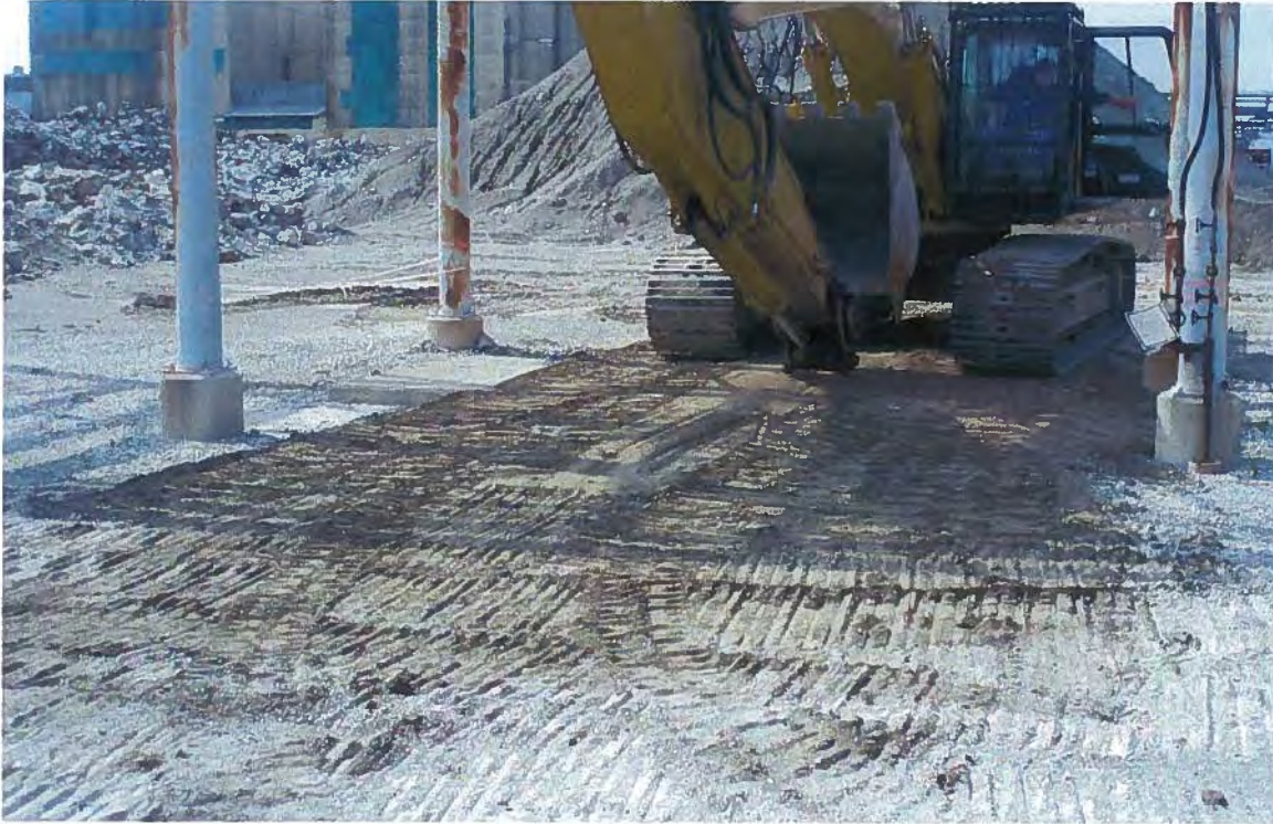
Photo # 3 Backfill of Former PCB Warehouse excavation.
