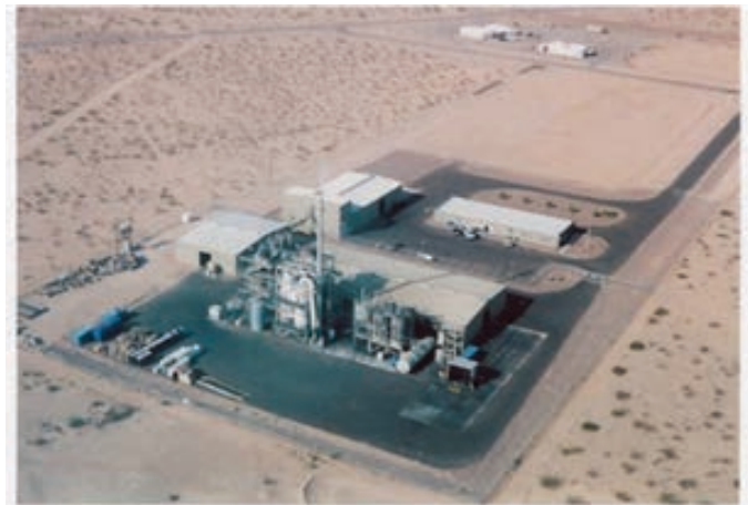
Evoqua Facility in Parker, AZ
