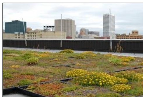
Figure 29: Lightweight and easy-to-maintain green roofs can be added to existing roofs.
