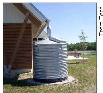
Figure 27: Cisterns can capture runoff from roofs and store it to be used for irrigation or other nonpotable uses
