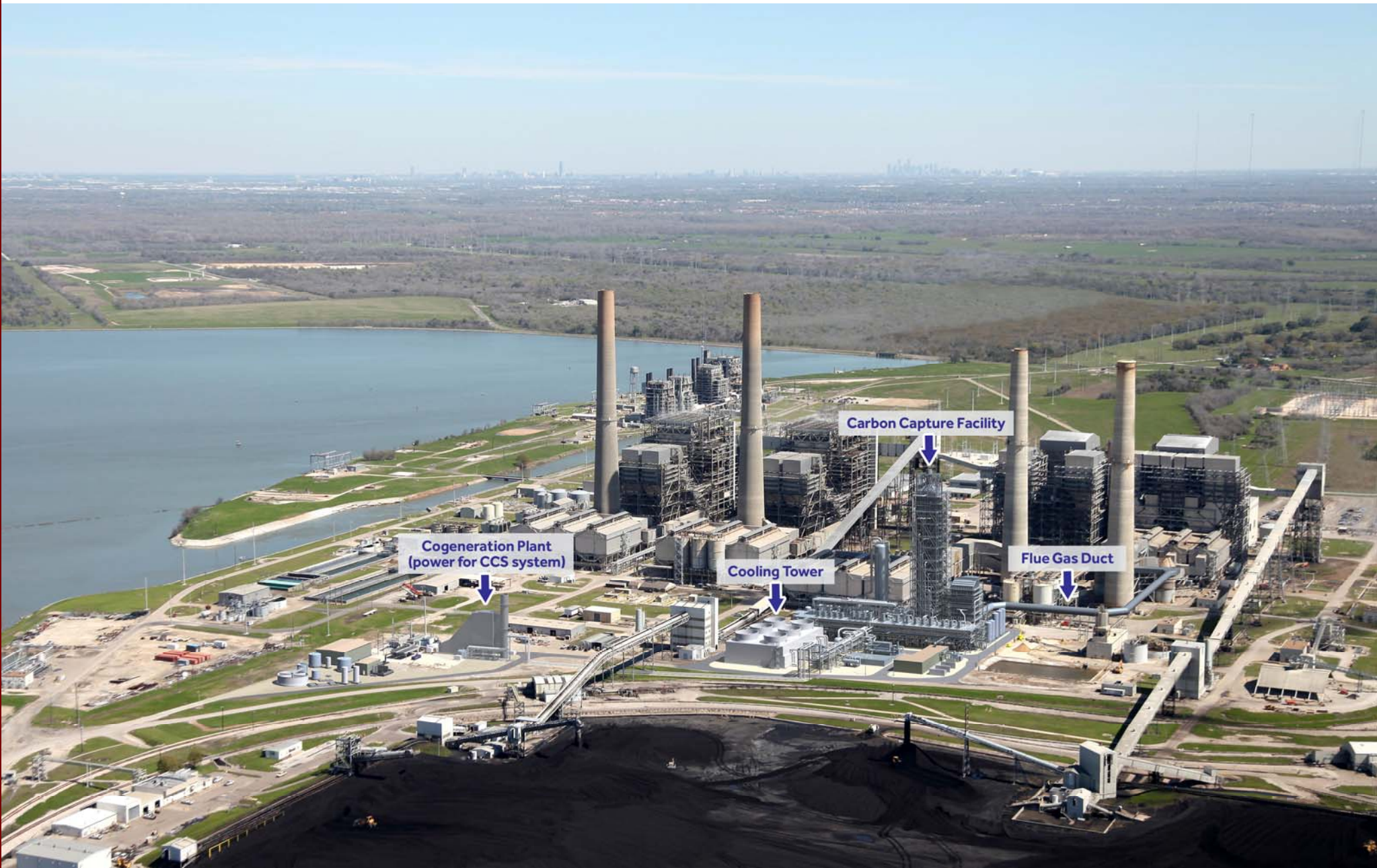
W.A. Parish Power Plant in Thompsons TX Proposed Carbon Capture Facility and Cogeneration Plant for the Carbon Capture System
