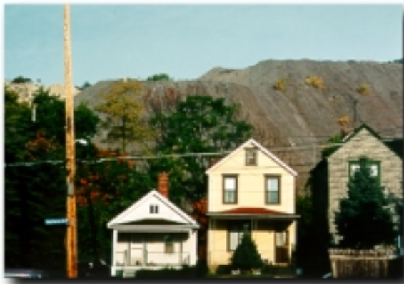
Slag Piles Tower Over Nearby Houses at the Nine Mile Run Site
