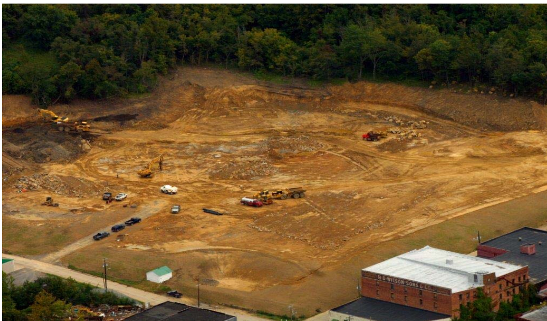
Site before construction
