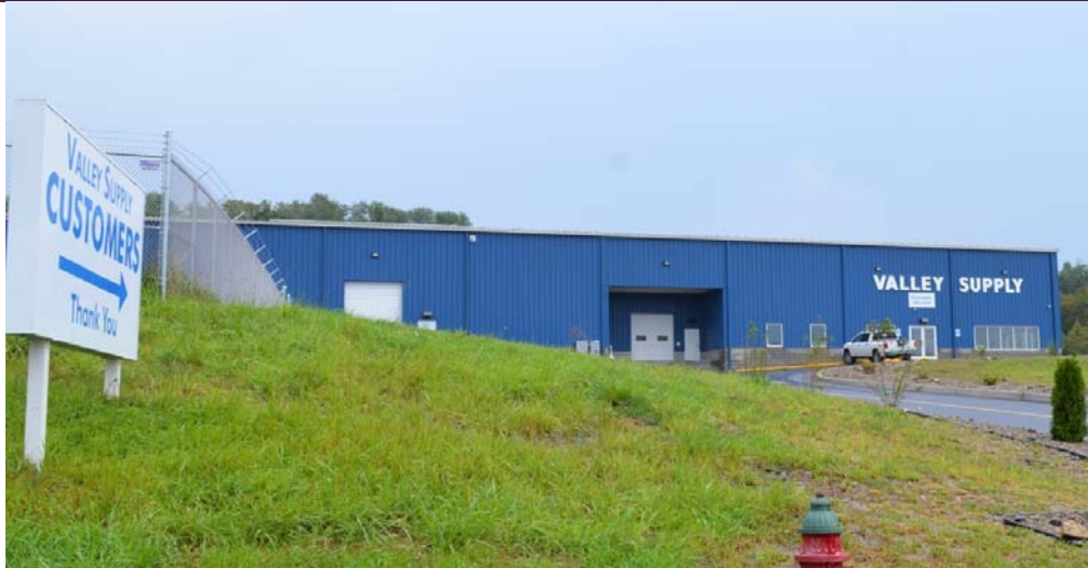
Site after construction
