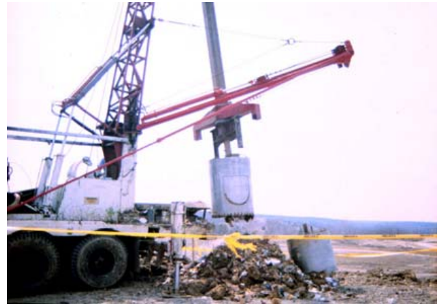
Figure C-10. LFG Well Drilling.
