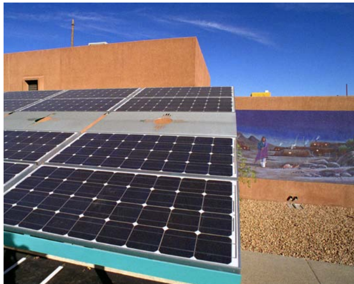
At the Indian Pueblo Cultural Center in Albuquerque, New Mexico, this photovoltaic carport delivers about 23 megawatt-hours of clean electricity to the local utility grid. Photo from Sandia National Laboratories, NREL/PIX 08978
