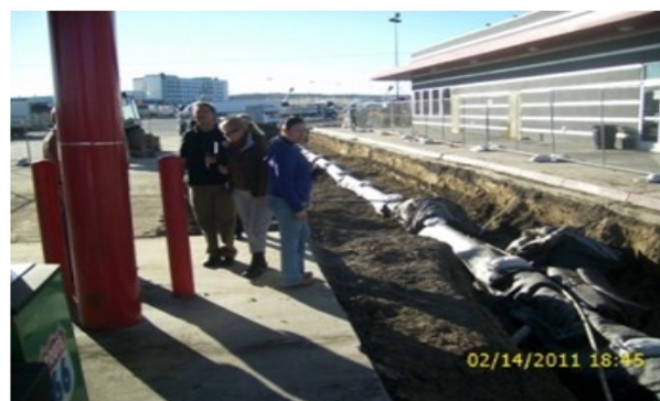
Trench where contaminated soil and free product were removed.
