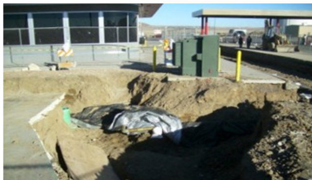
Tank pit where 2000 gallons of diesel had been released in about 15 minutes and flowed along the piping to the dispenser islands.
